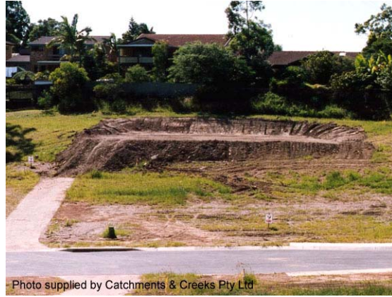
Photo 2 – Cut and fill building sites result in significant soil disturbance
