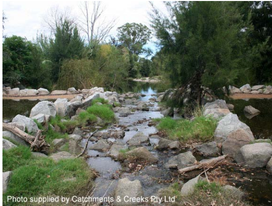
Photo 1 – Rock-lined fish ramp
