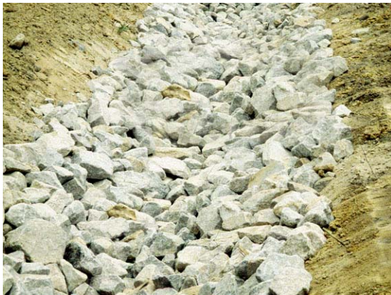
Photo 21 – Placement of the rock on the soil can result in erosion problems if significant lateral inflows occur
