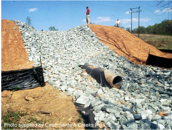
Photo 19 – Rock-lined spillway with well-defined crest profile
