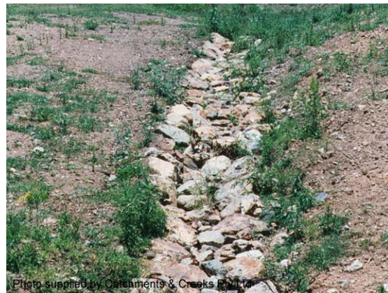
Photo 18 – Permanent, rock-lined batter chute
