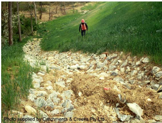
Photo 17 – Permanent, rock-lined batter chute
