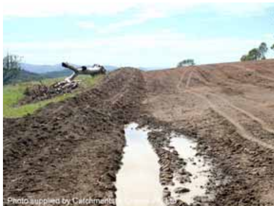
Photo 8 – Flow diversion bank down-slope of a future pipeline installation
