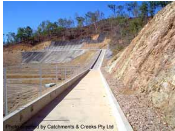
Photo 2 – Permanent diversion channel collecting stormwater runoff up-slope of a subdivision
