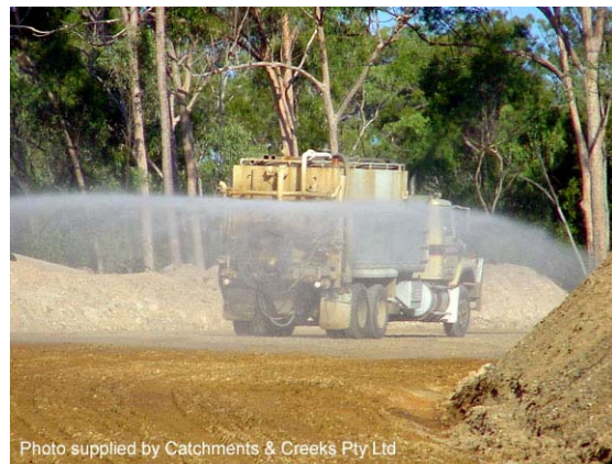
Photo 2 – Dust control using a water truck
