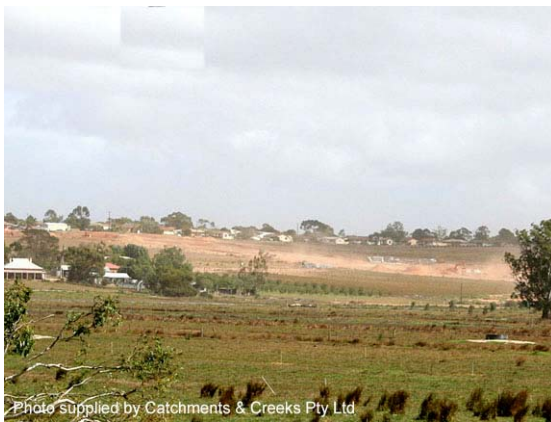
Photo 1 – Dust generation on a construction site
