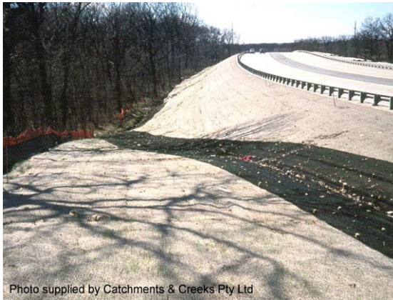
Photo 1 – Application of erosion control blankets and mats
