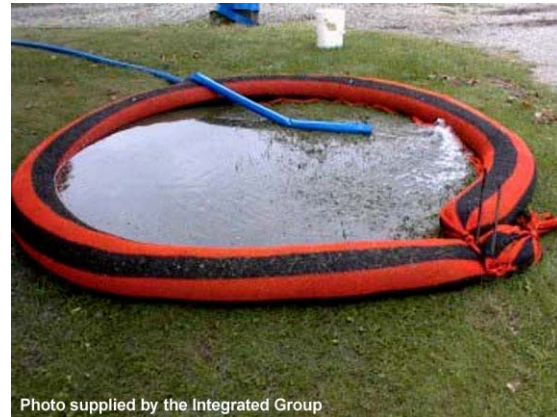
Photo 2 – Compost-filled sock used to form a filter pond
