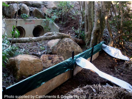
Photo 4 – Example of plywood used to form a sealed dam
