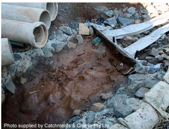
Photo 5 – Filter tube outlet structure within a confined channel
