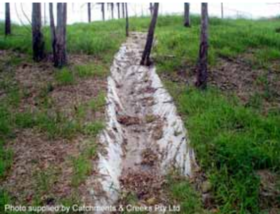
Photo 1 – Temporary chute lined with filter cloth
