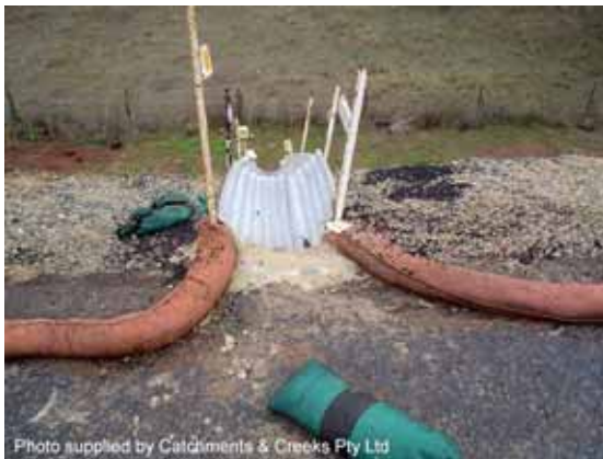
Photo 1 – Batter chute formed from corrugated sheet iron
