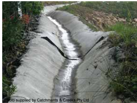
Photo 2 – Concrete lined catch drain
