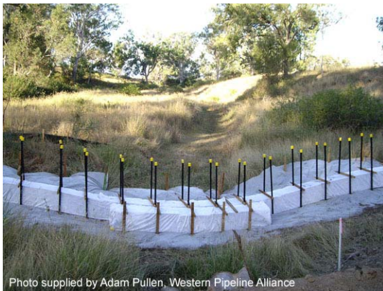
Photo 1 – Modular sediment trap
