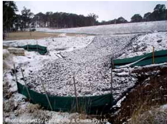
Photo 2 – Temporary rock mattress outlet structure at end of a Chute
