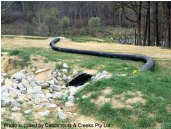
Photo 1 – Temporary Slope Drain with rock stabilisation at inlet and outlet
