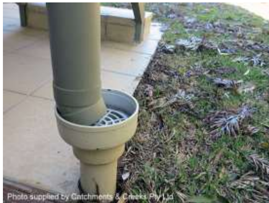
Downpipe 'connected' to the street
