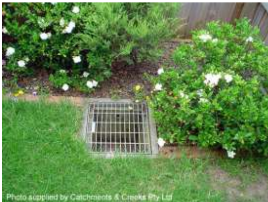
Grated stormwater inlet
