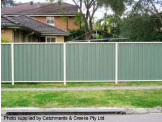
Raised fencing over an overland flow path
