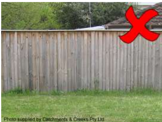
Solid fence blocking overland flows
