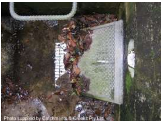
Outlet screen inside a detention tank
