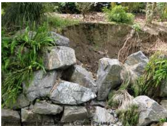
Failure of rock retaining wall
