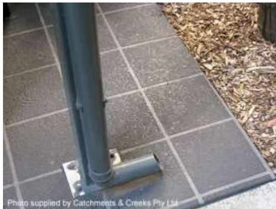
Free discharge of roof water drainage
