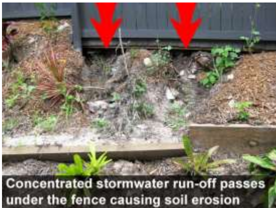
Stormwater erosion under a fence
