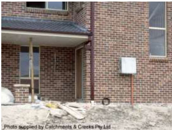
Roof water drainage on a new building
