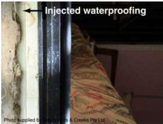
Injection of waterproofing sealer
