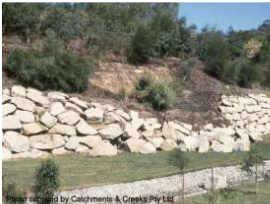
Failed rock retaining wall (landslip)
