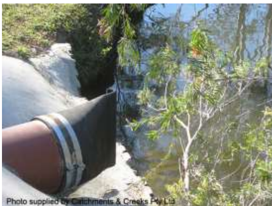
Rubber 'duckbill' backflow control
