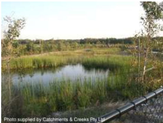
Stormwater treatment wetland
