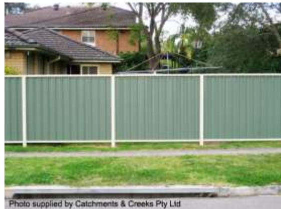
Elevated metal panel fencing
