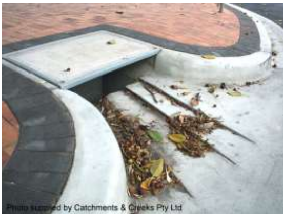
Roadside stormwater inlet
