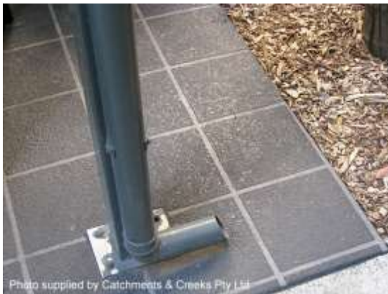
Discharge onto a garden bed
