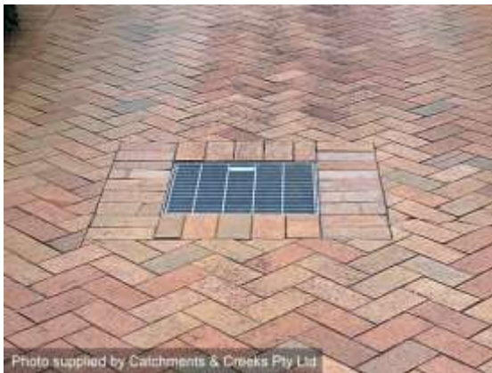
Stormwater inlet for minor storm flows
