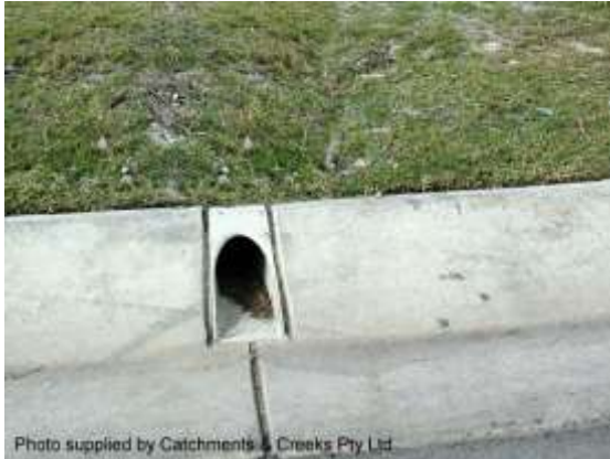
Stormwater 'kerb' outlet to a roadway
