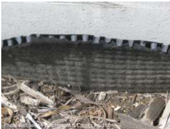
Drainage 'blanket' placed against a wall
