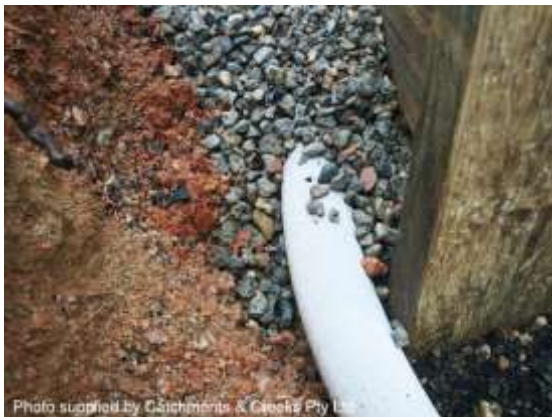
Subsoil drainage behind a retaining wall
