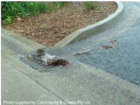
Roadside stormwater inlet
