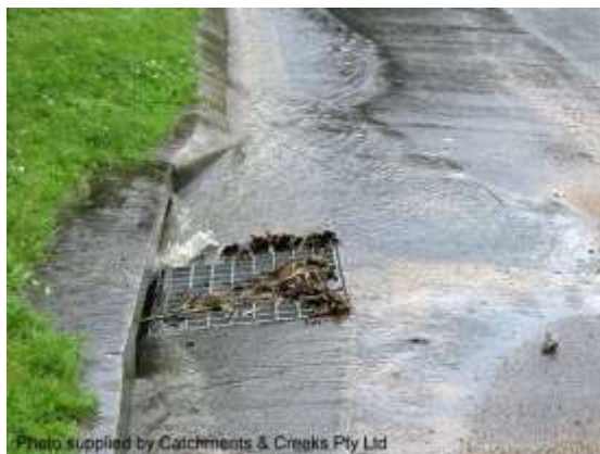
Roadside stormwater (kerb) inlet
