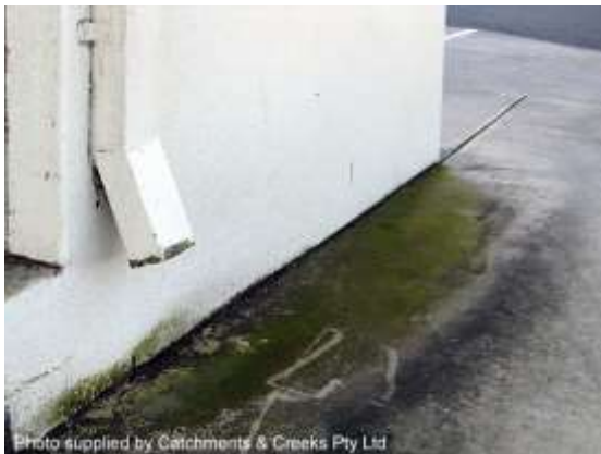
Old roof water downpipe
