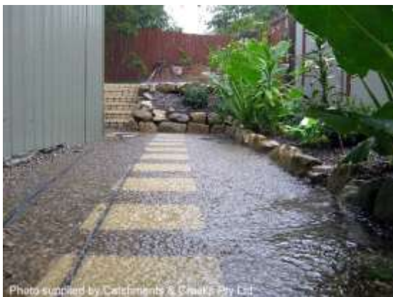
Recessed pathway carrying overland flow
