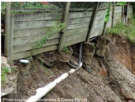
Landslip caused by stormwater discharges
