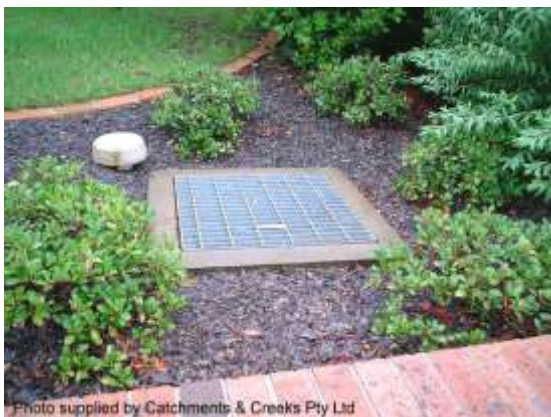
Residential stormwater 'field' inlet
