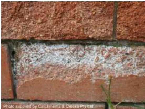
Salt damage from rising groundwater
