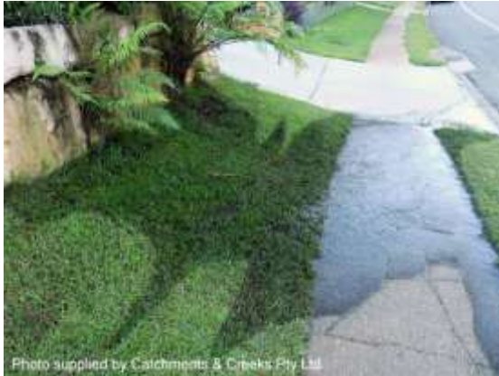
Seepage from a boulder wall
