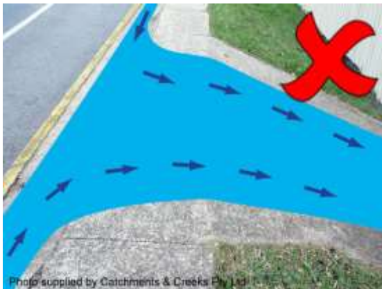
Driveway lowered which allows inflow
