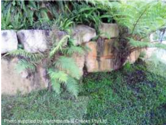
Groundwater seepage from a stone wall
