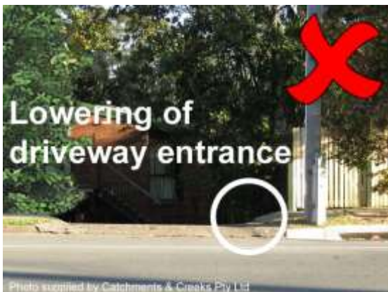
Driveway lowered below the footpath level
