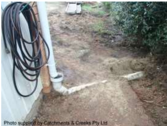
Installation of roof water drainage system
