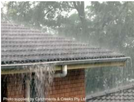
Overflowing roof gutter
