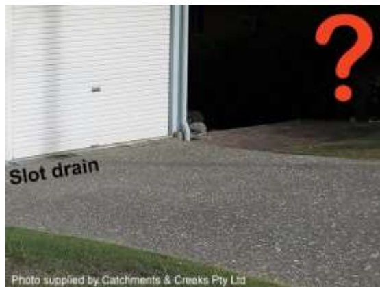
Slot drain located too close to the garage
