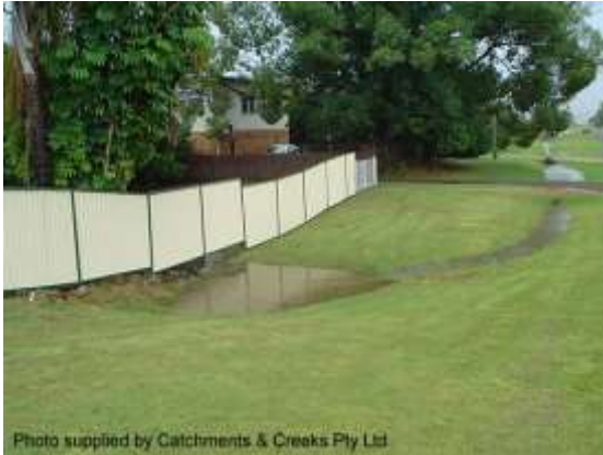
Stormwater inflow into a property
