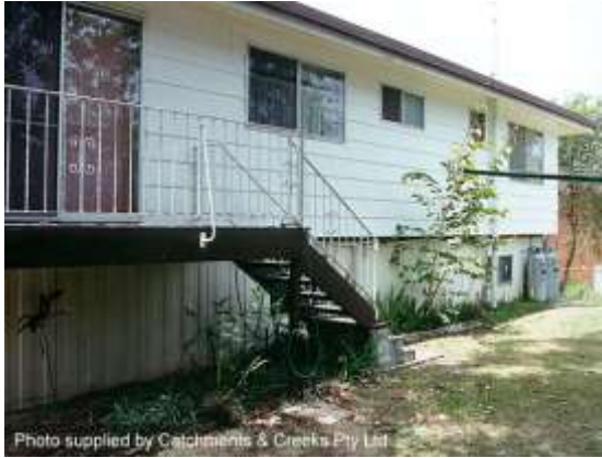
Earth fill placed against lower walls
