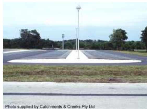
Gravel infiltration trench
