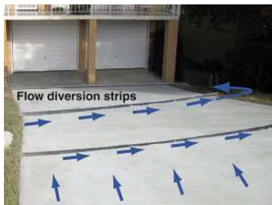
Flow diversion strips set in a driveway
