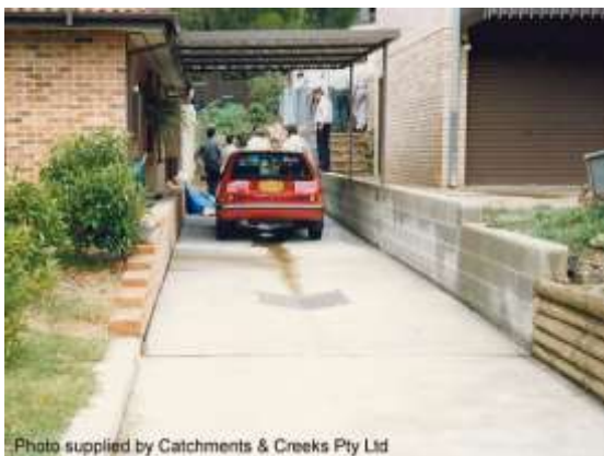
Recessed driveway & overland flow path
