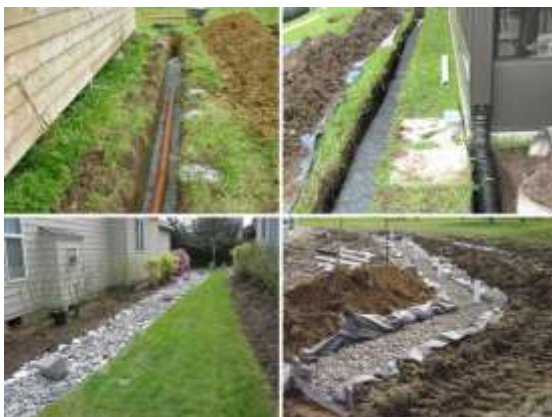
Soakage drains under construction
