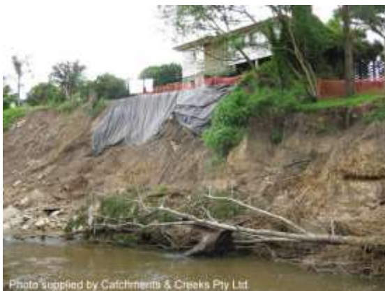
Creek bank failure (flood damage)
