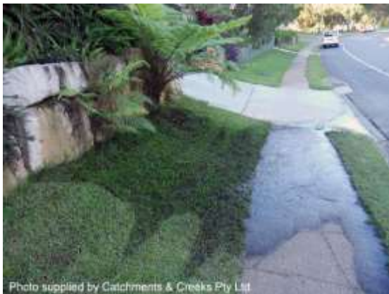
Groundwater seepage from a retaining wall
