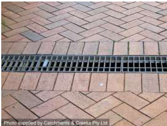
Slot drain with metal grate
