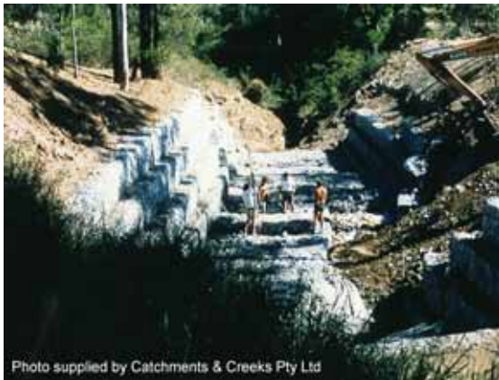
Photo 3 – Rock gabion and mattress channel stabilisation (during construction)
