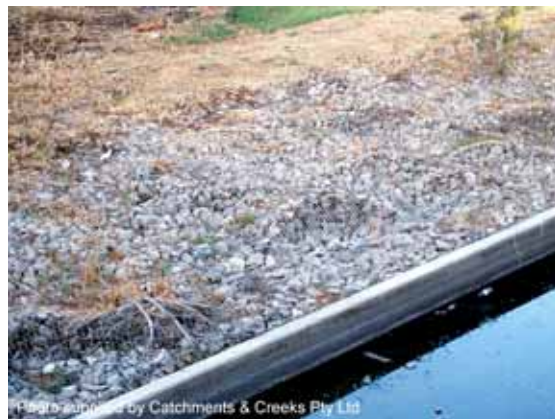
Photo 6 – Displacement of the rock can occur in areas of high shear stress (such a condition does not necessarily represent a structural failure)
