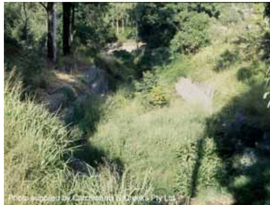
Photo 4 – Gabion structure during vegetation establishment phase – note; vegetation density can become excessive unless appropriate species are selected
