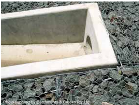
Photo 5 – Anchorage of gabions and rock mattresses to fixed objects using I-bolts set into the concrete and galvanised tie rods
