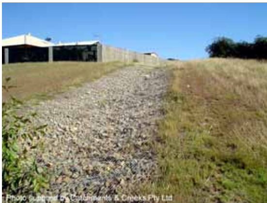
Photo 1 – Rock mattress-lined drainage chute
