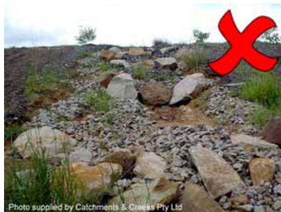
Photo 8 – Placement of a few large, anchor rocks down a steep slope will not help stabilise adjacent, under-sized rocks, and will likely cause flow diversion
