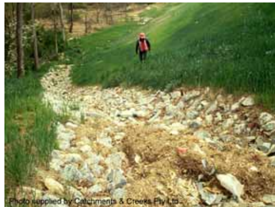
Photo 2 – Permanent, rock-lined batter chute
