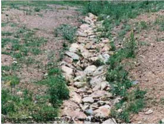
Photo 3 – An example of the rock-lining being correctly recessed into the topography
