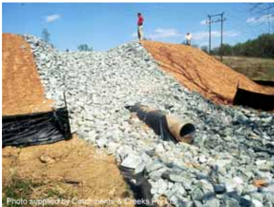
Photo 1 – Rock-lined emergency spillway of a sediment basin
