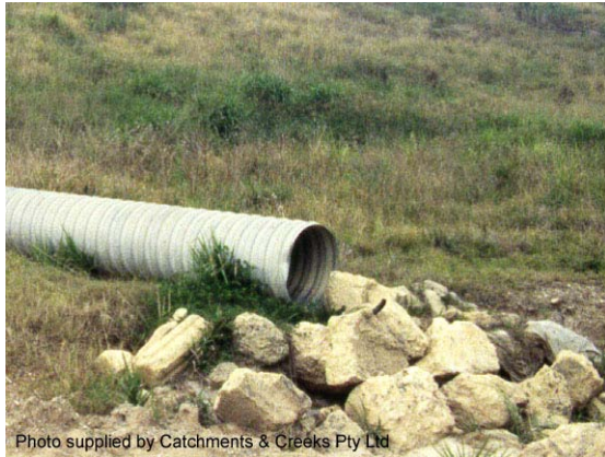
Photo 1 – Slope drain with rock-lined outlet structure
