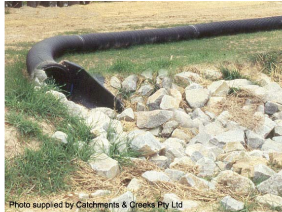
Photo 2 – Flexible-pipe slope drain with rock-lined outlet structure
