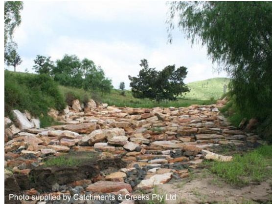
Photo 2 – Rock-lined gully chute
