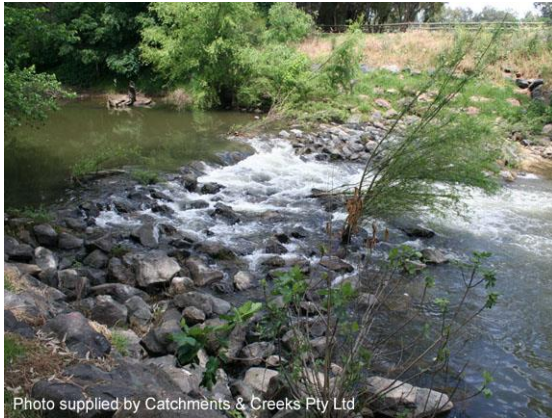
Photo 1 – Rock-lined waterway chute
