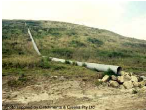
Photo 2 – Corrugated, steel pipe slope drain
