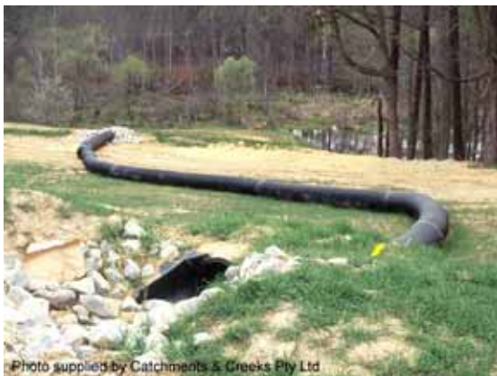
Photo 7 – Pipe directing flow to a sediment basin
