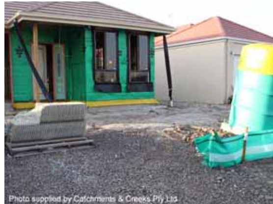
Photo 2 – Temporary downpipe
