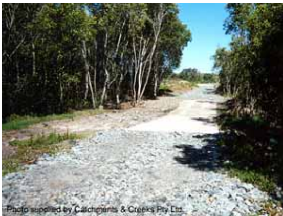
Photo 5 – Stabilised ford crossing of tidal backwater
