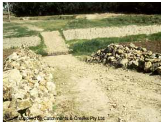
Photo 6 – Ford crossing of newly constructed stormwater drain
