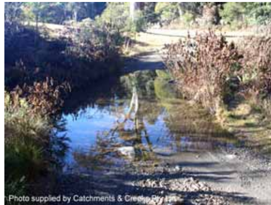
Photo 2 – Ford crossing of alluvial (gravel) stream
