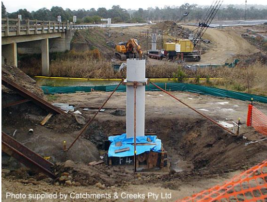
Bridge pier construction (NSW)
