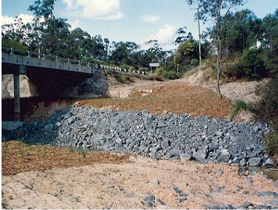
Rock placement upstream of a bridge
