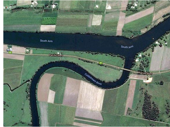
Pacific Highway, Coldstream River
