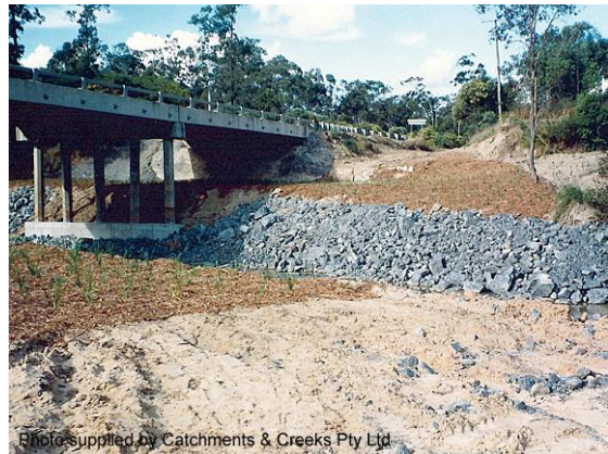
Rock placement on creek banks (1992)
