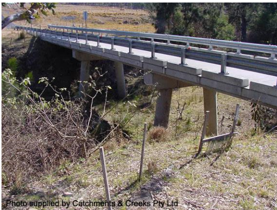
Bridge with minimal constriction (NSW)
