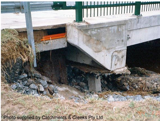
Flood damage to bridge abutment (Qld)
