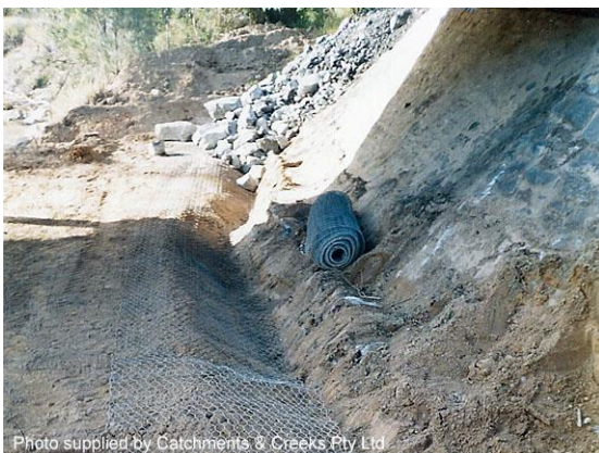
Trenching of rockfall netting, 1992
