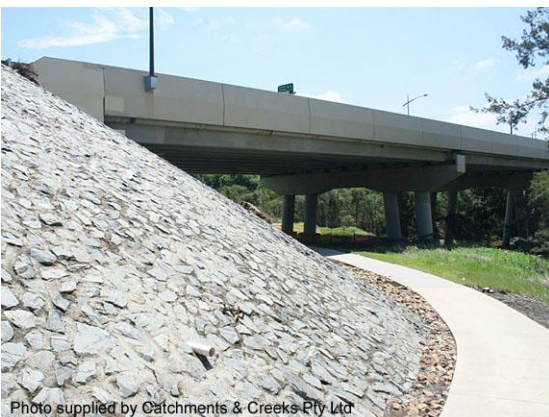
Grouted stone pitched abutment (Qld)
