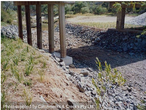
Rock placement on creek bed (1992)
