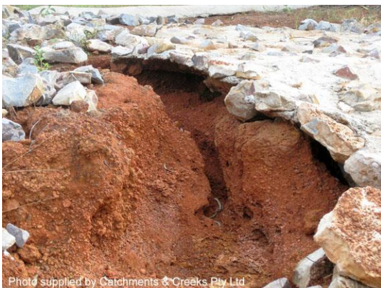
Failed stone pitching (NT)
