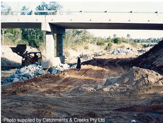
Overbank floodway stabilisation, 1992
