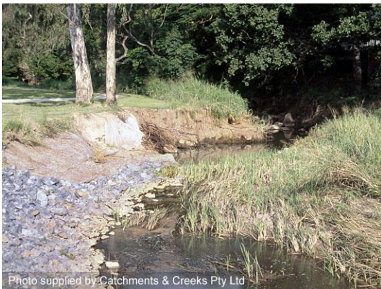
Bank erosion d/s of rock-stabilised bank
