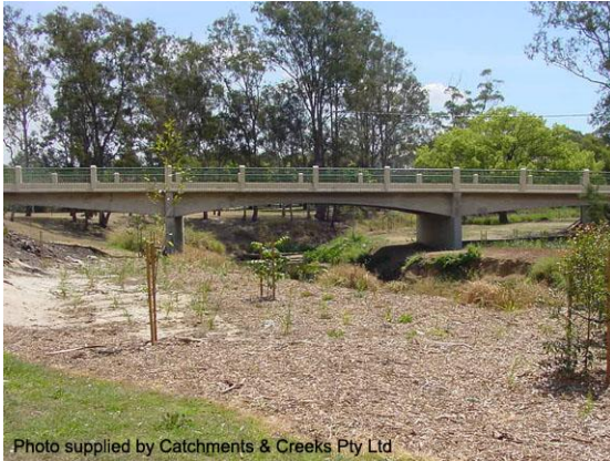
Bridge with no in-stream piers (Qld)
