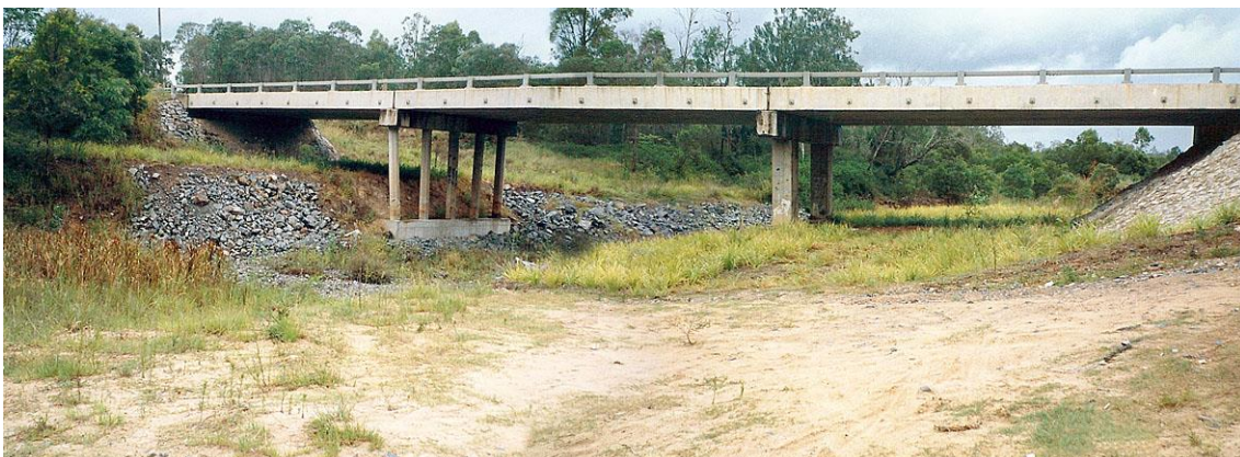
Finished bridge scour works, January 1994
