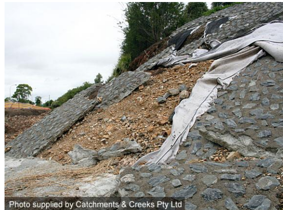
Same bridge post flood (2011)
