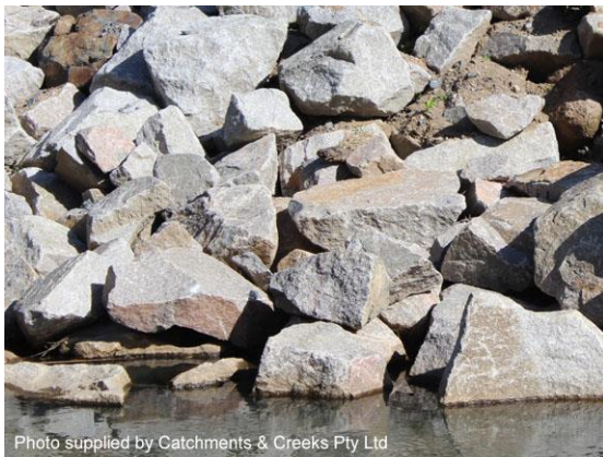
Rock riprap with open voids
