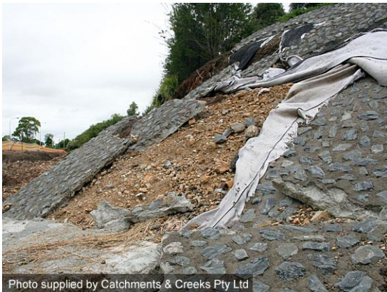
Flood damage to grouted stone pitching
