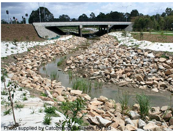
Reconstructed waterway channel (Qld)
