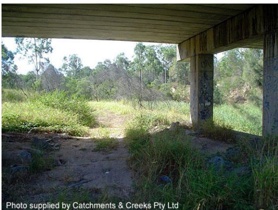
Overbank area under bridge deck, 2005
