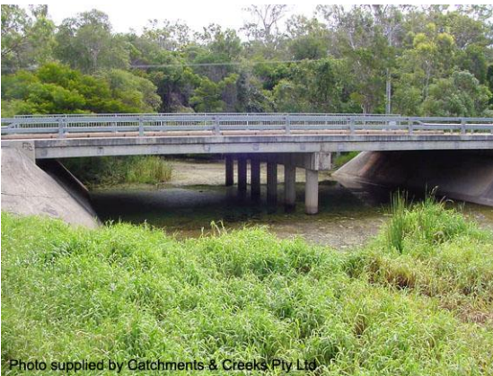
Concrete abutments (Qld)
