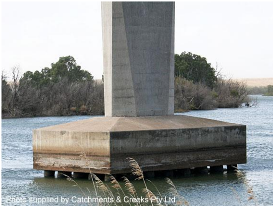
Bridge footing (SA)
