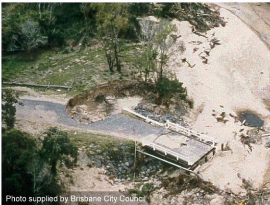
Flood damage to approach road
