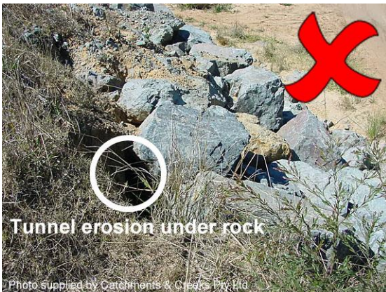
Tunnel erosion under rocks
