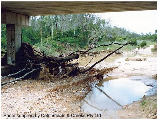
Scour hole formed by flood debris (Qld)
