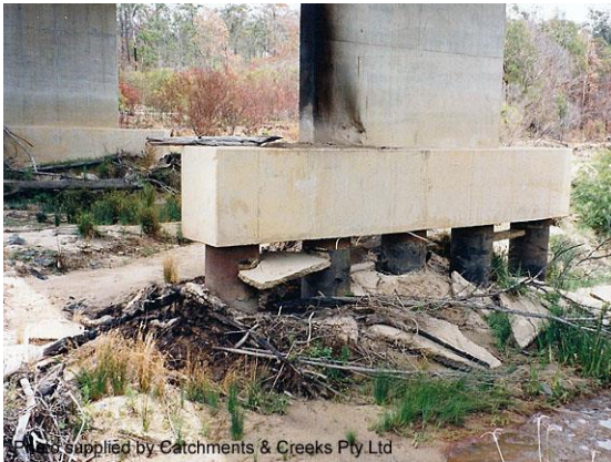
Logan Motorway, Oxley Creek, Qld
