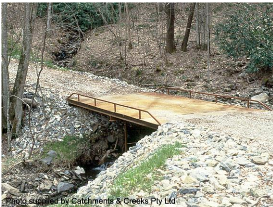
Minor bridge (USA)
