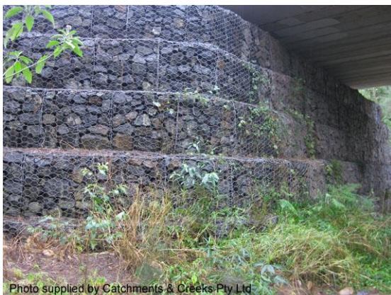
Gabion-protected bridge abutment
