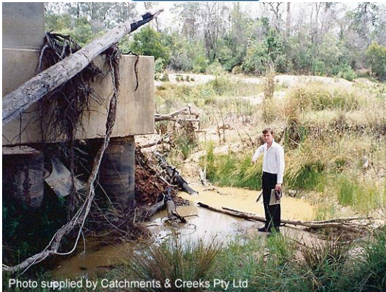
Photo supplied by Catchments & Creeks Pty Ltd
