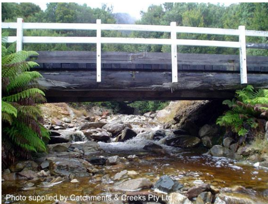
Minor bridge crossing (Tas)
