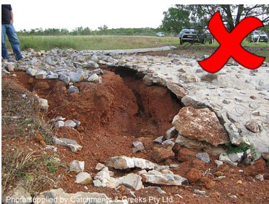
Grouted rock placed on dispersive soil
