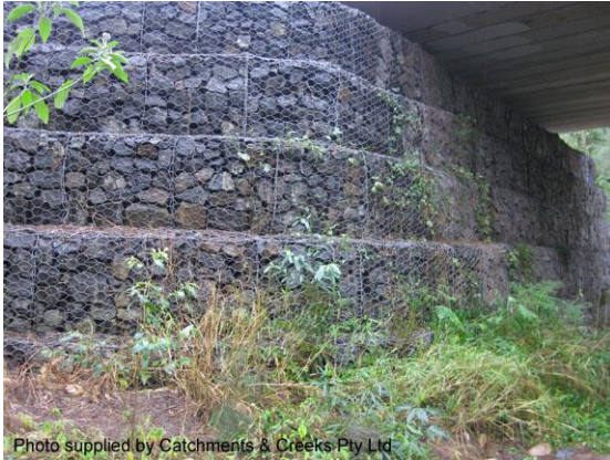
Gabion-protected bridge abutment (Qld)
