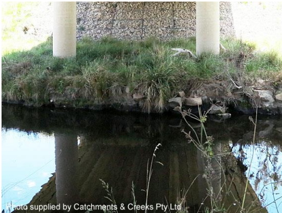
Vegetated rock stabilisation (NSW)
