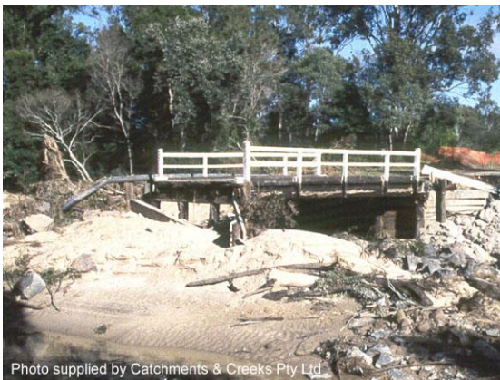
Timber bridge post May 1996 flood
