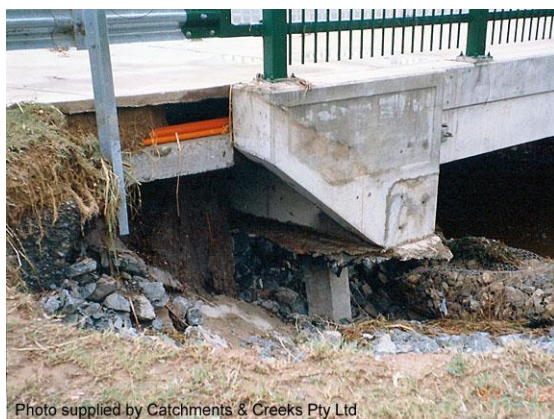
Damage to abutment footing, 1994
