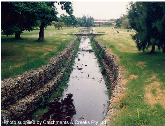
Gabion-lined storm drain (NSW)
