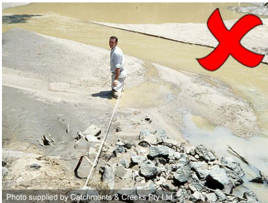
Weak sandy bed structure after a flood
