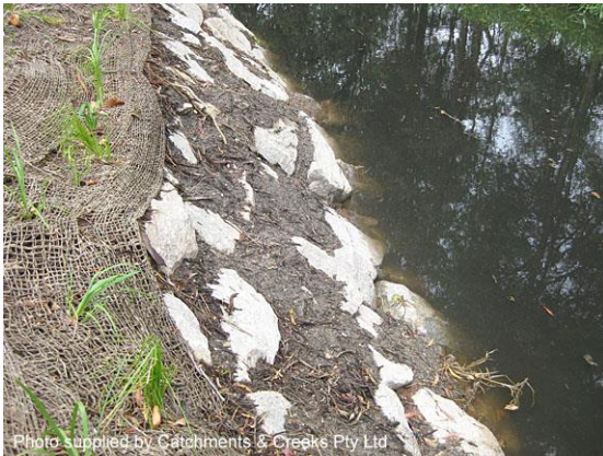
Voids filled with soil ready for planting
