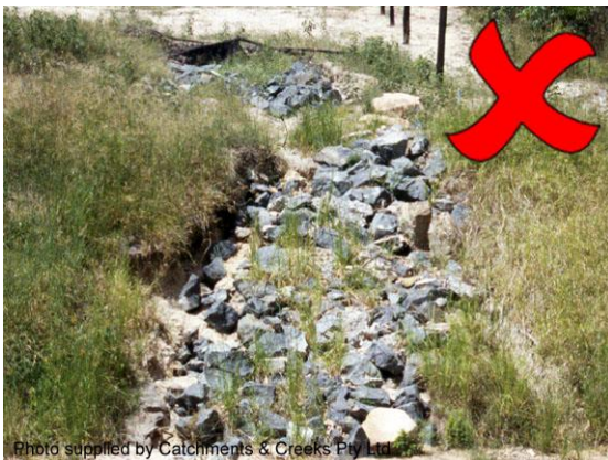
Batter chute placed on a dispersive soil
