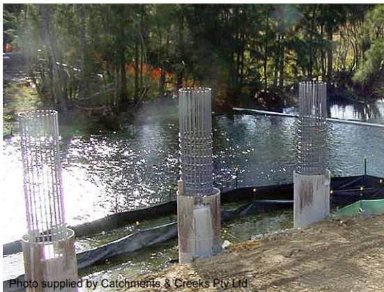
Bridge construction (NSW)
