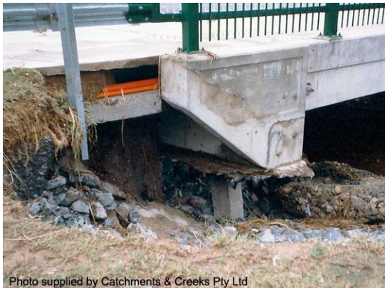
Flood damage to bridge abutment
