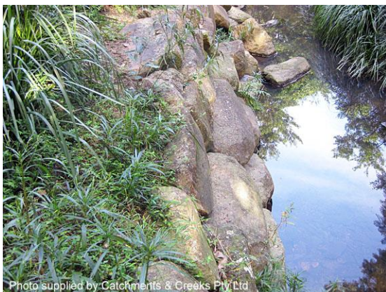
Rocks placed on a steep slope (Qld)
