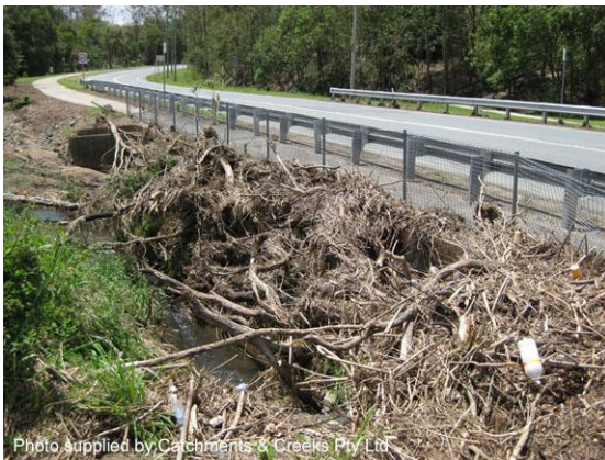
100% debris blockage of a road culvert
