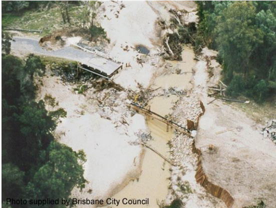
Flood damage to approach roads (Qld)
