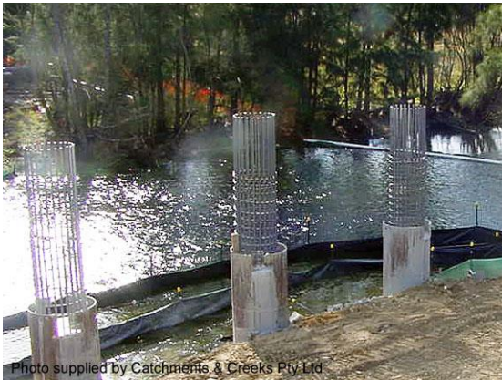
Bridge pier construction (NSW)
