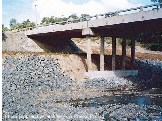
Tie-beam installed on east piers (1992)
