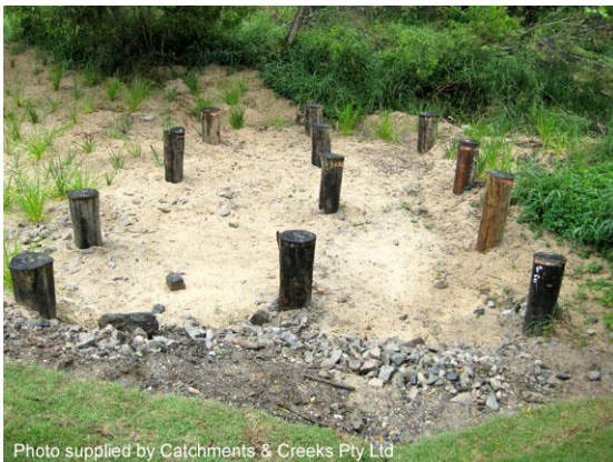
Pile field (Oxley Creek, Willawong)
