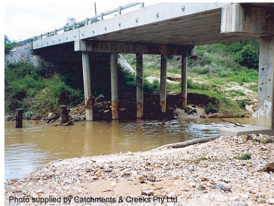
Post-1991 flood damage, east pier
