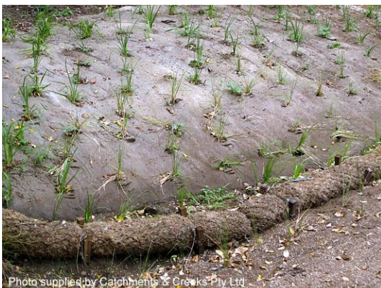
Coir 'geo-log' temporary toe protection
