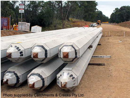
Bridge piles (Qld)
