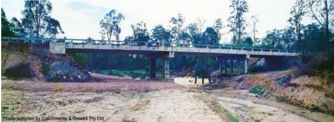
Pre-1991 flood showing existing flood damage, November 1991
