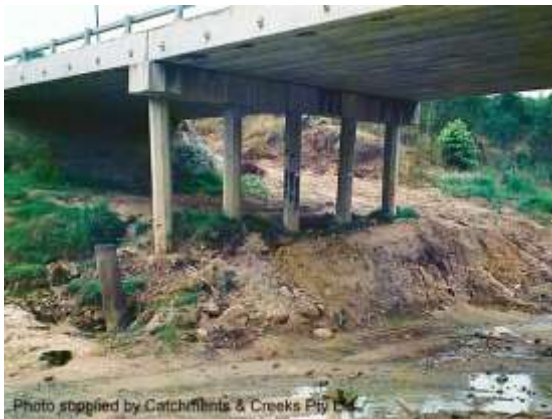
Pre-1991 flood, east pier
