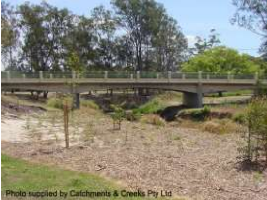
Bridge with no instream piers (Qld)
