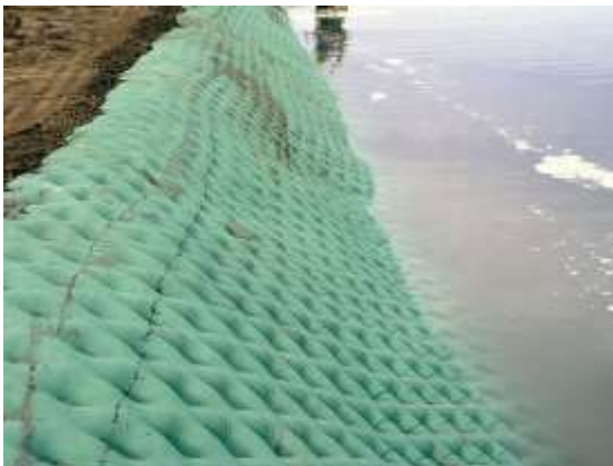
Grout-filled mattress
