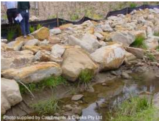
Larger rocks forming toe protection
