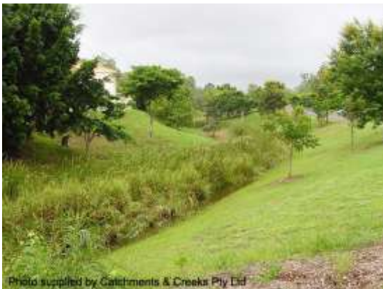
Constructed stormwater channel (Qld)
