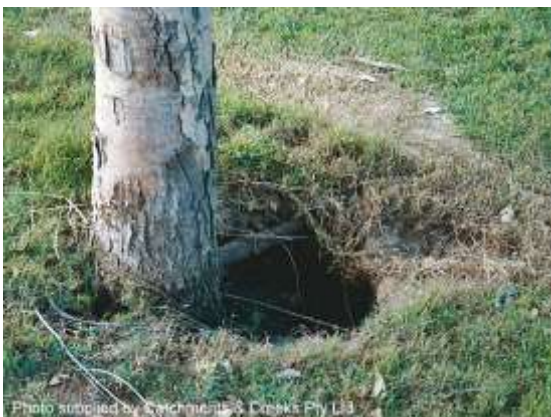
Scour pattern similar to a 'wide' pier
