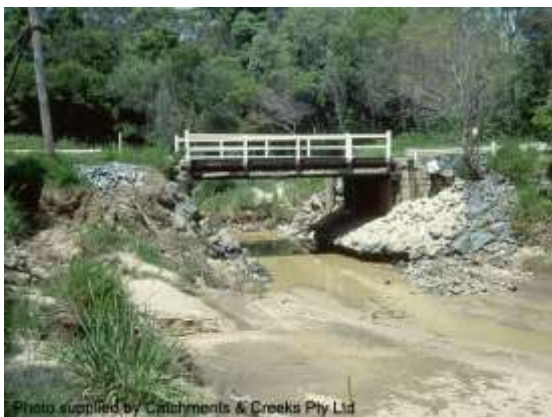
Original bridge prior to 1996 flood
