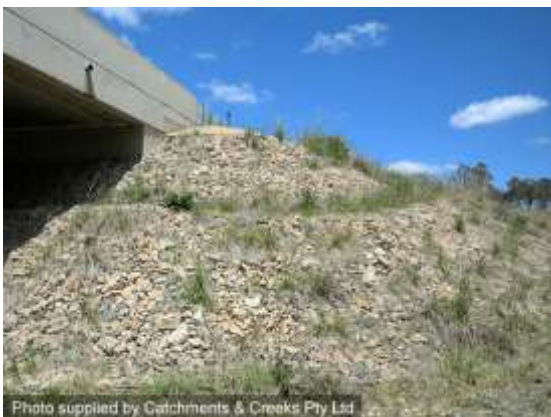
Vegetated rock mattresses (NSW)
