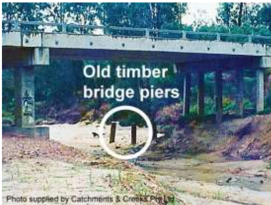
Old timber bridge piers (1991)
