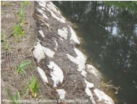
Voids filled with soil ready for planting
