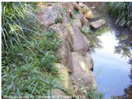
Rocks placed on a steep slope (Qld)
