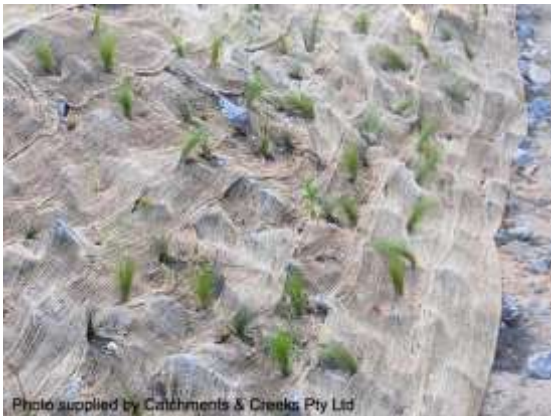
Planted rock covered with jute mesh
