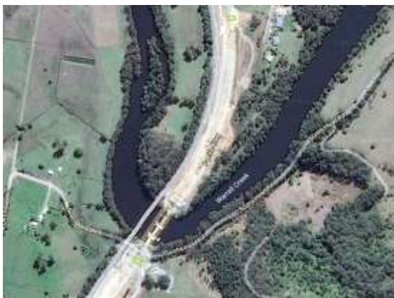
Pacific Highway, Warrell Creek
