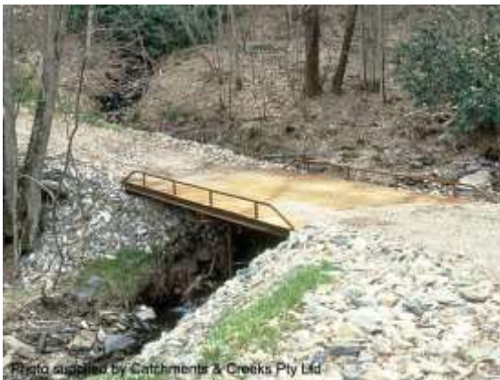
Minor bridge (USA)
