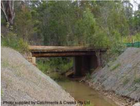
Single lane timber bridge (NSW)
