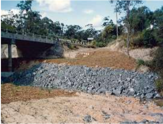
Rock placement upstream of a bridge
