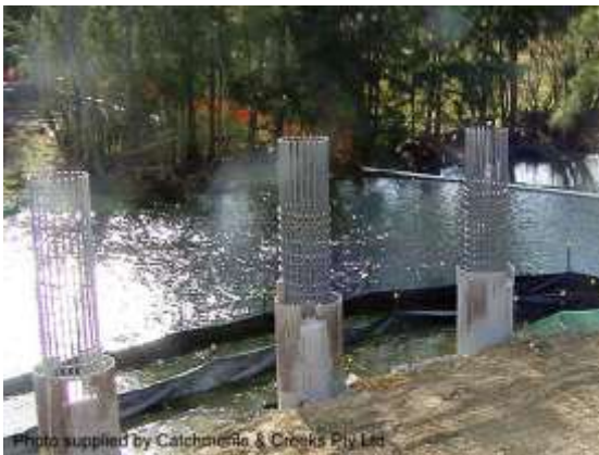
Bridge pier construction (NSW)
