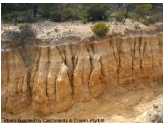
Fluting erosion in a dispersive soil
