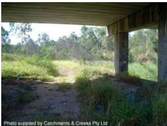
Overbank area under bridge deck, 2005
