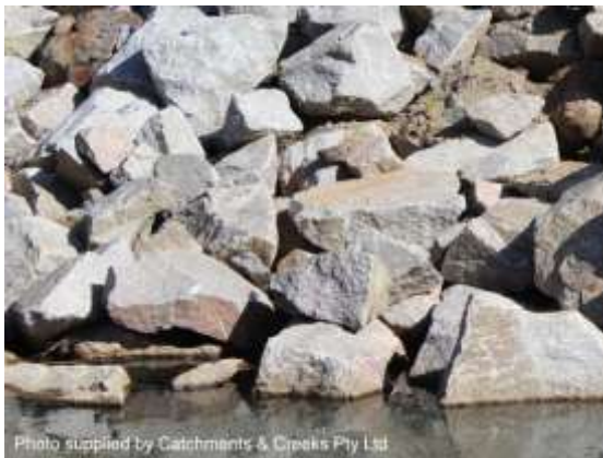
Rock riprap with open voids
