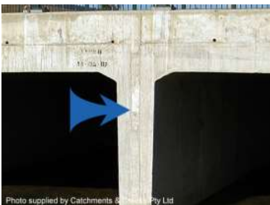
Gap between culvert legs filled with grout
