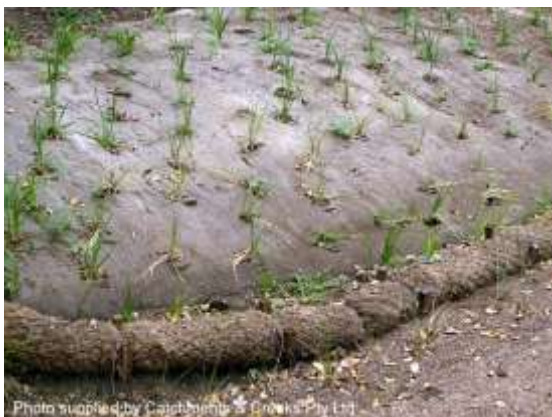
Coir 'geo-log' temporary toe protection
