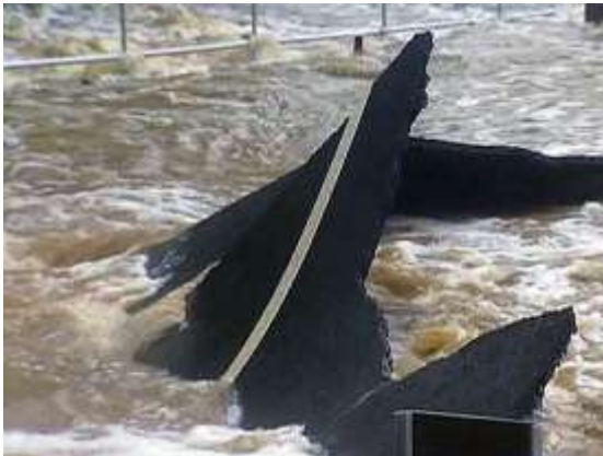
Pavement failure, Queensland, 2011
