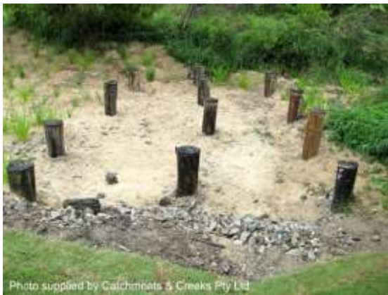
Pile field (Oxley Creek, Willawong)
