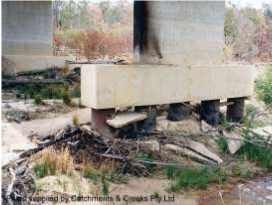
Exposed pier foundations (Qld)
