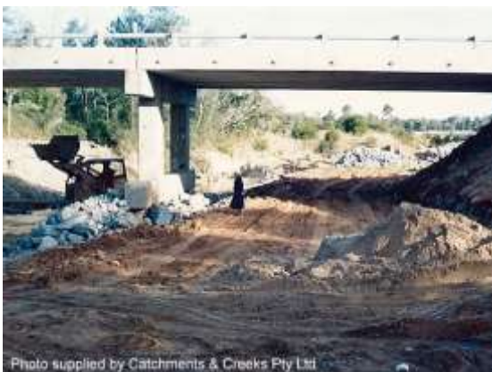
Vegetation cleared from under a bridge
