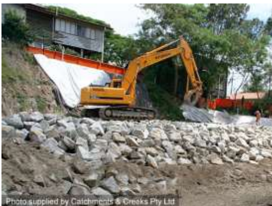
Rock placement over filter cloth
