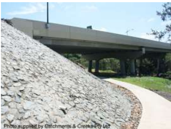
Grouted stone pitched abutment (Qld)
