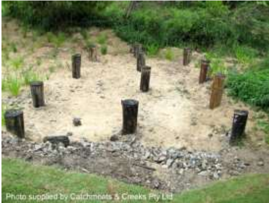
Pile field (Oxley Creek, Willawong, Qld)
