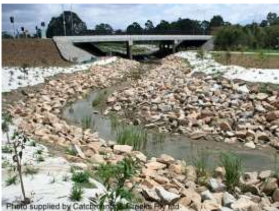
Reconstructed waterway channel (Qld)
