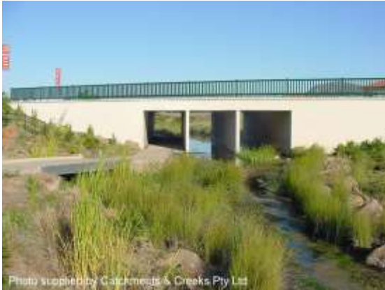
Constructed stormwater channel (Qld)
