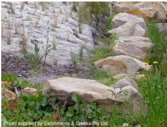
Large toe rock (NSW)
