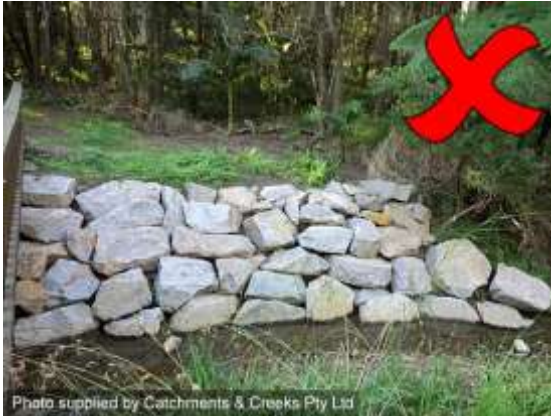
Non-vegetated rock stabilisation
