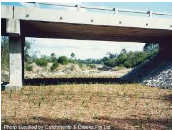
Scour protection measures (Qld)
