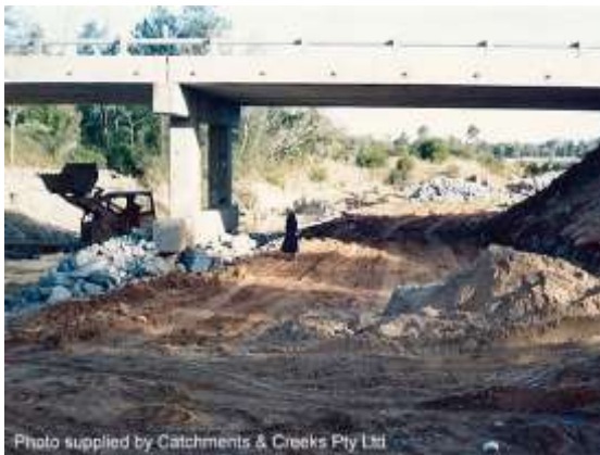
Overbank floodway stabilisation, 1992
