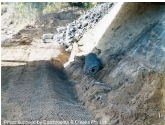
Trenching of rockfall netting, 1992
