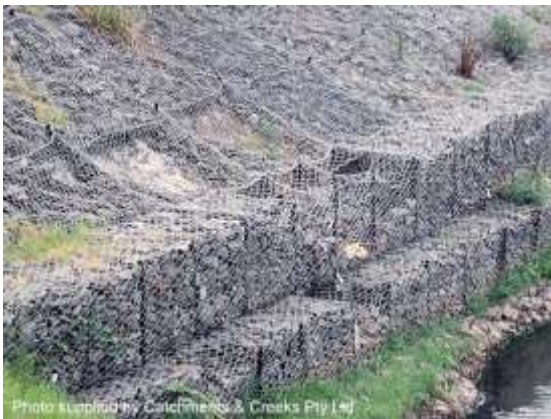
Bridge outlet, Fairfield, NSW
