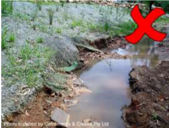
Erosion along toe of bank
