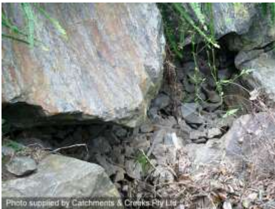
Small-rock filter layer (Qld)
