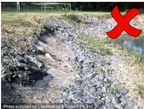
Rocks displaced down filter cloth
