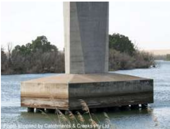
Bridge footing (SA)
