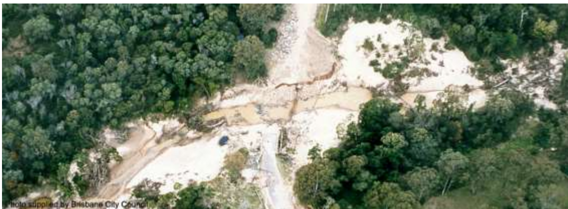
May 1996 flood damage (upstream is on the right-hand side)
