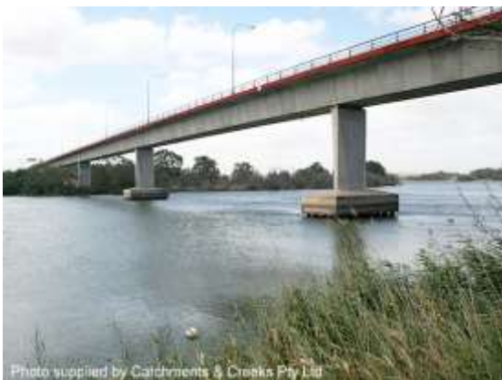
Major bridge crossing (SA)
