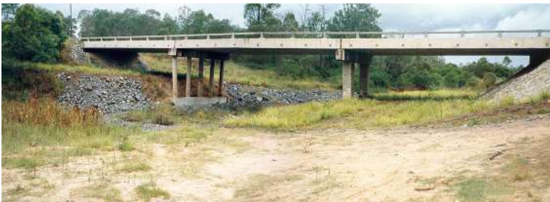
Finished bridge scour works, January 1994
