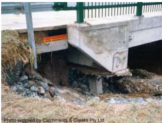
Damage to abutment footing, 1994
