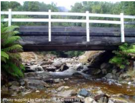
Minor bridge crossing (Tas)
