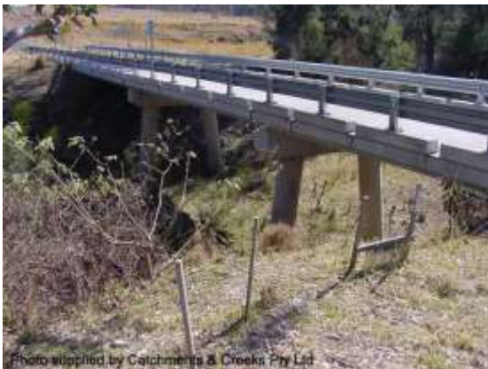
Bridge with minimal constriction (NSW)
