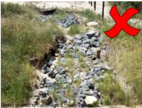
Batter chute placed on a dispersive soil
