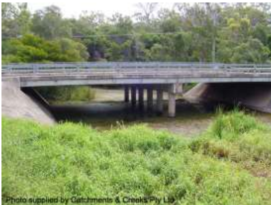
Concrete abutments (Qld)
