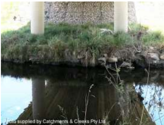
Vegetated rock stabilisation (NSW)
