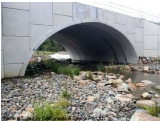
Arch bridge crossing (NSW)
