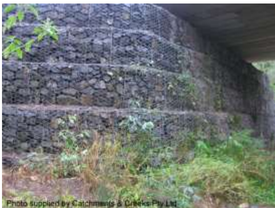
Gabion-protected bridge abutment
