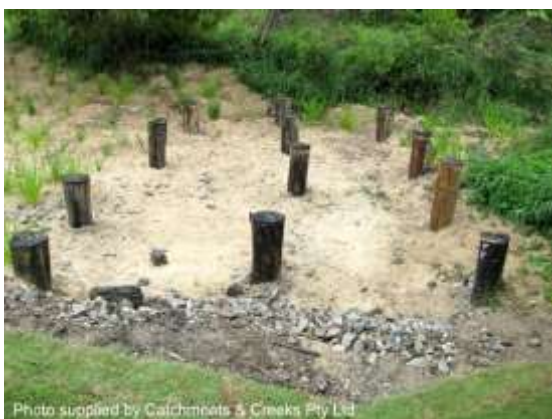
Pile field, Oxley Creek, 2010
