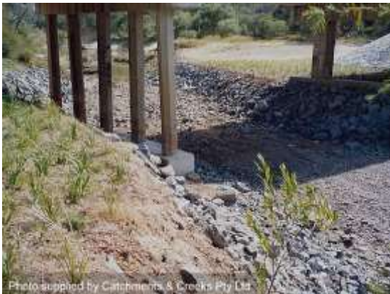
Rock placement on creek bed (1992)
