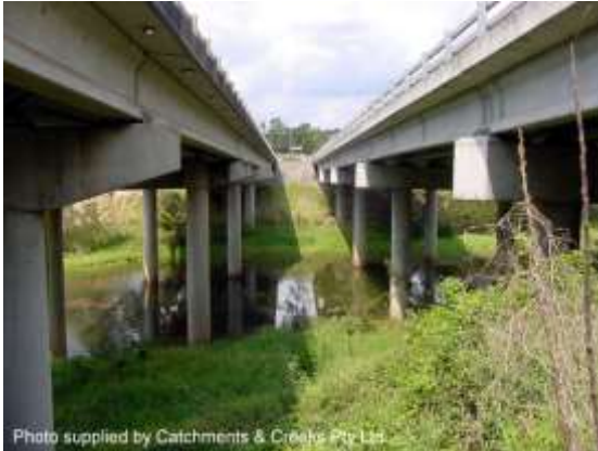
Twin bridge crossing (Qld)
