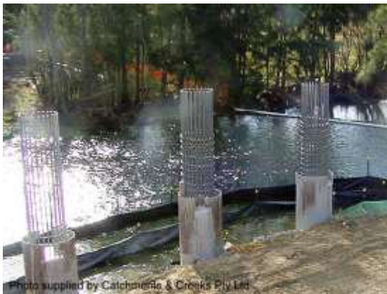
Bridge construction (NSW)
