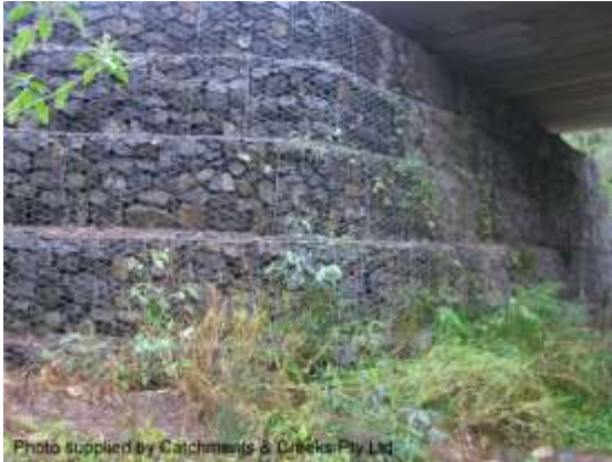
Gabion-protected bridge abutment (Qld)
