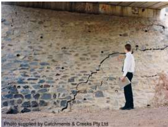
Abutment damage (Qld)
