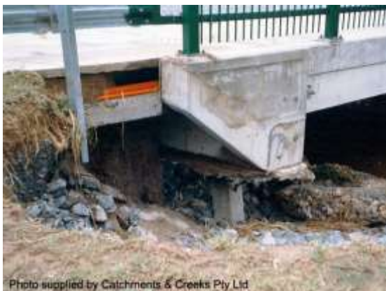
Flood damage to bridge abutment
