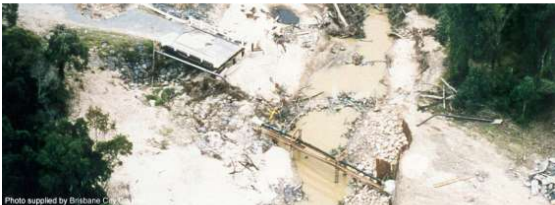
May 1996 flood damage (looking downstream)
