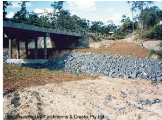
Rock placement on creek banks (1992)
