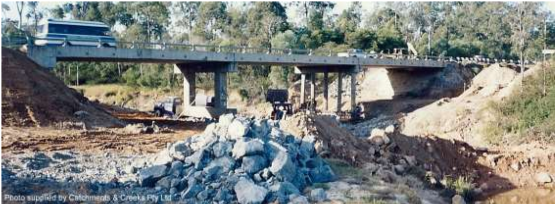
Rock stabilisation of the creek banks and creek bed (June 1992)
