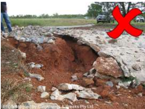
Grouted rock placed on dispersive soil
