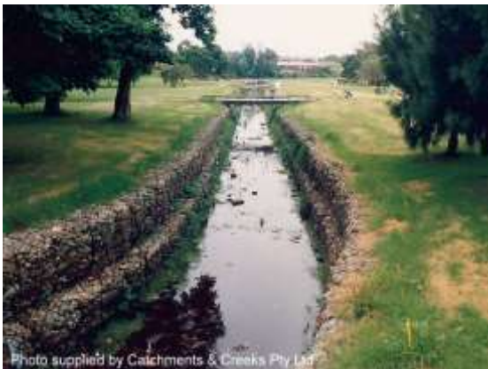
Gabion-lined storm drain (NSW)
