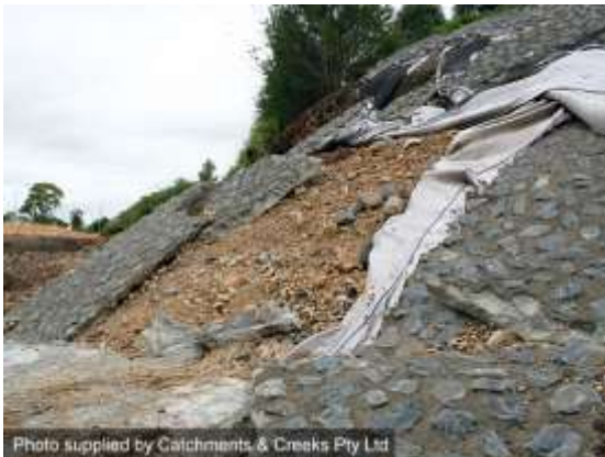
Flood damage to grouted stone pitching
