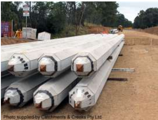
Bridge piles (Qld)
