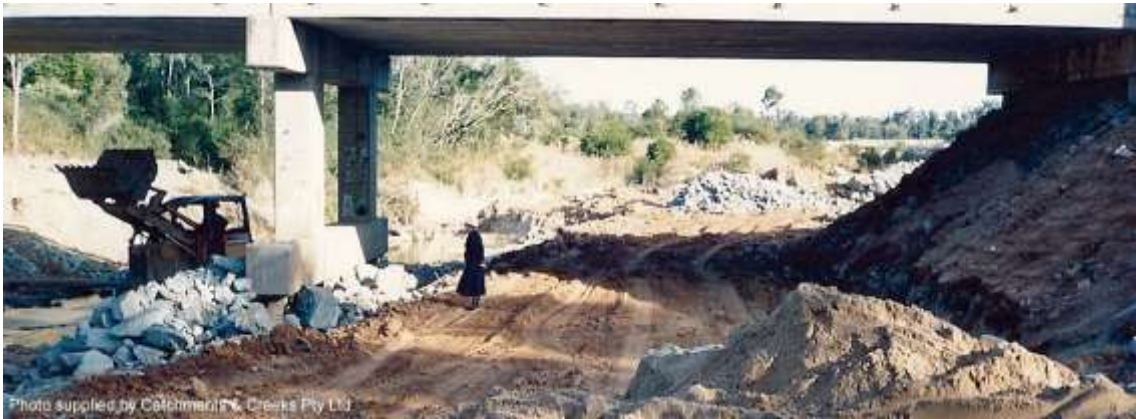
Rock stabilisation of the creek banks and creek bed (June 1992)
