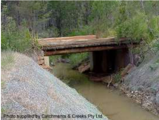
Minor bridge crossing (NSW)
