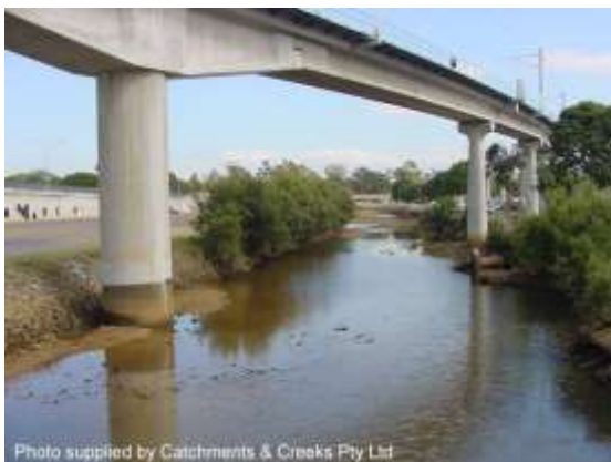
Airport Link, Schulz Canal, Brisbane
