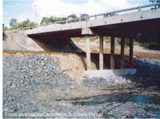
Tie-beam installed on east piers (1992)
