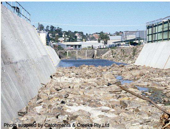
Grouted rock bed on concrete channel
