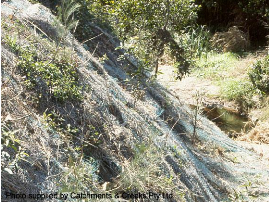
Synthetic matting placed on bank (1991)
