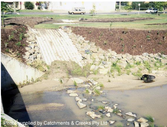
Maintenance access ramp (1997)
