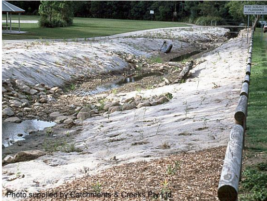
Pool-riffle system (2000)
