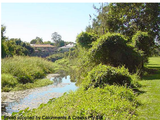
Looking downstream towards weir (2003)
