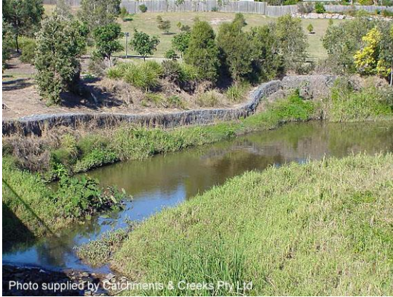
Looking upstream from bridge (2001)
