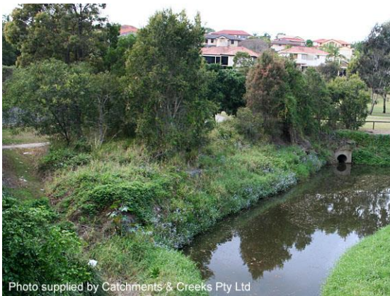
Looking upstream from bridge (2008)
