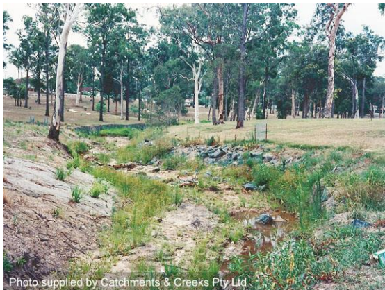
Looking d/s with works on right (1995)
