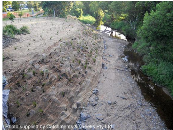
Placement of jute mesh, 13/12/12
