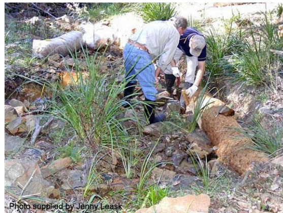
Toe stabilisation with jute logs (2012)
