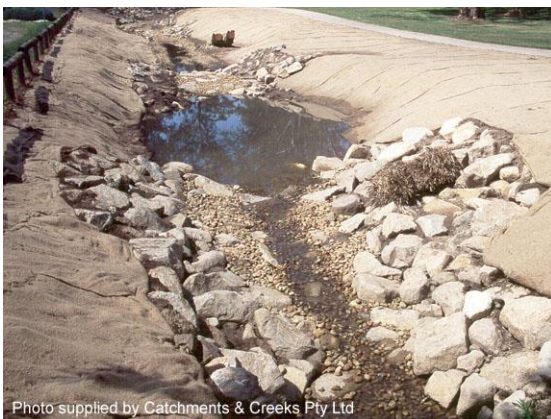
Pool-riffle system (2000)
