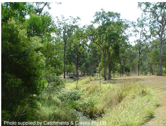
Looking d/s with works on right (2004)
