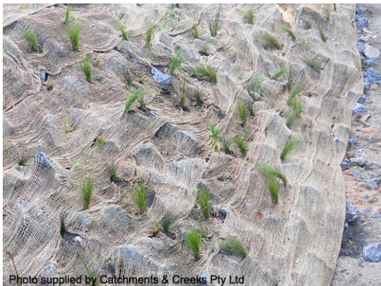
Placement of jute mesh, 13/12/12
