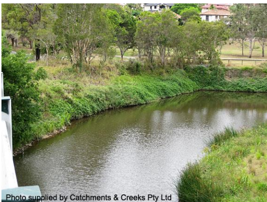
Looking upstream from bridge (2014)
