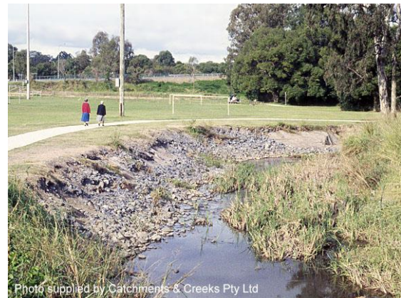
Downstream of footbridge (1996)
