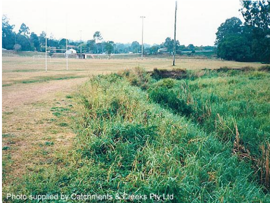
Downstream of footbridge (1992)
