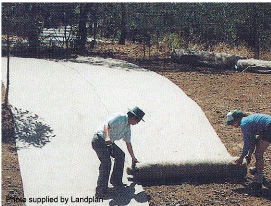
Placement of jute matting (1991)
