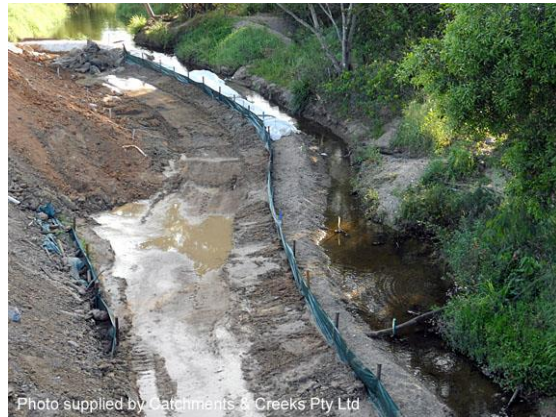
Instalment of sediment fence, 2/11/12
