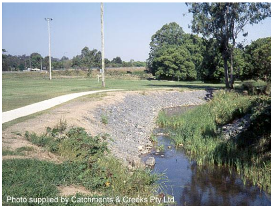
Downstream of footbridge (1995)
