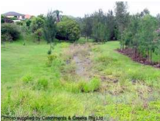
Looking downstream from culvert (2001)
