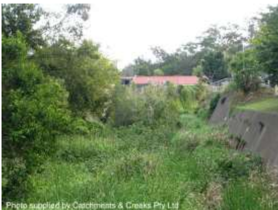
Looking upstream from footbridge (2014)
