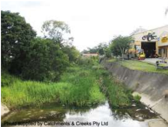
Looking upstream Magura St (2014)
