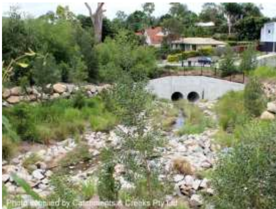
Modified creek channel u/s of Tilquin St
