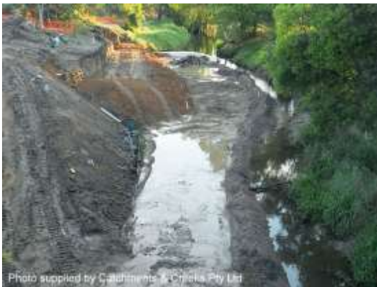
Placement of fill, 31/10/12
