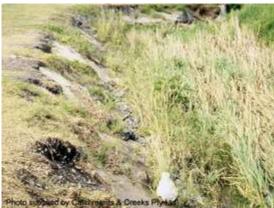
Downstream of footbridge (1997)
