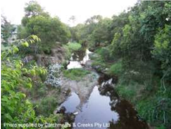
Eroded bank on left, 28/9/12
