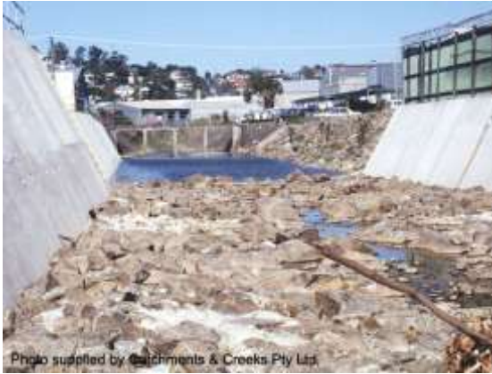
Looking d/s to Magura St footbridge
