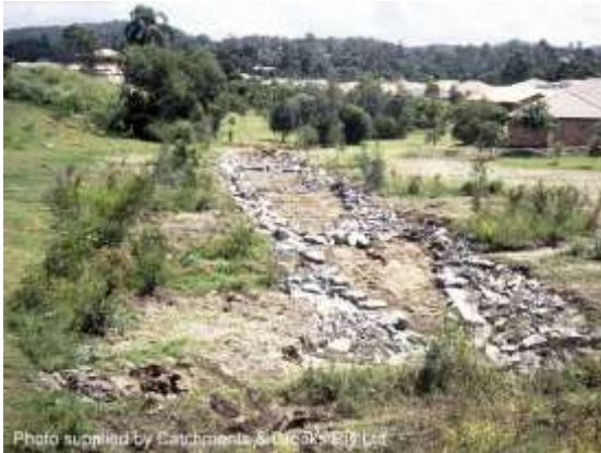
Looking downstream from culvert (1997)
