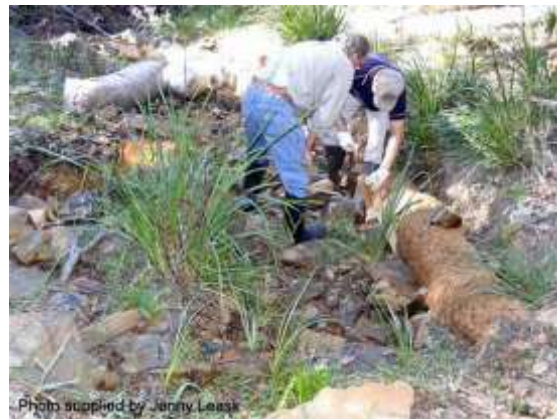
Toe stabilisation with jute logs (2012)
