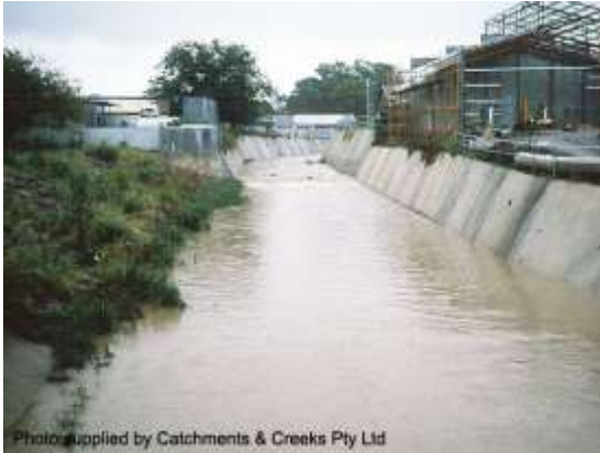
Looking upstream Magura St (1998)
