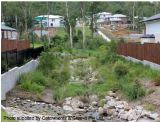
Looking downstream (February 2013)
