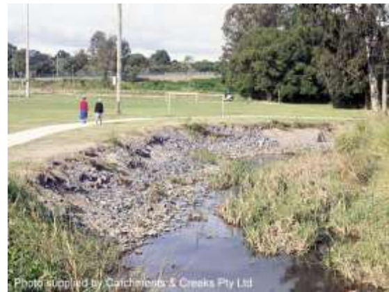
Downstream of footbridge (1996)
