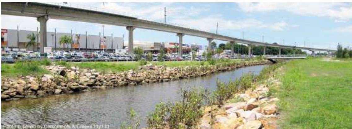
Looking downstream towards the footbridge (2014)
