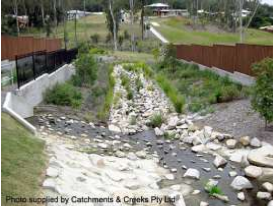
Looking d/s from Settlement Rd (2012)
