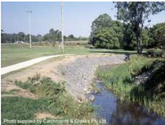
Downstream of footbridge (1995)
