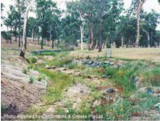
Looking d/s with works on right (1995)
