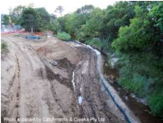
Final bank shaping, 7/11/12
