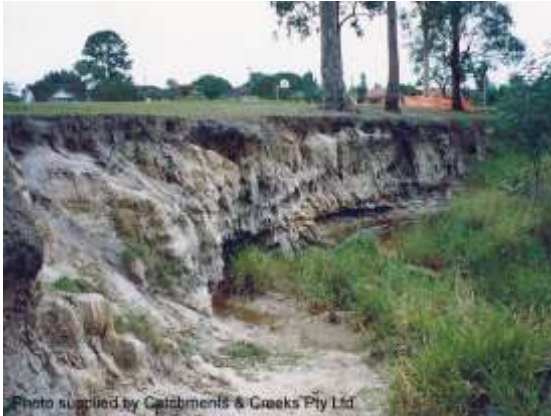
Severe bank erosion, Inala, Qld
