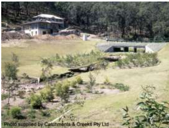
Damage to landscaping by storm (1996)
