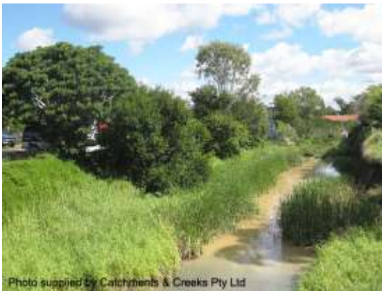
Looking upstream Magura St (2011)
