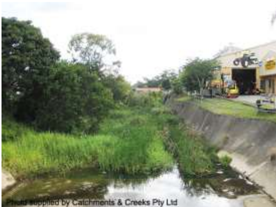
Looking upstream Magura St (2014)
