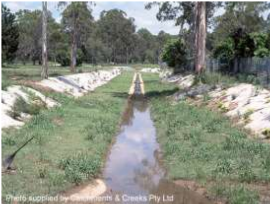
Formed channel with concrete low-flow
