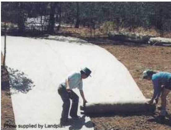
Placement of jute matting (1991)
