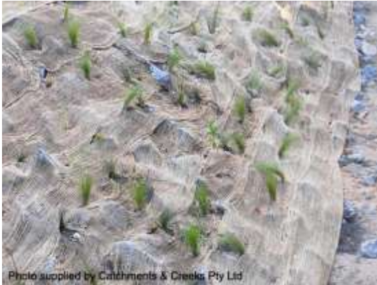
Placement of jute mesh, 13/12/12
