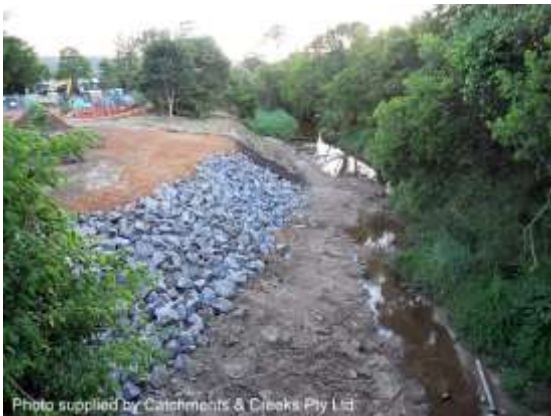
Final rock placement, 30/11/12
