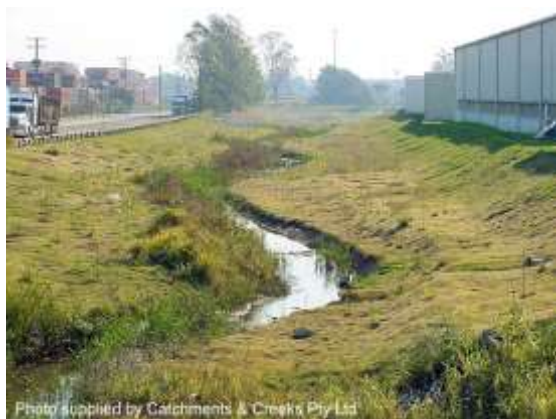
Looking downstream from culvert (2000)
