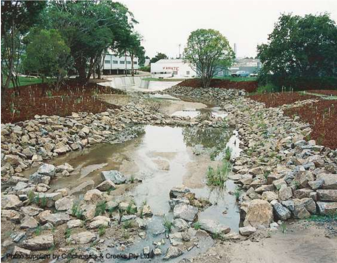
Looking downstream from the Wardell Street off ramp (1997)
