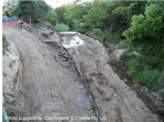
Establish flow diversion bund, 24/10/12
