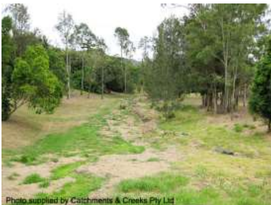
Looking downstream from culvert (2014)
