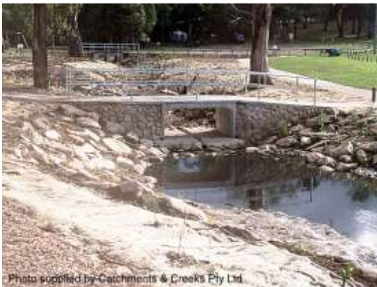
New footbridge (d/s of junction, 2000)
