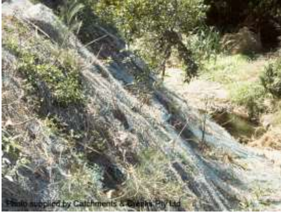
Synthetic matting placed on bank (1991)
