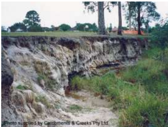
Bank erosion looking upstream (1993)
