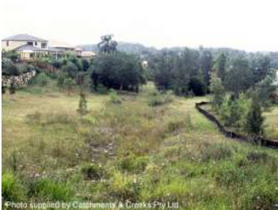
Looking downstream from culvert (1998)
