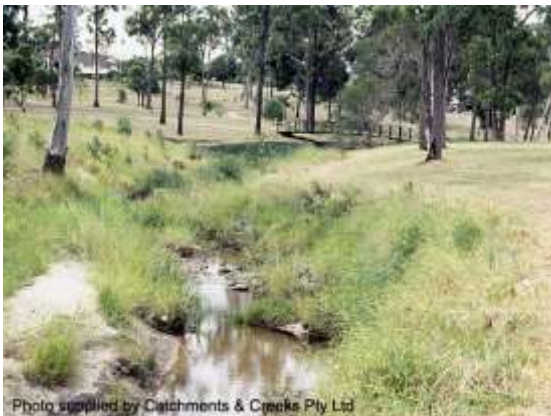
Looking d/s with works on right (1996)
