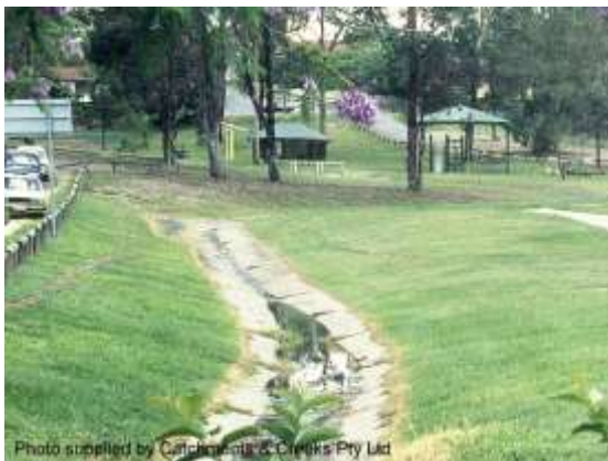
Original concrete drain (1998)
