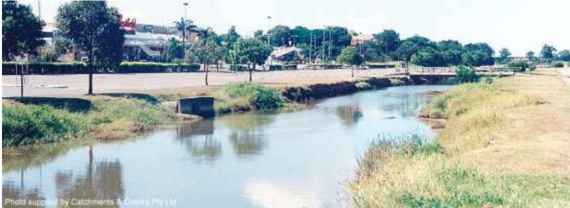
Looking downstream towards the footbridge (1996)
