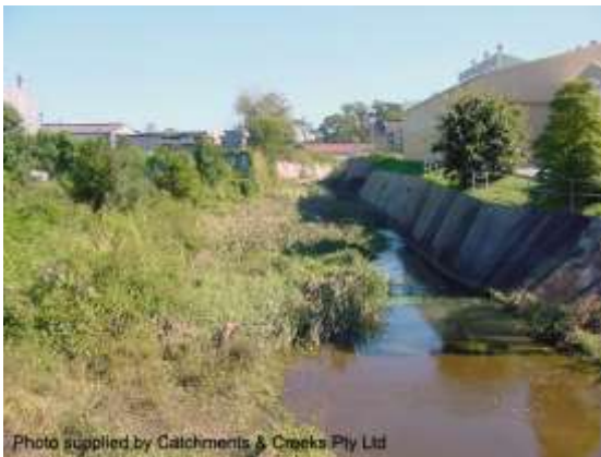
Looking upstream Magura St (2003)
