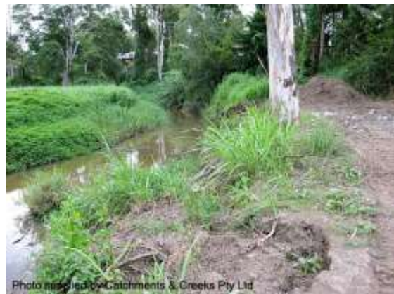
Looking upstream (January, 2011)
