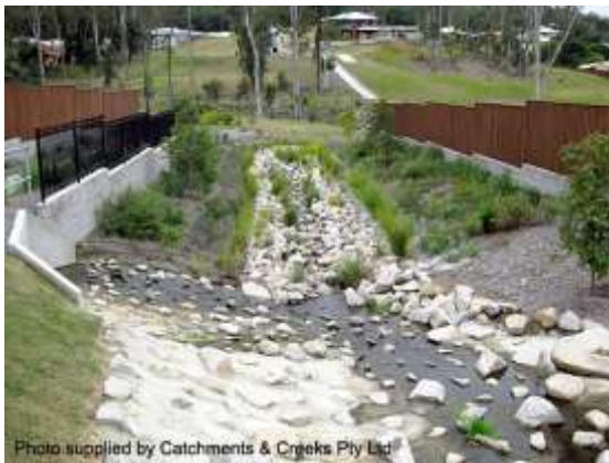
Constructed drainage channel
