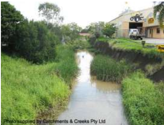
Looking upstream Magura St (2011)
