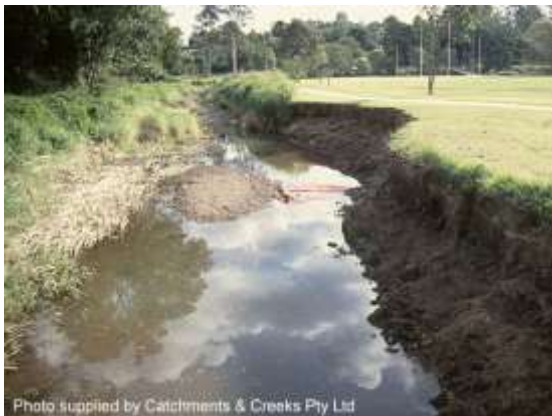
Upstream of footbridge (1996)
