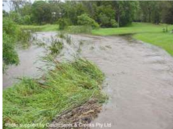
Looking u/s from Ferny Way culvert (2001)
