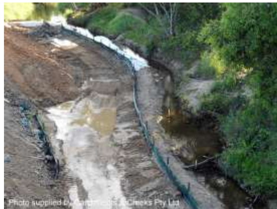
Instalment of sediment fence, 2/11/12
