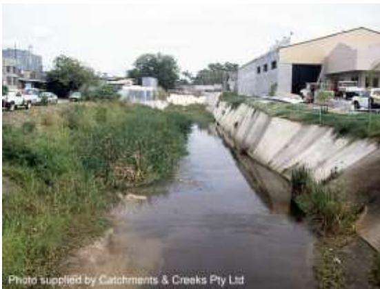
Looking upstream Magura St (1999)
