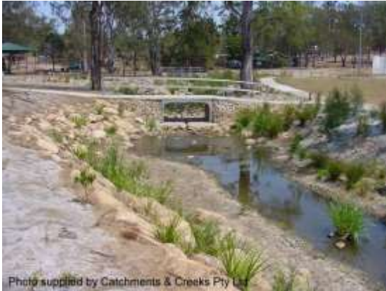
Looking u/s to footbridge (2000)
