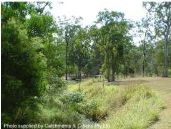
Looking d/s with works on right (2004)
