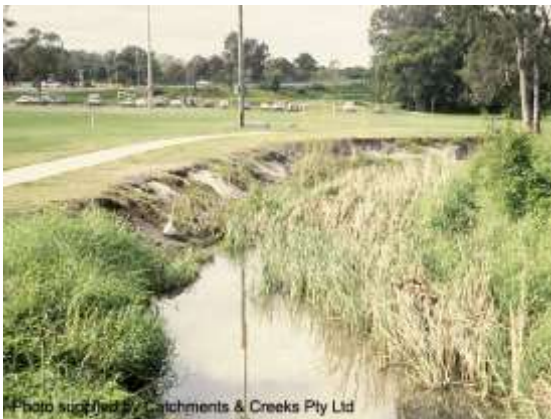
Downstream of footbridge (1997)
