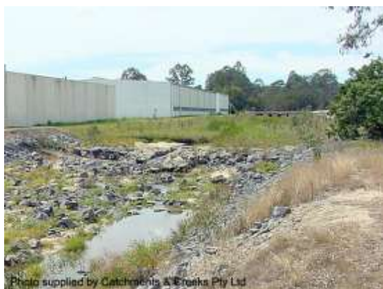
Looking upstream from drop structure
