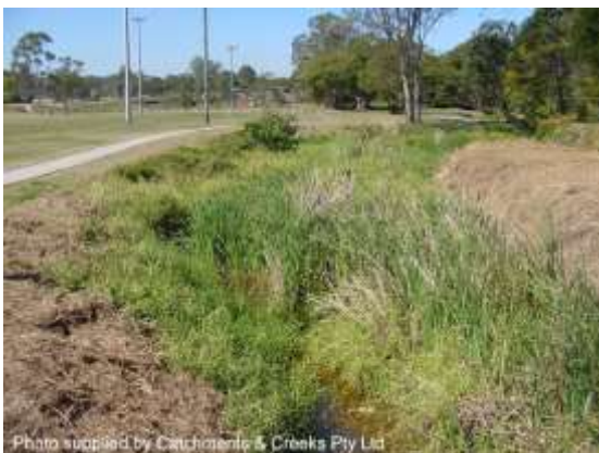
Downstream of footbridge (2000)
