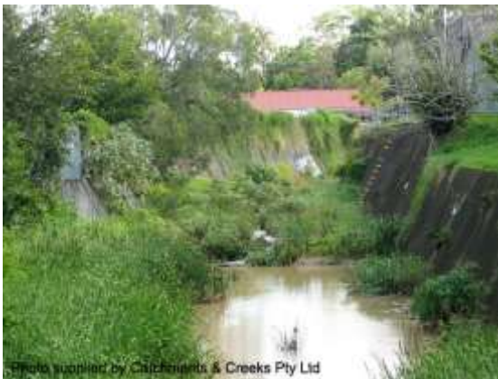
Looking upstream from footbridge (2011)
