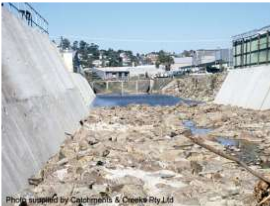
Grouted rock bed on concrete channel
