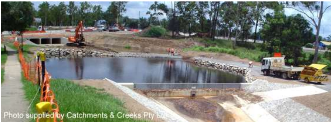
Construction of stormwater treatment wetland upstream of Ferny Way culvert (2004)
