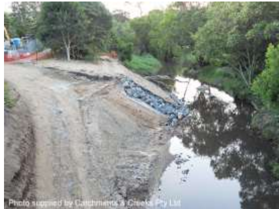
Placement of rock, 20/11/12
