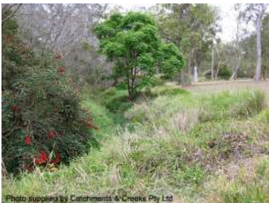
Looking d/s with works on right (2014)
