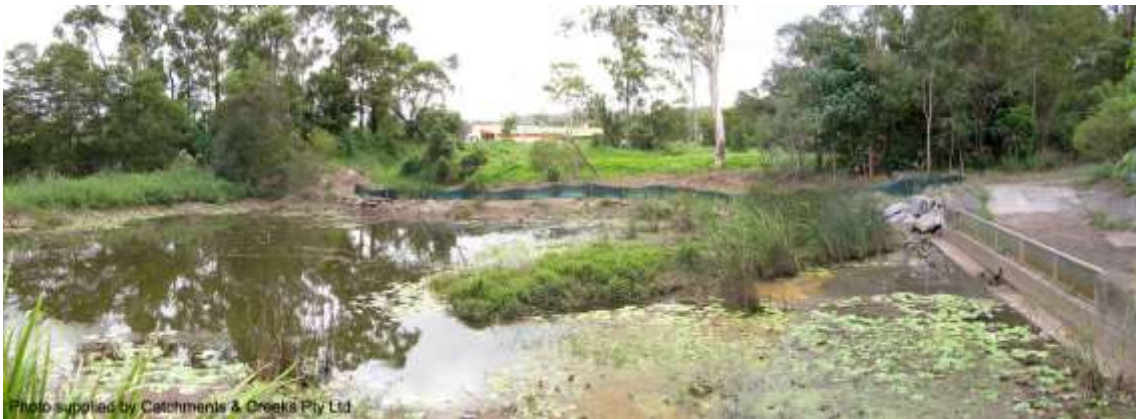
Re-construction of creek bank, January 2011 (Kedron Brook in background)
