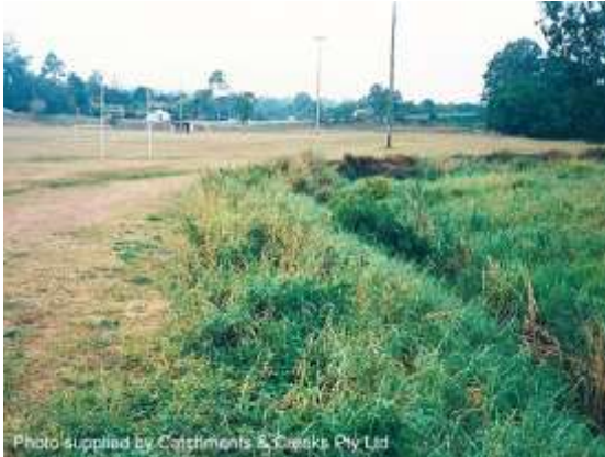
Downstream of footbridge (1992)
