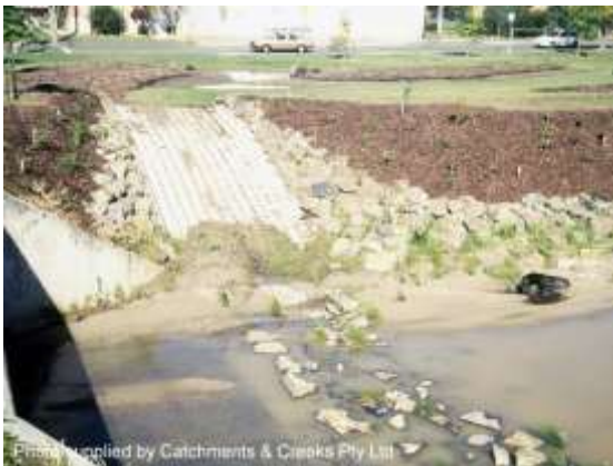
Maintenance access ramp (1997)
