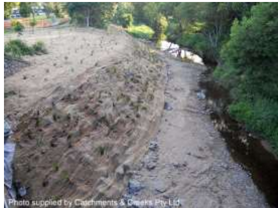
Placement of jute mesh, 13/12/12
