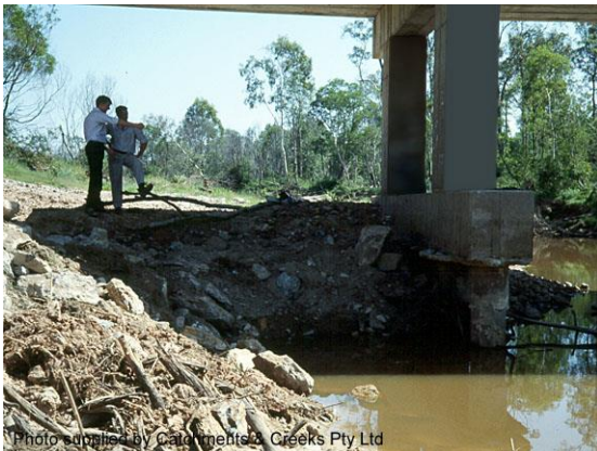
Erosion of bridge pier foundations (Qld)
