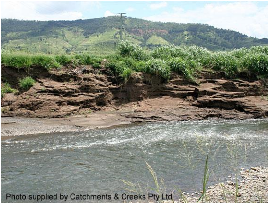
Flood scour of a creek bank (Qld)
