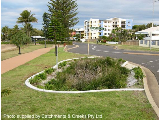
Roadside stormwater treatment (Qld)
