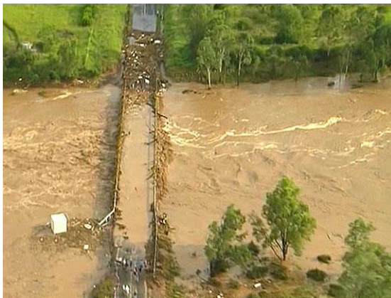
Flow conditions just below the bridge deck
