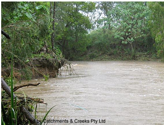
Subcritical flow causing bank erosion
