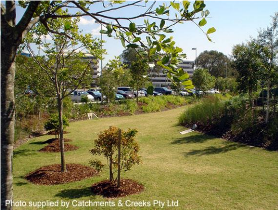
Stormwater detention basin (Qld)
