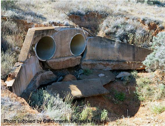
Damage to a road culvert (NSW)
