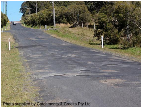
Heavily 'patched' bitumen road (NSW)
