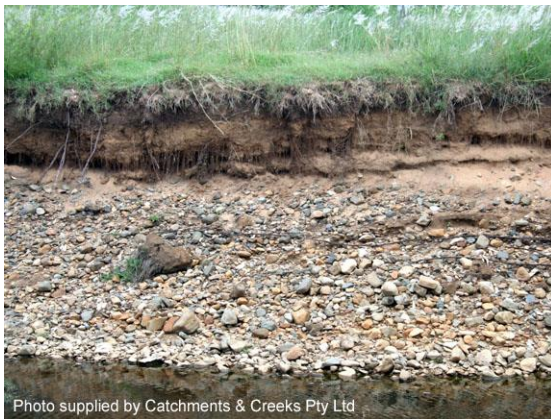
Gravel-filled creek bank (Qld)
