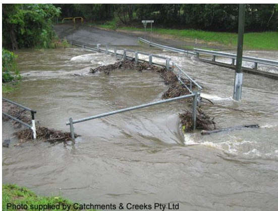
Backwater effects of a culvert crossing
