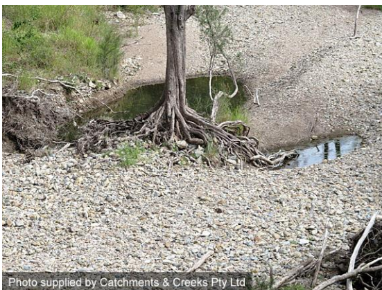
Bed erosion around the base of a tree
