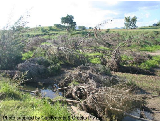
Flood damage to vegetation (Qld)
