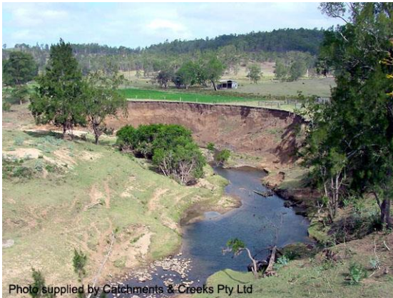
Bank erosion, Clarence River (NSW)
