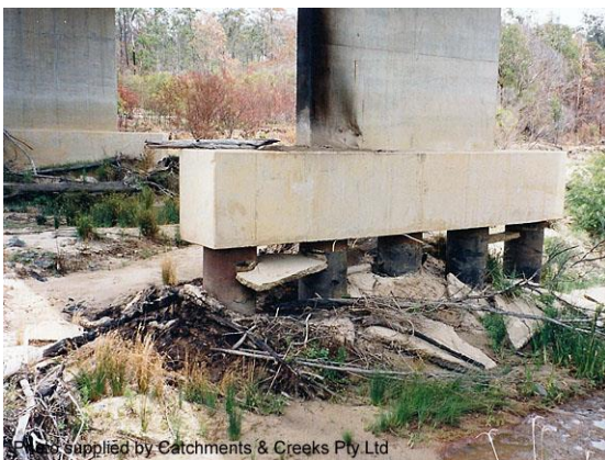
Lowering of a creek bed under a bridge
