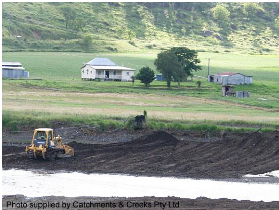
In-channel repair works after a flood (Qld)
