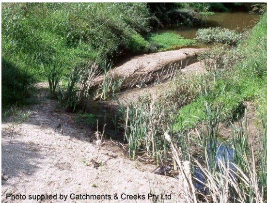
Unnatural sediment in an urban creek
