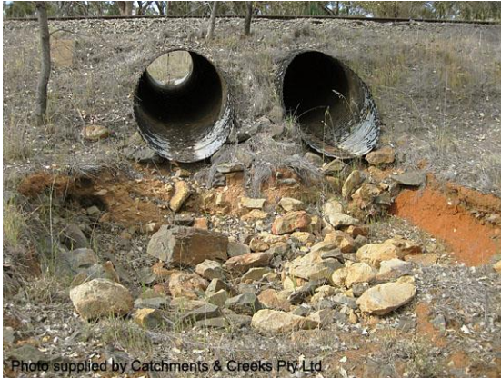
Outlet of a pipe culvert (NSW)
