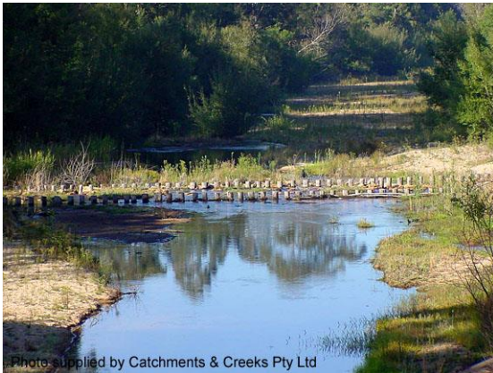
Pile field bed stabilisation (Vic)
