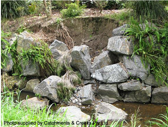
Failed rock stabilisation (Qld)
