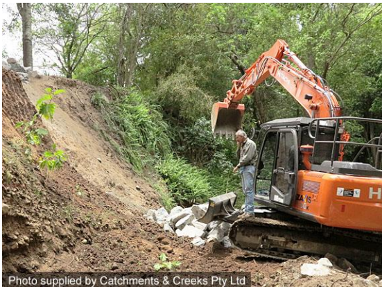
Post-flood bank repairs (Qld)
