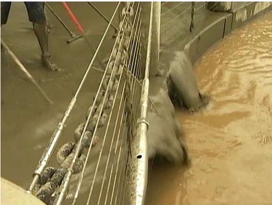
Sweeping the silt back into the river
