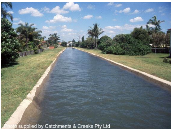
High tide backing-up into a coastal drain
