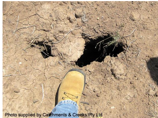
Tunnel erosion (Qld)
