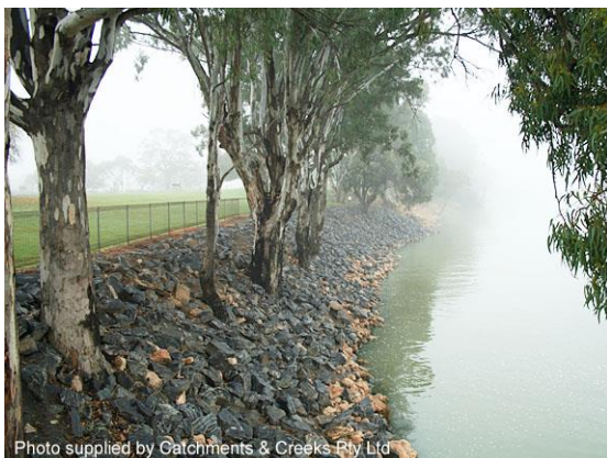
Rock stabilisation of a river bank (NSW)
