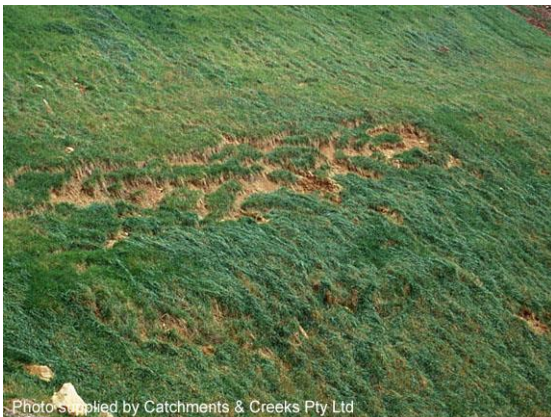
Gravity-induced stress cracks on a slope
