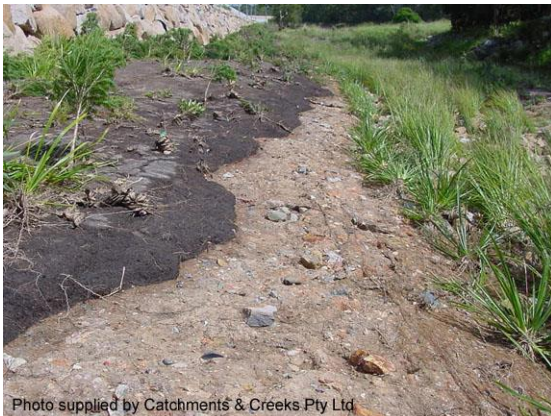
Flood damage to a grass-lined channel
