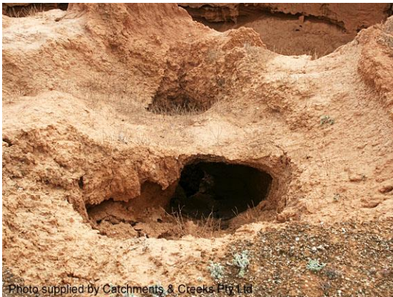
Tunnel erosion (SA)
