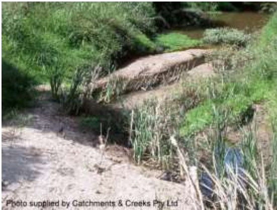
Unnatural sediment in an urban creek
