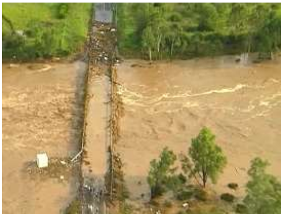
Flow conditions just below the bridge deck
