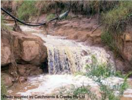
Soil scour (Qld)
