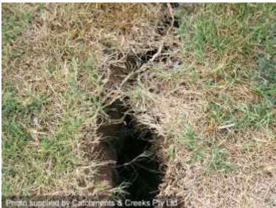
Crack several metres from a creek bank
