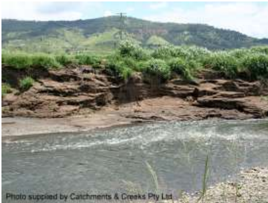
Flood scour of a creek bank (Qld)
