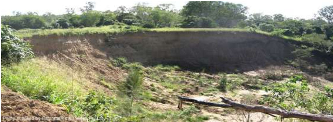
Post-flood, slip circle bank slump, Bundaberg, Queensland, 2011
