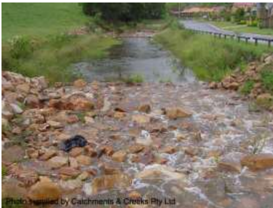
Constructed rock riffle (Qld)
