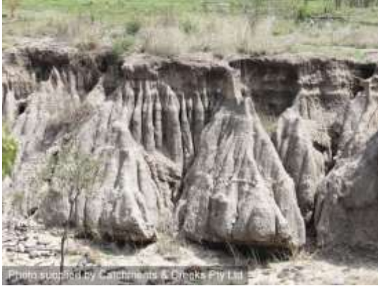
Fluting erosion (Qld)
