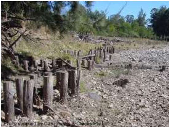
Pile field toe stabilisation (NSW)
