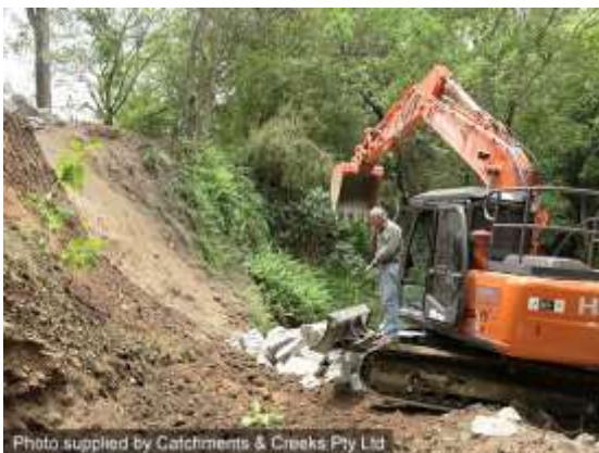
Post-flood bank repairs (Qld)
