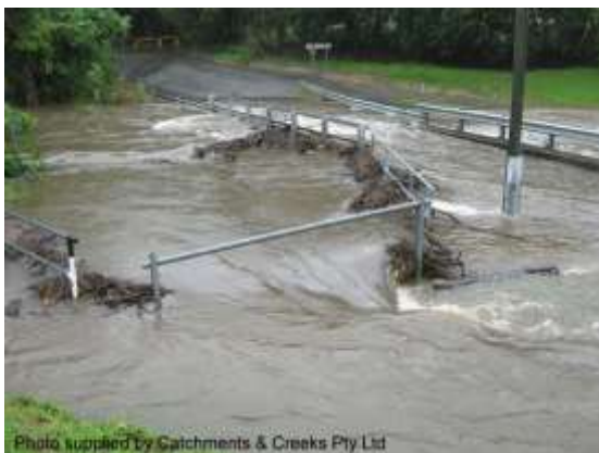
Backwater effects of a culvert crossing
