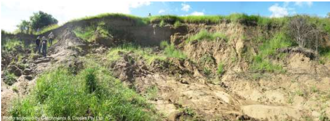
Post-flood, slip circle bank slump, Bundaberg, Queensland, 2011
