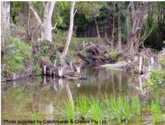
Artificial log groyne (NSW)
