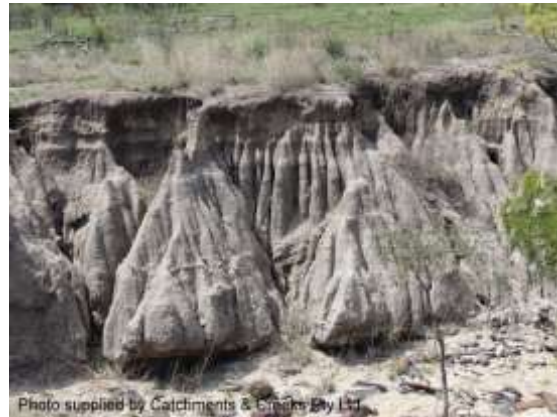
Fluting of a gully bank (Qld)
