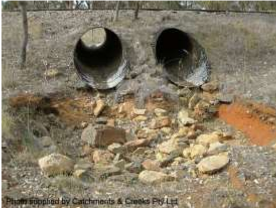
Outlet of a pipe culvert (NSW)
