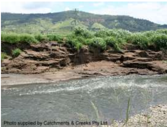
Bank scour (Qld)
