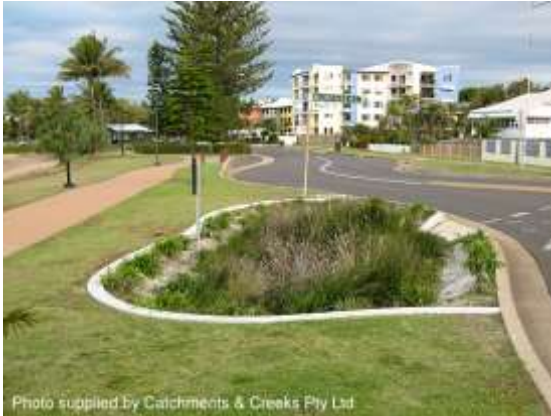
Roadside stormwater treatment (Qld)
