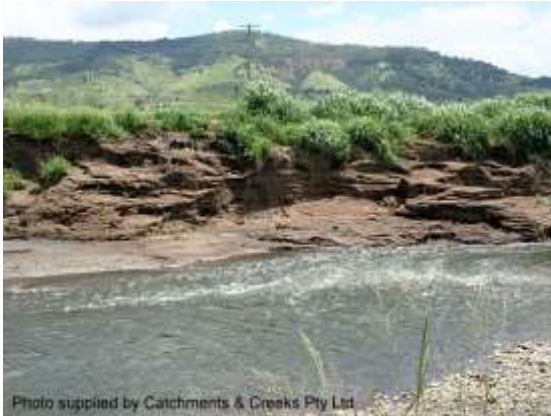
Soil scour caused by high velocity flows
