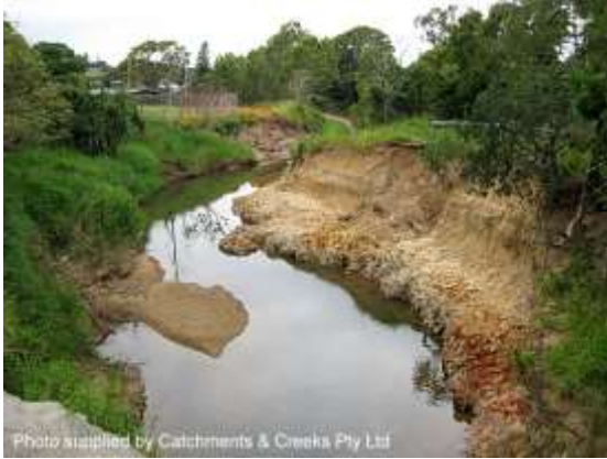
Bank scour (Qld)
