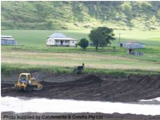
In-channel repair works after a flood (Qld)
