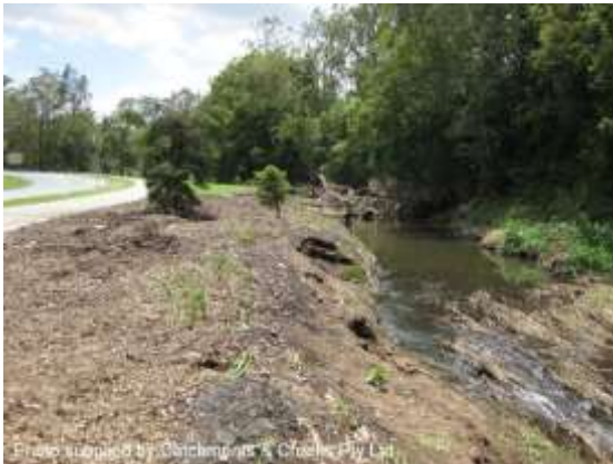
Erosion caused by aggressive weed control
