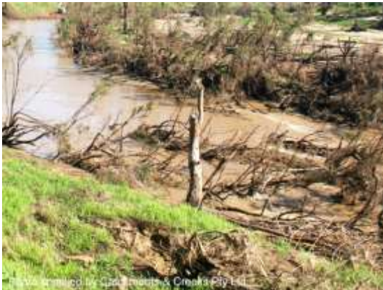
Flood damage to riparian vegetation (Qld)
