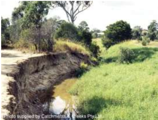
Photo supplied by Catchments & Creeks Pty Ltd Erosion along a shaded north bank (Qld)
