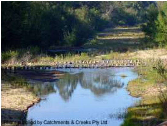
Pile field bed stabilisation (Vic)
