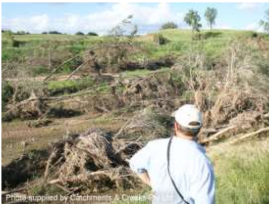
Flood damage to Lockyer Creek, 2011
