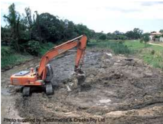
Sediment removal from an urban creek
