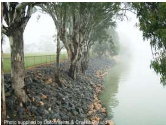
Rock stabilisation of a river bank (NSW)
