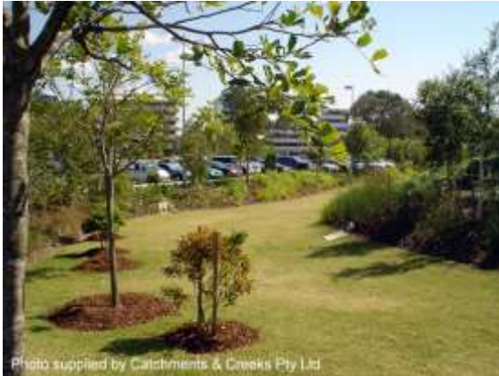
Stormwater detention basin (Qld)
