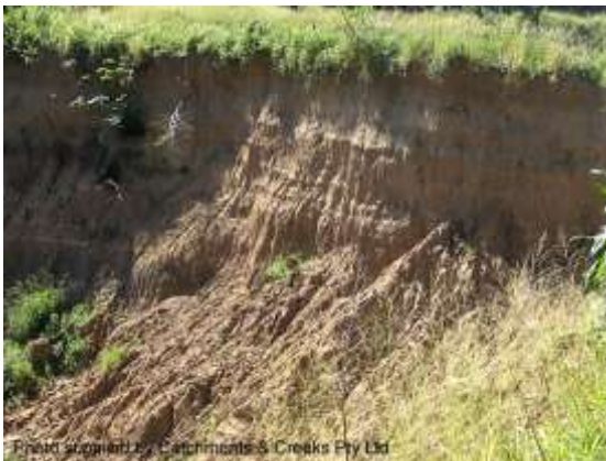
Bank slump (Qld)
