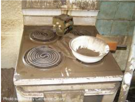
Silt deposited within a flooded home
