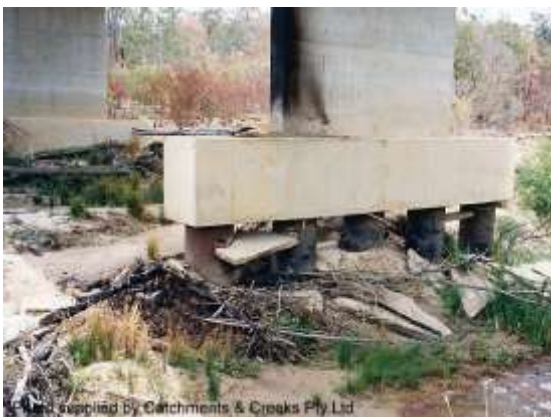
Lowering of a creek bed under a bridge
