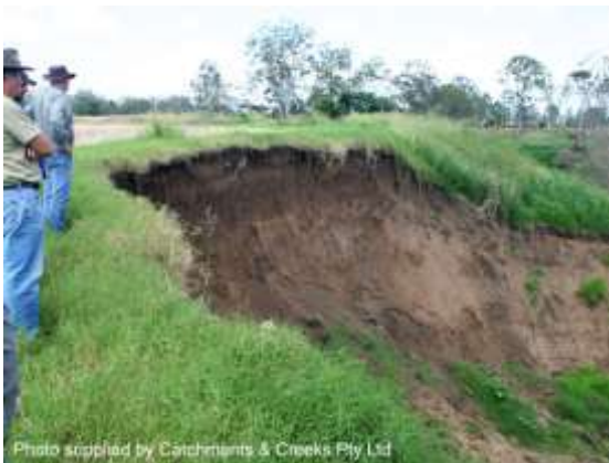
Bank slumping (Qld)
