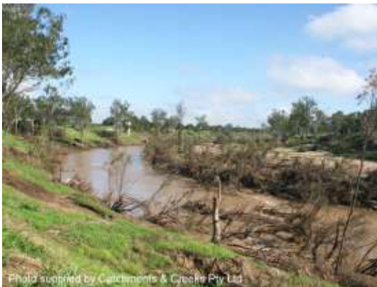
Vegetation damage, Brisbane River, 2011
