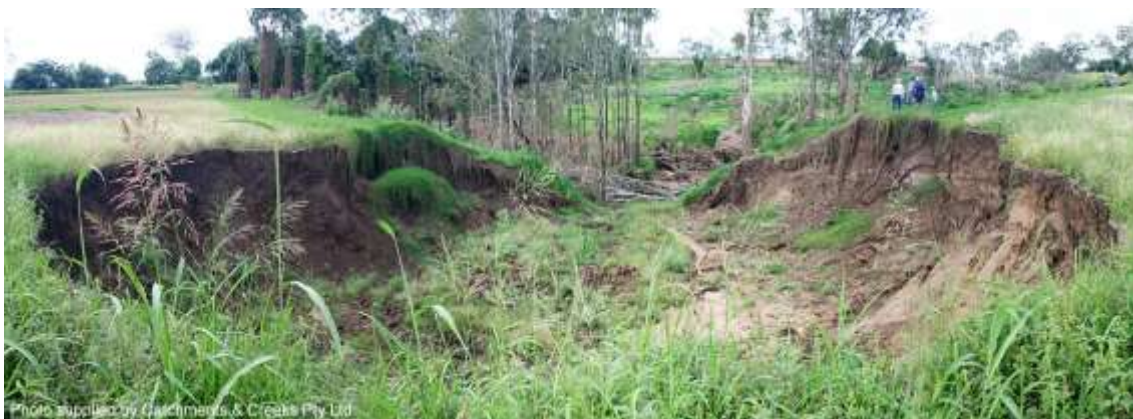
Post-flood, slip circle bank slump, Lockyer Creek, Queensland, 2011
