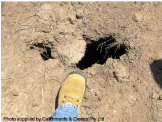
Deep rilling and tunnel erosion (Qld)
