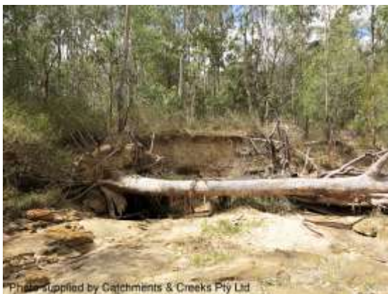
Tree falls after bank undercutting
