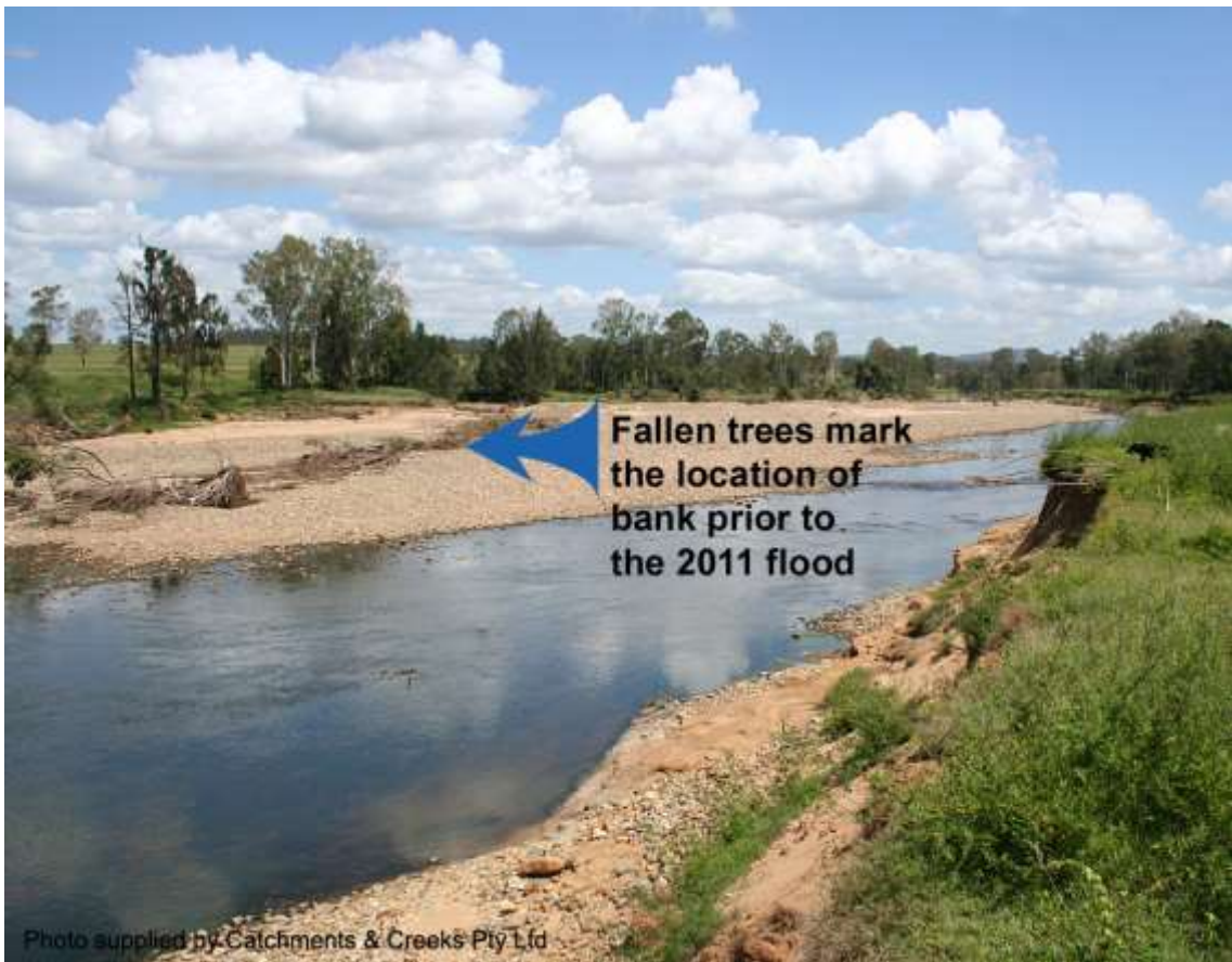
Buaraba Creek, Buaraba, Queensland (2011 flood damage)
