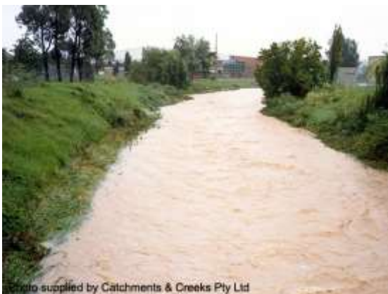
Constructed drainage channel (NSW)
