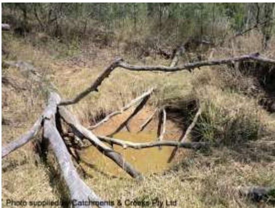
Scour hole within an overland flow path
