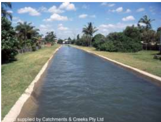
High tide backing-up into a coastal drain
