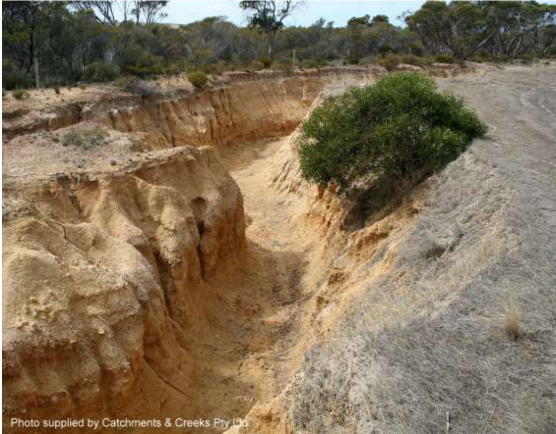
Gully erosion within a dispersive soil, Port Lincoln, South Australia
