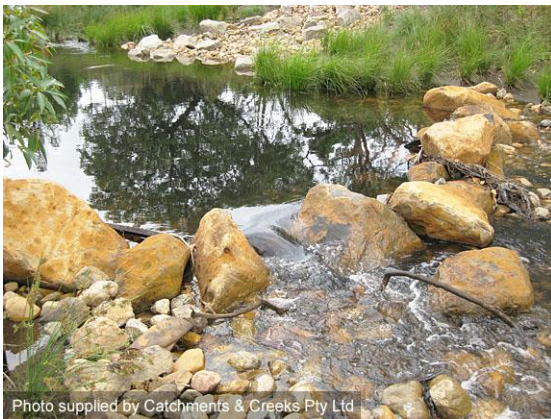
Constructed rock weir (Qld)
