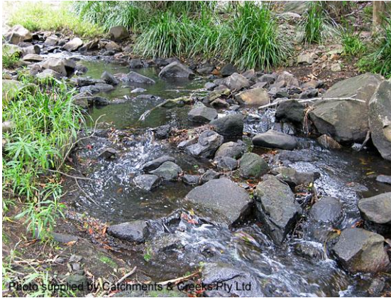
Photo supplied by Catchments & Creeks Pty Ltd Constructed riffle in a clay-based creek
