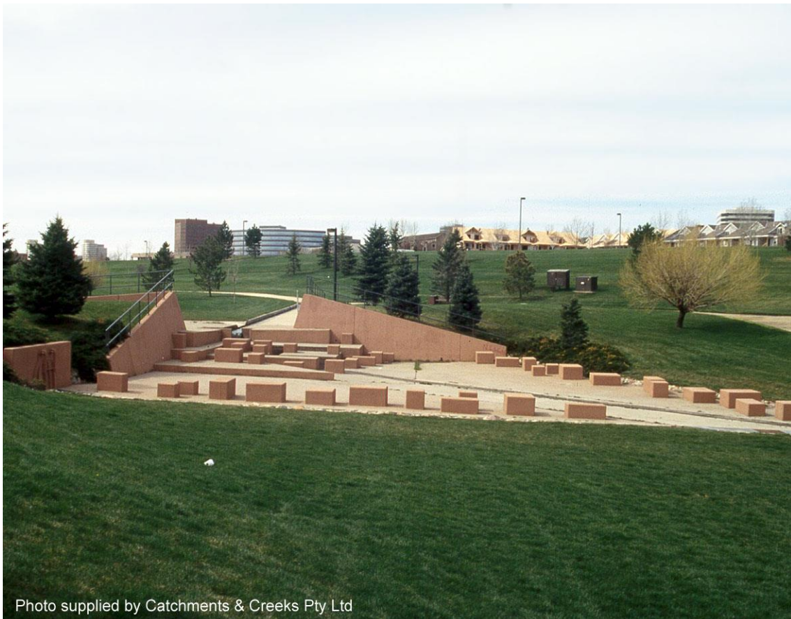
Decorative drop structure with energy dissipation blocks (Denver, Colorado, USA)
