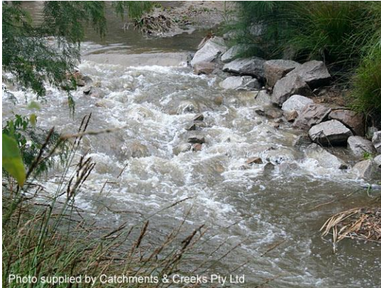
Flow over a constructed riffle (Qld)
