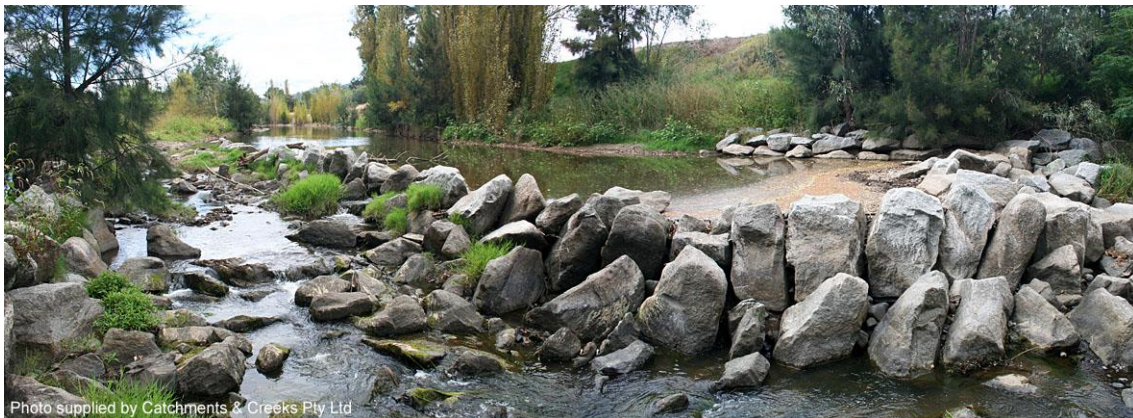
Rock ramp fishway looking upstream from the base of the fishway (Tamworth)
