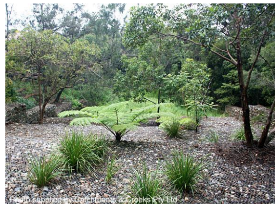
Same stepped gabion spillway (2010)
