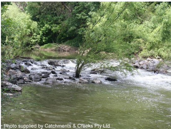
Constructed rock ramp/chute (NSW)
