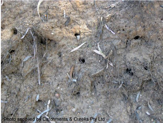
Bird nests in an eroded creek bank (Qld)
