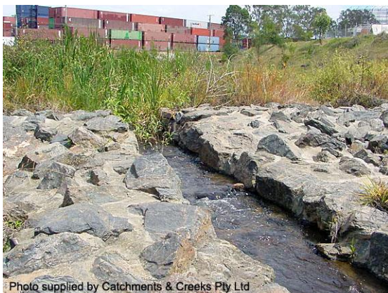
Concrete-grouted low-flow channel (QLD)
