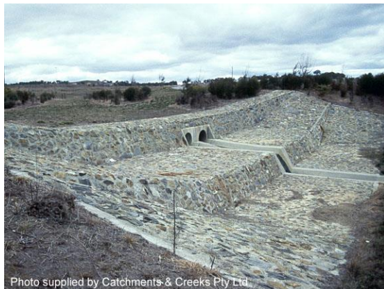
Grouted rock stepped drop structure (ACT)
