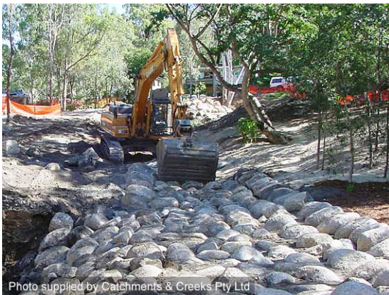
Rock-lined batter chute (Qld)
