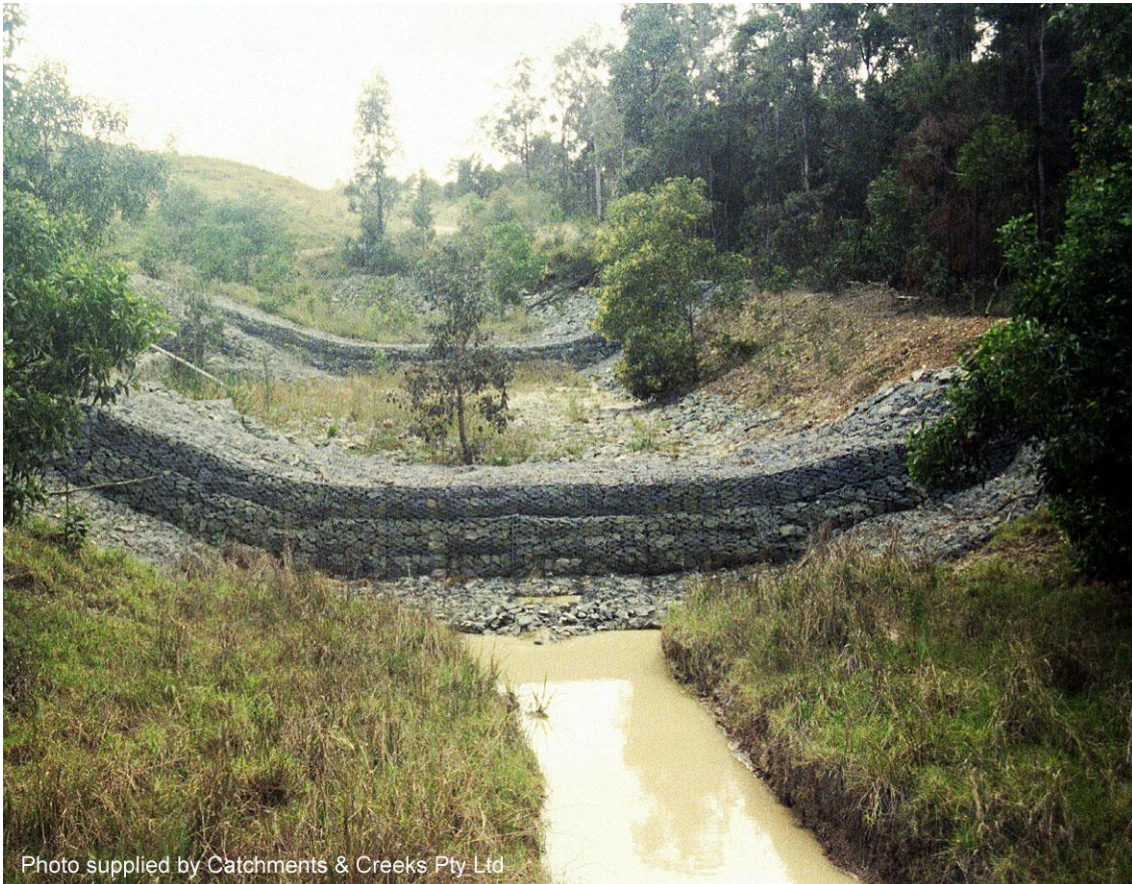
Gabion drop structures (Qld)
