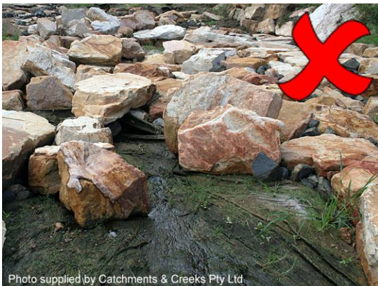
Single layer of rock on filter cloth
