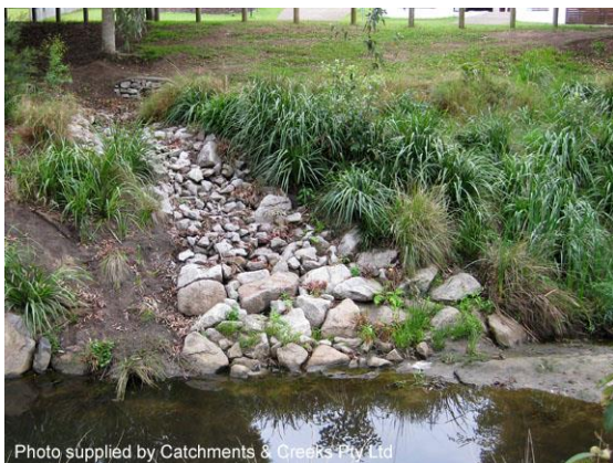
Stormwater inflow 'batter chute' (Qld)
