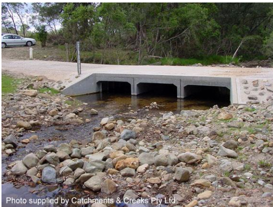
Stabilised drop-inlet at a road culvert
