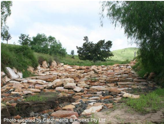
Rock chute stabilising gully erosion (Qld)
