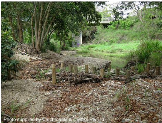
Logs trimmed to a suitable height (Qld)
