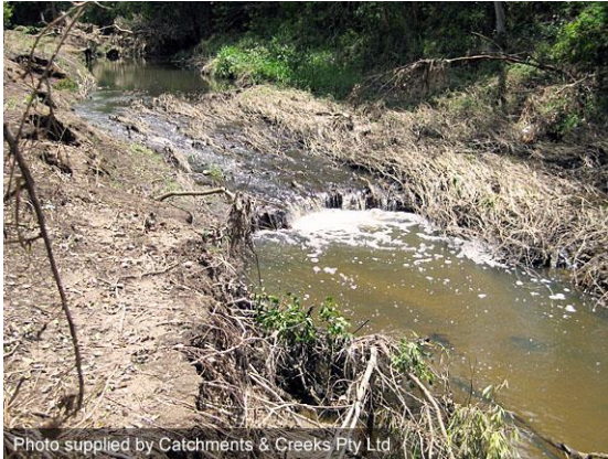
Head-cut erosion (Qld)
