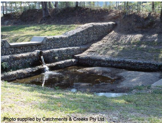
Gabion drop structure (Qld)
