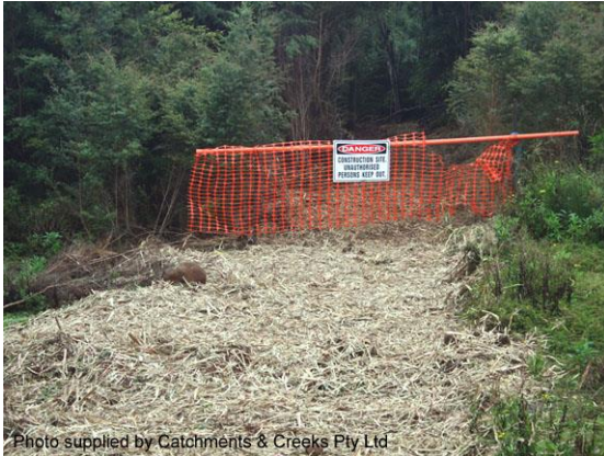
Restoration of a site access pathway
