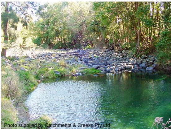
Pool downstream of a rock ramp (NSW)
