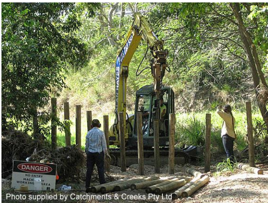
Driving piles into the sand bed (Qld)
