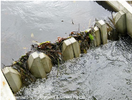
Debris blockage of fishway (Qld)
