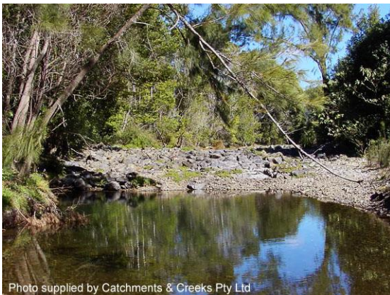
Pool downstream of a rock chute (NSW)
