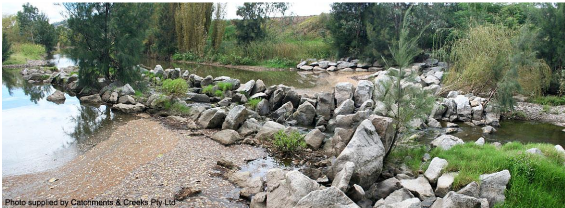
Rock ramp fishway viewed from the right bank (Tamworth)
