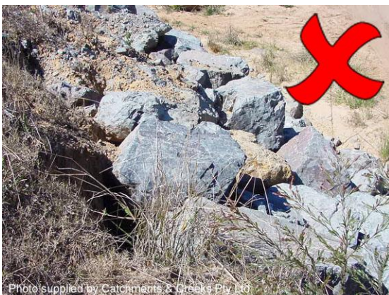
Erosion under rocks on a dispersive soil
