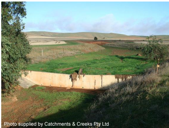
Vertical drop structure (SA)
