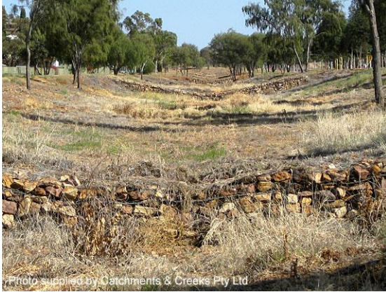
Photo supplied by Catchments & Creeks Pty Ltd Several gabion drop structures (NT)
