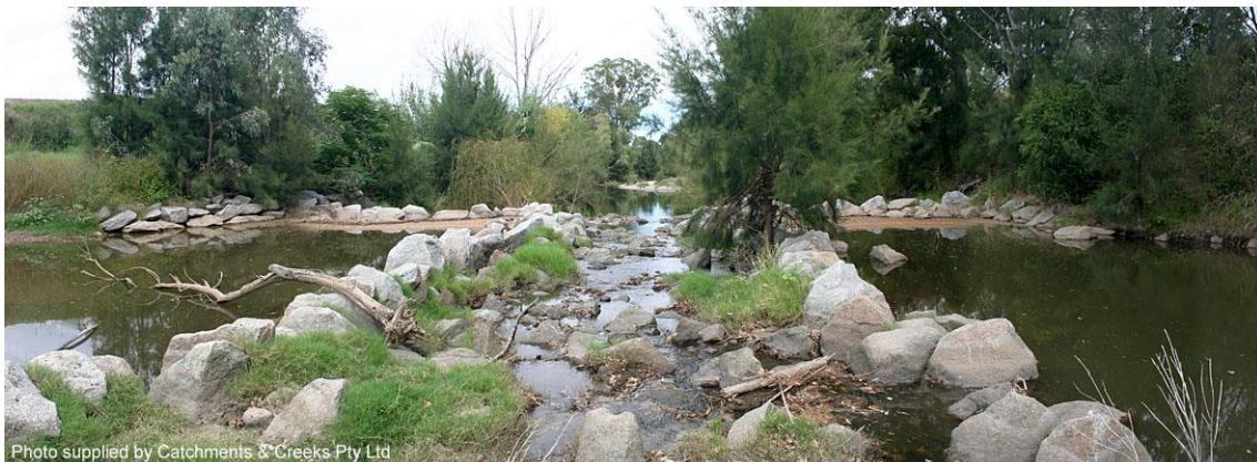
Rock ramp fishway looking downstream from the top of the fishway (Tamworth)
