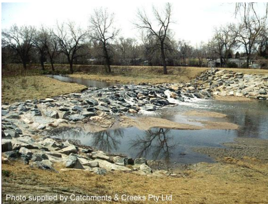
Grouted rock drop structure (USA)
