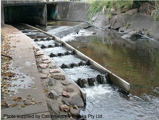
Precast concrete fishway (Qld)
