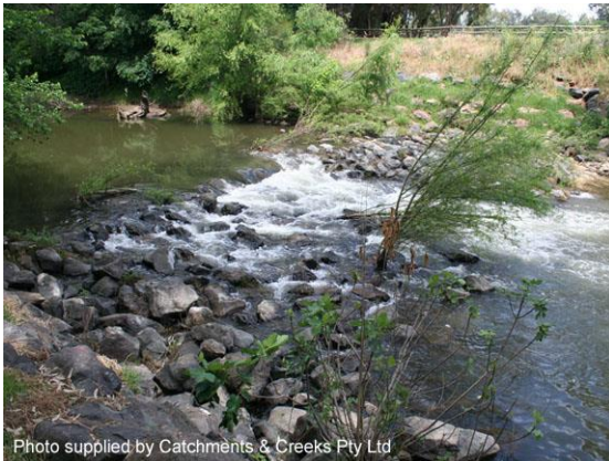
Constructed riffle (NSW)
