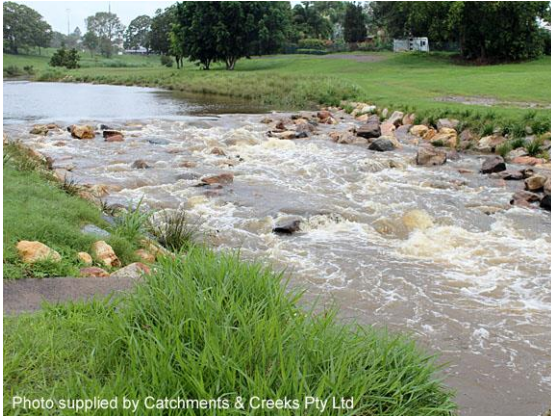
Constructed riffle (Qld)
