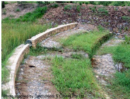
Stepped gabion drop structure (Qld)
