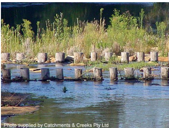
Pile field (Vic)
