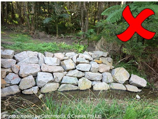
Open-void rock work can attract weeds
