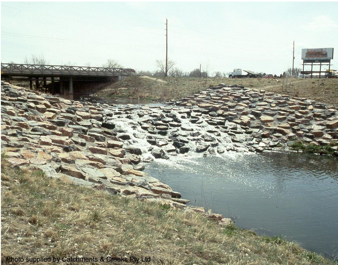
Grouted rock drop structure (Denver, Colorado, USA)
