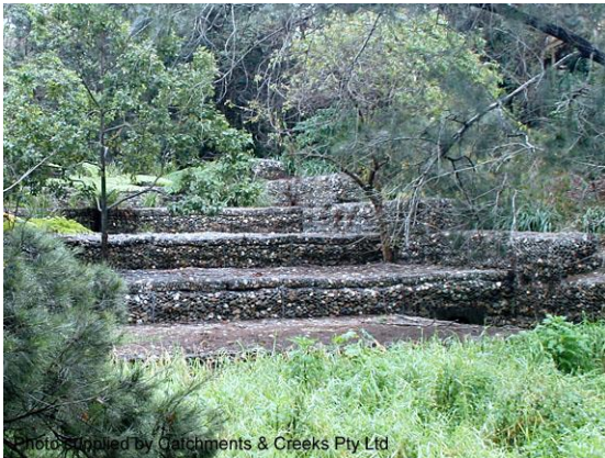
Photo supplied by Catchments & Creeks Pty Ltd Stepped gabion spillway (Qld)
