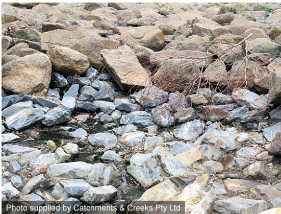
Rock filter layer (blue) under surface rock
