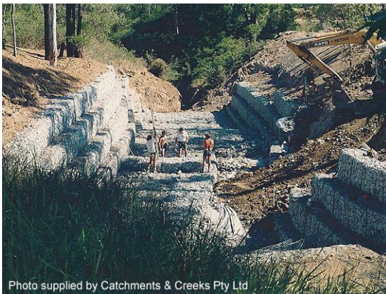
Gabion-lined channel in construction (Qld)
