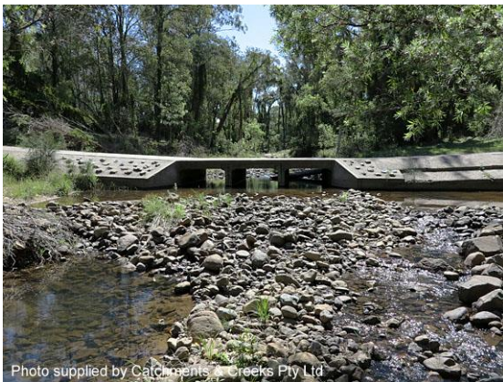
Stabilised outlet pool at a road culvert
