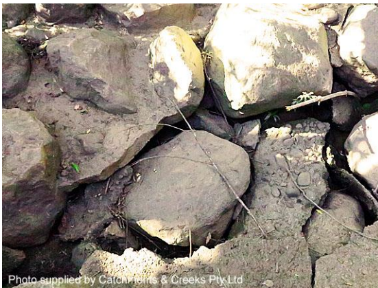
Failed grouted rock (Qld)
