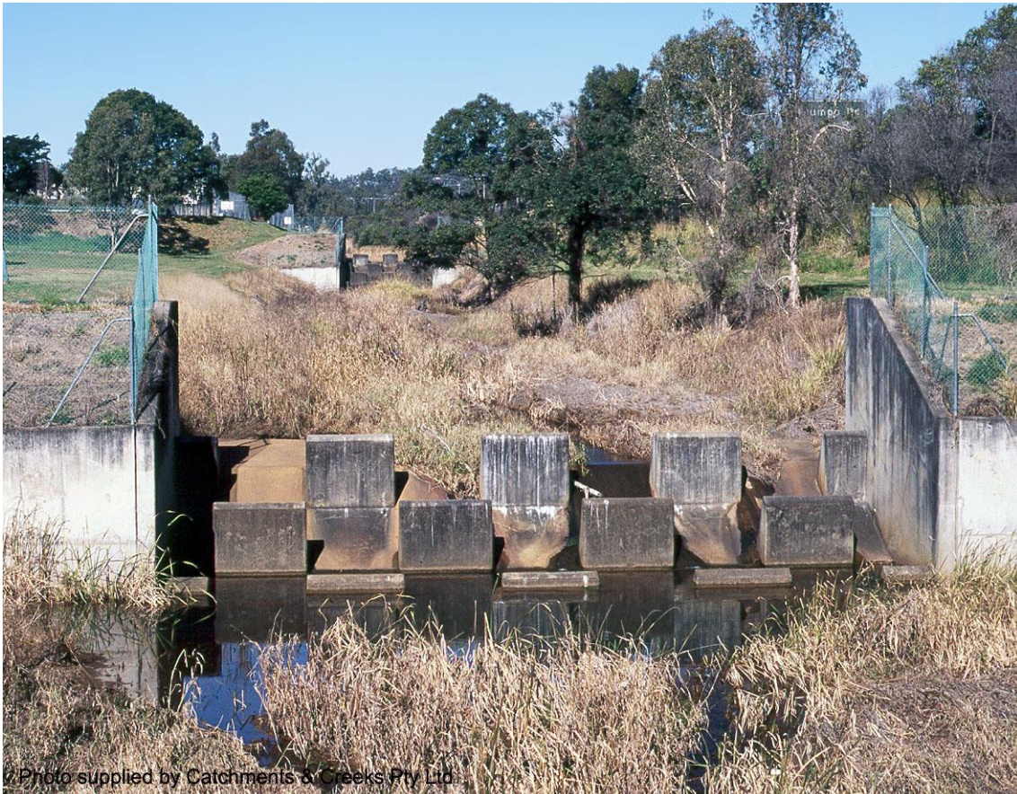
Baffled drop structure (Qld)
