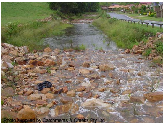
Constructed stormwater channel (Qld)
