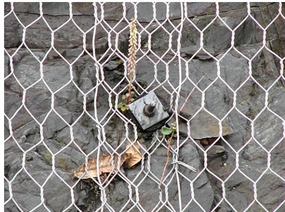
Rockfall netting (anchored to rock)
