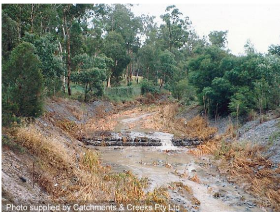
Gabion-lined drainage channel (Qld)
