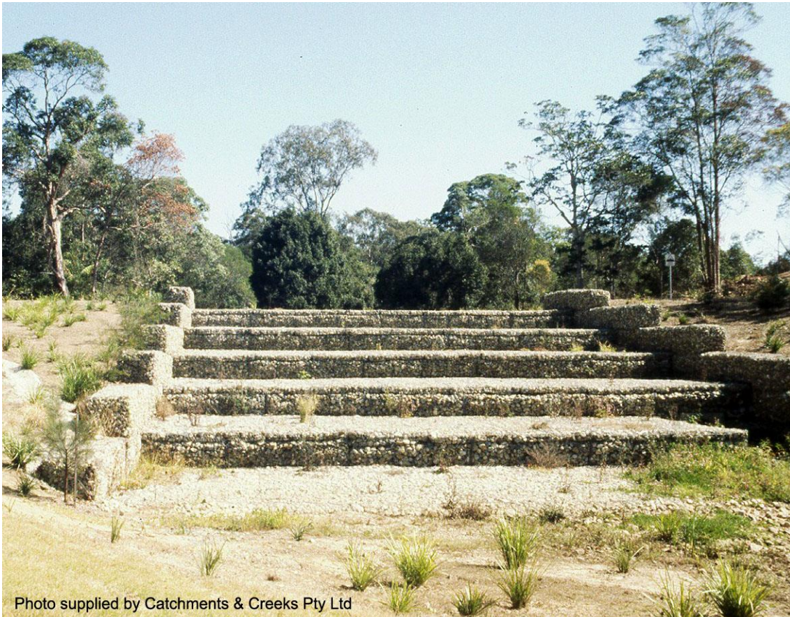
Stepped, gabion spillway (Qld)
