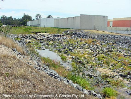
Energy dissipation basin at base of chute
