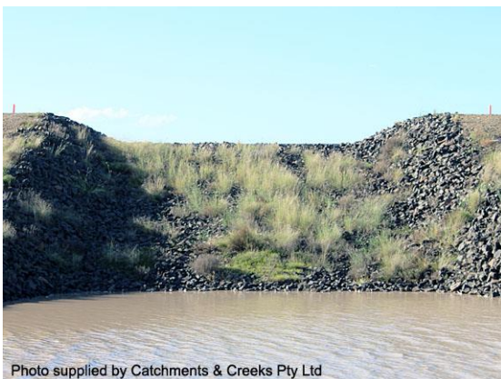
Rock-lined spillway (Qld)
