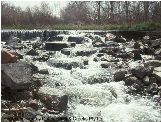
Photo supplied by Catchments & Creeks Pty Ltd Drop structure fishway (USA)
