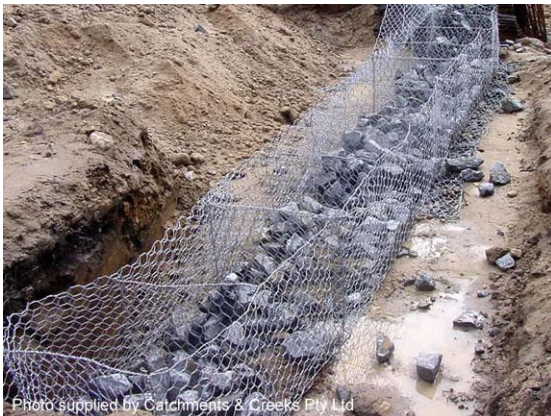
Gabions (during construction)
