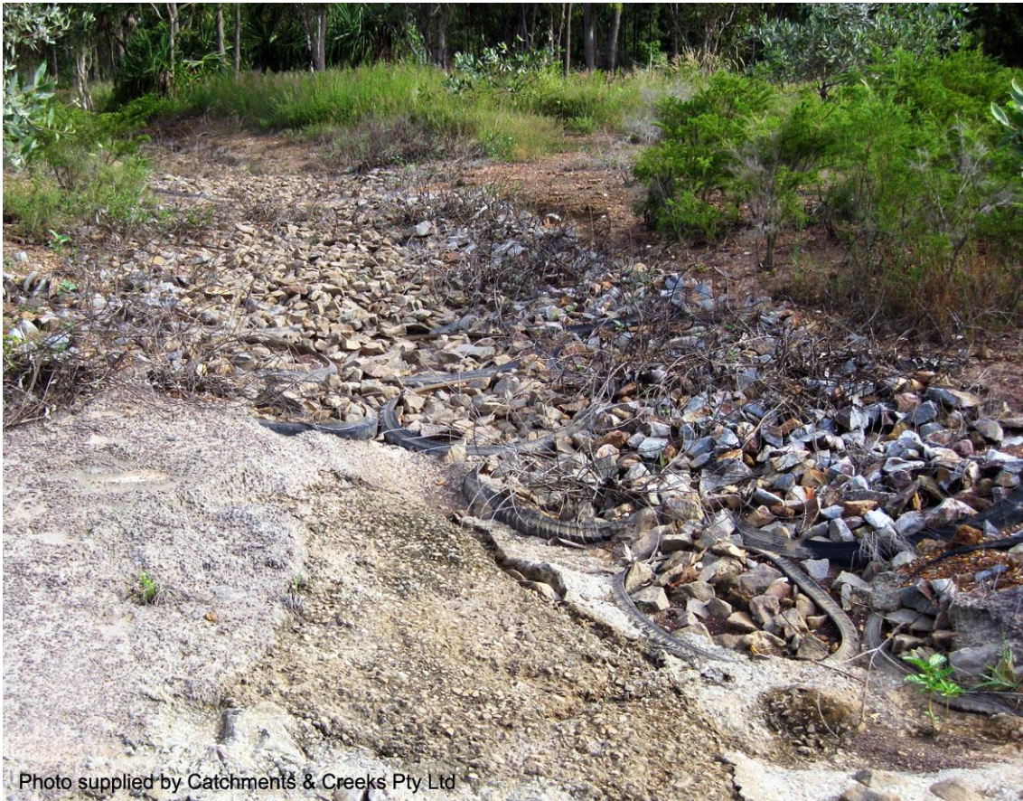
Rock and tyre chute (NT)
