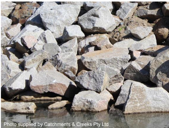
Fractured rock (Qld)
