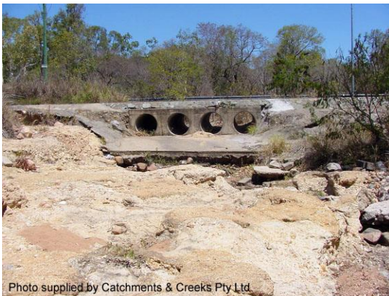
Potential site for a ridge rock ramp (Qld)
