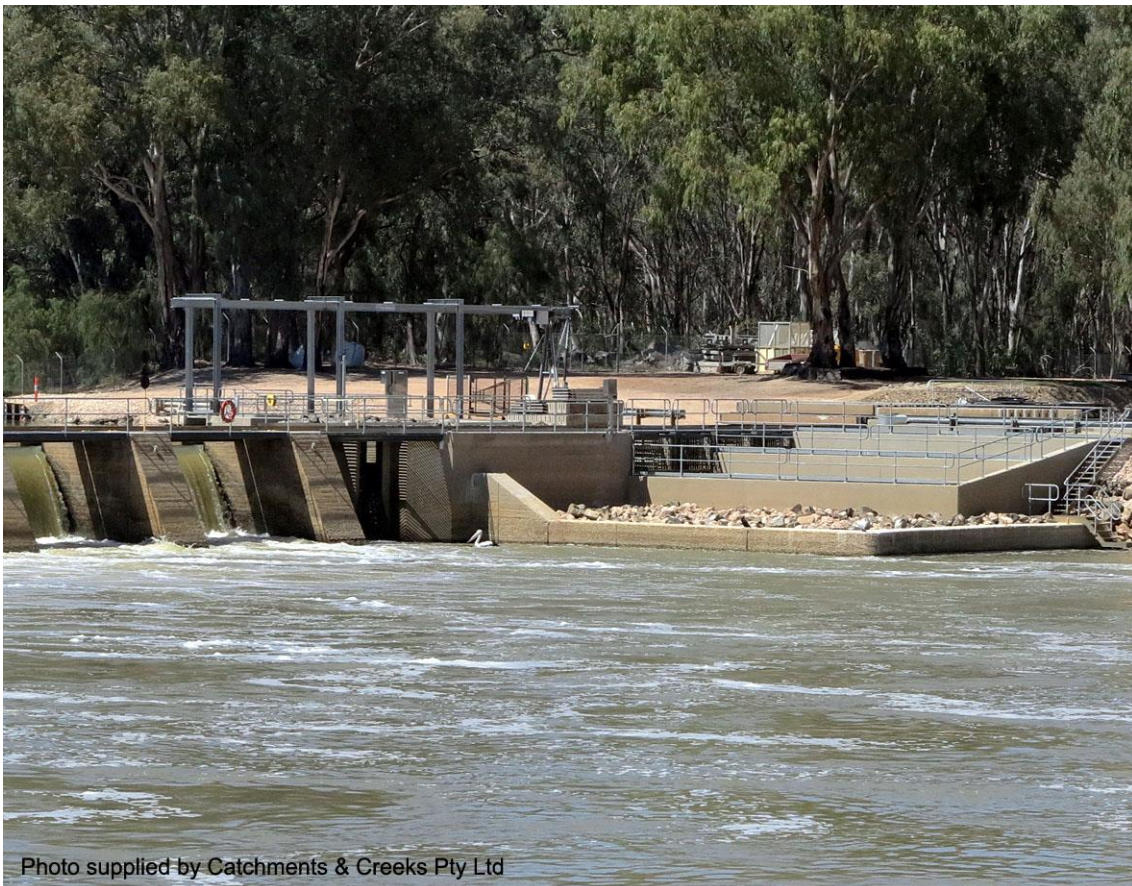
Bypass fishway, Lock No. 10, Murray River, Victoria
