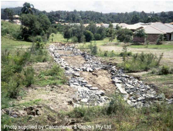
Recessed rock check dams (Qld)
