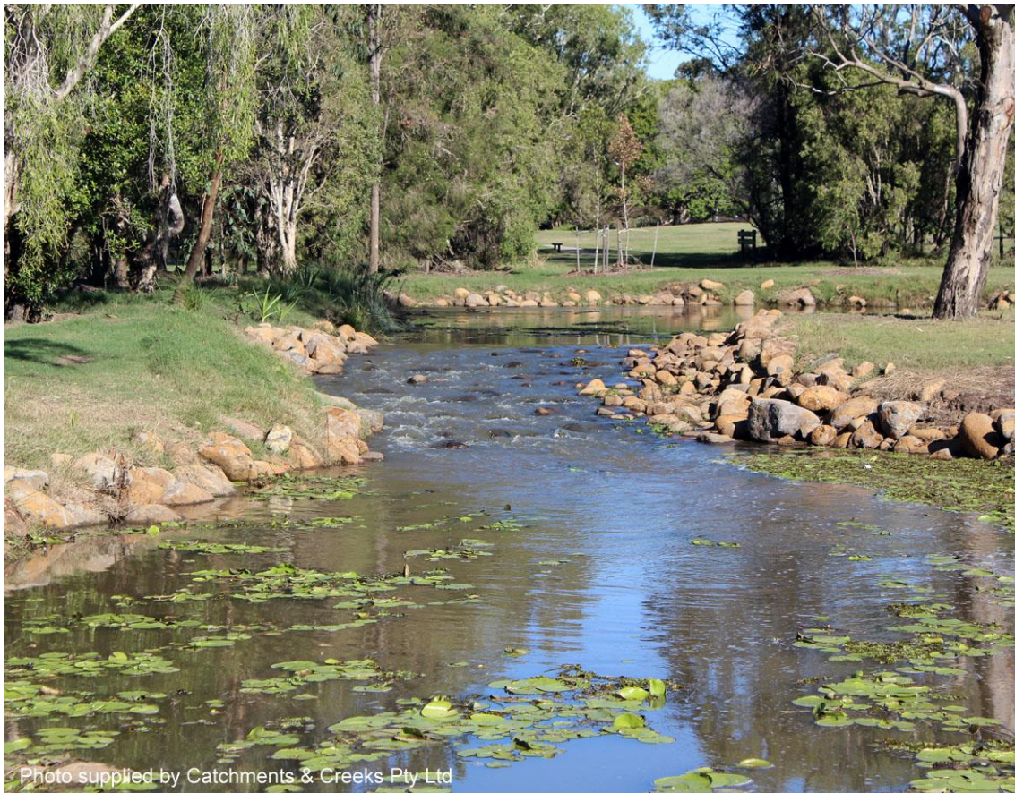
Riffle zone with a bypass fishway channel, Bundaberg, Queensland
