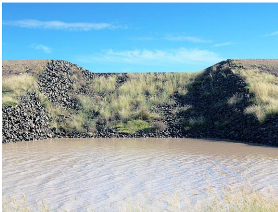
Trapezoidal dam spillway crest (Qld)
