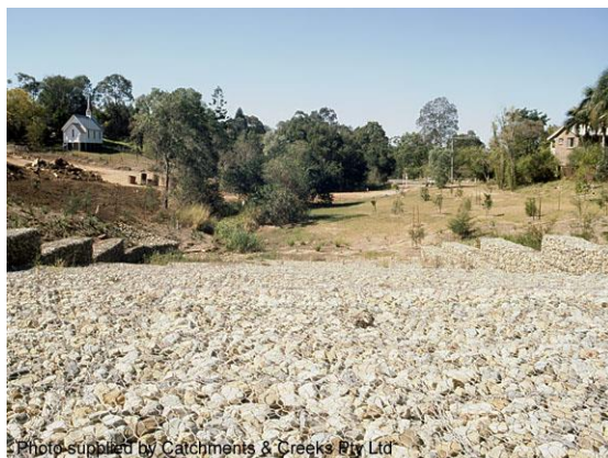
Stepped gabion spillway (1992)
