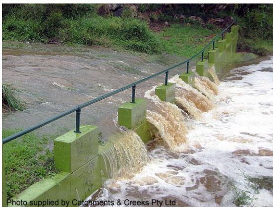
Vertical drop structure (Qld)
