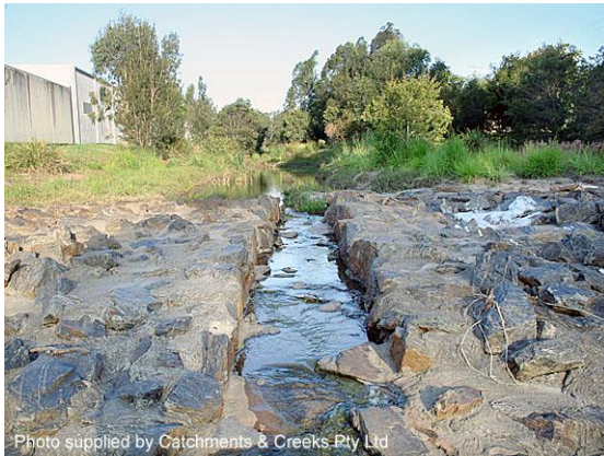
Low-flow channel cut through weir crest
