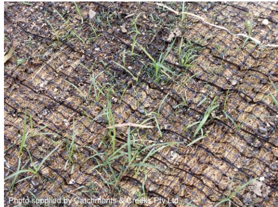
Erosion control mat (composite material)
