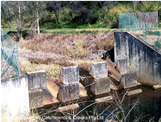
Baffled drop structure (Qld)
