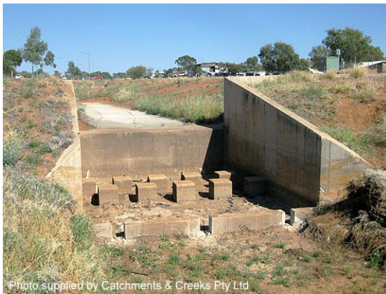
Vertical, baffled drop structure (NT)
