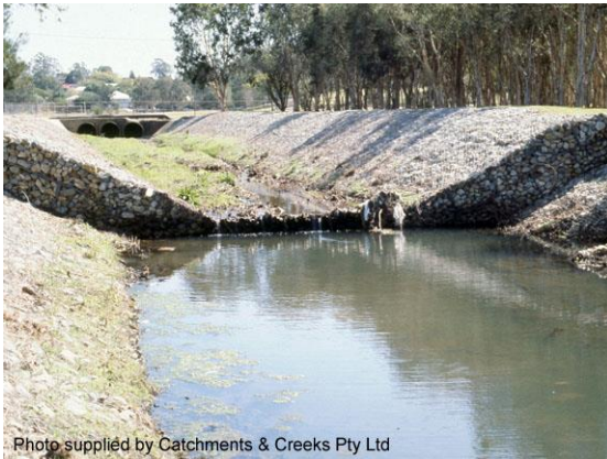
Gabion channel and drop structure
