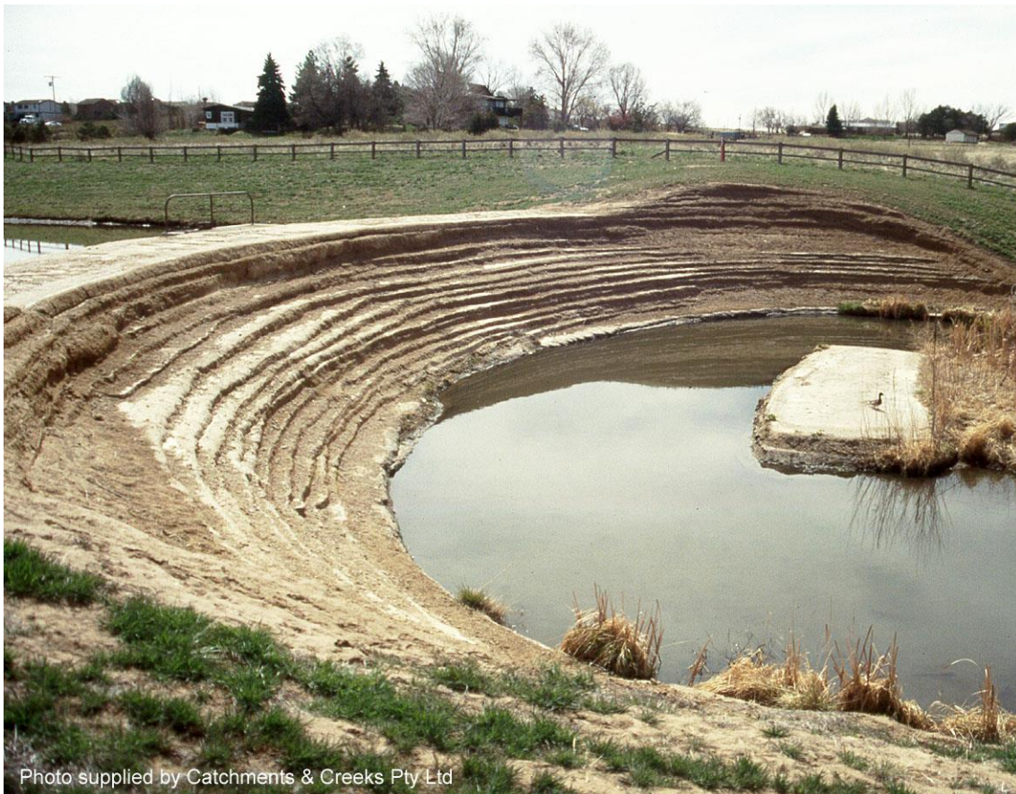
Soil-cement drop structure (Denver, Colorado, USA)
