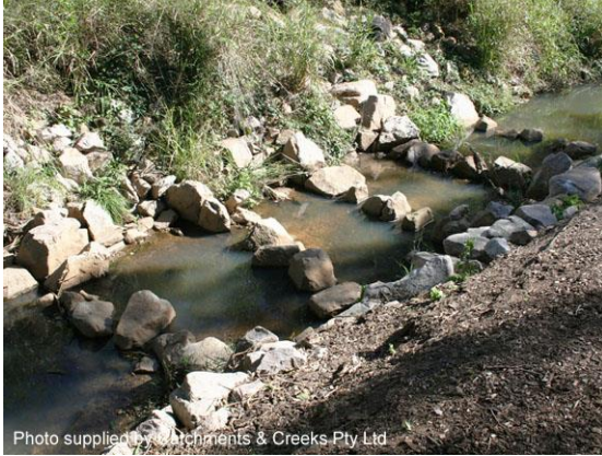
Ridge rock ramp (Qld)
