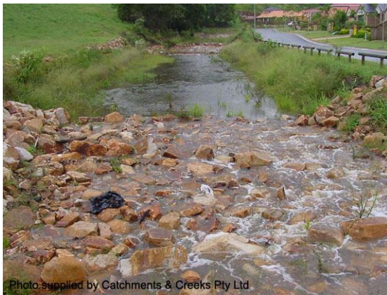
Constructed riffle (Qld)
