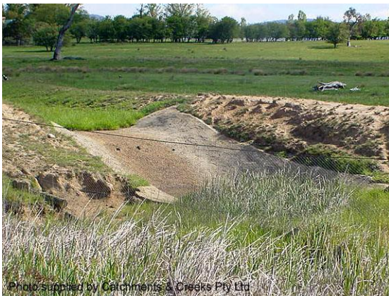
Concrete chute (NSW)
