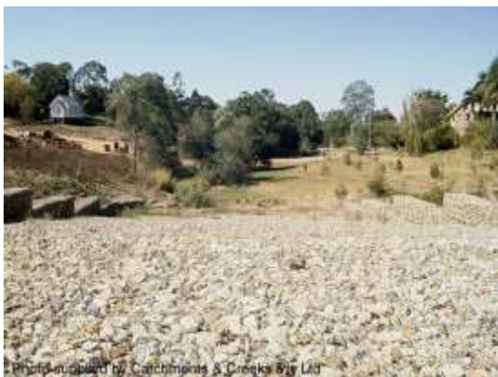
Stepped gabion spillway (1992)
