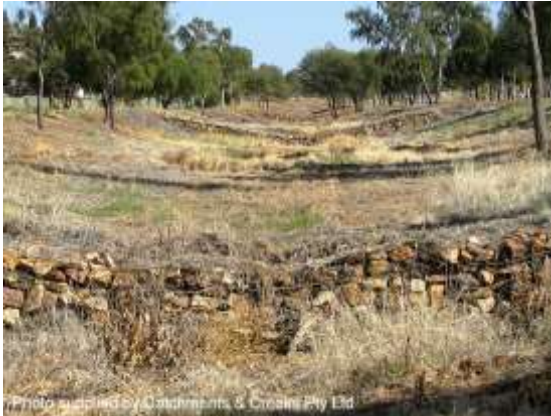
Several gabion drop structures (NT)
