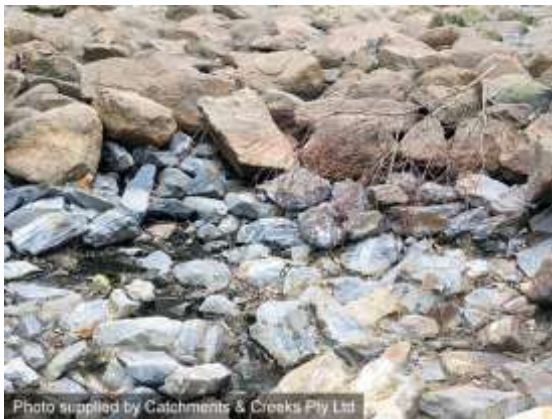
Rock filter layer (blue) under surface rock
