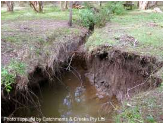
Head-cut erosion (Qld)
