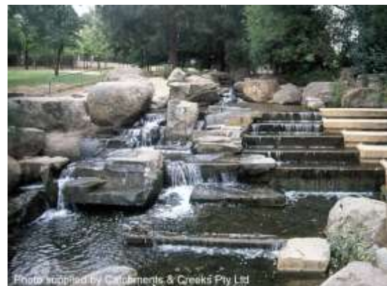
Grouted rock stepped spillway (ACT)
