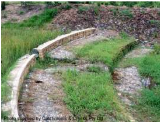
Stepped gabion drop structure (Qld)
