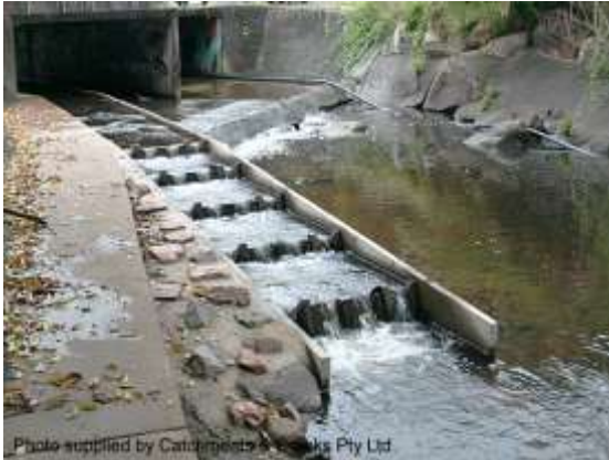
Precast concrete fishway (Qld)
