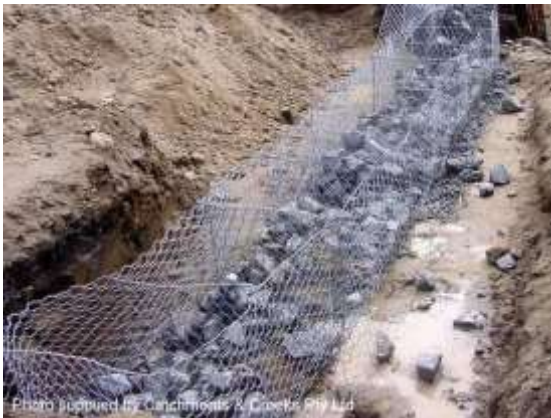
Gabions (during construction)
