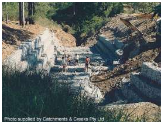
Gabion-lined channel in construction (Qld)
