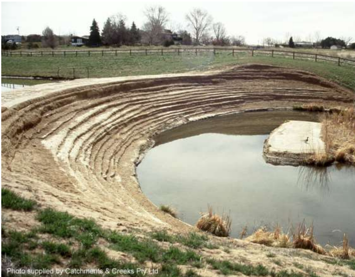
Soil-cement drop structure (Denver, Colorado, USA)
