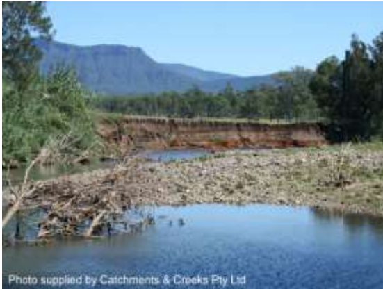
Natural creek erosion (Qld)
