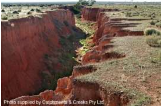
Extreme effects of a lowering gully bed
