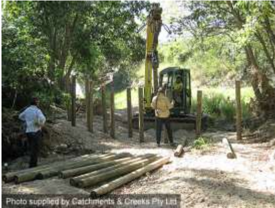
Initial placement of logs (Qld)
