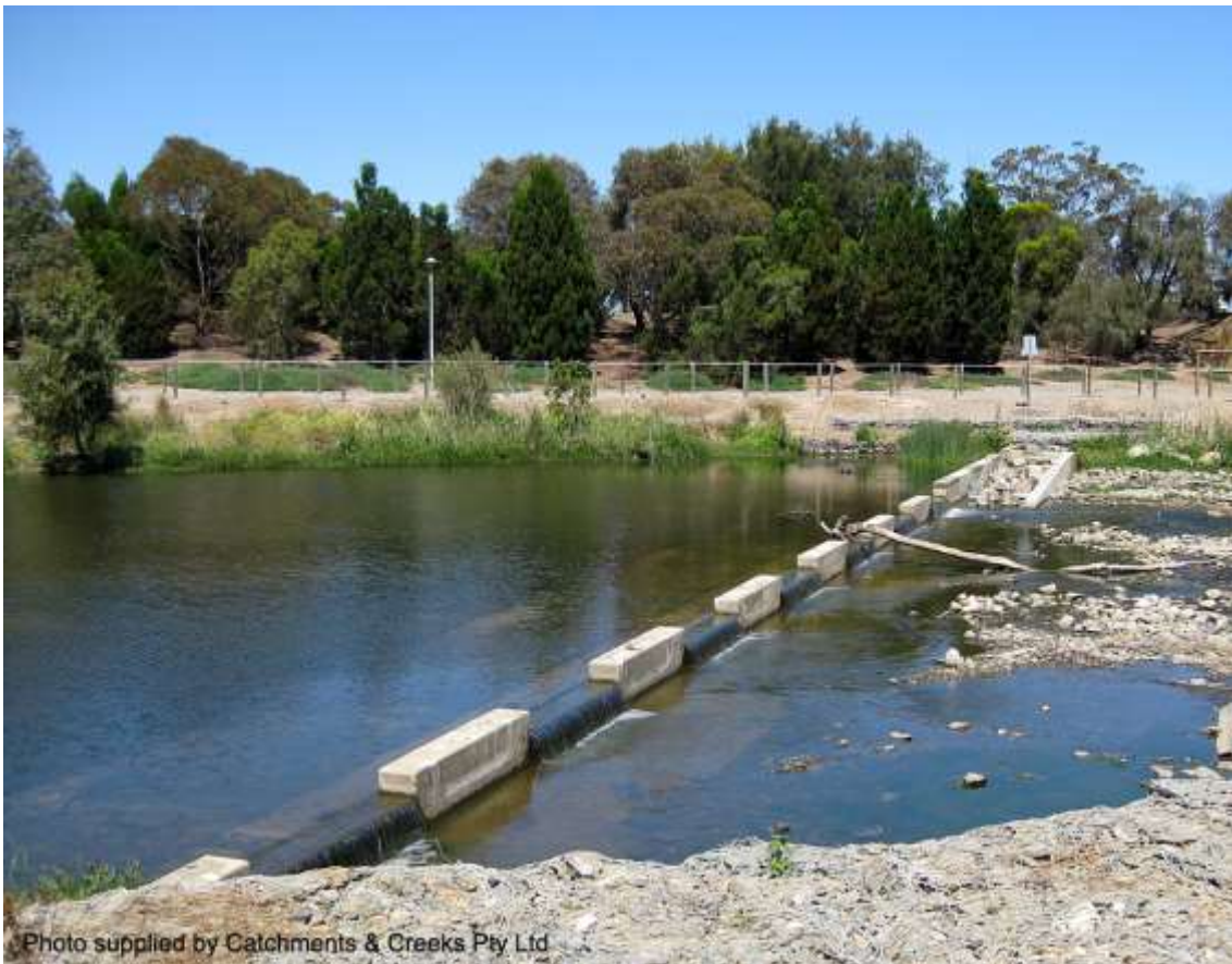
Concrete weir with fishway (Torrens River, SA)
