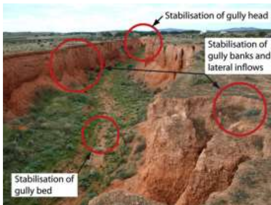
Treatment of gully erosion (SA)
