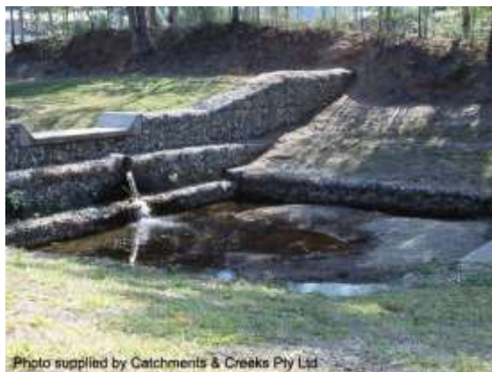
Gabion drop structure (Qld)
