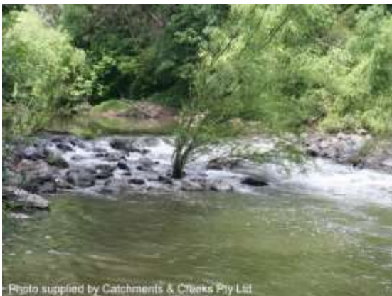
Constructed rock ramp/chute (NSW)
