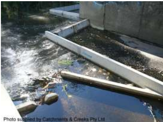
Upstream end of fishway (Qld)
