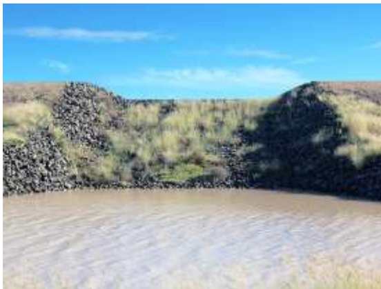
Trapezoidal dam spillway crest (Qld)
