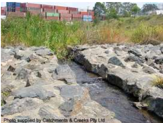
Low-flow channel set in grouted rock
