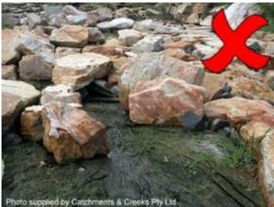
Single layer of rock on filter cloth
