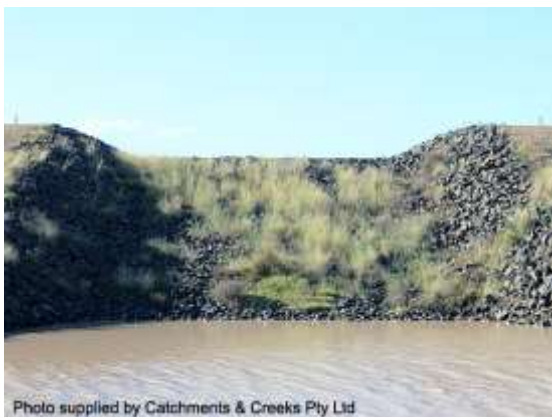
Rock-lined spillway (Qld)
