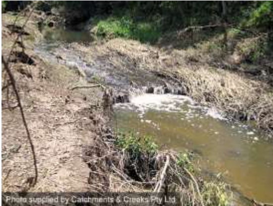
Head-cut erosion (Qld)
