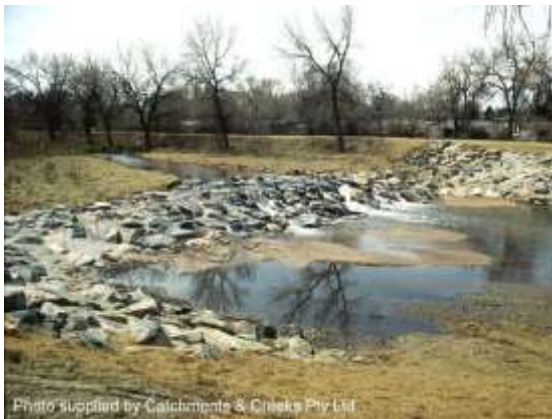
Grouted rock drop structure (USA)
