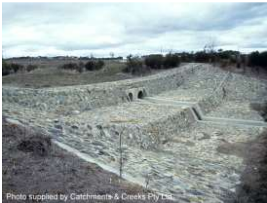
Grouted rock stepped drop structure (ACT)
