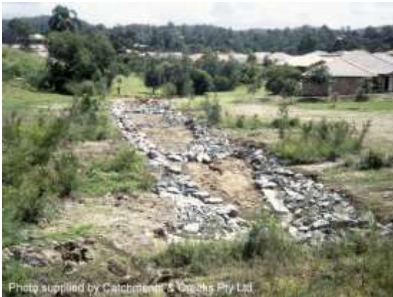
Recessed rock check dams (Qld)
