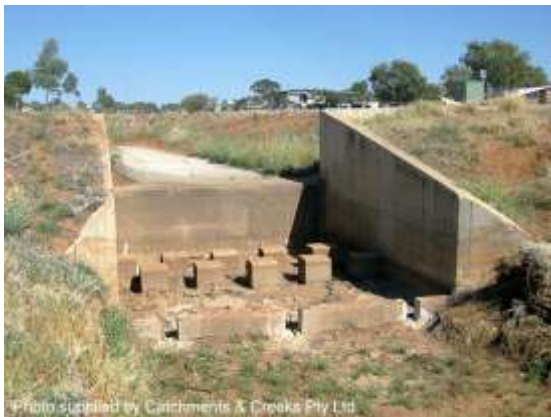
Vertical, baffled drop structure (NT)
