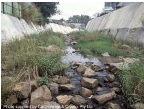
Rocks grouted to concrete channel (Qld)
