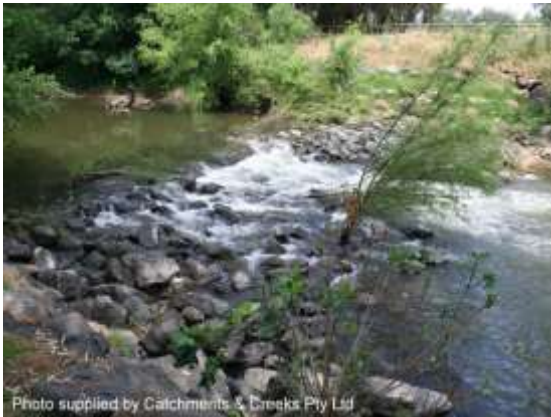
Constructed riffle (NSW)
