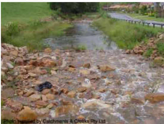
Constructed stormwater channel (Qld)
