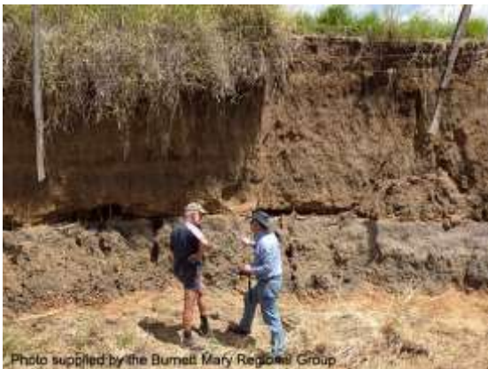
Bank undercutting (Qld)
