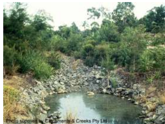
Example of constructed plunge pool
