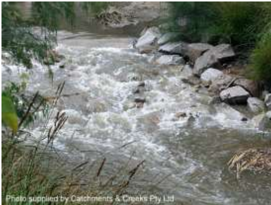
Constructed rock chute (Qld)
