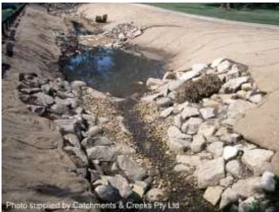
Constructed pool-riffle system (Qld)
