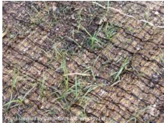
Erosion control mat (composite material)
