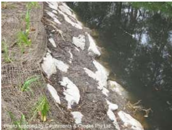
Voids filled with soil prior to planting (Qld)
