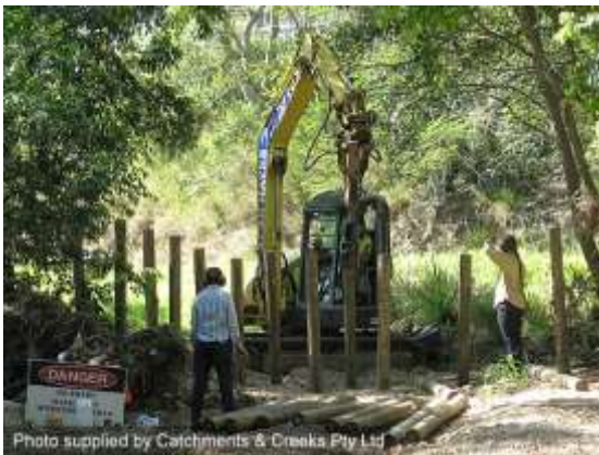
Driving piles into the sand bed (Qld)
