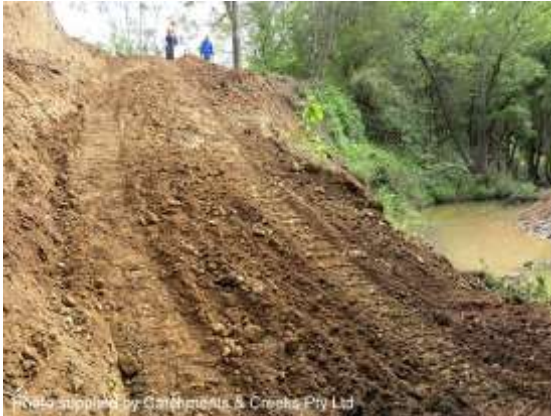
Access ramp cut down a creek bank (Qld)
