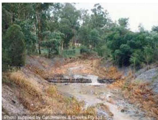
Gabion-lined drainage channel (Qld)
