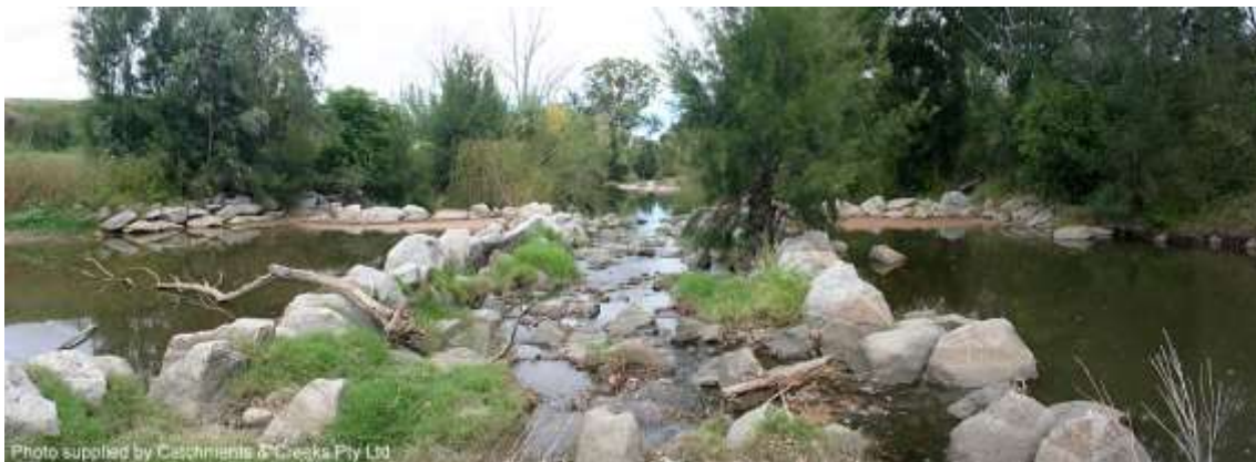
Rock ramp fishway looking downstream from the top of the fishway (Tamworth)
