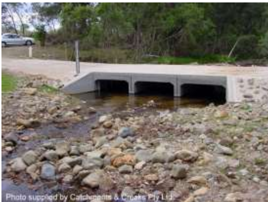
Stabilised drop-inlet at a road culvert
