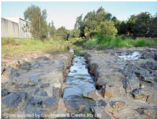
Low-flow channel cut through weir crest
