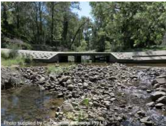
Stabilised outlet pool at a road culvert
