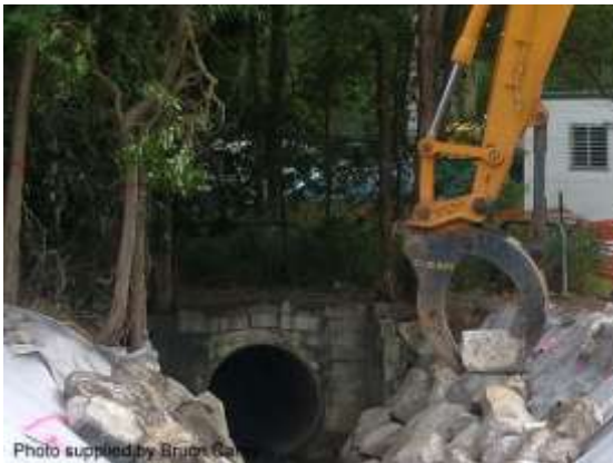
Individual placement of rocks (Qld)
