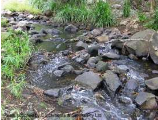
Constructed riffle in a clay-based creek
