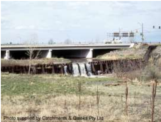
Steel sheet piling drop structure (USA)
