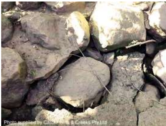
Failed grouted rock (Qld)
