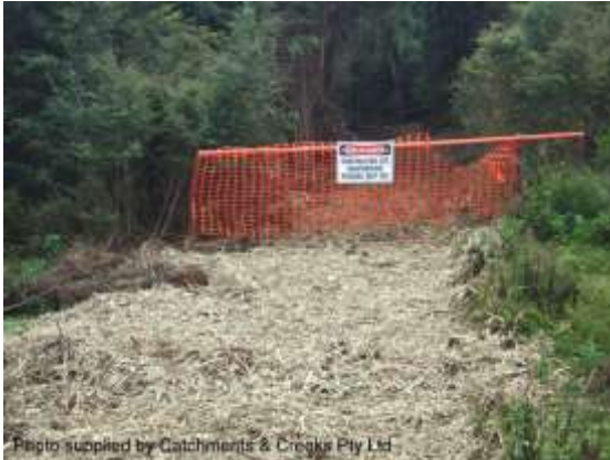
Restoration of a site access pathway
