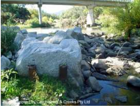
Habitats formed by placement of boulders
