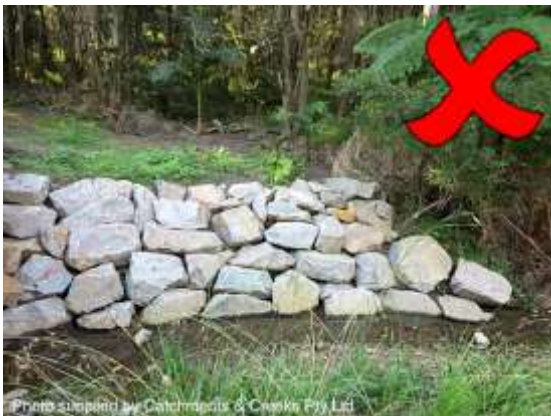
Open-void rock work can attract weeds
