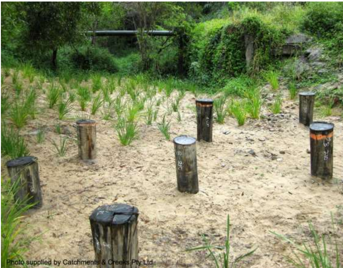
A pile field formed in the bed of a sand-based creek (Qld)
