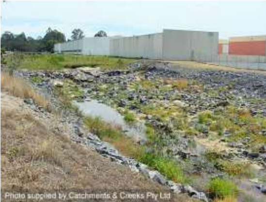
Energy dissipation basin at base of chute
