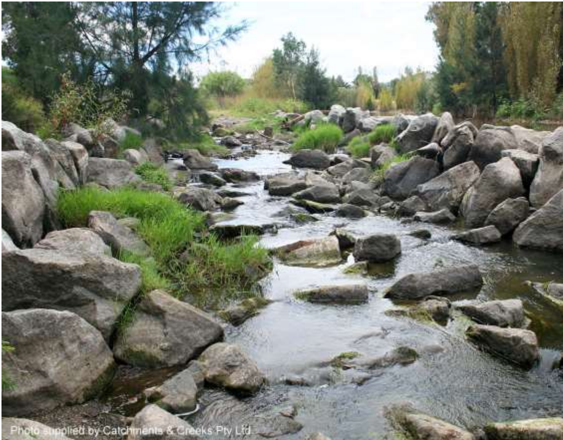
Constructed rock ramp (fishway) in Tamworth, NSW
