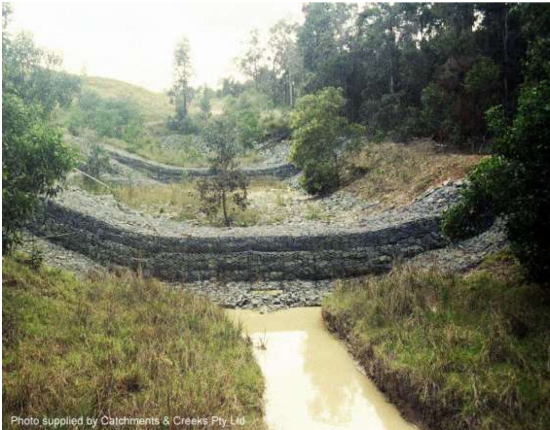
Gabion drop structures (Qld)
