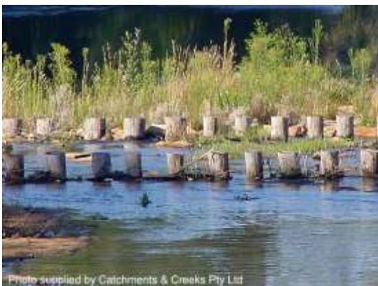
Pile field (Vic)
