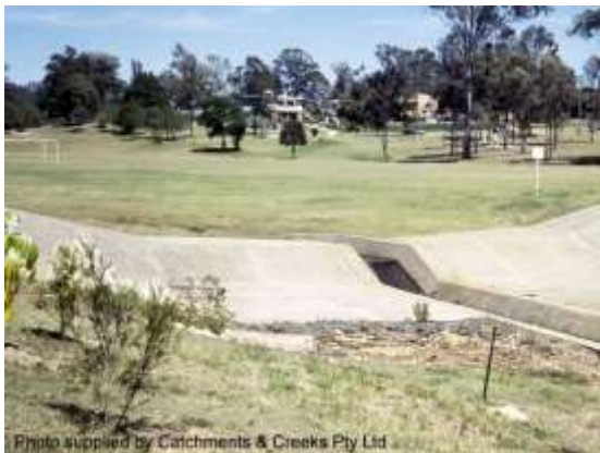
Trapezoidal, inclined drop structure (Qld)
