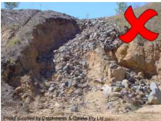
Rocks placed on a dispersive soil
