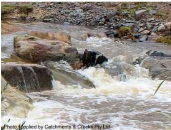
Constructed rock riffle (Qld)
