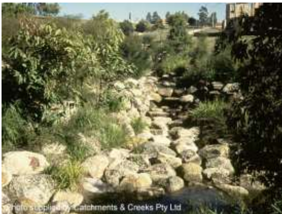
Grouted rock chute (Qld)
