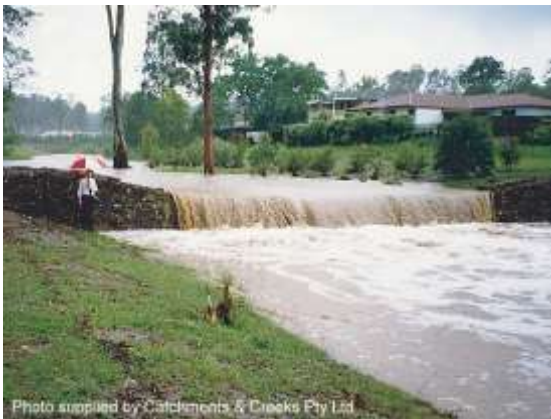
Gabion drop structure (Qld)
