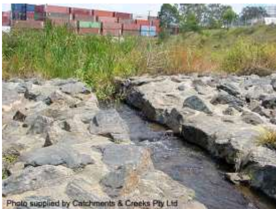
Concrete-grouted low-flow channel (QLD)
