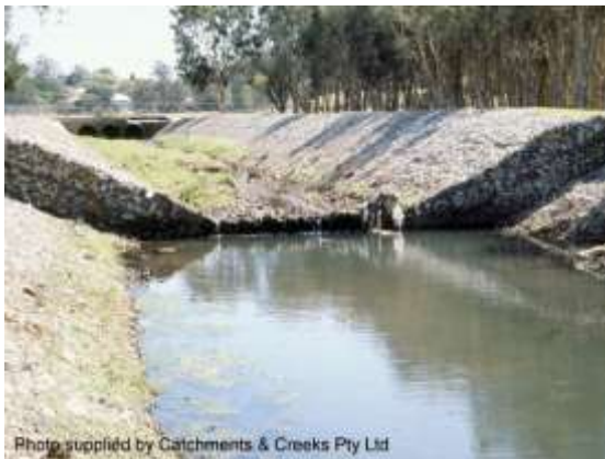
Gabion channel and drop structure
