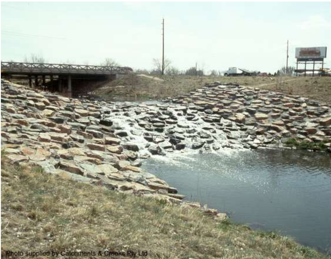
Grouted rock drop structure (Denver, Colorado, USA)
