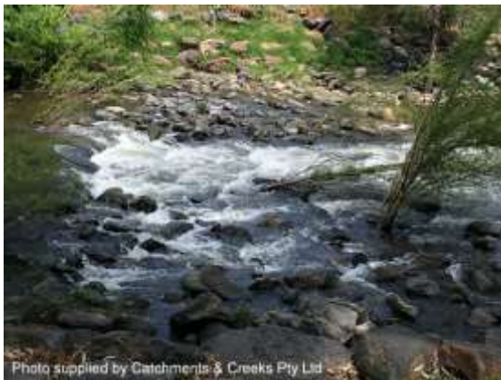
Rock ramp (NSW)
