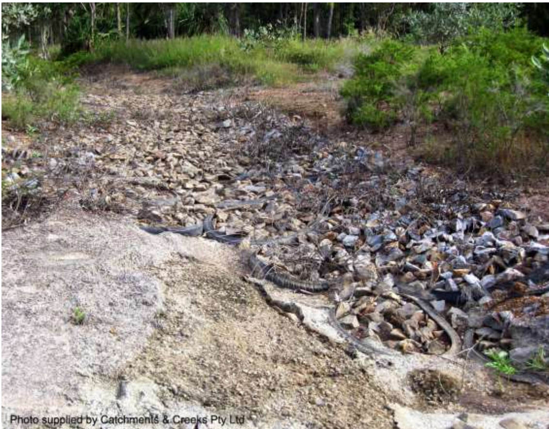
Rock and tyre chute (NT)
