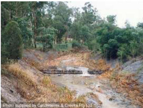
Weed control of rock mattresses (Qld)
