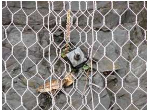
Rockfall netting (anchored to rock)
