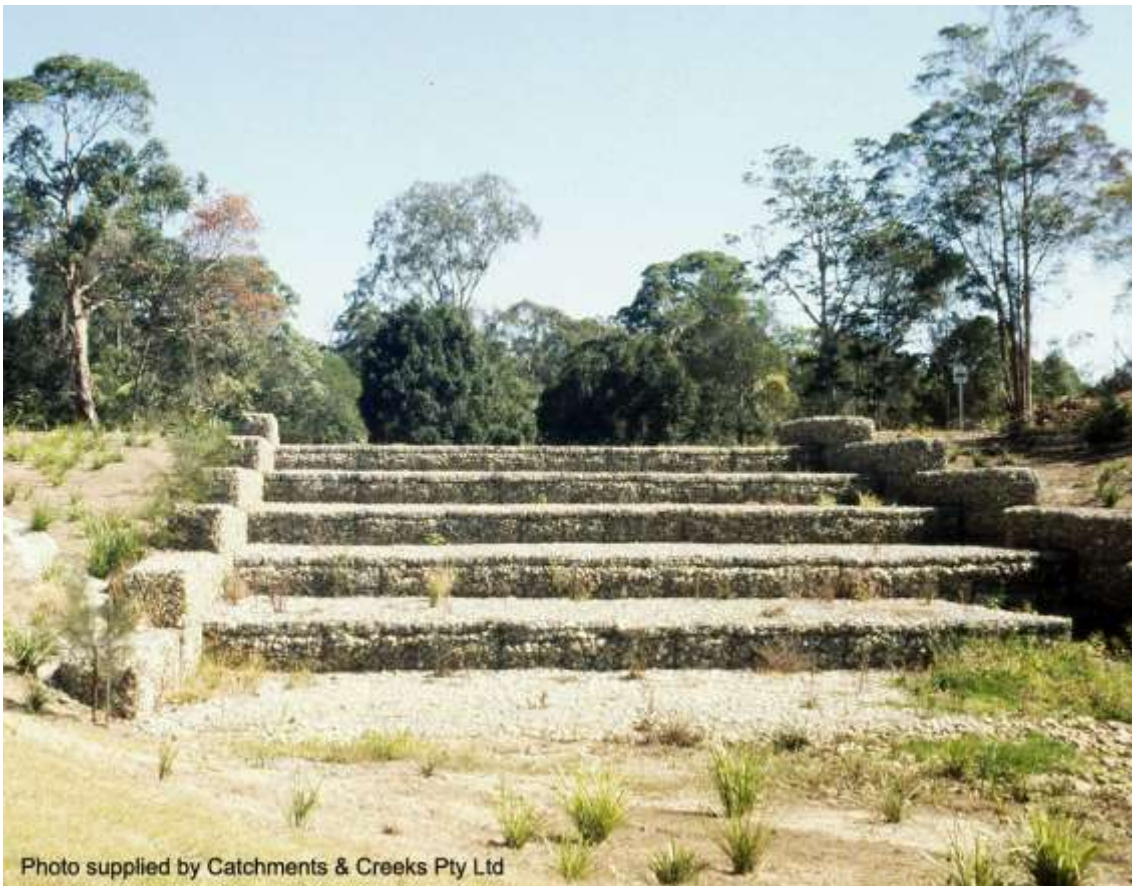
Stepped, gabion spillway (Qld)
