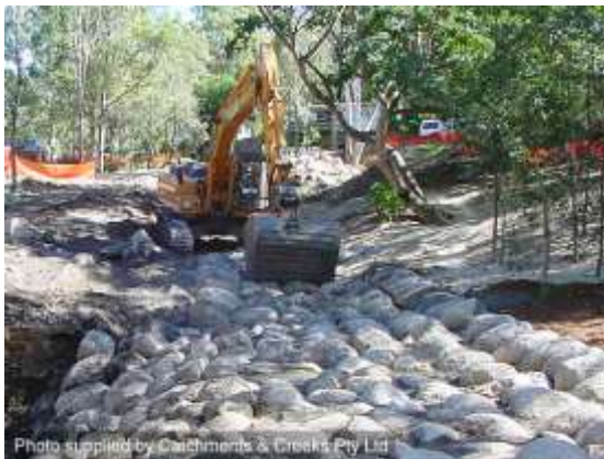
Rock-lined batter chute (Qld)
