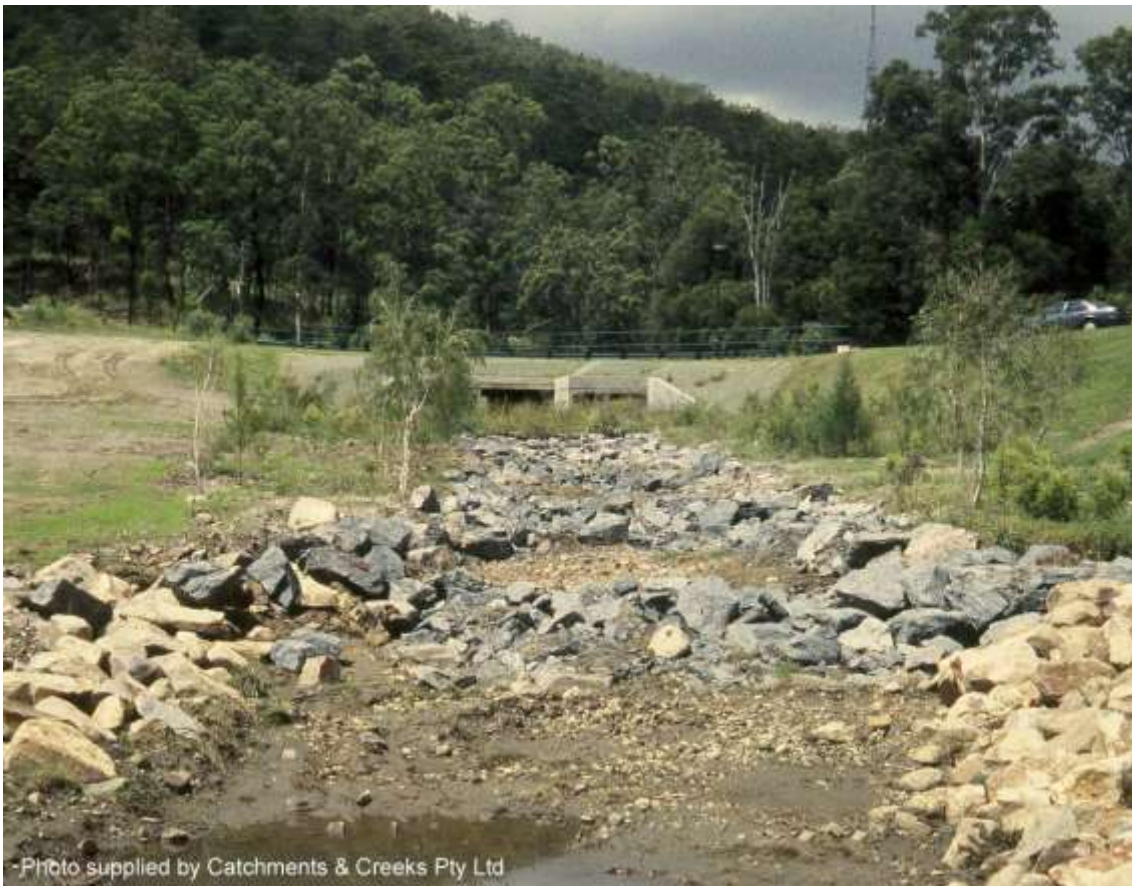
A series of partially exposed recessed rock check dams forming a pool-riffle system
