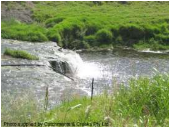
A 'barrier' to fish passage (Qld)
