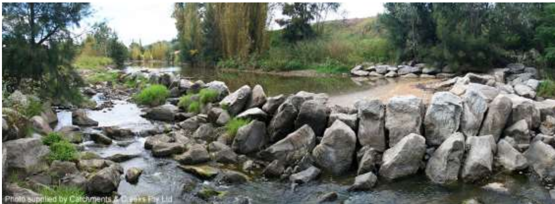
Rock ramp fishway looking upstream from the base of the fishway (Tamworth)
