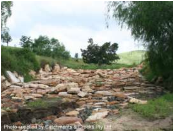
Rock chute stabilising gully erosion (Qld)
