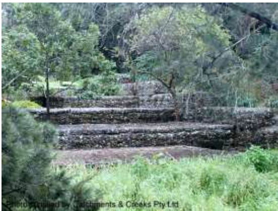
Stepped gabion spillway (Qld)
