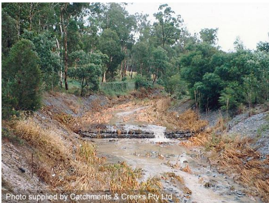
Weeds poisoned in a rock mattress drain
