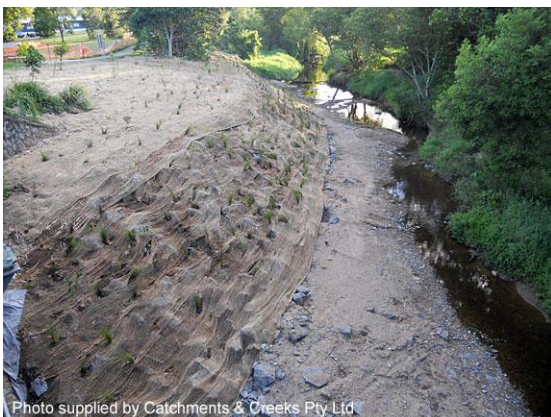
Placement of jute mesh (13/12/12)
