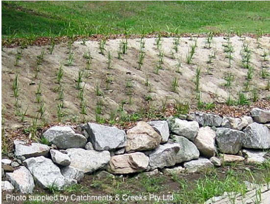
Rock toe protection (Qld)
