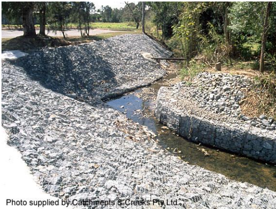
Gabion-lined channel bend (Qld)
