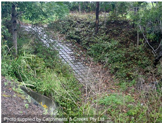
Concrete flex mat maintenance ramp (Qld)
