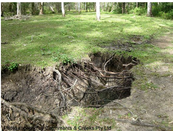
Initial stages of lateral bank erosion (Qld)
