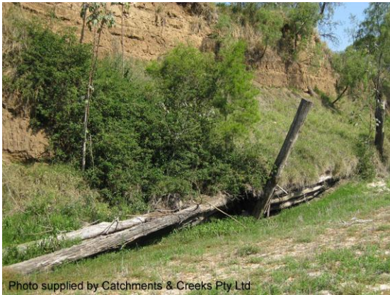
Retard fencing used as toe protection (Qld)
