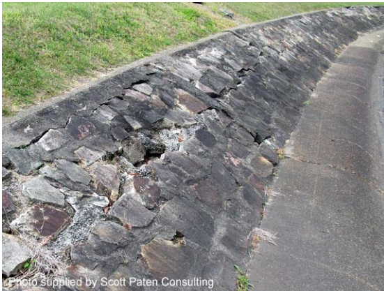
Failure of stone pitching (Qld)
