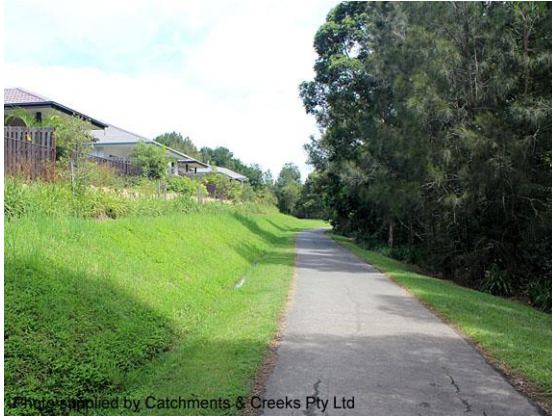
Photo supplied by Catchments & Creeks Pty Ltd Benching of an urban creek bank (Qld)
