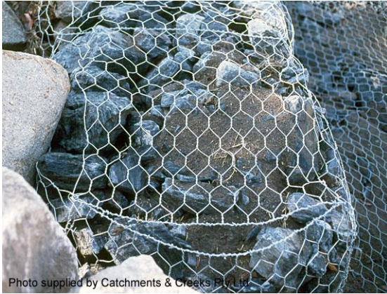
Gabion filled with soil and rock (Qld)
