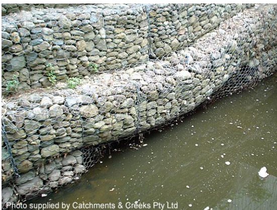
Macquarie Park drop structure (2003)
