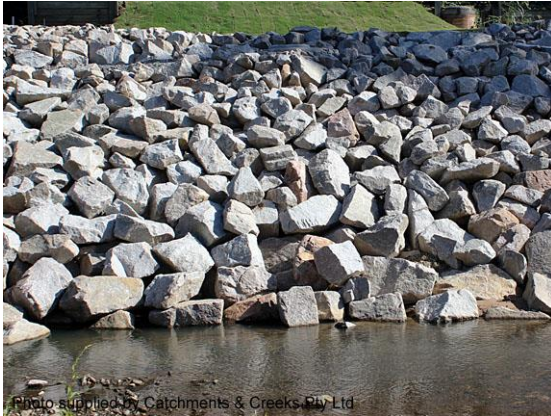
Non-vegetated rock stabilisation
