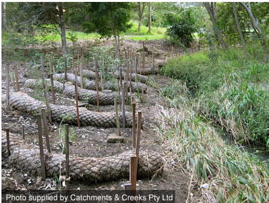
Geo log bank protection (Qld)
