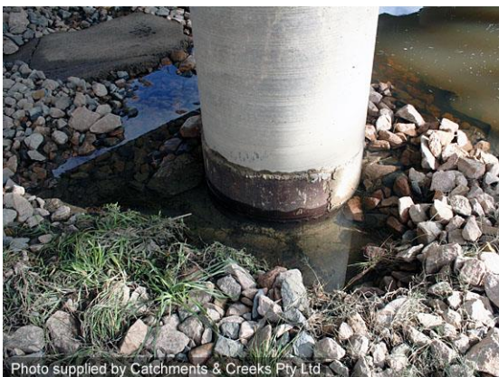
Scour around a bridge pier (Qld)
