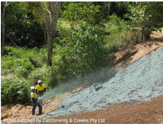
Hydraulically-applied blanket (Qld)
