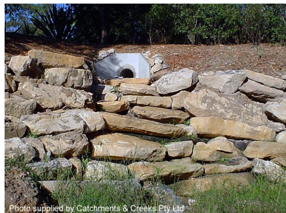
Stepped batter chute (NSW)
