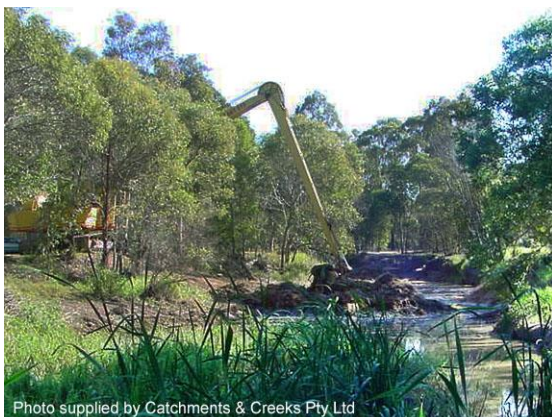
Desilting using a long-reach excavator
