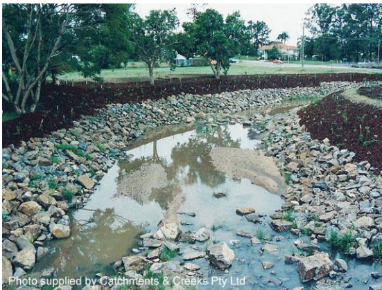
Rock placement on a channel bend (Qld)
