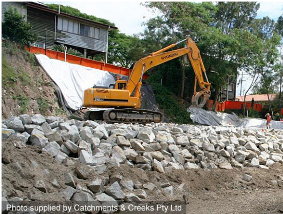
Rock placement over filter cloth (Qld)
