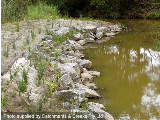
Vegetated rock stabilisation of bank (Qld)
