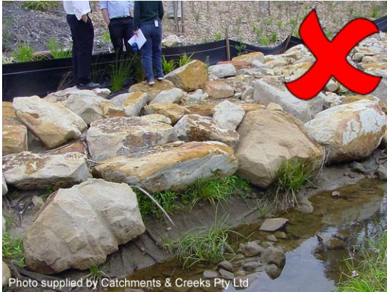
Undermining of toe rock
