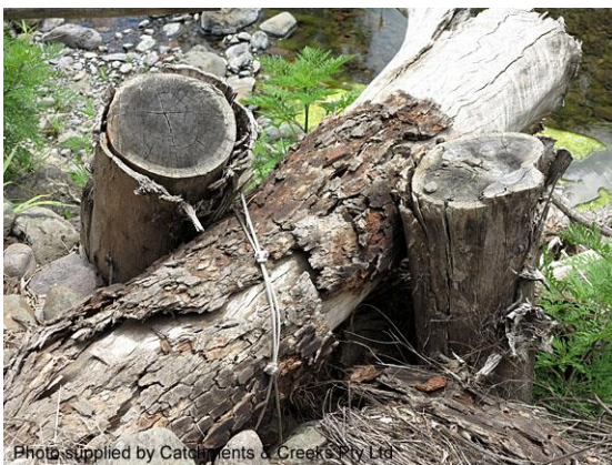
Part of the anchorage system (Qld)
