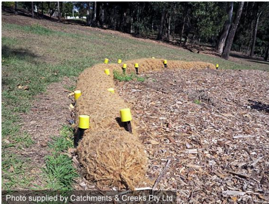
Geo log flow diversion bank (Qld)
