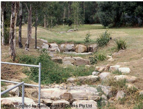
Stepped batter chute (Qld)
