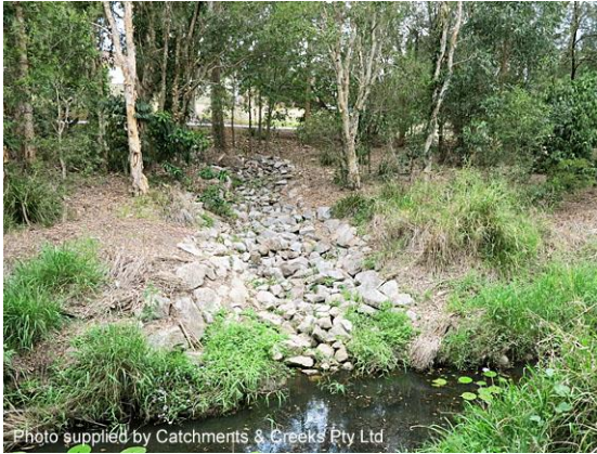
Rock-lined batter chute (Qld)
