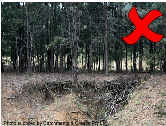
Undermining of bank vegetation
