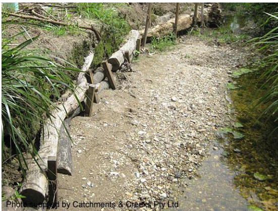
Timber log toe protection (Qld)
