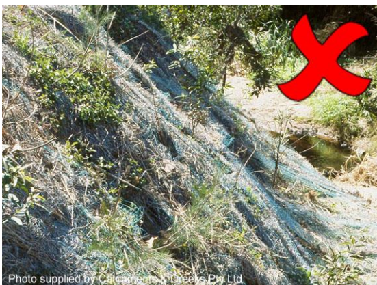
Plastic-reinforced erosion control mat
