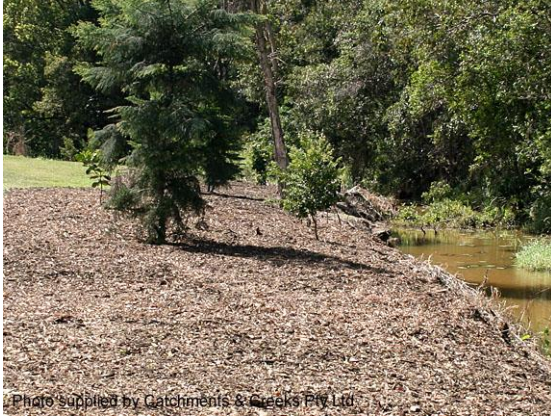
Loose mulch applied to a creek bank
