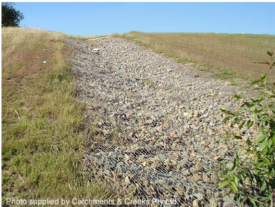
Rock mattress batter chute (Qld)
