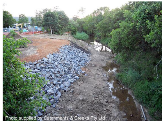
Final rock placement (30/11/12)
