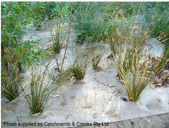
Jute erosion control blanket (SA)
