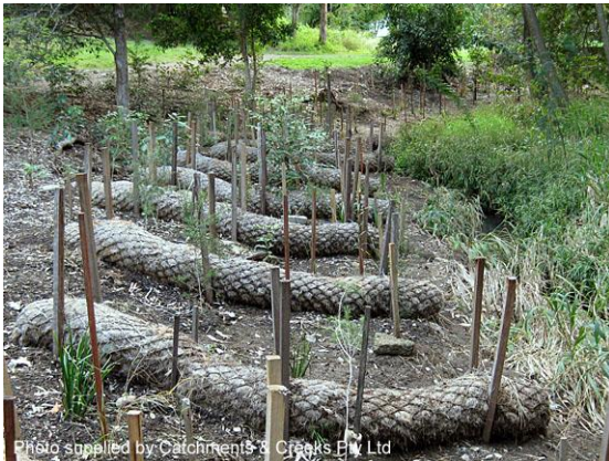
Geo log used to protect new plants (Qld)
