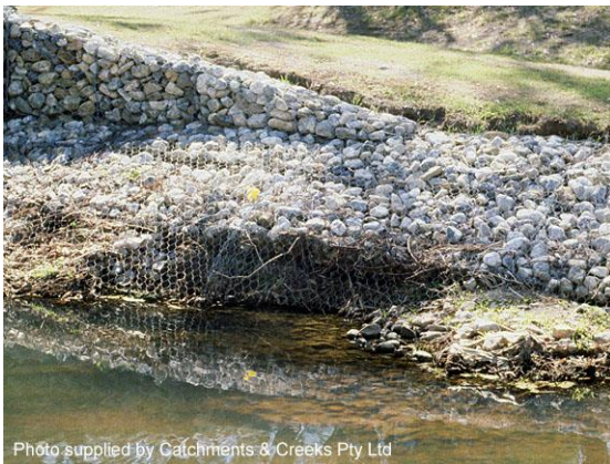
Sandy Creek drop structure (1991)
