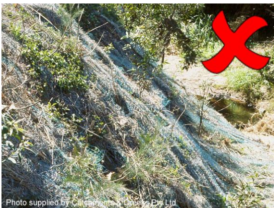
Plastic-reinforced erosion control mat
