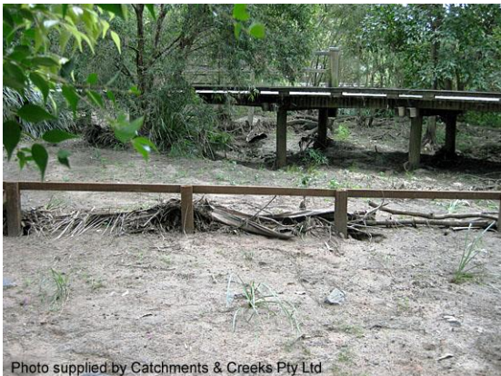
Overbank, timber, retard fence (Qld)
