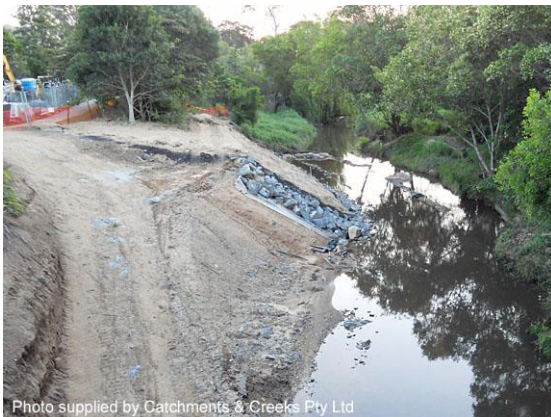
Placement of rock (20/11/12)
