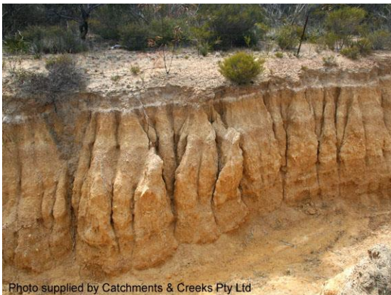
Fluting erosion in a dispersive soil (SA)
