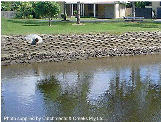
Flexible concrete mat bank protection
