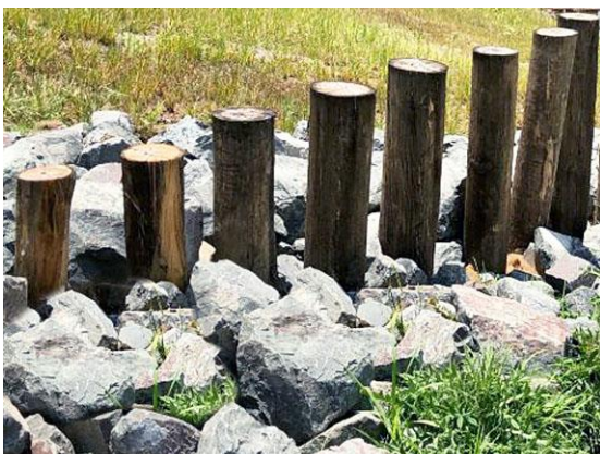
Pile field flow control vanes (Qld)
