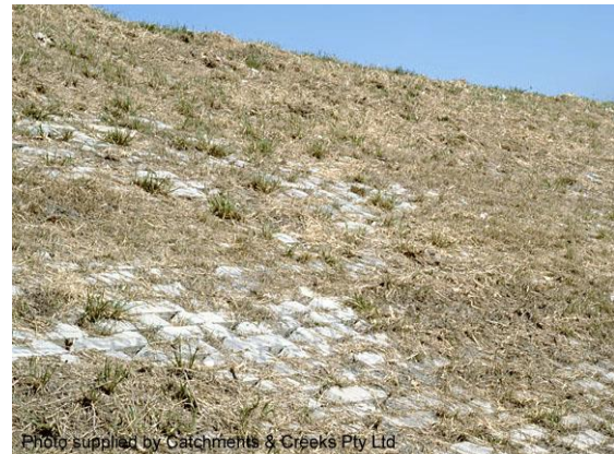
Vegetated concrete mat bank protection
