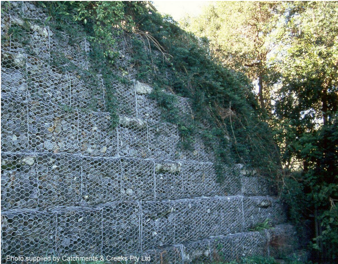
Gabion creek bank retaining wall (Qld)
