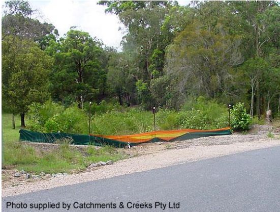
Stiff grass chute currently off-line (Qld)
