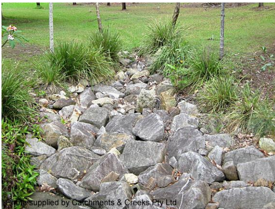
Rock-lined batter chute (Qld)
