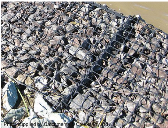
Plastic cage gabion (Qld)
