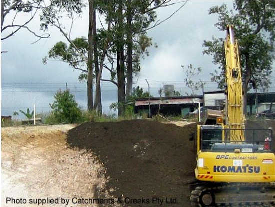
Placement of topsoil on a bank (NSW)
