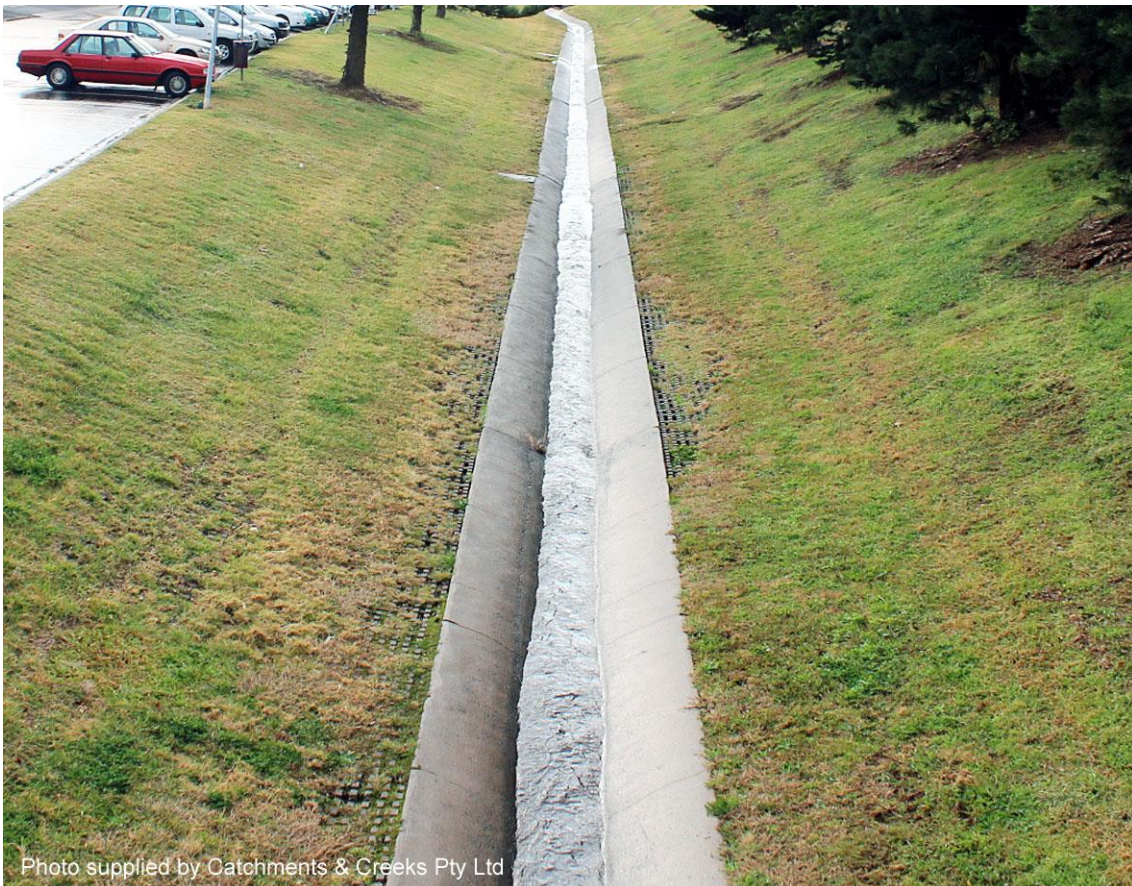
Vegetated porous pre-cast concrete pavers (Qld)
