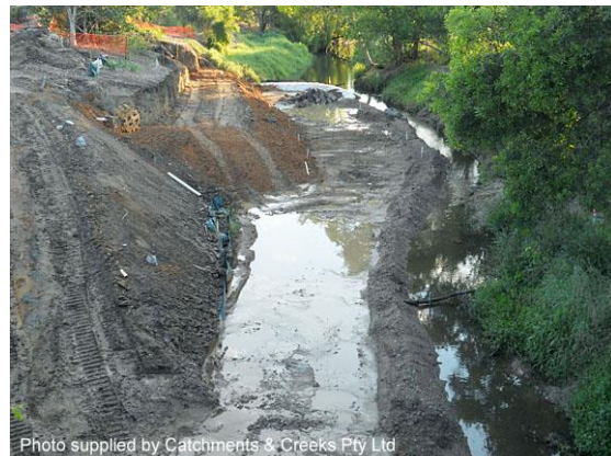
Placement of fill (31/10/12)
