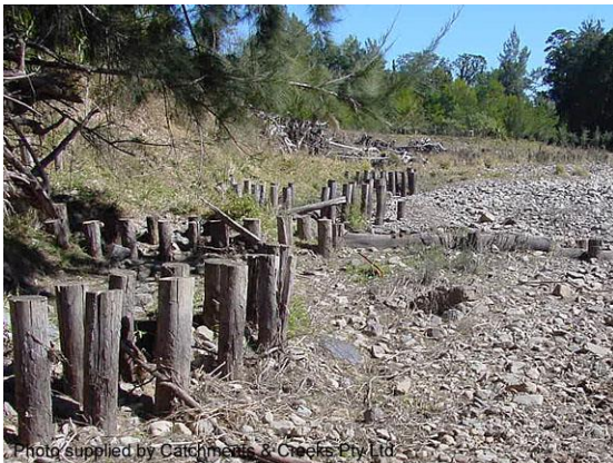
Pile field toe protection (NSW)
