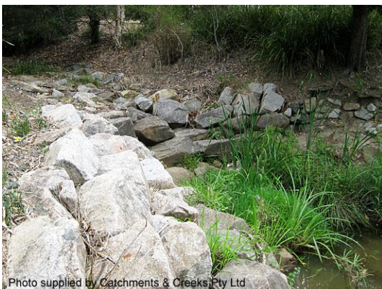
Stepped batter chute (Qld)
