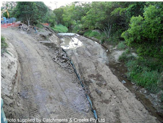
Establish flow diversion bund (24/10/12)
