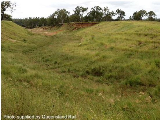
Gully stabilisation with vetiver grass (Qld)
