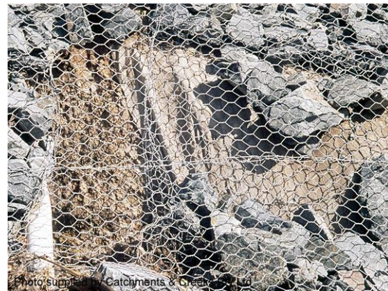
Alexandra Hills drop structure (1995)
