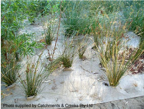
Jute erosion control blanket (SA)
