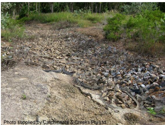
Rock-filled car tyre batter chute (NT)
