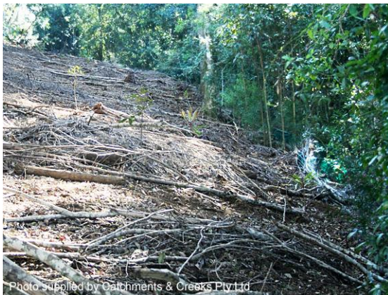
Brushing of overbank area (Qld)
