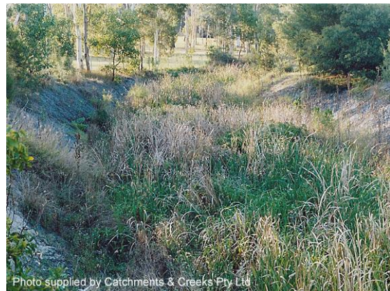
Weed invasion of the same drain (left)
