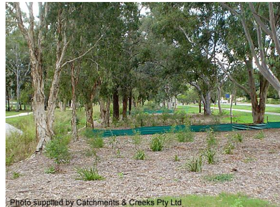
Sediment fence retard fencing (Qld)
