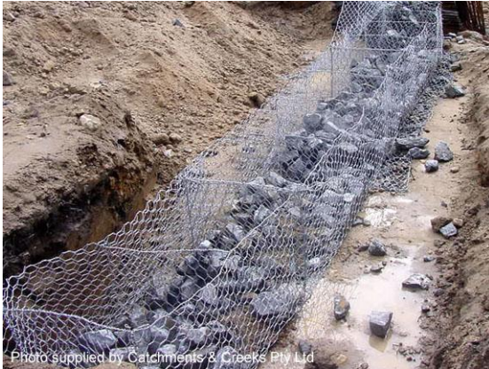
Construction of a gabion wall (Qld)
