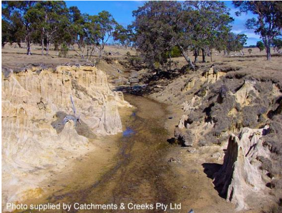
Erosion of a dispersive soil (NSW)
