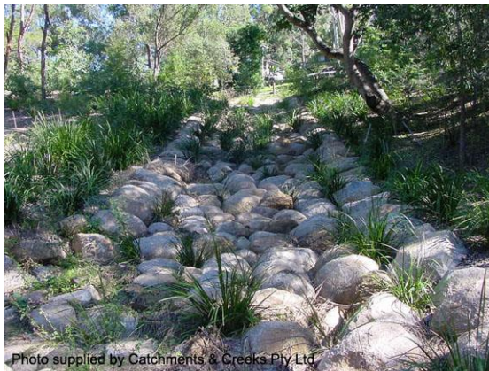
Partially-vegetated batter chute (Qld)
