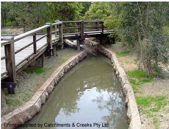
Concrete-lined stormwater drain
