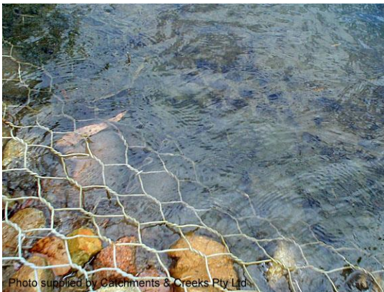
Rock mattress in a waterway environment
