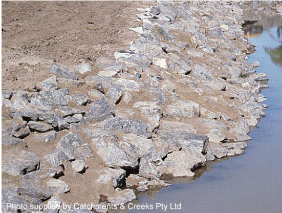
Soil-filled voids ready for planting (1999)
