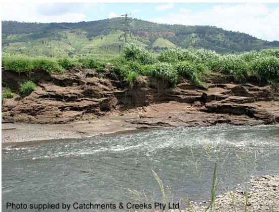
Flood-induced bank scour (Qld)
