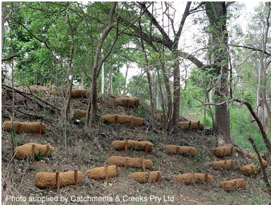
Geo log bank protection (Qld)
