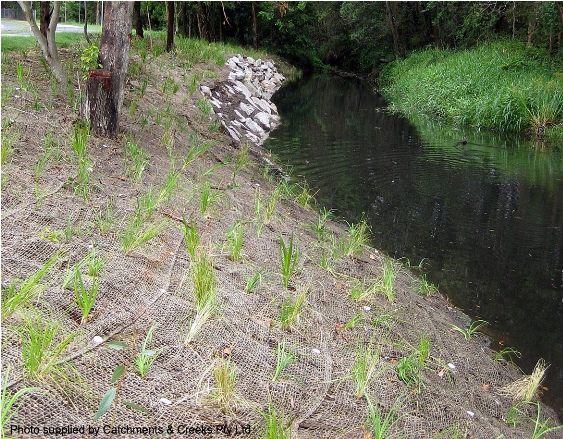
Bank reshaping and revegetation (Qld)
