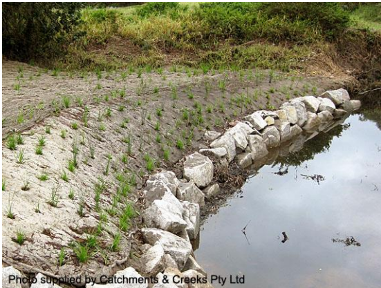
Rock protection of the lower bank (Qld)
