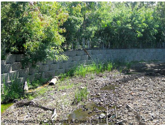
Concrete block retaining wall
