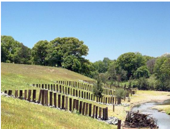
Timber 'pin groyne' (Qld)
