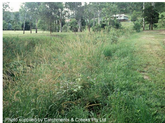
Weed invasion of the same drain (left)
