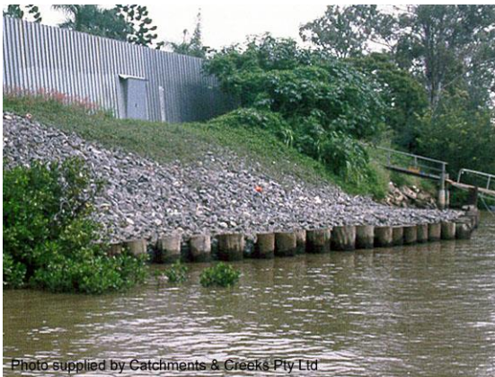
Pile field toe protection (Qld)
