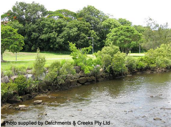
Vegetated rock stabilisation (Qld)
