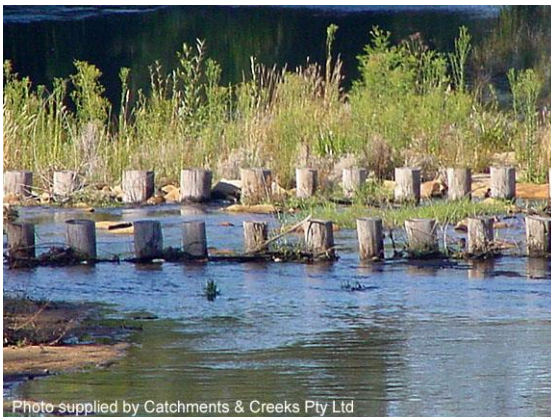
Pile field bed control structure (Vic)
