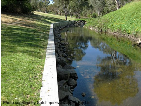
Vertical retaining wall
