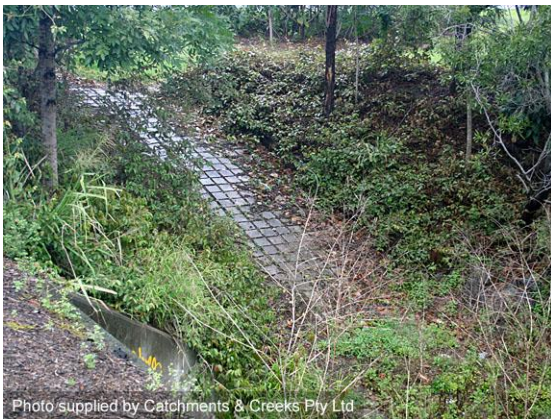
Flexible modular concrete mat (Qld)
