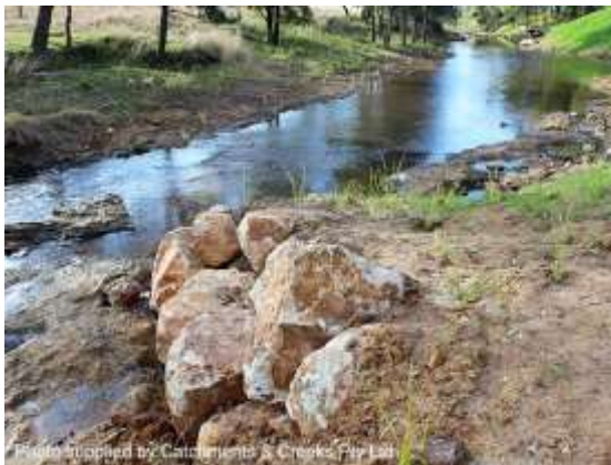
Rock groyne (Qld)
