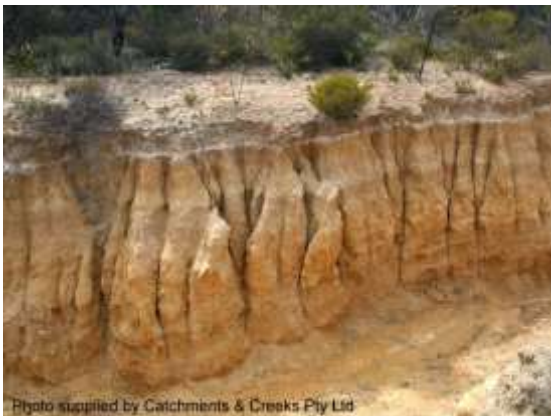
Fluting erosion in a dispersive soil (SA)
