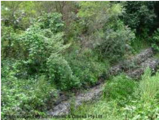
Vegetated gabion wall (Qld)
