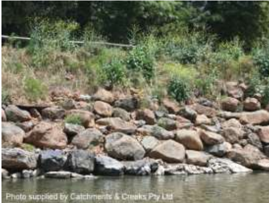
Partial vegetated bank stabilisation (NSW)
