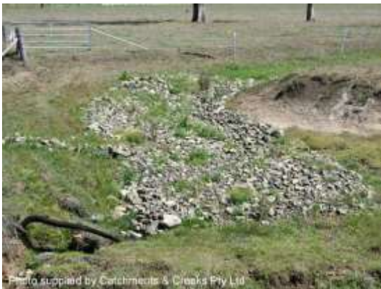
Stabilised stock access ramp (Qld)
