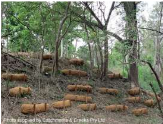
Geo log bank protection (Qld)
