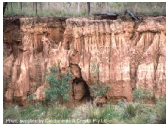
Fluting and tunnel erosion (Qld)
