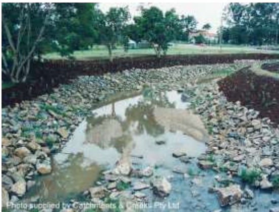
Rock placement on a channel bend (Qld)
