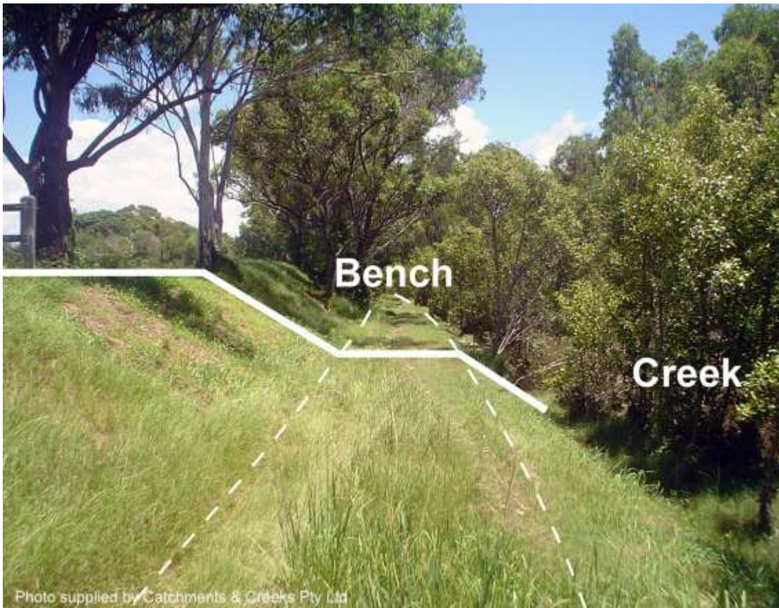
Benching of a creek bank to form a maintenance berm (Qld)
