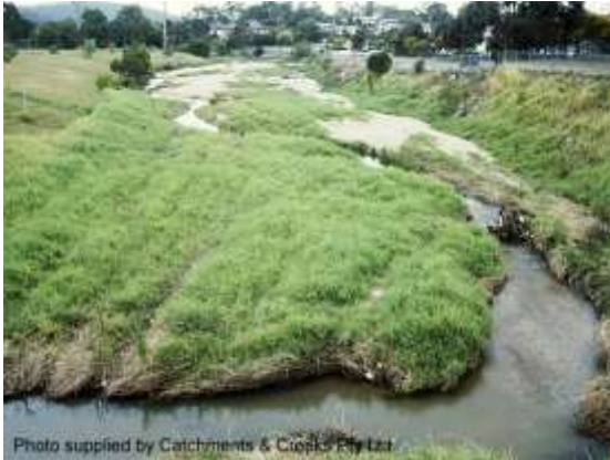
Bed sediment stabilised with grasses
