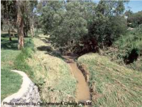
Grasses flattened by floodwater (Qld)
