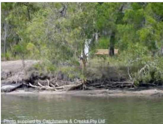
Wave-induced bank erosion (Qld)
