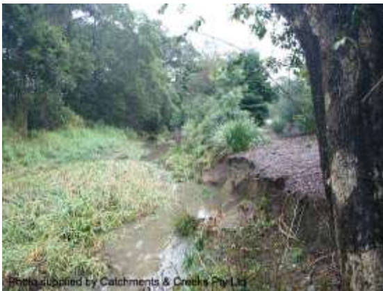
Looking upstream, November 2010
