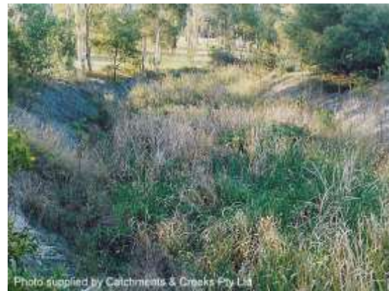
Weed invasion of the same drain (left)
