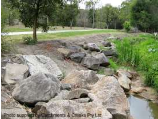
Rock groynes (Qld)
