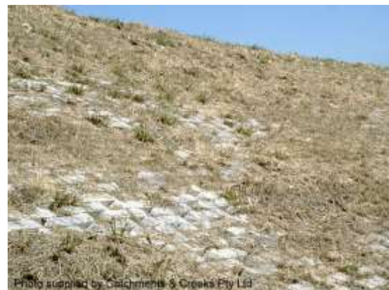
Vegetated concrete mat bank protection
