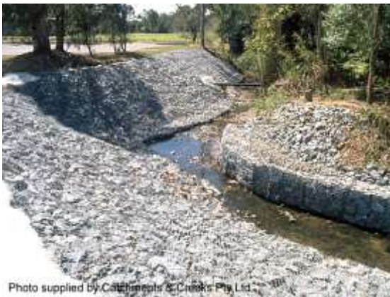
Gabion-lined channel bend (Qld)
