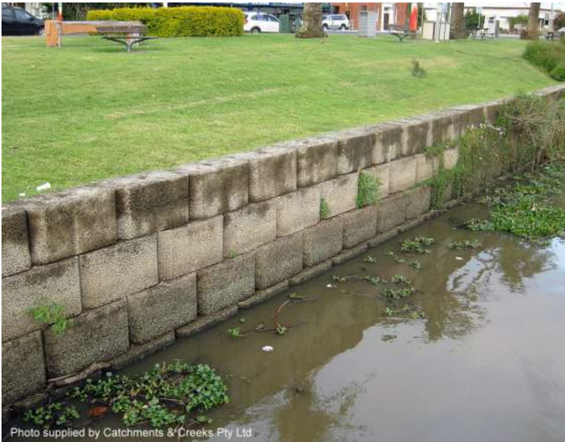
Concrete block river retaining wall
