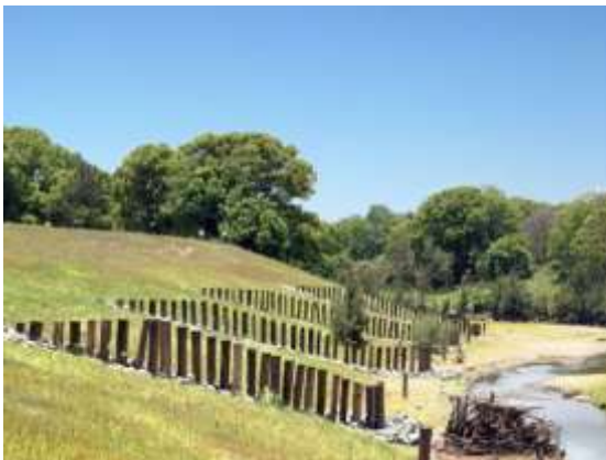
Timber 'pin groyne' (Qld)
