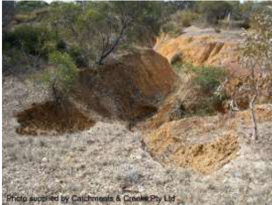
Lateral bank erosion (SA)
