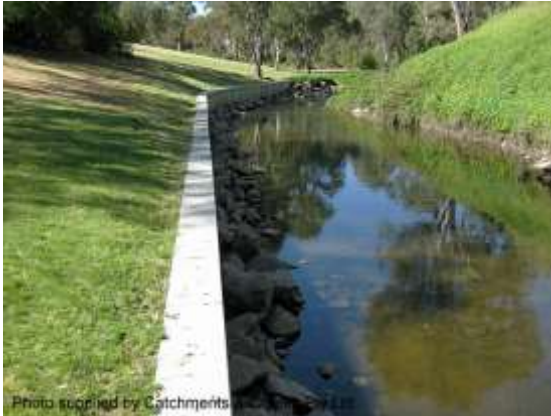
Vertical retaining wall
