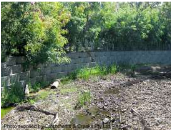
Concrete block retaining wall
