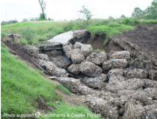
Jim Finimore Park drop structure (2008)
