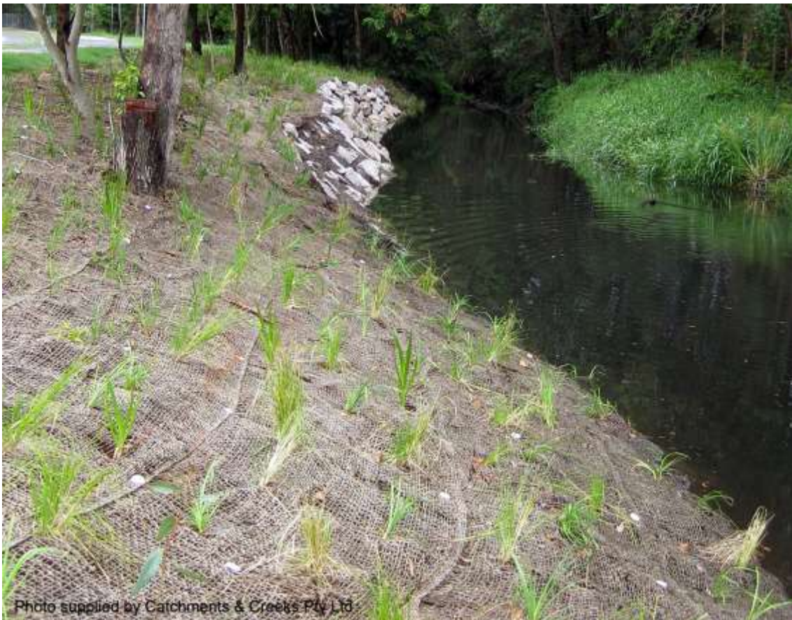
Bank reshaping and revegetation (Qld)
