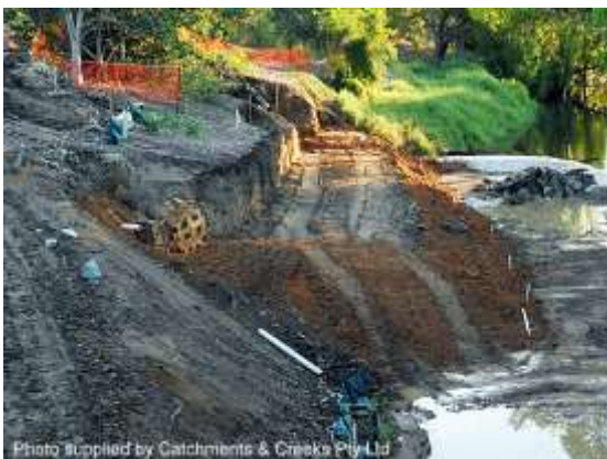
Benching to provide equipment access
