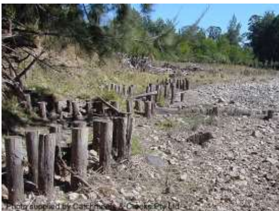
Pile field toe protection (NSW)
