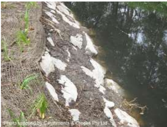
Voids filled with soil prior to planting
