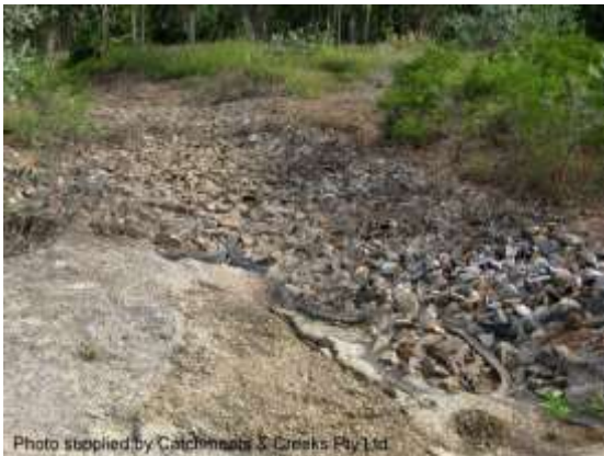
Rock-filled car tyre batter chute (NT)
