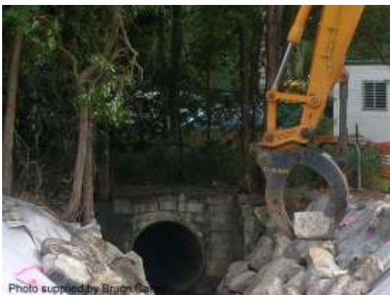
Individual placement of rocks (Qld)
