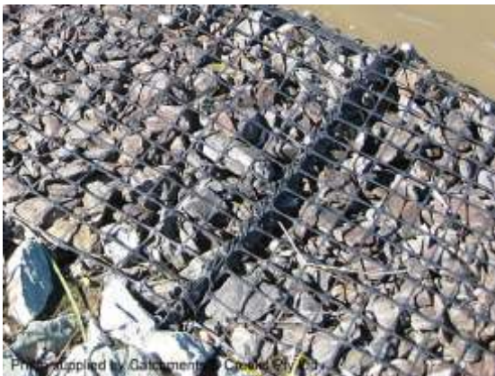
Plastic cage gabion (Qld)
