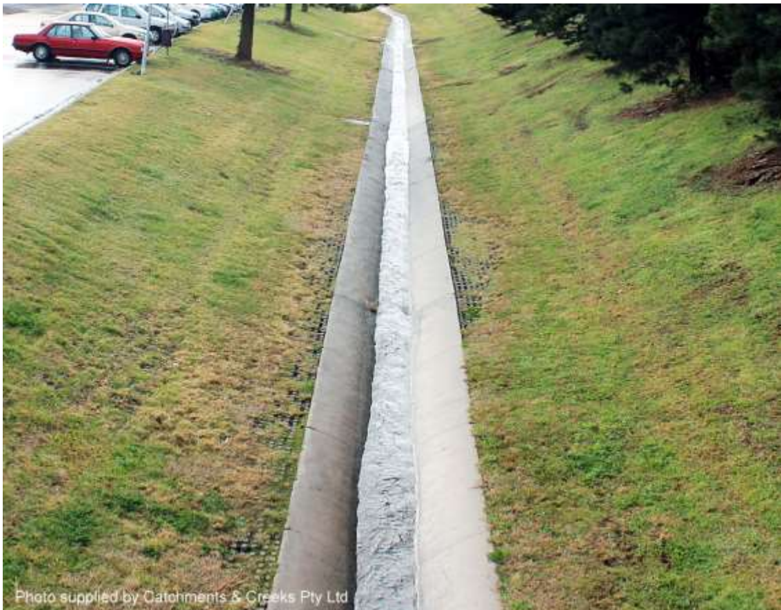
Vegetated porous pre-cast concrete pavers (Qld)
