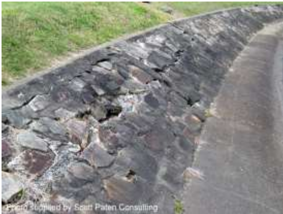
Failure of stone pitching (Qld)
