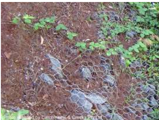
Mulch covered rock mattress (Qld)
