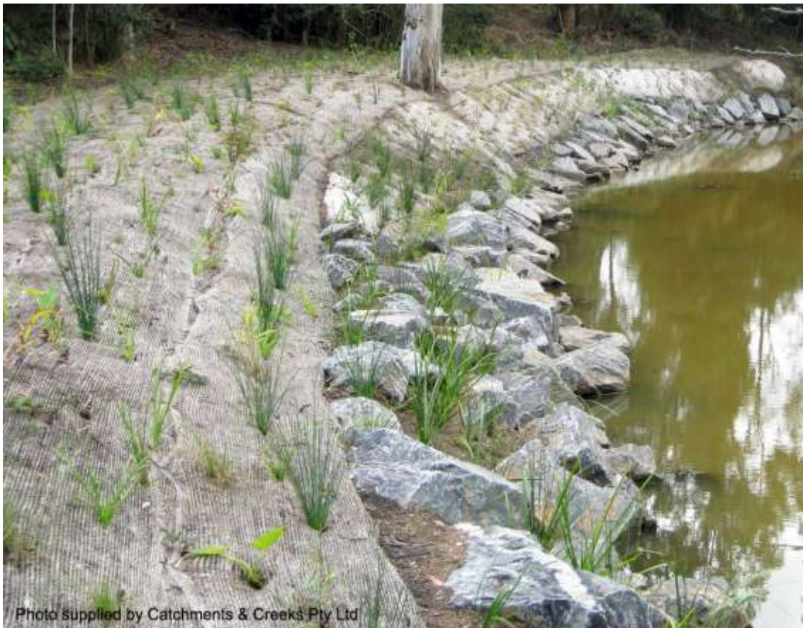
Vegetated rock stabilisation of a creek bank (Qld)
