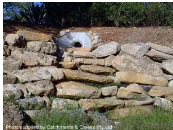
Stepped batter chute (NSW)
