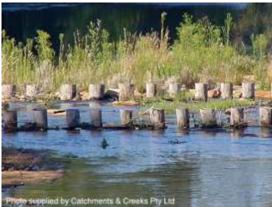
Pile field bed control structure (Vic)
