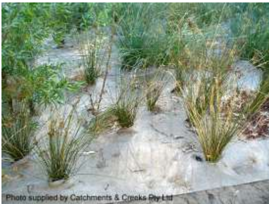
Jute erosion control blanket (SA)
