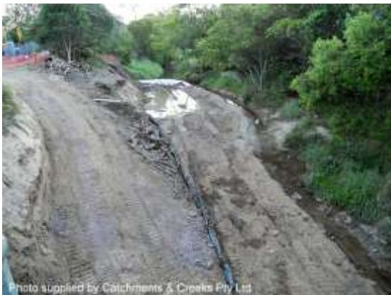
Establish flow diversion bund (24/10/12)
