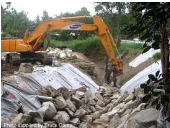
Rock placement (Qld)
