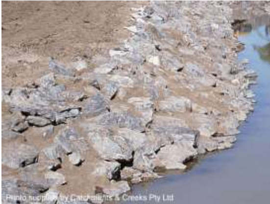
Soil-filled voids ready for planting (1999)
