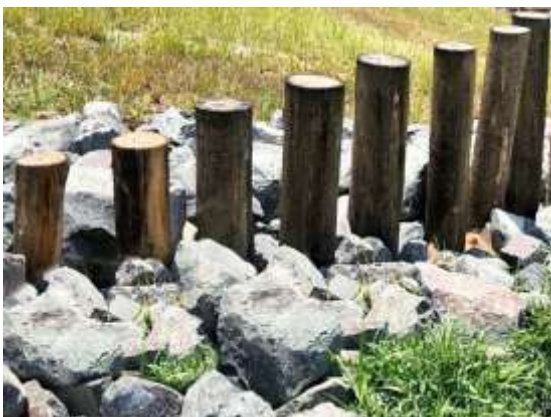
Pile field flow control vanes (Qld)
