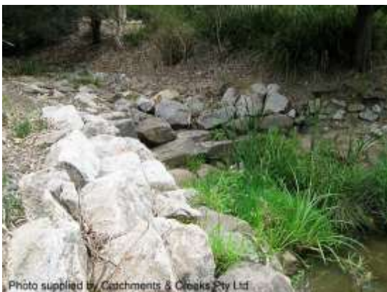
Stepped batter chute (Qld)
