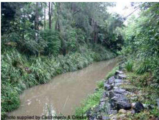
Fully established creek bank (2010)
