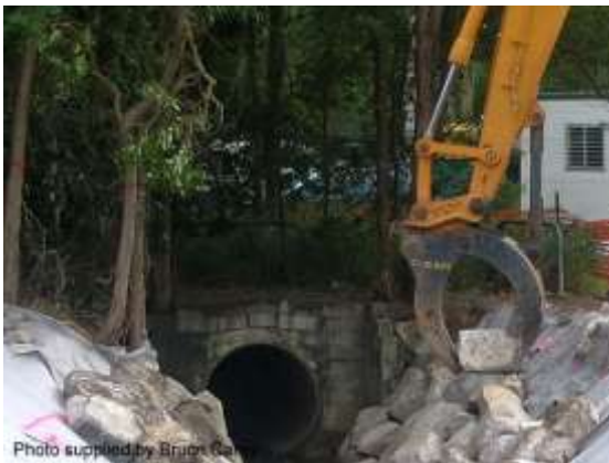
Individual placement of rocks (Qld)
