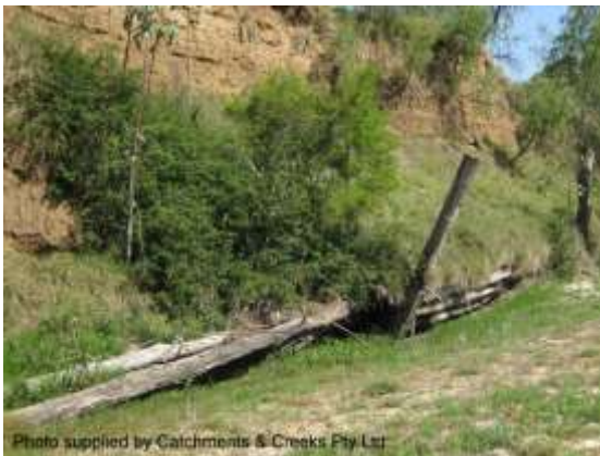
Retard fencing used as toe protection (Qld)
