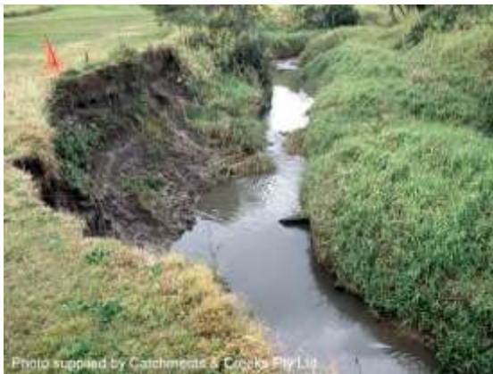
Erosion (left), grassed sediment (right)
