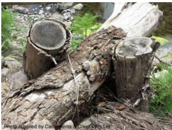
Part of the anchorage system (Qld)
