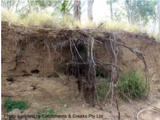
Bank undercutting (Qld)
