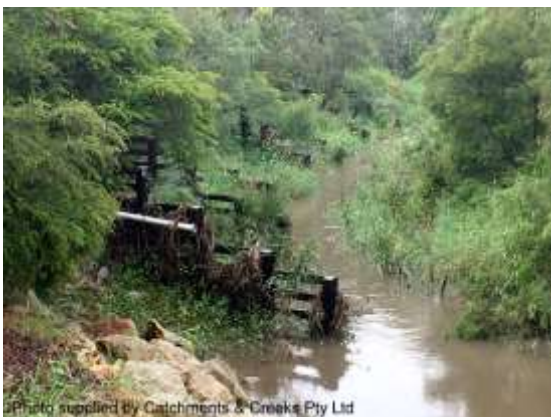
Establishment of vegetation along the bank
