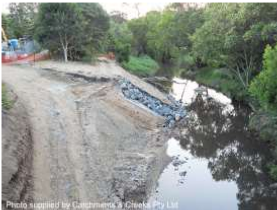
Placement of rock (20/11/12)
