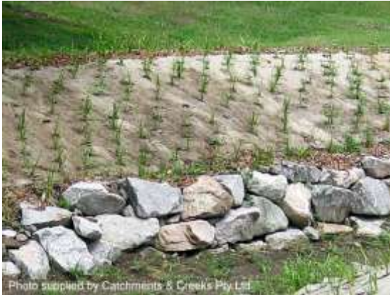
Rock toe protection (Qld)
