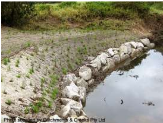
Rock protection of the lower bank (Qld)
