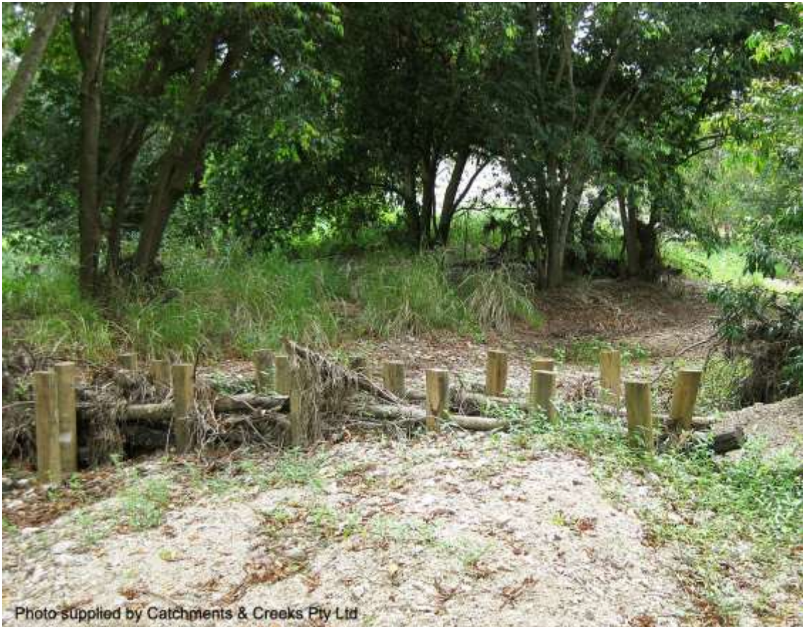
Pile field used to stop flows cutting a new channel through a low bench (Qld)
