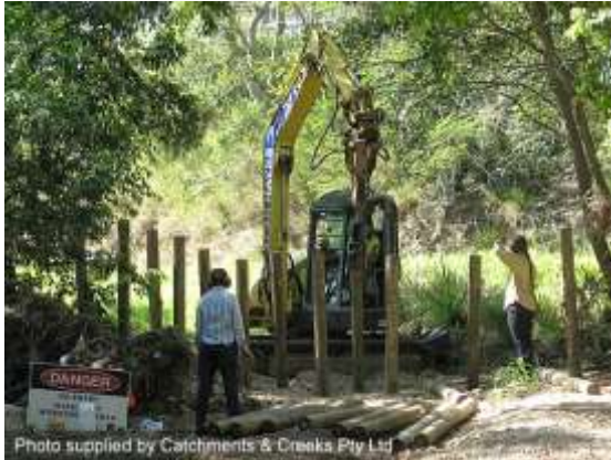
Installation of a pile field (Qld)
