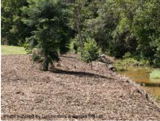
Loose mulch applied to a creek bank
