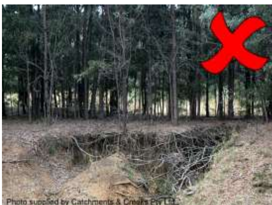
Undermining of bank vegetation
