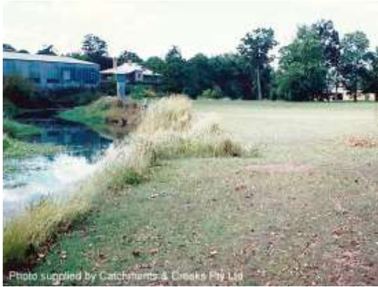
Looking downstream towards weir
