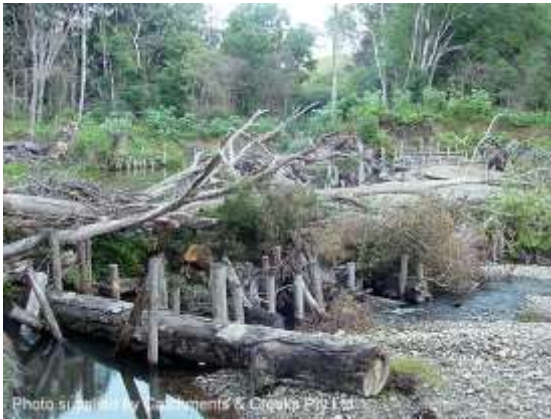
Pile field groyne (NSW)
