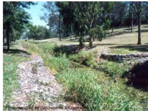
Weed invasion of the same drain (left)
