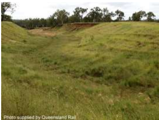
Gully stabilisation with vetiver grass (Qld)
