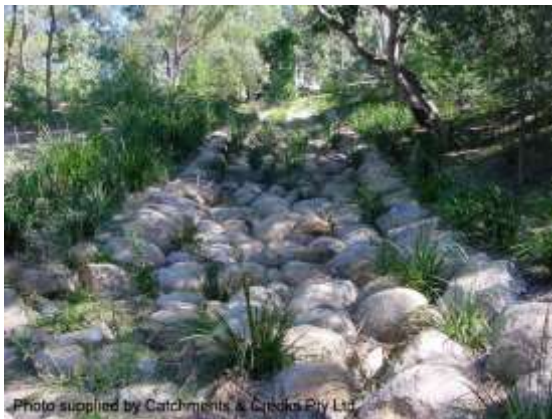
Partially-vegetated batter chute (Qld)
