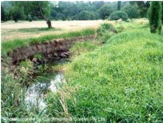
Bank erosion (left), sediment (right)
