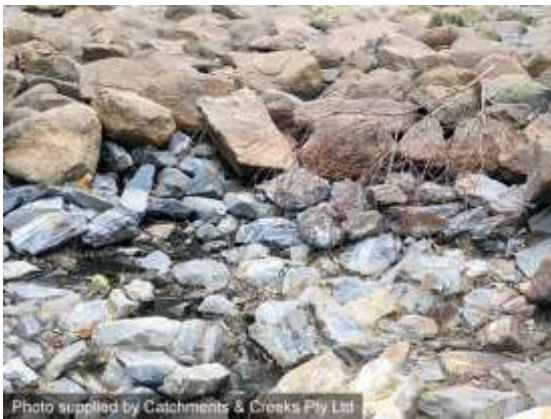
Rock filter layer (blue) under surface rock
