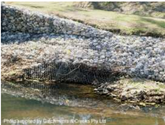
Sandy Creek drop structure (1991)
