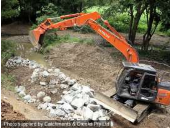
Bank stabilisation with rock (Qld)
