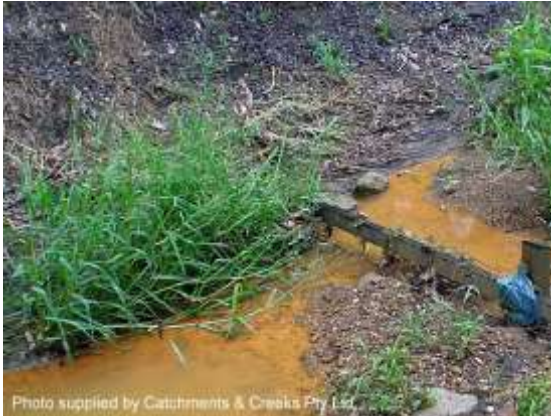
Sedimentation around a retard fence (Qld)
