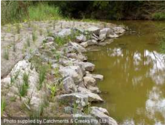
Vegetated rock stabilisation of bank (Qld)
