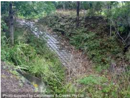
Concrete flex mat maintenance ramp (Qld)
