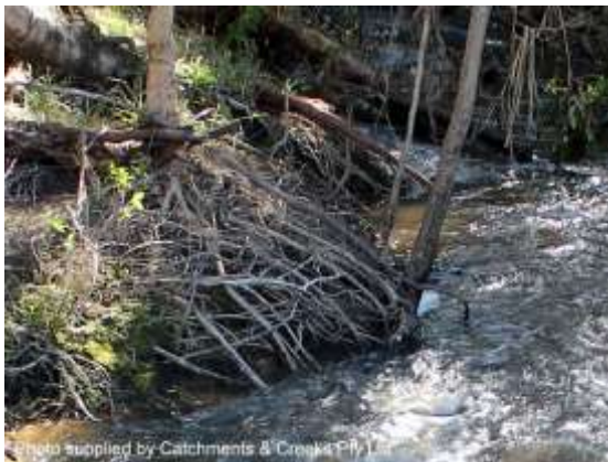
Exposed tree roots (Qld)
