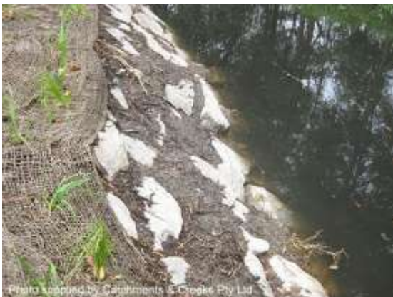
Voids filled with soil ready for planting
