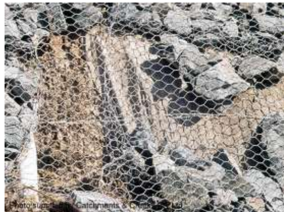
Alexandra Hills drop structure (1995)
