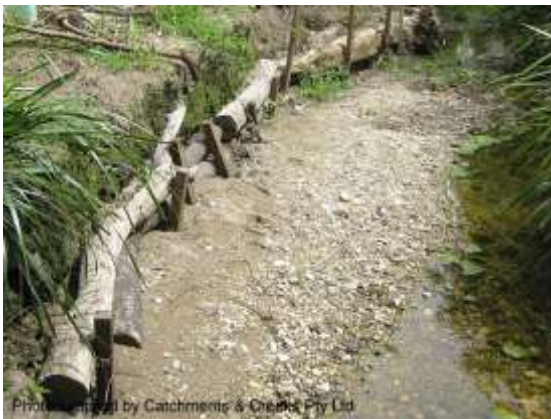
Timber log toe protection (Qld)
