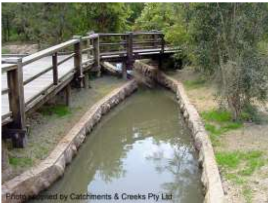
Concrete-lined stormwater drain
