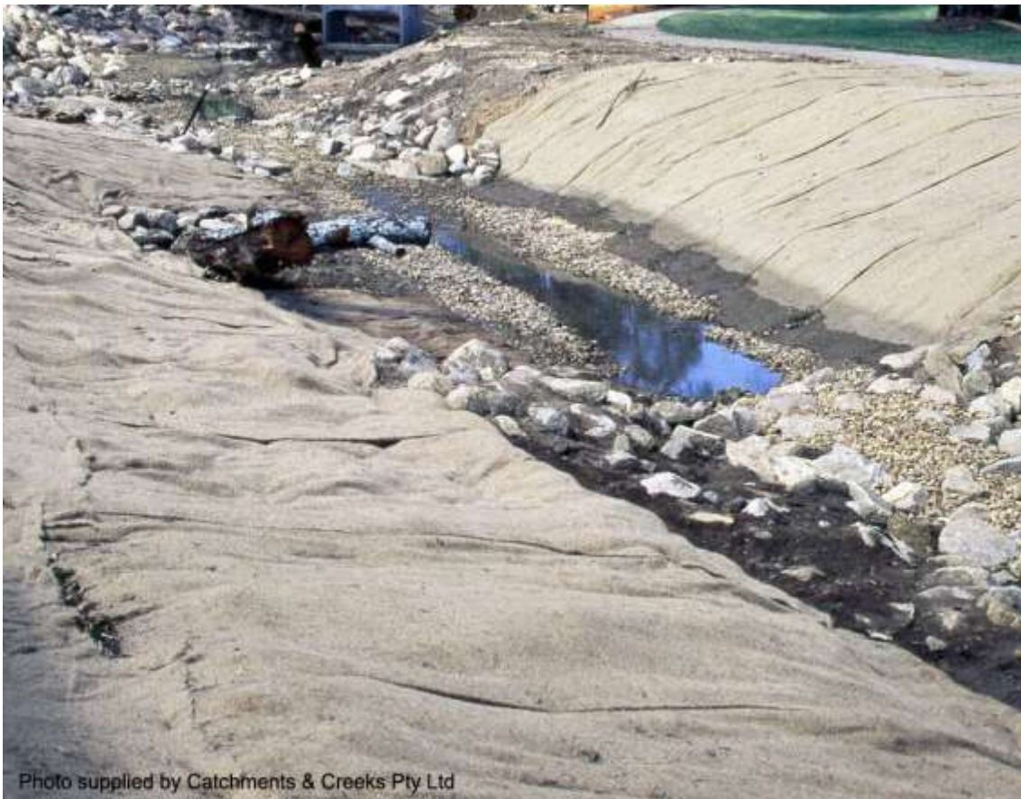
Bio-degradable 'jute' erosion control blankets prior to planting (Qld)
