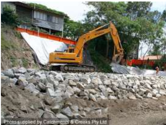
Rock placement over filter cloth (Qld)
