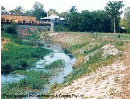
Looking downstream towards weir
