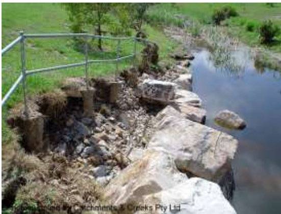
Soil erosion behind a retaining wall
