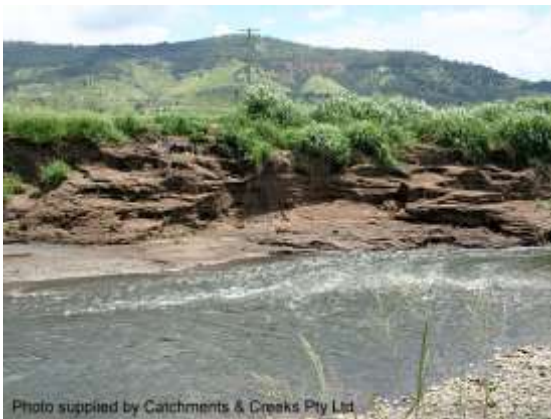
Flood-induced bank scour (Qld)
