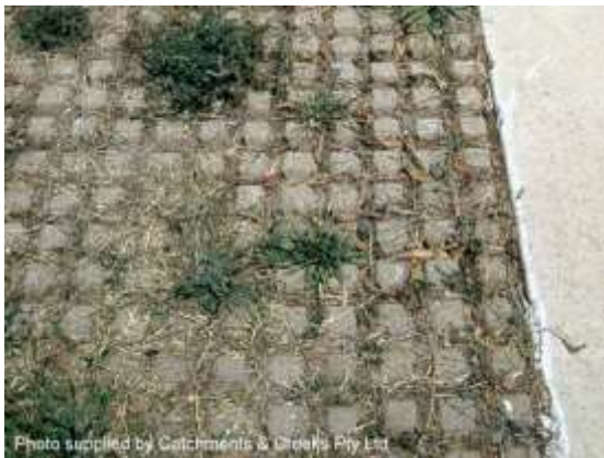
Porous concrete pavers (ACT)
