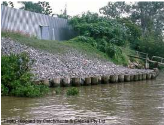
Pile field toe protection (Qld)
