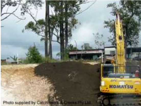
Placement of topsoil on a bank (NSW)
