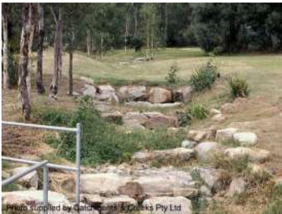
Stepped batter chute (Qld)
