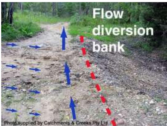
Diversion of stormwater runoff (NSW)
