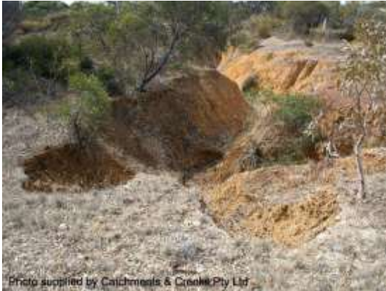
Lateral bank erosion (SA)
