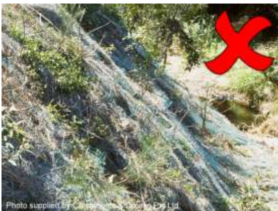
Plastic-reinforced erosion control mat
