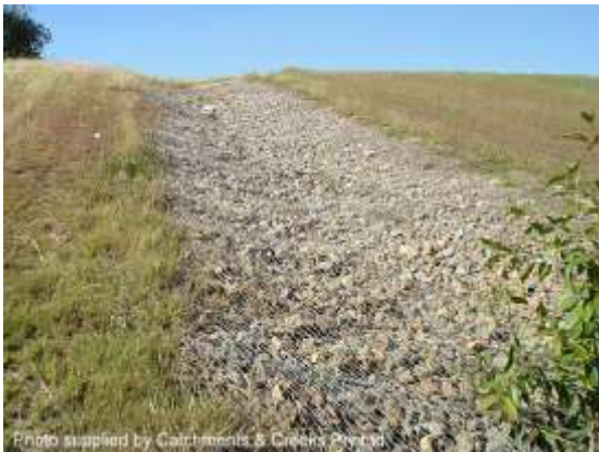
Rock mattress batter chute (Qld)
