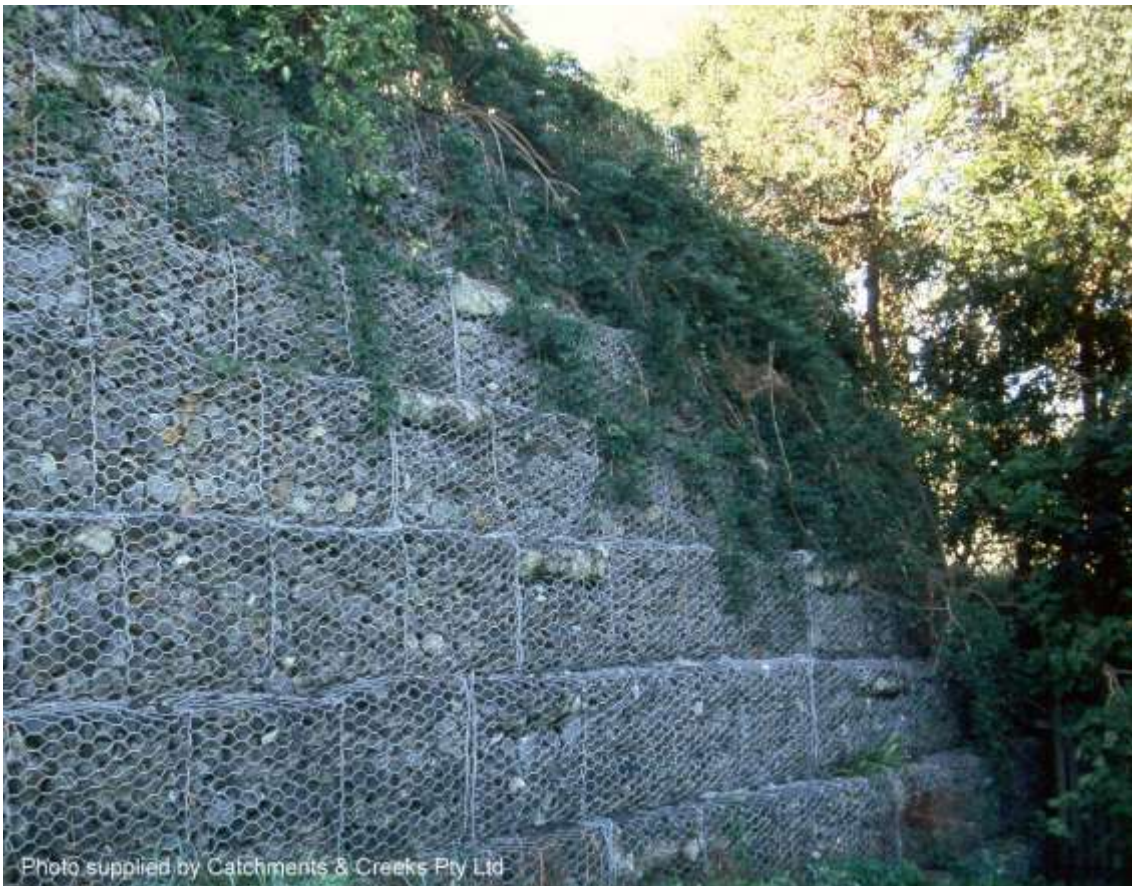
Gabion creek bank retaining wall (Qld)
