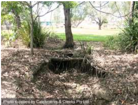
Stormwater-induced lateral bank erosion
