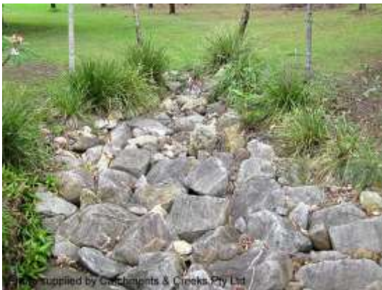
Rock-lined batter chute (Qld)
