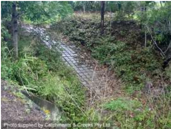
Flexible modular concrete mat (Qld)
