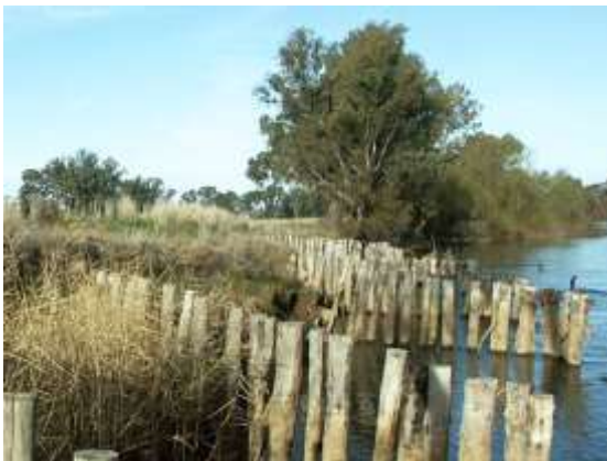
Pile groynes (Vic)
