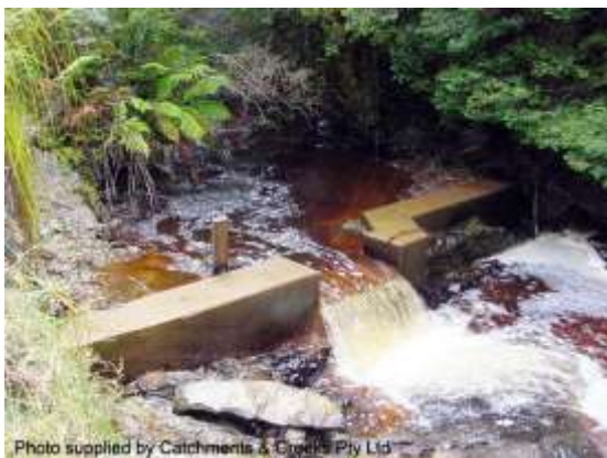
Flow monitoring weir (Tas)
