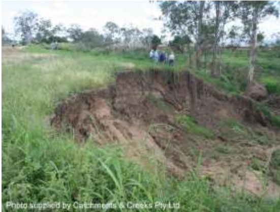
Bank slump (Qld)
