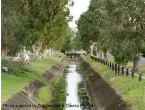
Concrete-lined stormwater drain (Qld)
