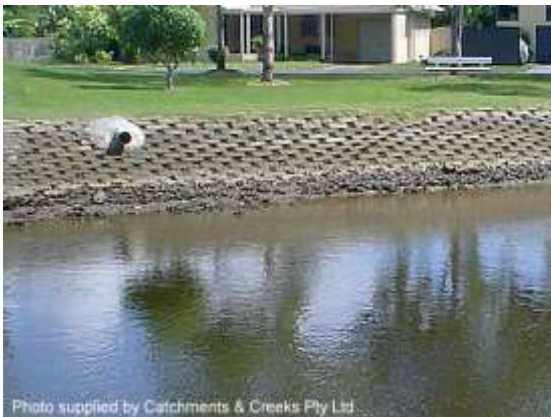
Flexible concrete mat bank protection
