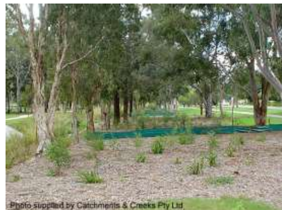
Sediment fence retard fencing (Qld)
