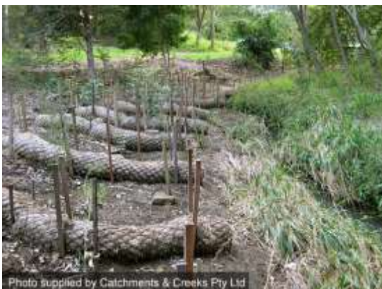
Geo log bank protection (Qld)
