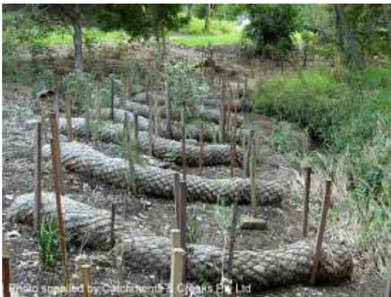
Geo log used to protect new plants (Qld)
