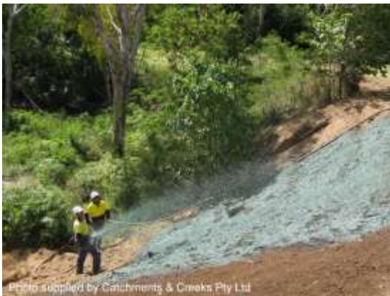
Hydraulically-applied blanket (Qld)
