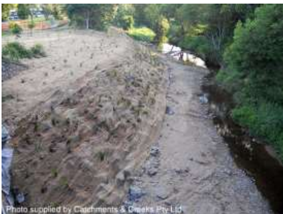
Placement of jute mesh (13/12/12)
