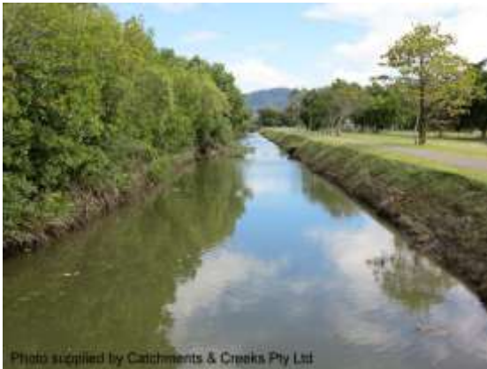
'Greening' of an old storm drain (Qld)
