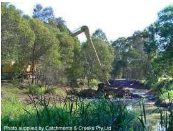
Desilting using a long-reach excavator
