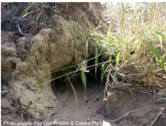
Outlet of a tunnel near a creek (Qld)
