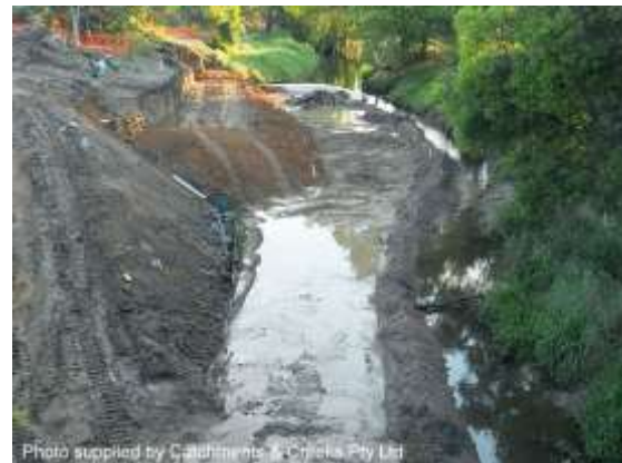
Placement of fill (31/10/12)
