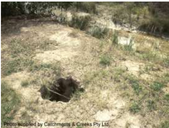
Entrance to a tunnel near a creek (Qld)
