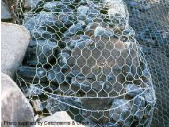
Gabion filled with soil and rock (Qld)
