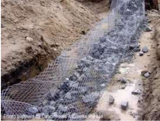
Construction of a gabion wall (Qld)
