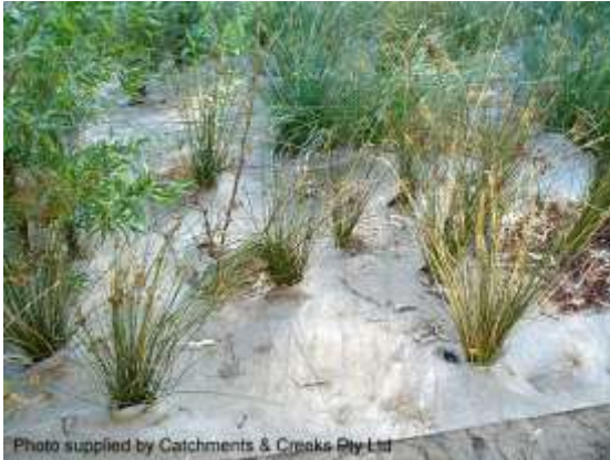
Jute erosion control blanket (SA)
