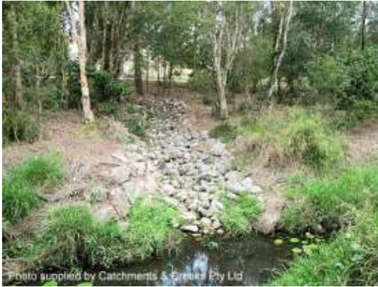
Rock-lined batter chute (Qld)
