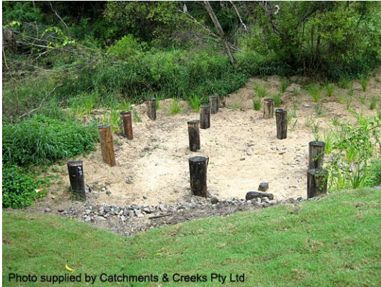
Pile field (Qld)
