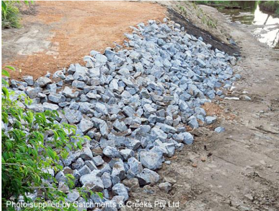
Rock stabilisation pre-planting (Qld)
