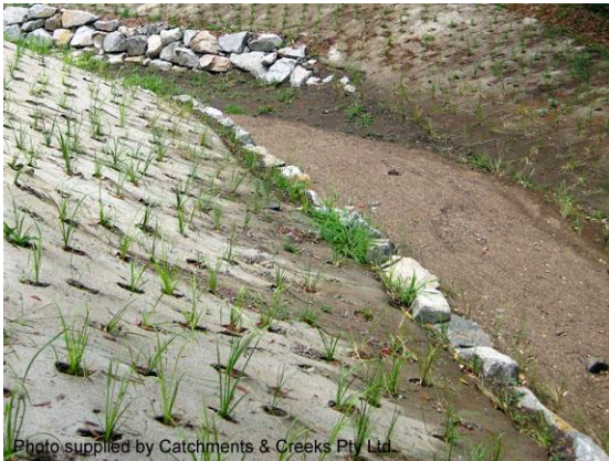
Inside bank with toe protection (Qld)
