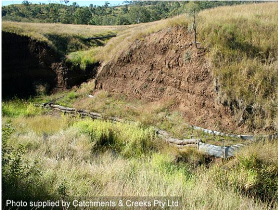
Retard fencing used in gully erosion (Qld)
