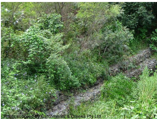
Vegetated gabion wall (Qld)
