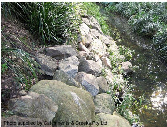
Placed rock bank stabilisation (Qld)
