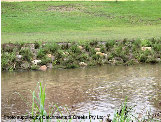
Vegetated rock stabilisation (Qld)
