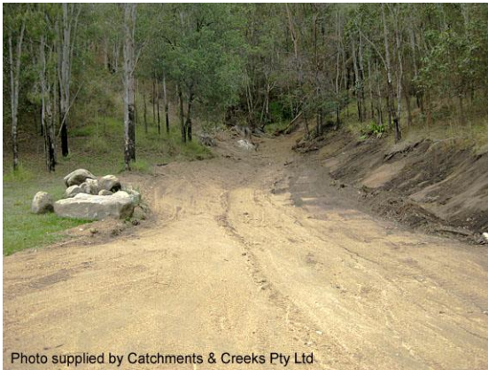
Treated slope prior to planting (Qld)
