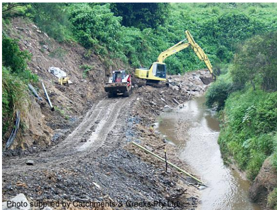
Equipment access (Qld)
