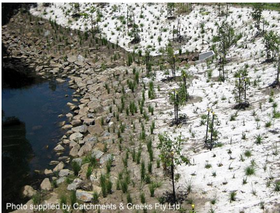
Bank revegetation with toe rock (Qld)
