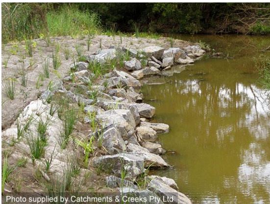
Vegetated rock stabilisation (Qld)
