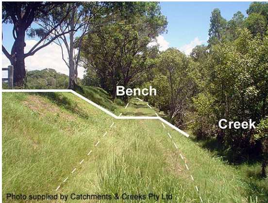
Benching of a creek bank (Qld)
