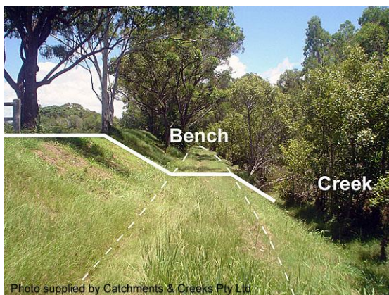
Maintenance berm (Qld)
