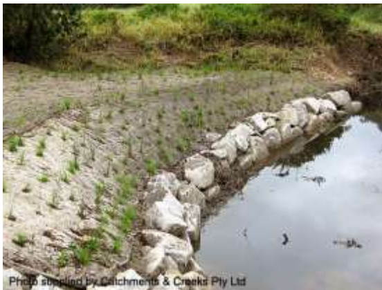
Rock toe protection (Qld)
