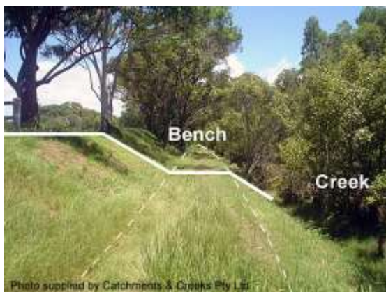
Maintenance berm (Qld)
