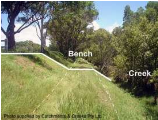
Benching of a creek bank (Qld)
