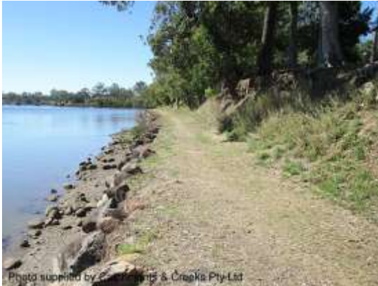
Benching of a river bank (Qld)
