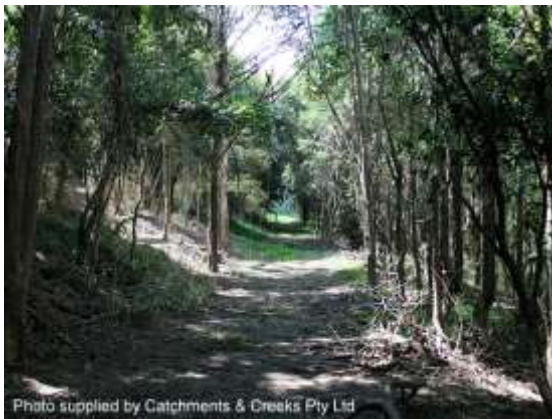
Benching of a river bank (Qld)
