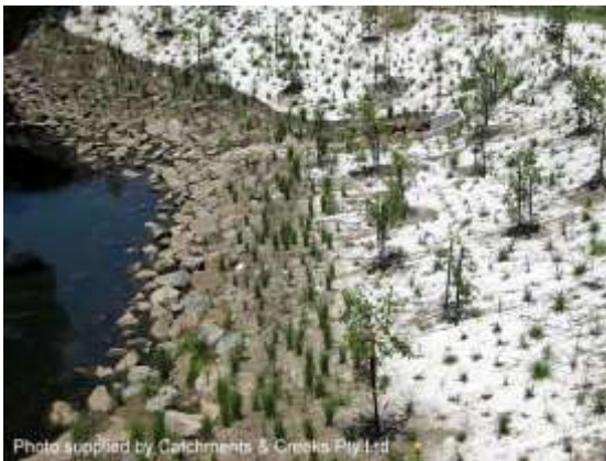
Bank revegetation with toe rock (Qld)
