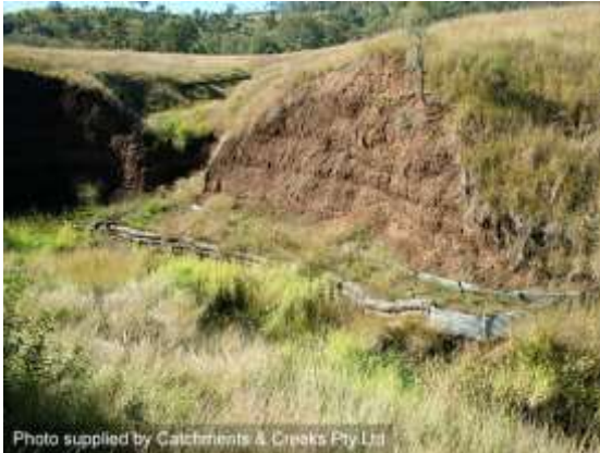
Retard fencing used in gully erosion (Qld)
