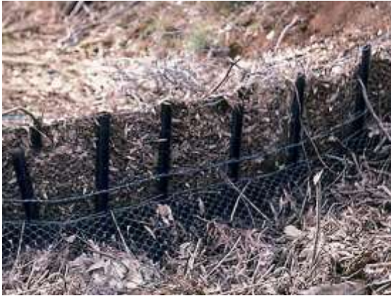
Mulch collecting on a wire mesh fence
