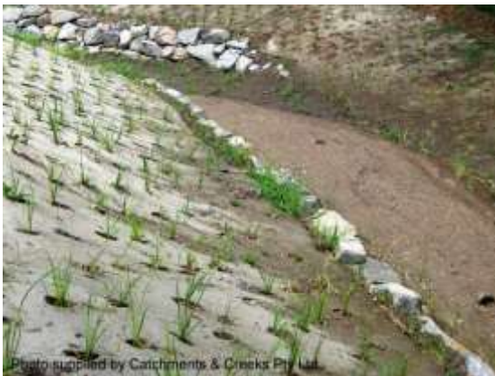
Inside bank with toe protection (Qld)
