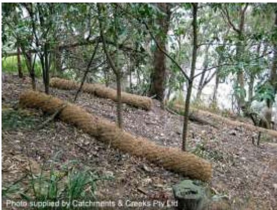
Geo logs placed on a creek bank (Qld)
