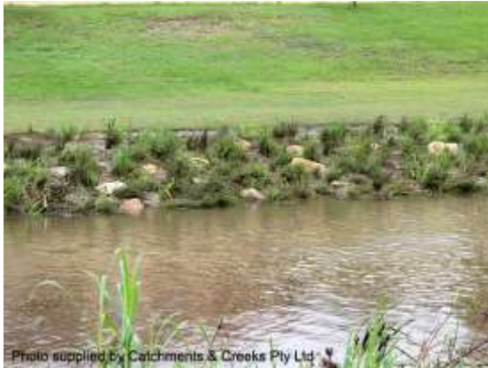
Vegetated rock stabilisation (Qld)
