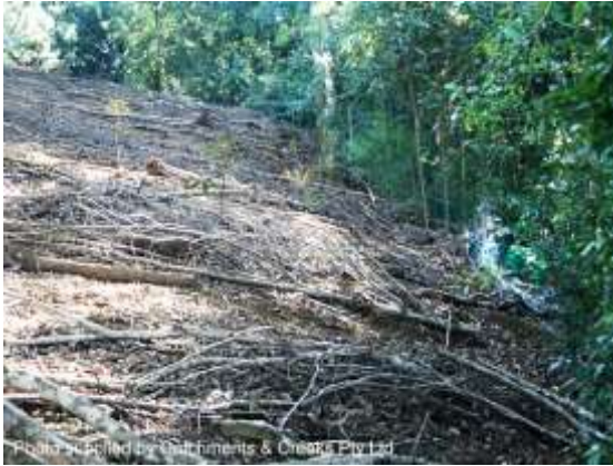
Brushing of overbank area (Qld)
