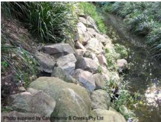
Placed rock bank stabilisation (Qld)
