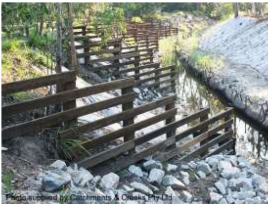
Timber groynes (Qld)
