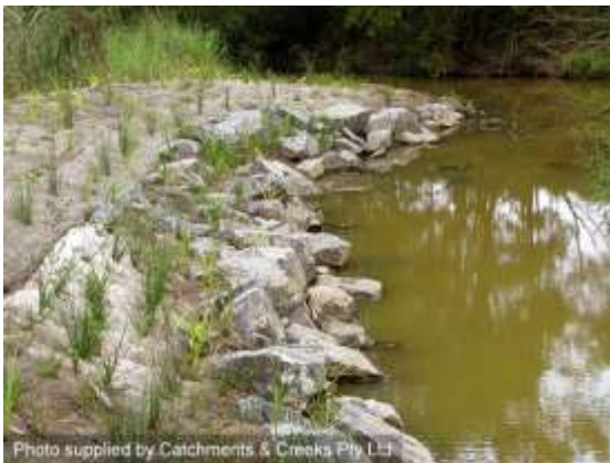
Vegetated rock stabilisation (Qld)
