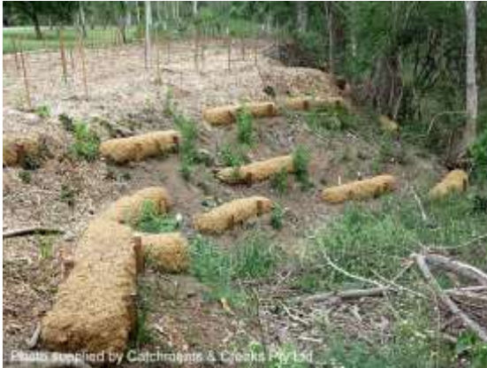
Geo logs placed on a creek bank (Qld)
