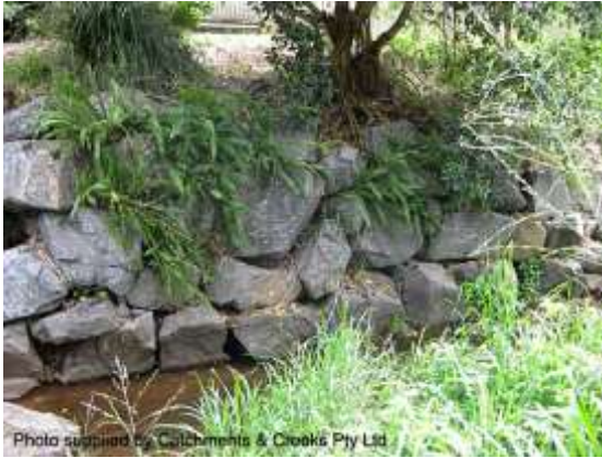
Stacked boulder wall (Qld)
