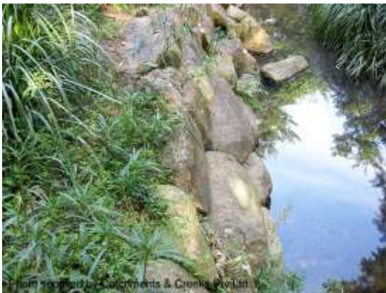
Stacked boulder wall (Qld)
