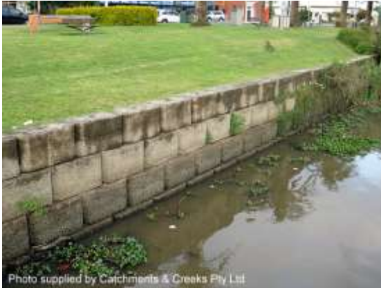
Retaining wall (NSW)
