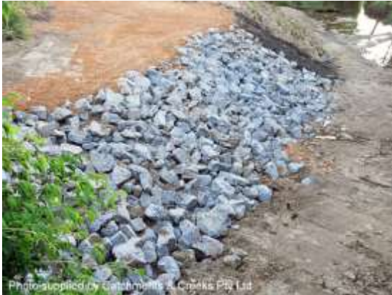
Rock stabilisation pre-planting (Qld)
