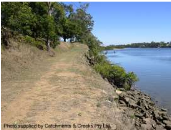
Benching of a river bank (Qld)
