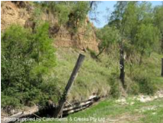
Old benched brushwood stabilisation (Qld)
