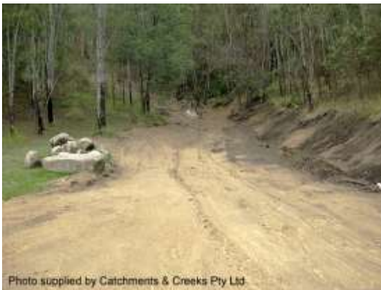
Treated slope prior to planting (Qld)
