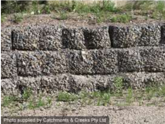
Gabion retaining wall (Qld)
