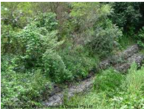
Vegetated gabion wall (Qld)
