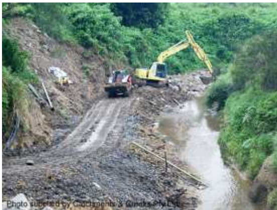
Equipment access (Qld)
