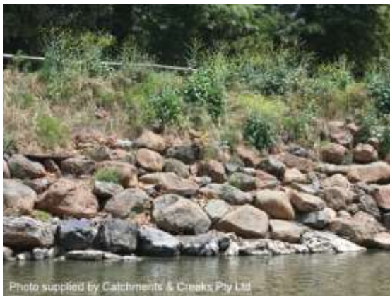
Vegetated rock stabilisation (NSW)
