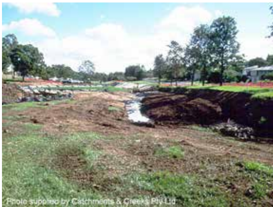
Construction phase, May 2000
