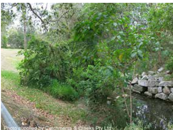
Looking downstream from outlet (2014)
