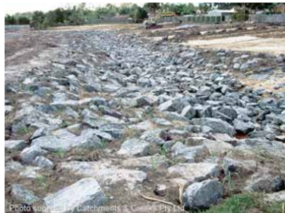
Sewer pipe crossing (1999)
