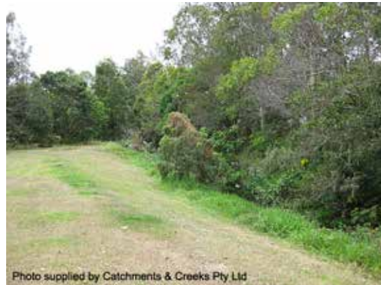
Looking d/s just d/s from the outlet (2014)
