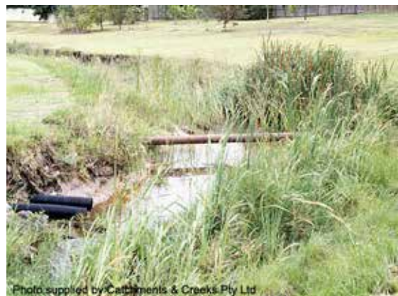
Exposed Ag-pipe & sewer crossing (1997)
