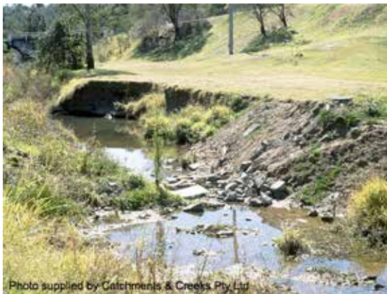
Protection of sewer with rubble (1991)
