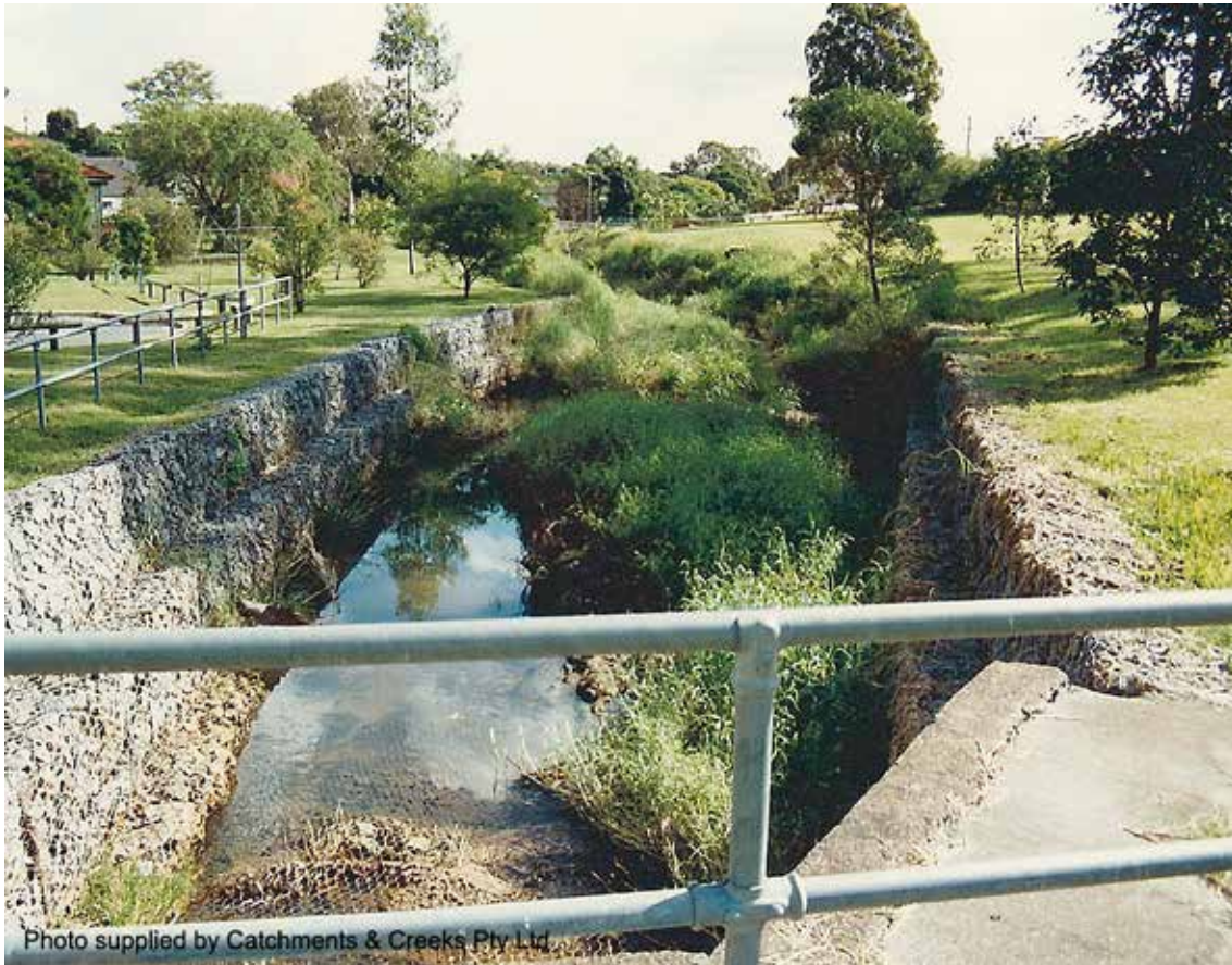
Looking downstream from the main stormwater outlet (pre-works, 1996)
