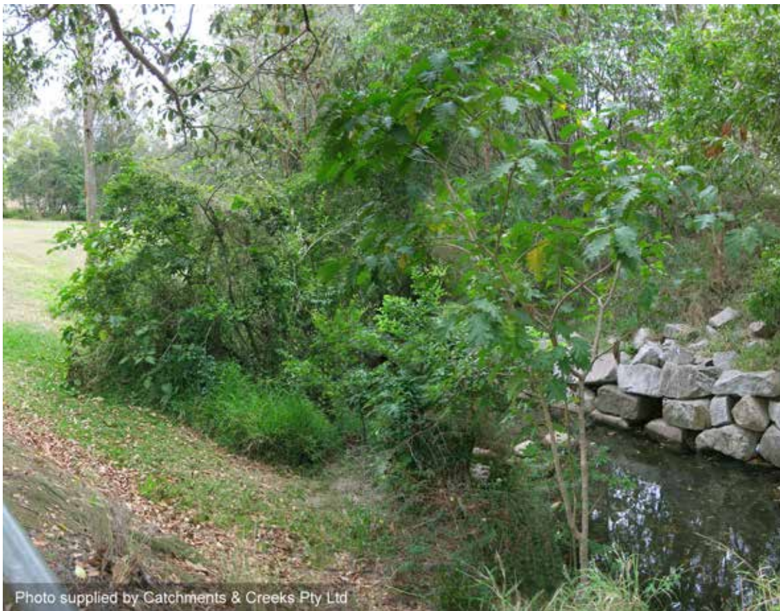
Looking downstream from the main stormwater outlet (2014)
