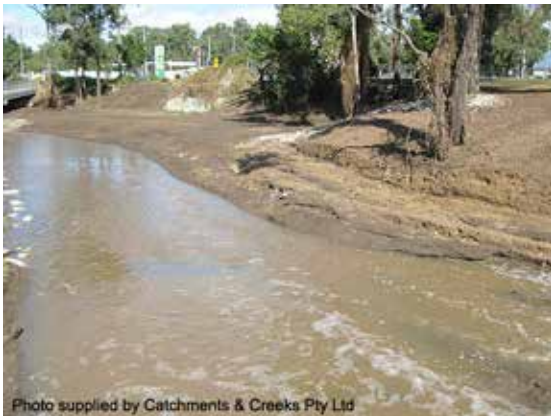
Downstream of Ferny Way (May, 2009)
