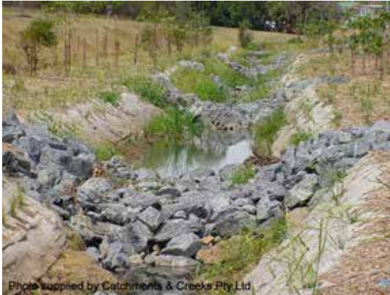
Constructed pool-riffle system (2001)
