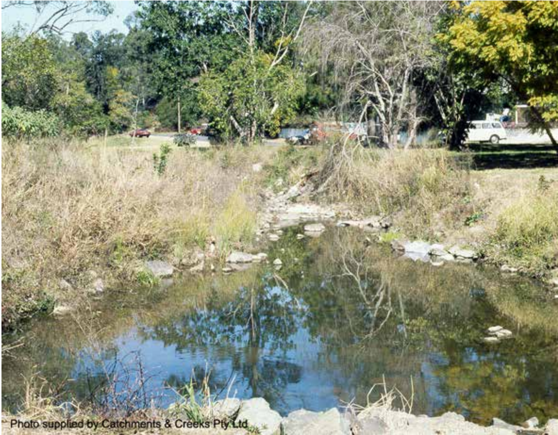
Looking downstream from the Moggill Road culvert (1991)
