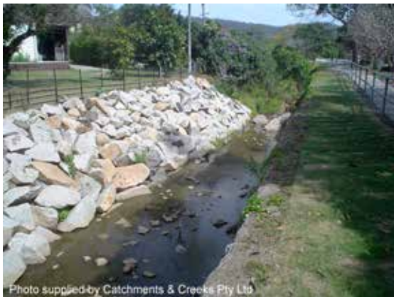
Upstream end of works (2005)
