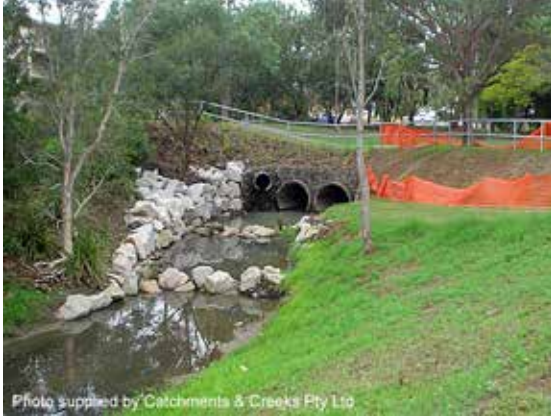
Looking downstream from outlet (2005)
