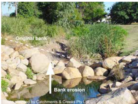
Bank erosion adjacent rock riffle (2002)
