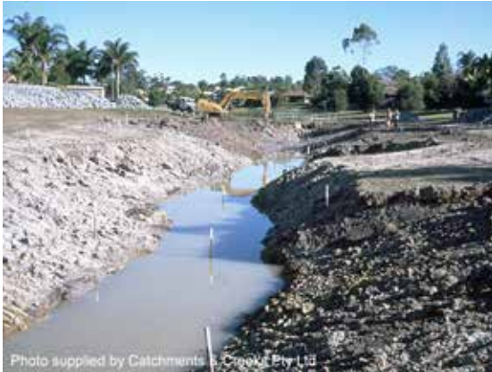
Looking u/s, construction phase (1999)
