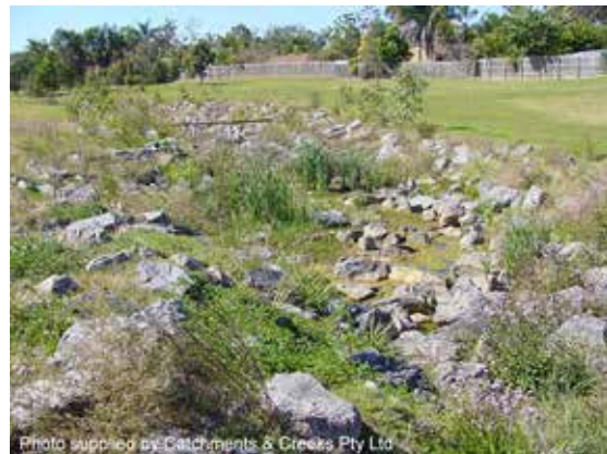
Sewer pipe crossing (2000)
