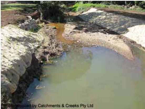
Looking d/s from footbridge (Aug, 2009)
