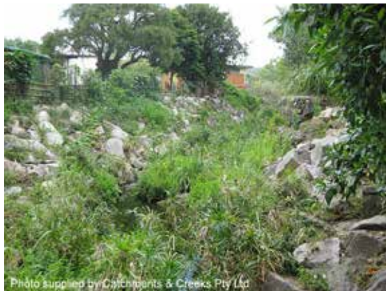
Upstream end of works (2012)
