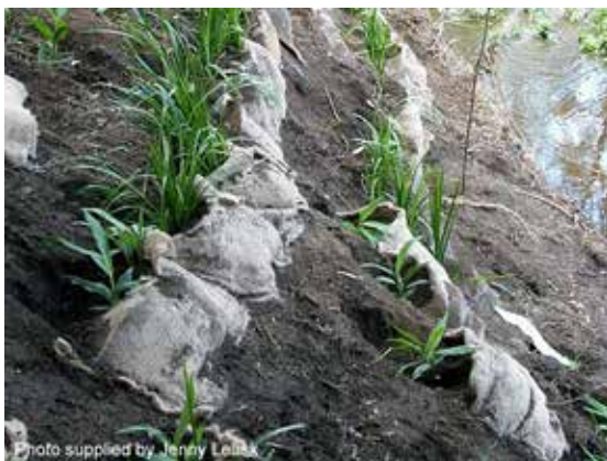
Jute bagging planting technique (2005)
