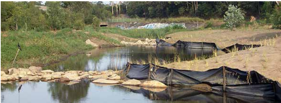
Looking downstream to culvert (2001)
