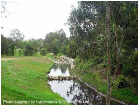
Looking d/s just d/s from the outlet (2005)
