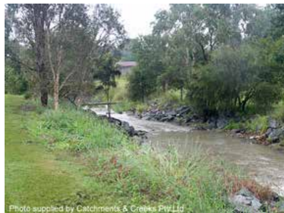
Sewer pipe crossing (2010)
