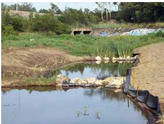
Looking downstream to culvert (2001)
