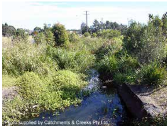
Looking down drainage channel (2007)
