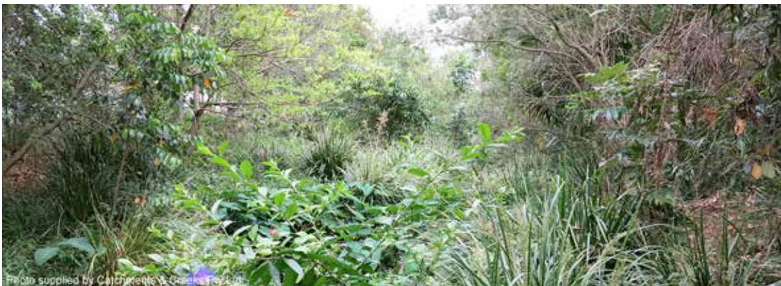
Looking downstream to culvert (2014)
