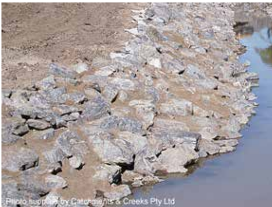
Soil-filled voids ready for planting (1999)
