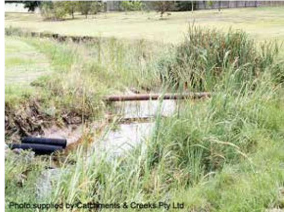
Sewer pipe crossing (1997)
