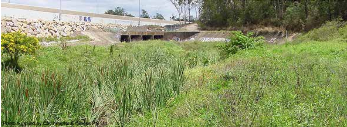
Looking downstream to culvert (2000)
