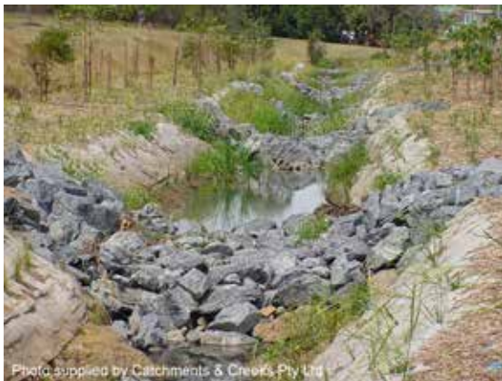
Pool-riffle system (looking upstream)
