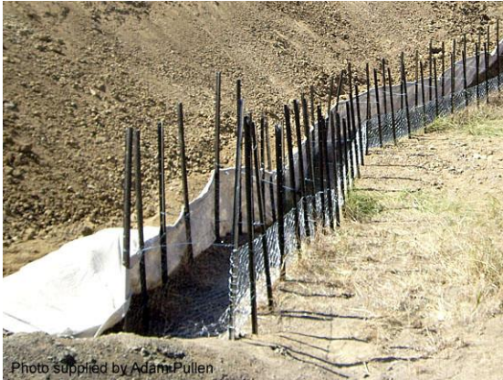
Installation of a sediment weir (Qld)
