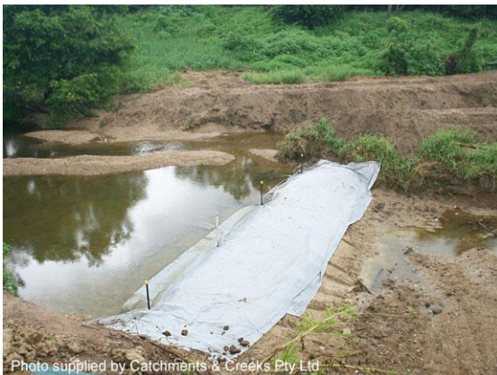
Cofferdam covered in filter cloth (Qld)
