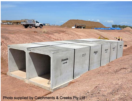
Culvert construction in a dry channel (NT)
