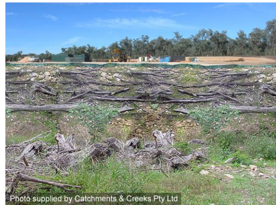
Brushwood used to stabilise a batter
