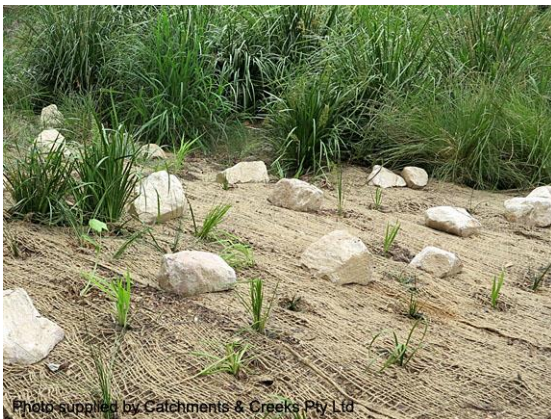
Jute mesh with additional rock anchors
