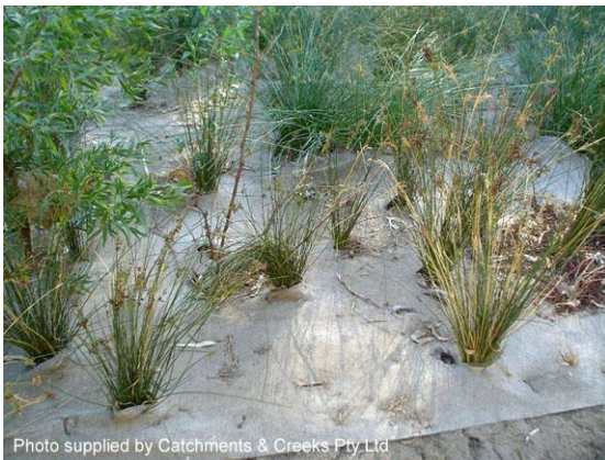
Jute erosion control blanket
