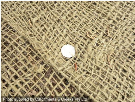
Jute mesh pinned to a creek bank
