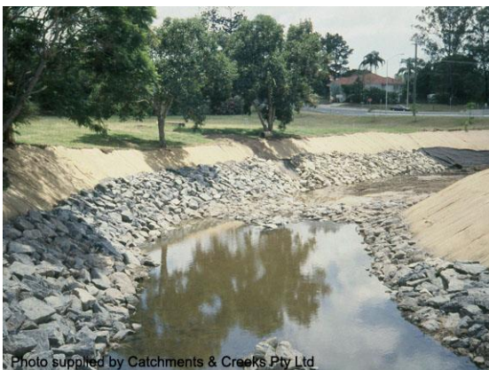
Rock stabilisation on channel bend
