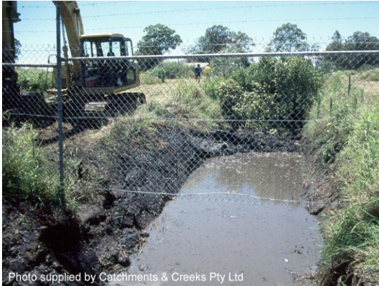
De-silting a storm drain outlet (Qld)
