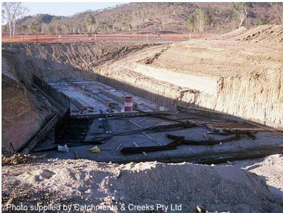
Construction of a culvert base slab (Qld)
