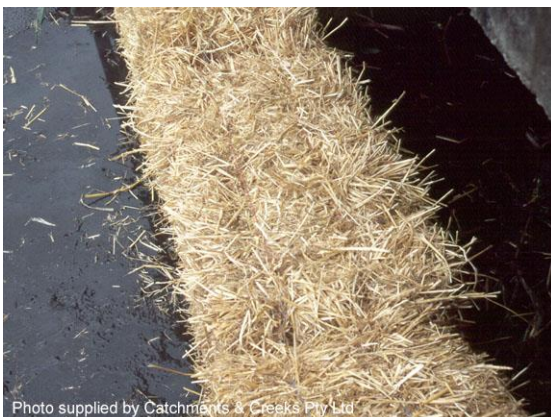
Straw bale flow diversion bank (Qld)
