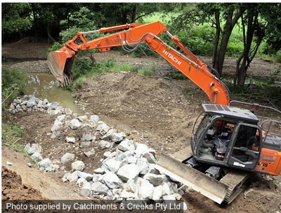
Placement of rock (November 2015)
