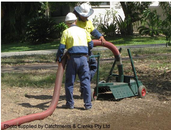
Mulch/compost flow diversion berm (Qld)
