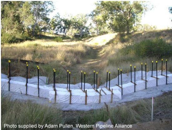
Modular barrier in an overland flow path
