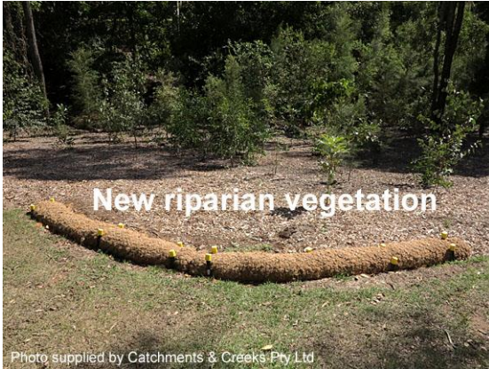
Coir logs protect new plants (Qld)
