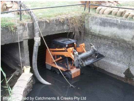
De-watering the storm drain
