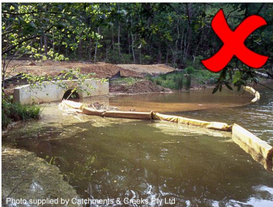
Construction of a stormwater outlet (USA)
