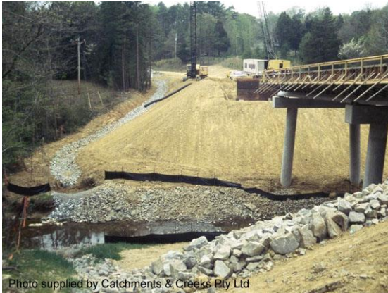
Bridge construction (USA)
