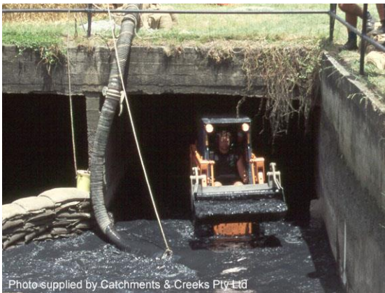
Sediment removed from the storm drain
