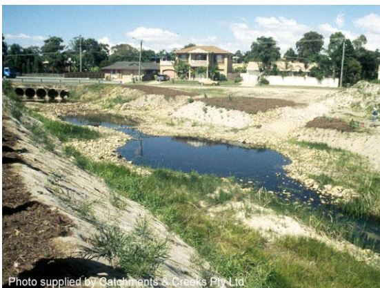
Permanent sediment extraction ponds
