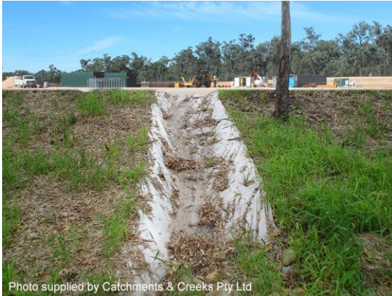
Temporary drainage chute (Qld)
