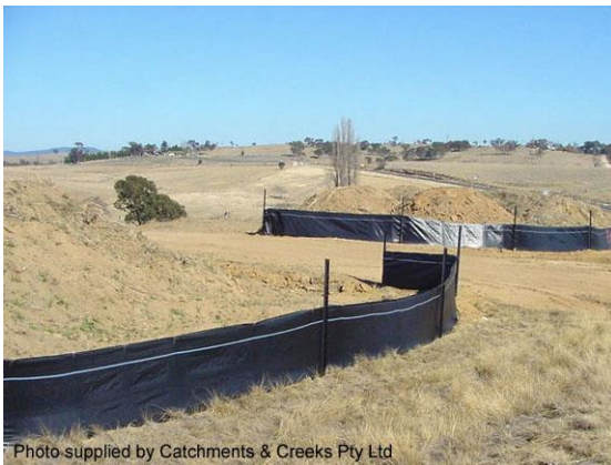
Sediment control down-slope of stockpile
