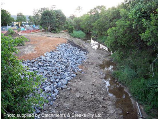
Downstream rock stabilisation
