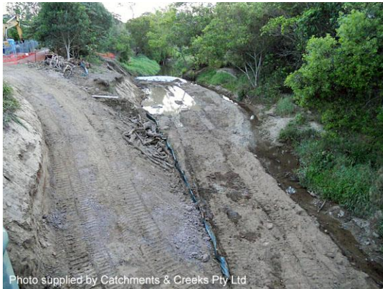
Isolation of the work area
