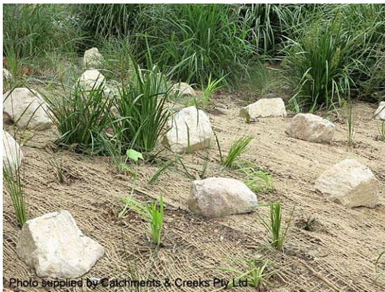
Jute mesh anchored with rocks
