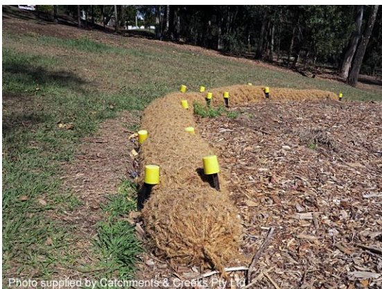
Temporary flow diversion bank (Qld)
