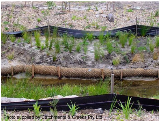
Toe protection (NSW)
