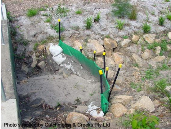
Sed-fence used during drain maintenance
