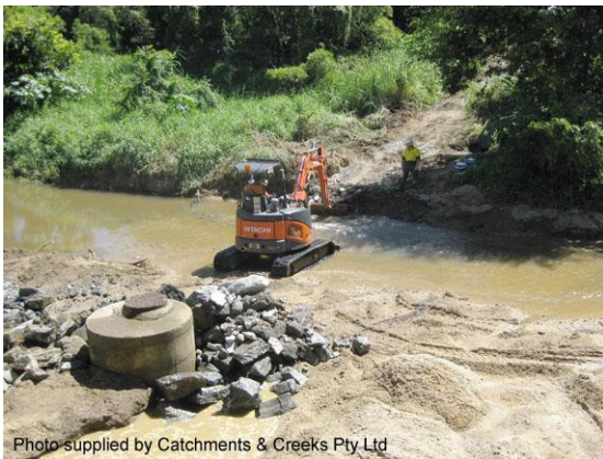
Maintenance of in-channel sewer pit
