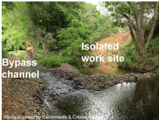
Bypass channel in a gravel-based creek
