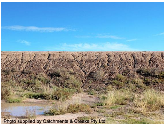
Rilling that extends to top of bank
