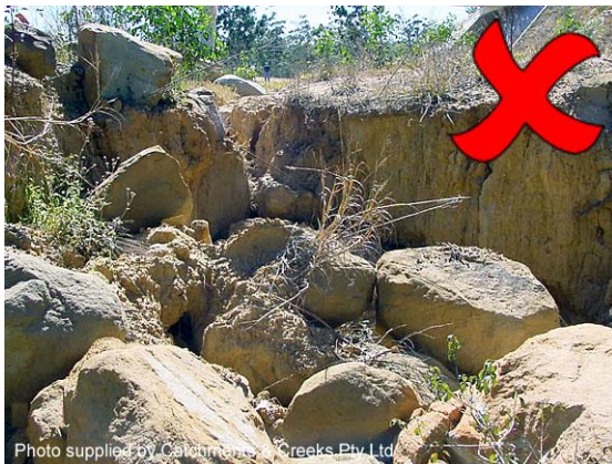
Collapsed dispersive soil bank
