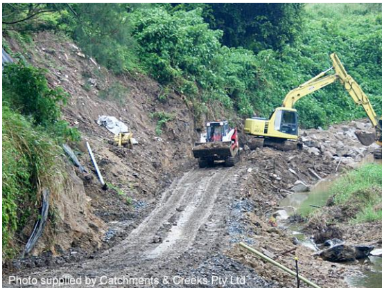
A bench formed to allow vehicle access
