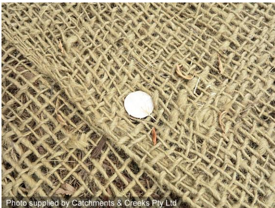
Jute mesh pinned to a creek bank
