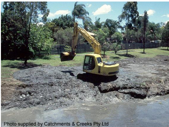
Excavated material placed on creek bank
