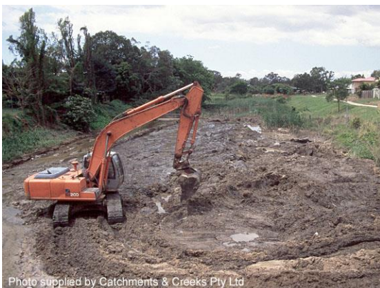
Creek de-silting (Qld)
