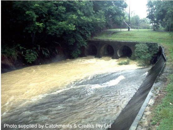
Sediment-laden stormwater runoff
