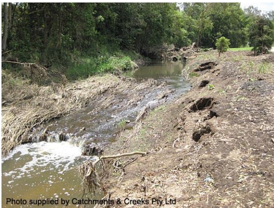
Post November 2008 flood
