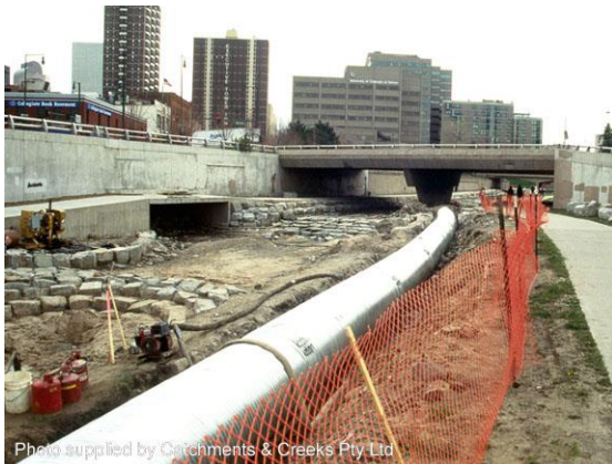
Stream flows pass through the steel pipe
