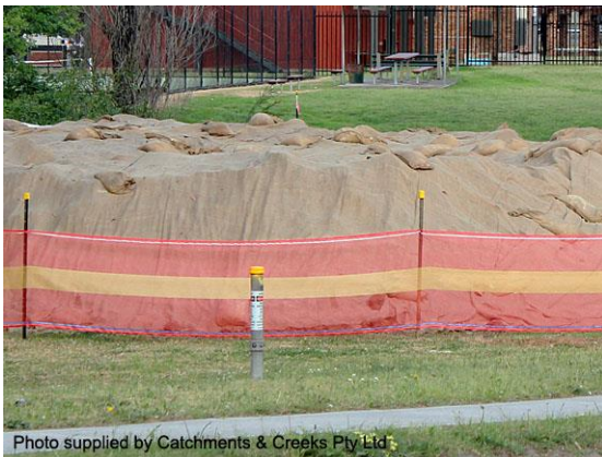
Soil stockpile covered with hessian (NSW)
