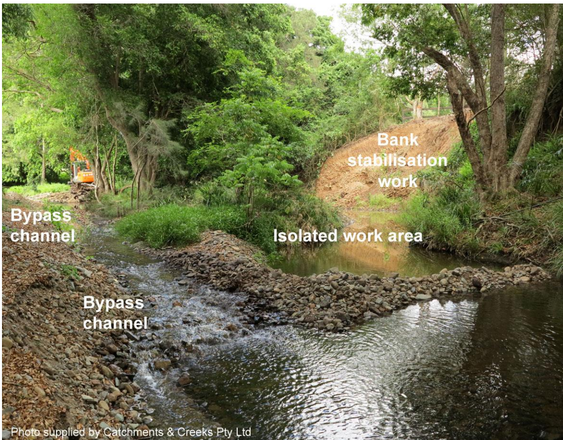
Cedar Creek with the bypass channel on the left and the work site on the right
