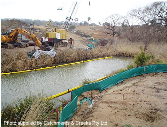
Bridge construction (NSW)
