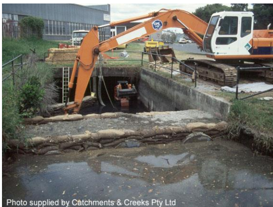
Cofferdam with tide gates (Qld)
