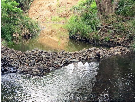
Rock filter dam downstream of work area
