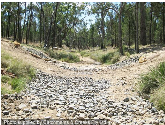
Rock stabilised vehicle crossing
