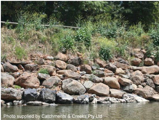
Partial vegetated bank stabilisation
