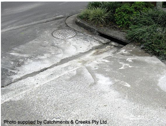
Cement runoff from a work site
