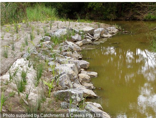
Vegetated rock stabilisation of bank
