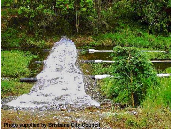
Filter tube embankment (Qld)
