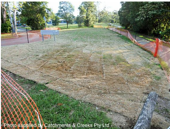
Turfing of overbank disturbance
