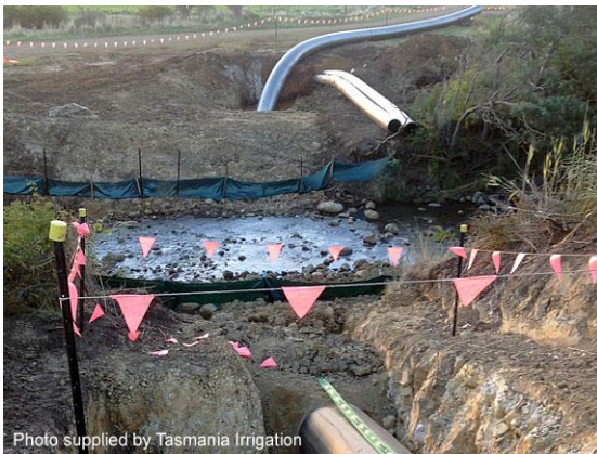
Pipeline installation (Tasmania Irrigation)
