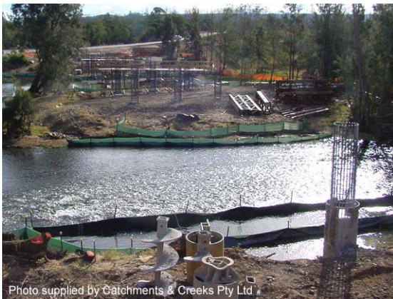
Photo supplied by Catchments & Creeks Pty Ltd Bridge construction (NSW)
