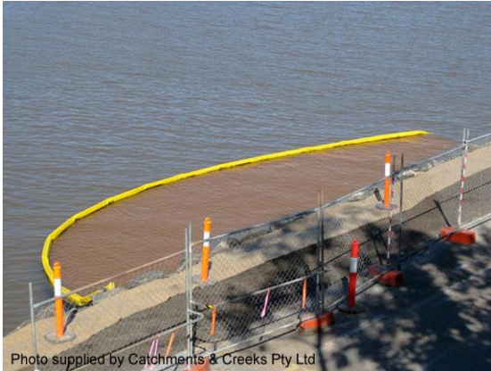
Riverwall repairs (Qld)
