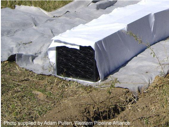
Modular sediment barrier being installed
