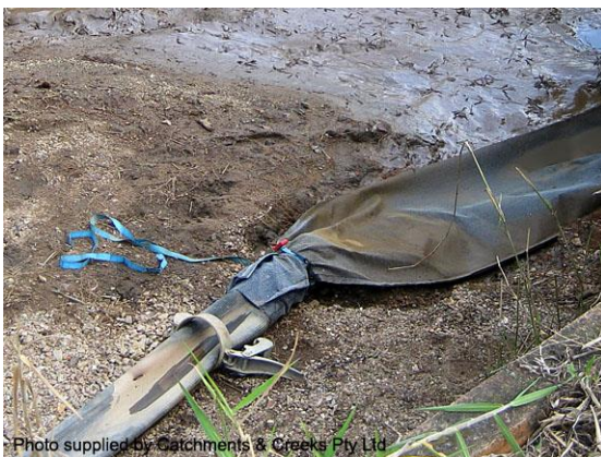
Water pumped directly into a filter tube
