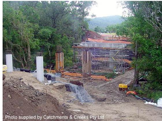
Bridge construction (Qld)
