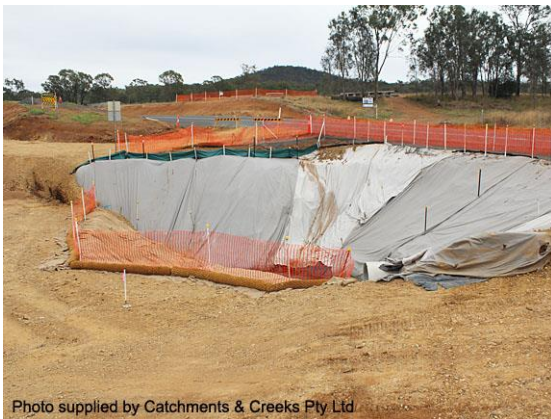
Embankment stabilised with filter cloth
