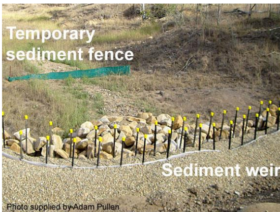
Sediment fence in an overland flow path
