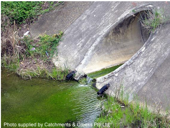
Inflow of nutrient-rich stormwater runoff
