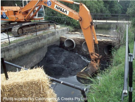
Sediment stockpiled inside the drain
