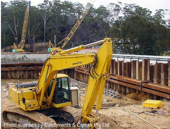
Sheet piling isolation barrier (NSW)
