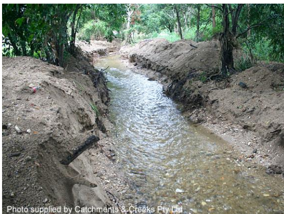
Bypass cut through a sandy bench (Qld)
