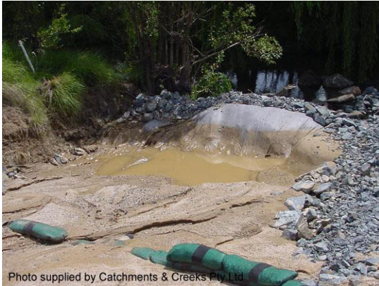
Type 2 (off-stream) sediment trap (NSW)
