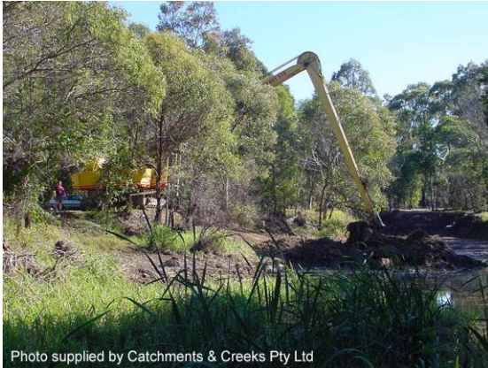
Channel maintenance (Qld)
