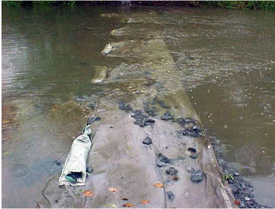
Flows overtop a rock filter dam (Qld)
