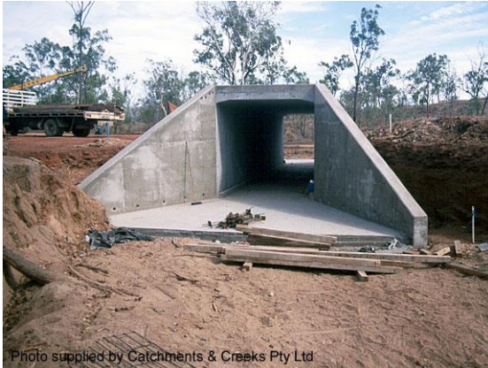
Culvert construction in a dry creek bed
