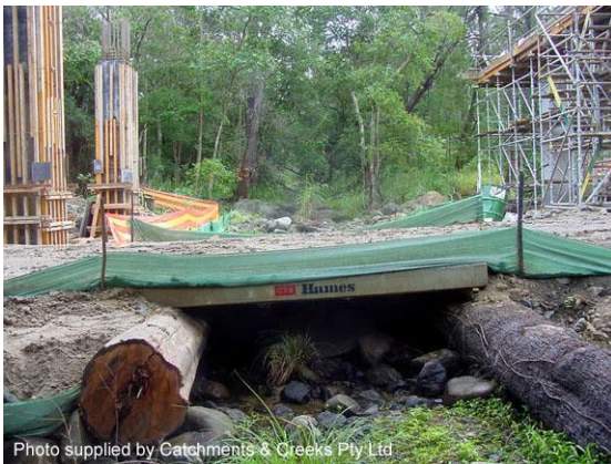
Temporary access construction bridge
