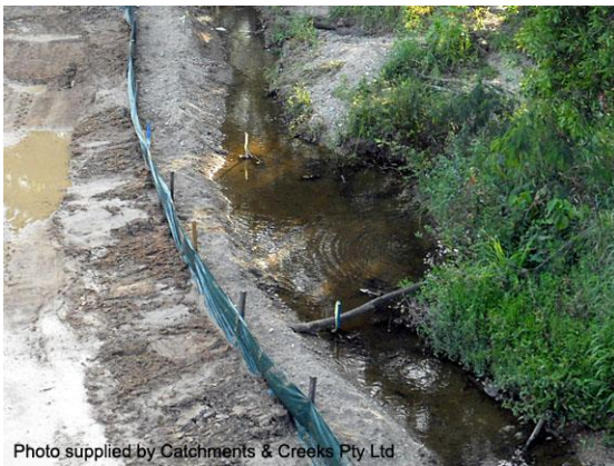
Sediment fence isolation barrier
