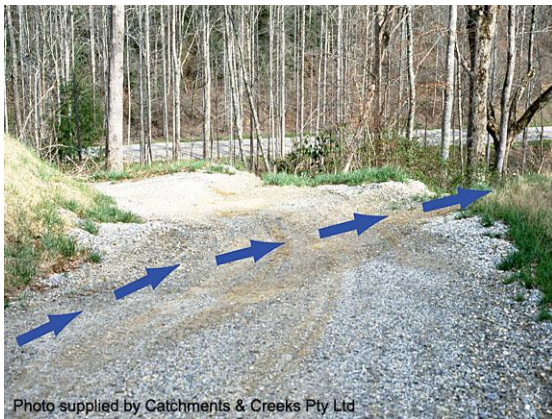
Flows diverted off access track
