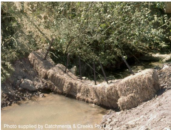
Temporary straw bale barrier
