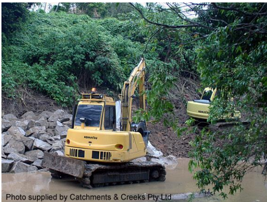
Rock placement on a creek bank
