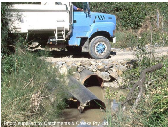
Temporary pipe culvert (Qld)
