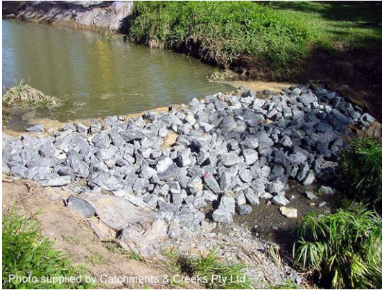
Rock filter dam (Qld)
