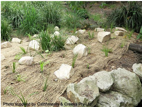
Jute mesh with additional rock anchors
