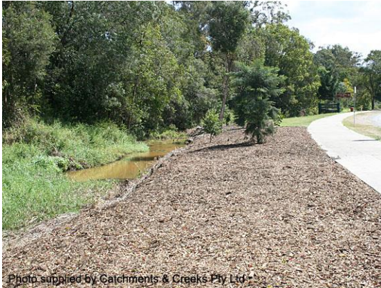
Vegetation clearing and weed removal
