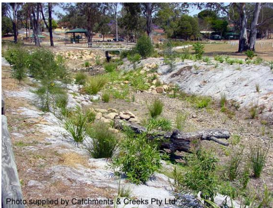
Constructed drainage channel (Qld)
