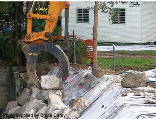
Rock placement over filter cloth (Qld)
