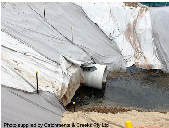
Filter cloth stabilisation of a cofferdam
