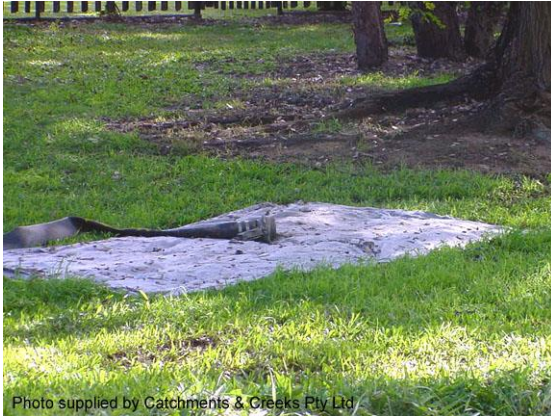
Pump discharging onto filter cloth
