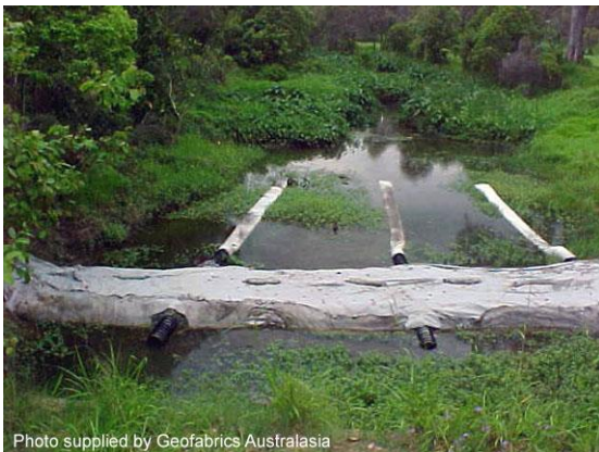
Instream filter tube sediment trap (Qld)
