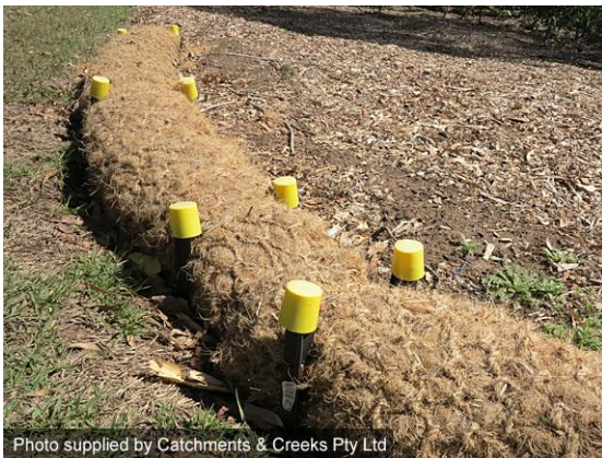
Temporary flow diversion bank (Qld)
