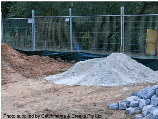
Sediment fence down-slope of stockpiles
