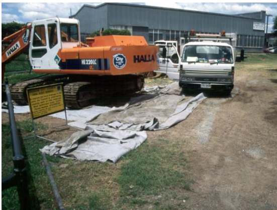
Truck loading area
