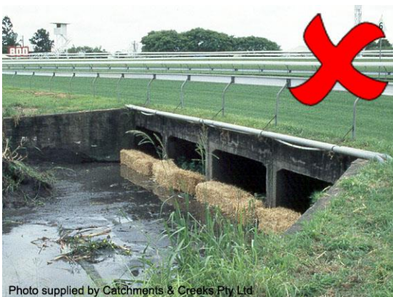
Straw bales placed on a concrete apron
