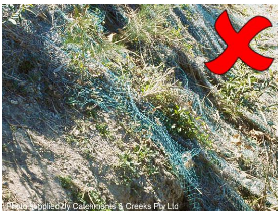
Synthetic reinforced erosion control mat
