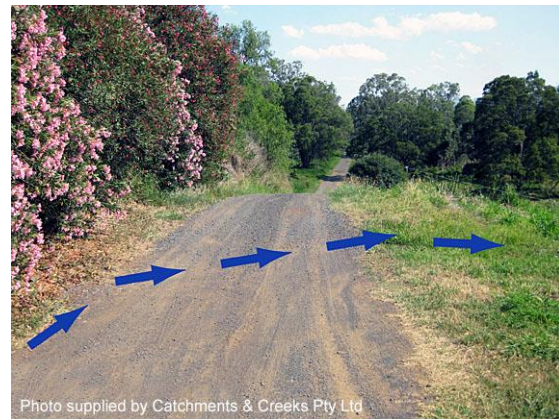
Cross bank placed at top of descent
