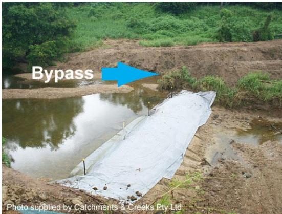
Earth cofferdam with bypass channel (Qld)
