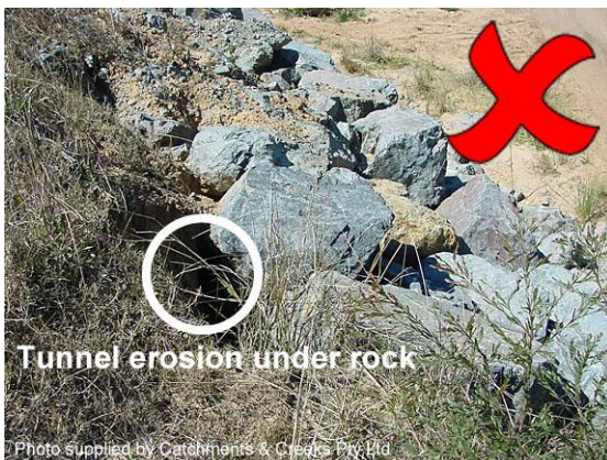
Tunnel erosion under rocks
