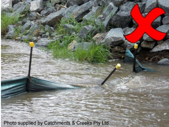
Failed sediment fence (north of NSW)
