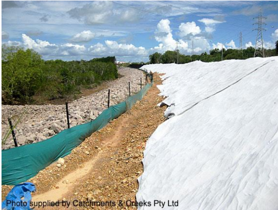
Long-term stockpile cover with filter cloth
