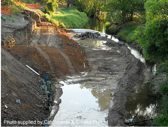
Reconstruction of the eroded bank
