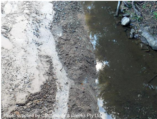
Flow diversion berm
