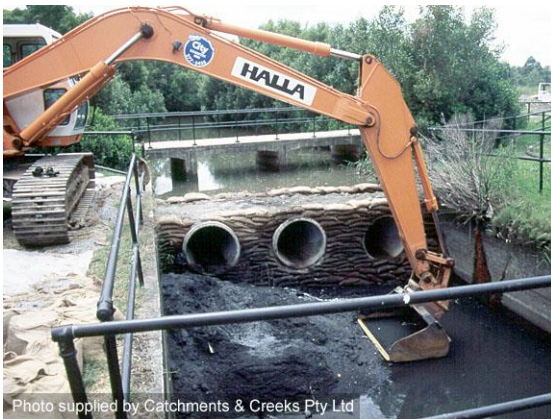
A cofferdam isolates the work area
