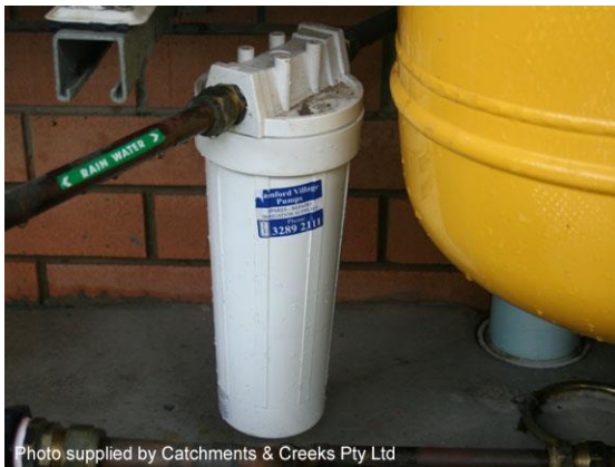
Cartridge filter (rainwater filter)
