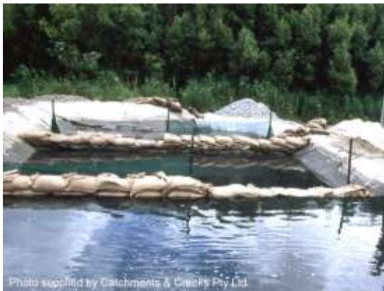
Outflow from the settling pond
