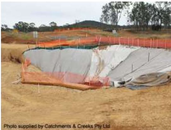
Embankment stabilised with filter cloth
