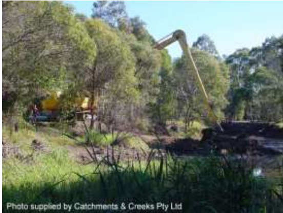
Channel maintenance (Qld)
