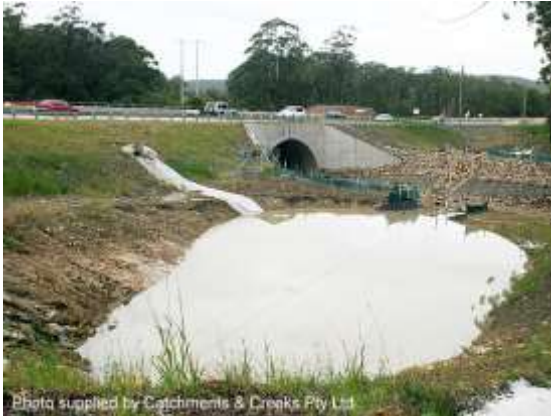
Sediment basins (Type 1 sediment trap)
