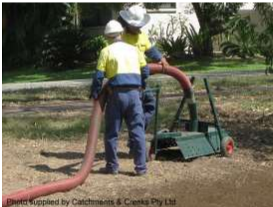
Mulch/compost flow diversion berm (Qld)
