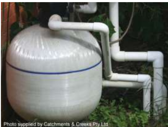
Sand filter (swimming pool filter)
