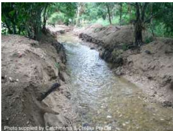
Bypass cut through a sandy bench (Qld)
