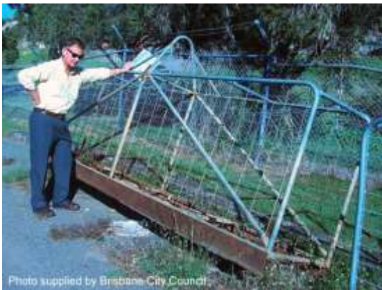
Sediment filter cage (Qld)
