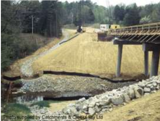
Bridge construction (USA)
