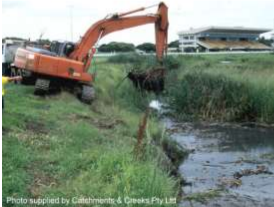
De-silting a storm drain (Qld)
