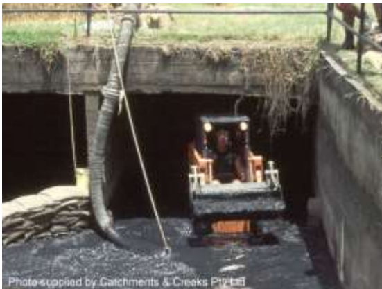
Sediment removed from the storm drain
