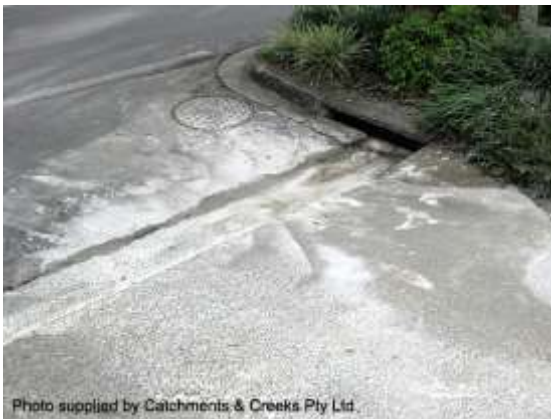
Cement runoff from a work site
