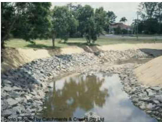
Rock stabilisation on channel bend
