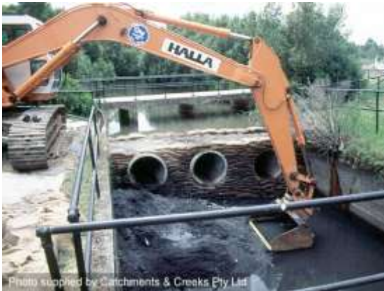
A cofferdam isolates the work area
