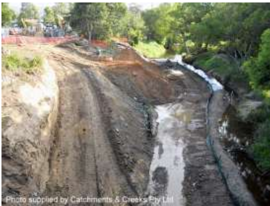
Diversion of stream flows (Qld)
