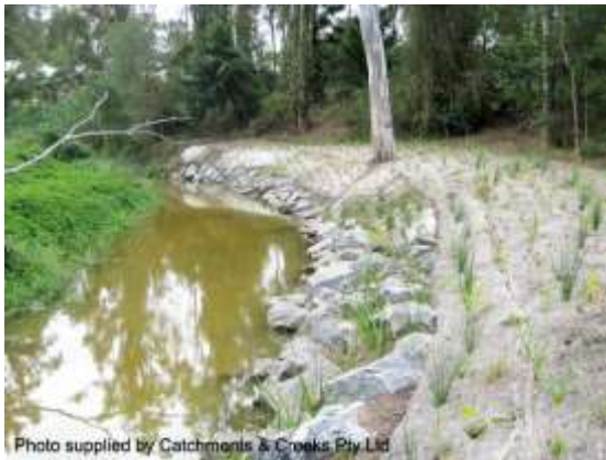
Plants integrated into rock protection (Qld)
