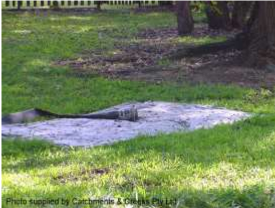
Pump discharging onto filter cloth
