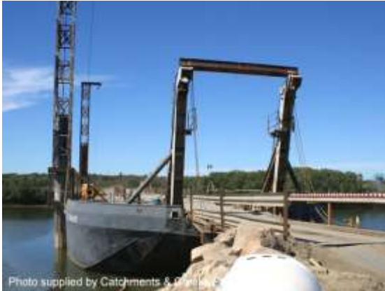
Photo supplied by Catchments & Creeks Pty Ltd Barge acting as a bridge crossing (Qld)
