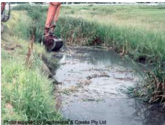
De-silting an urban creek (Qld)
