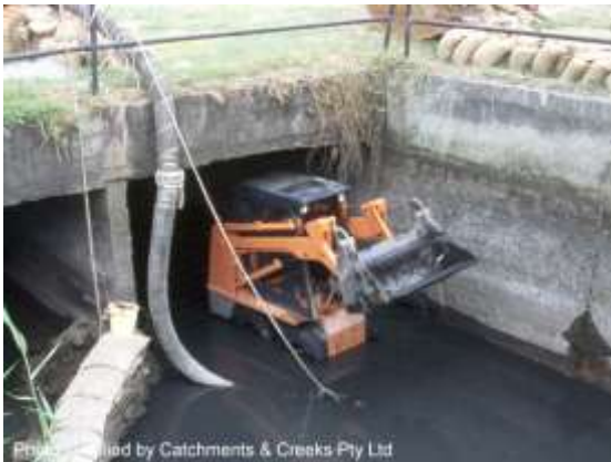
De-watering the storm drain
