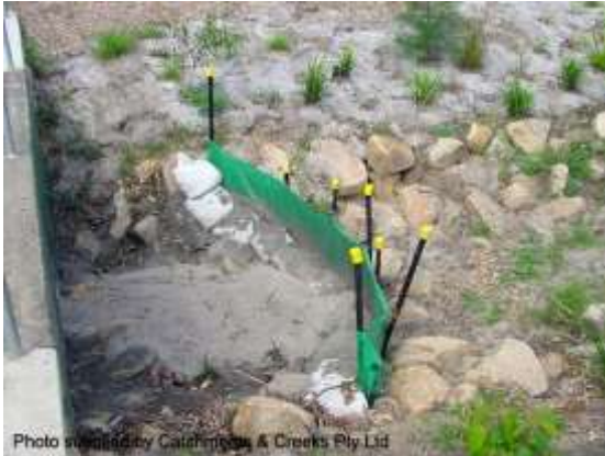
Sed-fence used during drain maintenance
