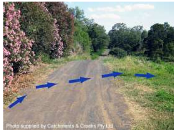
Cross bank placed at top of descent
