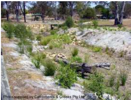
Constructed drainage channel (Qld)
