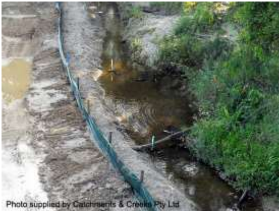
Sediment fence isolation barrier
