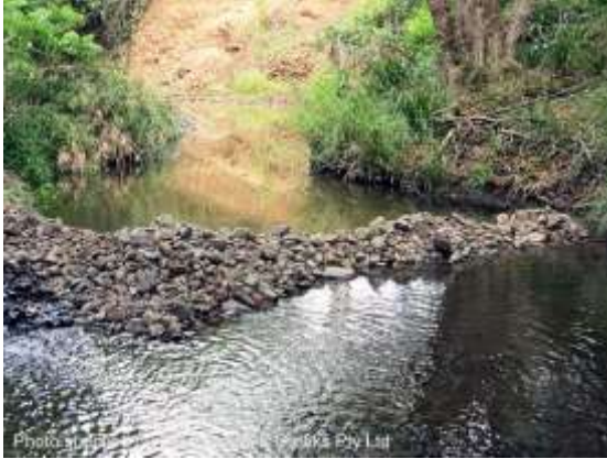
Rock filter dam downstream of work area
