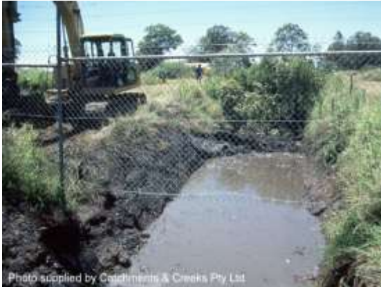
De-silting a storm drain outlet (Qld)
