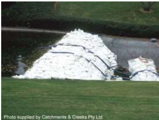
Sandbag cofferdam (USA)
