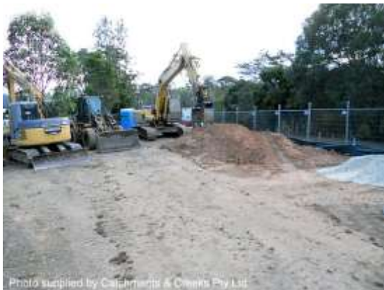
Site office and stockpile area
