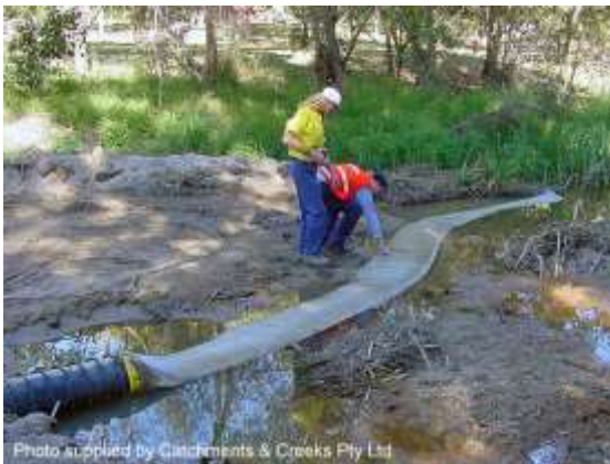
Use of a filter tube to treat water (Qld)
