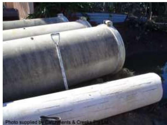
Standpipe (foreground) prior to installation
