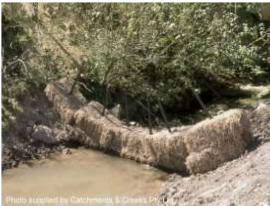
Temporary straw bale barrier
