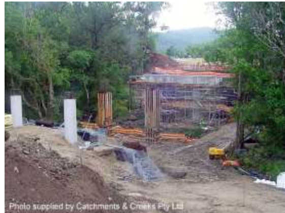
Bridge construction (Qld)
