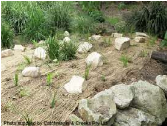
Jute mesh with additional rock anchors
