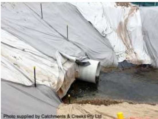
Filter cloth stabilisation of a cofferdam
