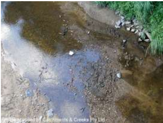
Removal of rock filter dam
