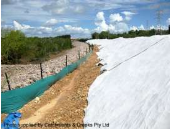
Long-term stockpile cover with filter cloth
