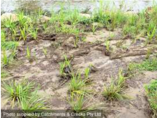
Flood damage to site revegetation
