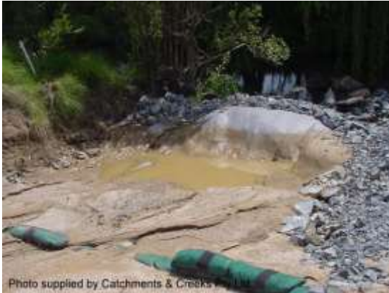
Type 2 (off-stream) sediment trap (NSW)
