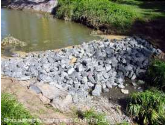
Rock filter dam (Qld)
