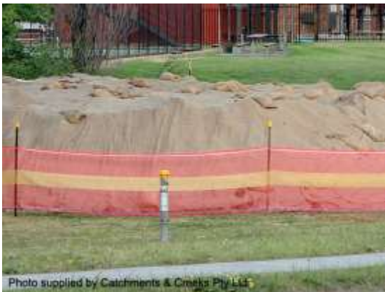
Soil stockpile covered with hessian (NSW)
