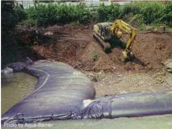
Isolation barrier (HSI Services, USA)
