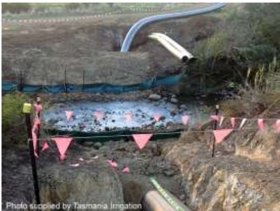
Pipeline installation (Tasmania Irrigation)
