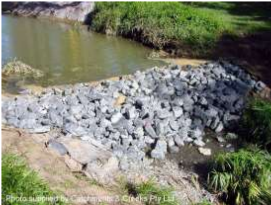
Rock filter dam (Qld)
