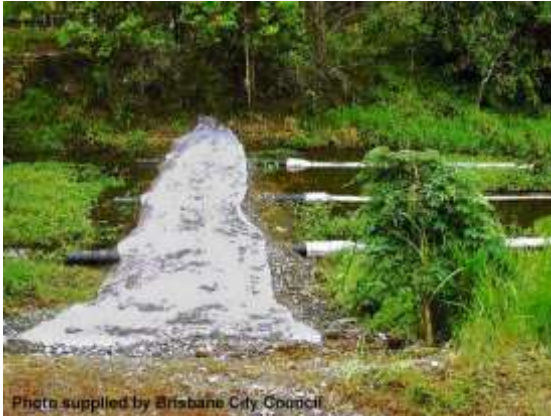
Filter tube embankment (Qld)
