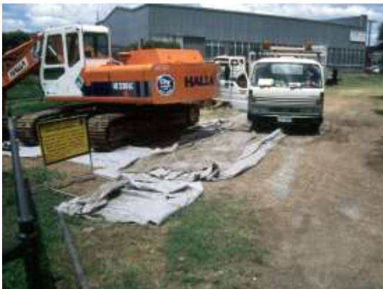
Truck loading area
