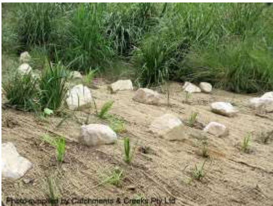
Jute mesh with additional rock anchors
