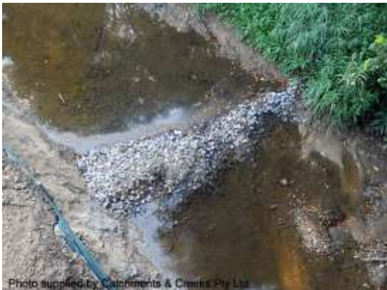
Rock filter dam
