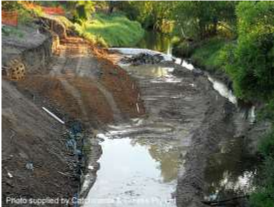
Reconstruction of the eroded bank
