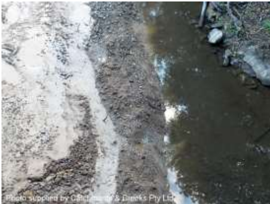
Flow diversion berm
