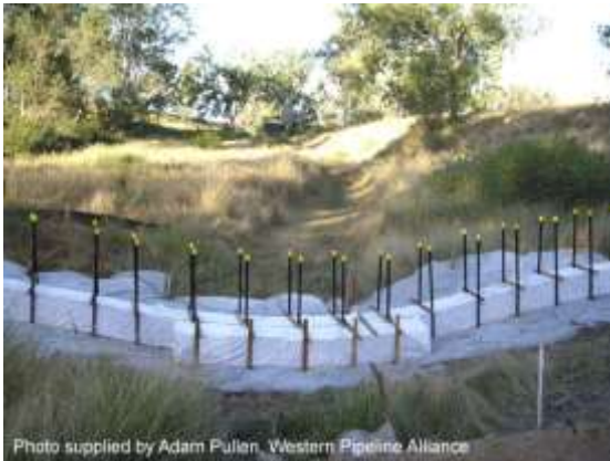
Modular barrier in an overland flow path
