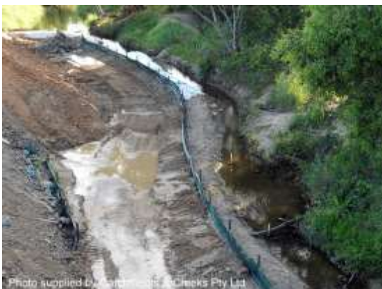
Flow diversion system (Qld)
