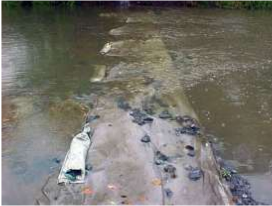
Flows overtop a rock filter dam (Qld)
