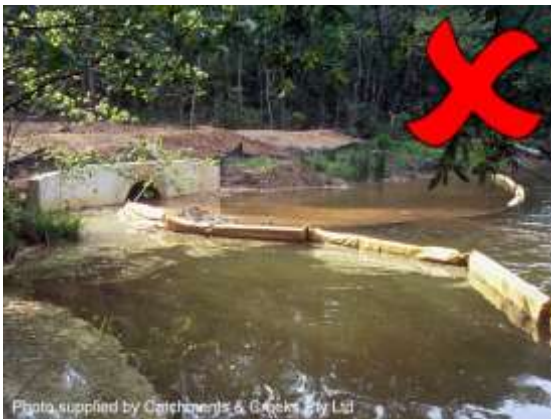
Construction of a stormwater outlet (USA)
