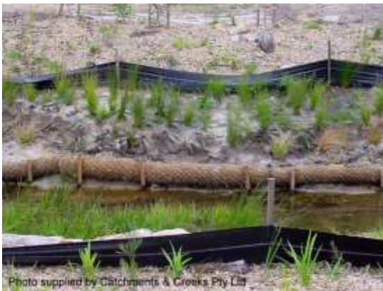
Toe protection (NSW)
