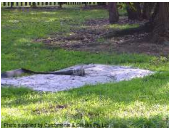
Pumping water to a grass filter bed
