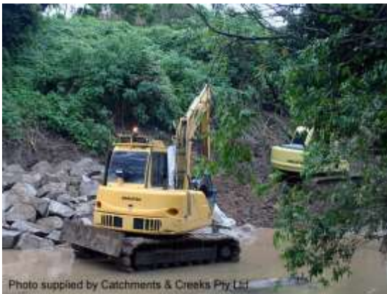
Rock placement on a creek bank
