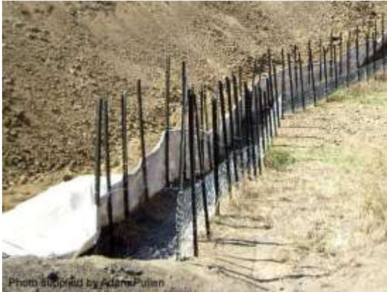
Installation of a sediment weir (Qld)
