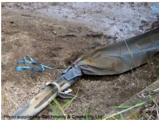
Water pumped directly into a filter tube
