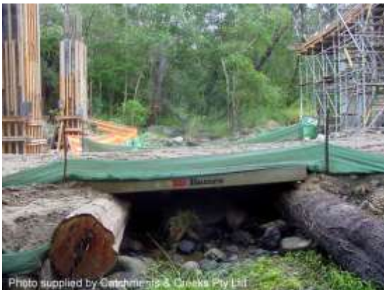
Photo supplied by Catchments & Creeks Pty Ltd Temporary access construction bridge
