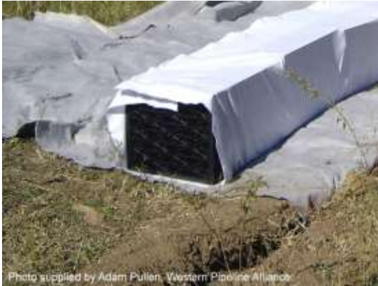
Modular sediment barrier being installed
