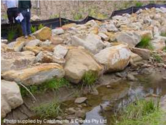
Larger rocks forming toe protection
