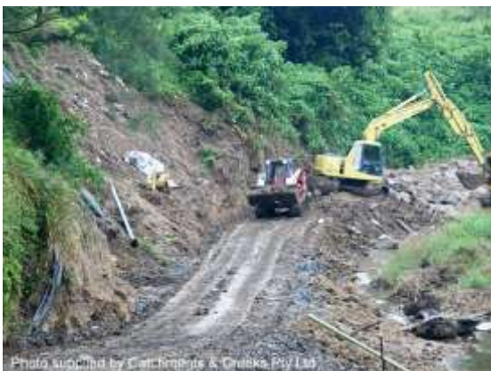
A bench formed to allow vehicle access
