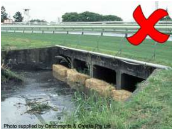
Straw bales placed on a concrete apron
