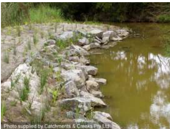
Vegetated rock stabilisation of bank
