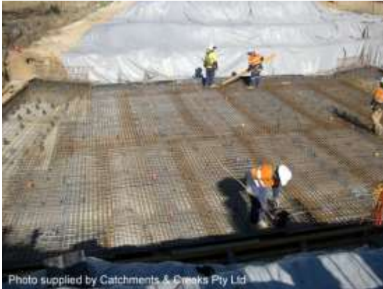
Construction of a culvert base slab (Qld)
