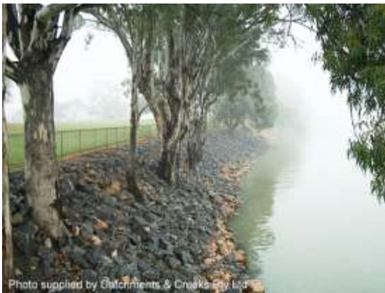
River bank stabilisation (NSW)
