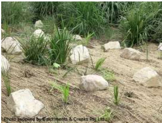
Jute mesh anchored with rocks
