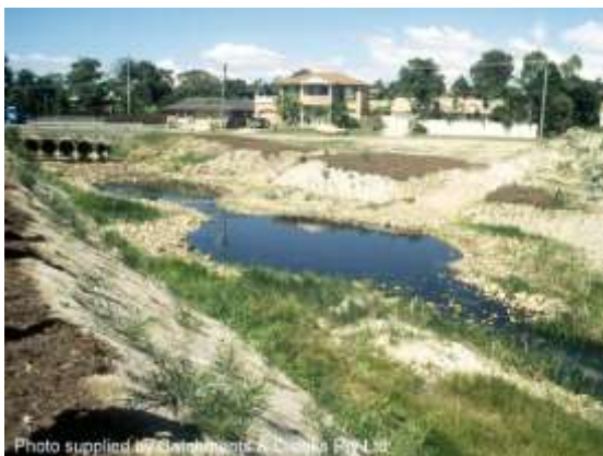
Permanent sediment extraction ponds
