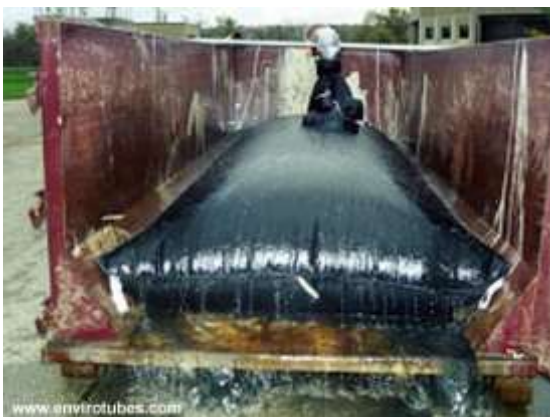
Filter bag contained in a rubbish skip
