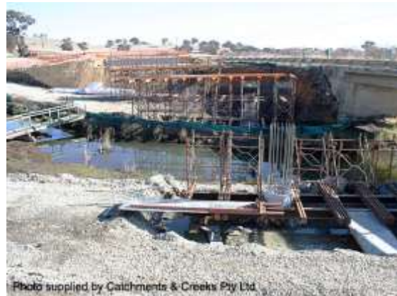
Bridge construction (NSW)
