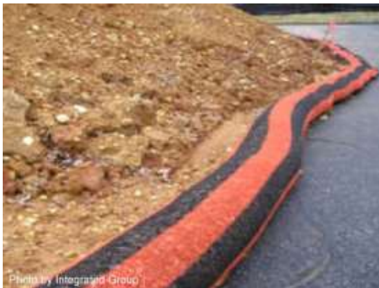
Type 2 sediment filter (compost berm)
