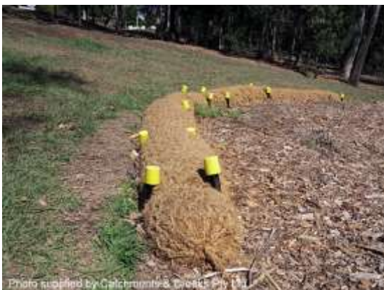
Temporary flow diversion bank (Qld)
