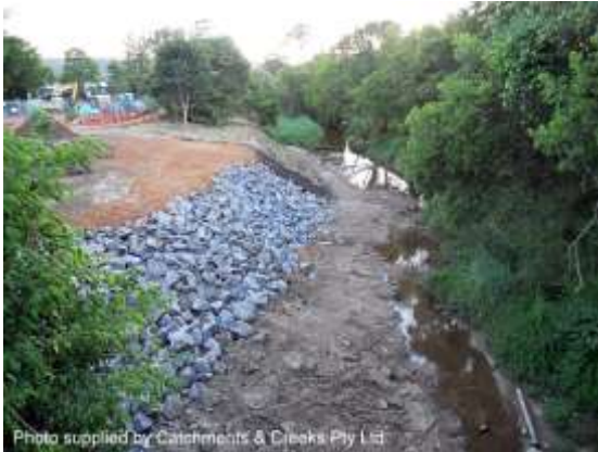
Downstream rock stabilisation
