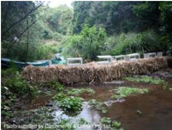
Straw bales placed on a rocky creek bed
