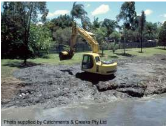
Excavated material placed on creek bank
