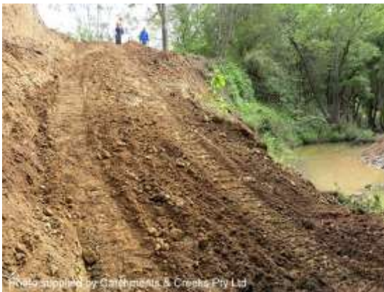
Access ramp down creek bank
