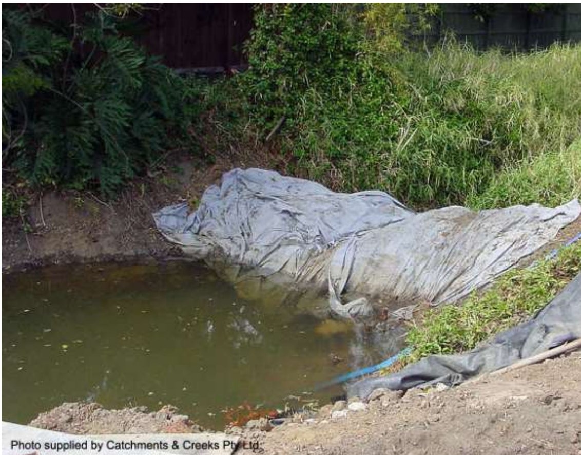
Rock filter dam wrapped in filter cloth (Qld)
