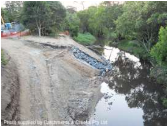
Upstream rock stabilisation
