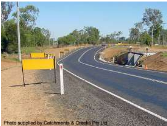
Temporary bypass road (Qld)
