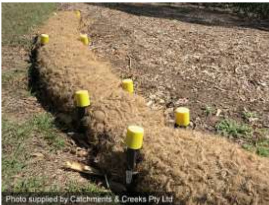
Temporary flow diversion bank (Qld)
