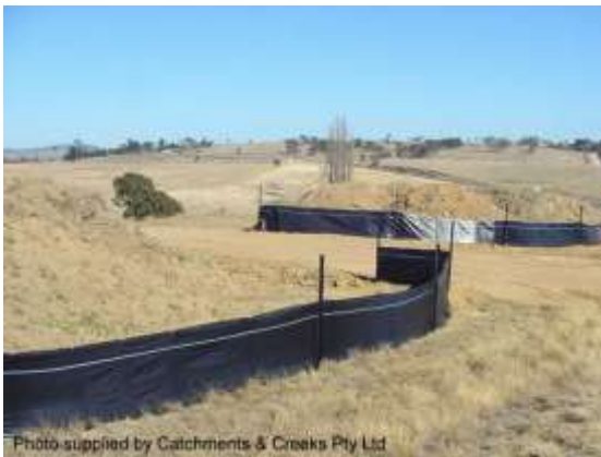
Sediment control down-slope of stockpile
