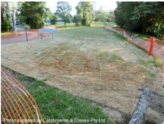
Turfing of overbank disturbance
