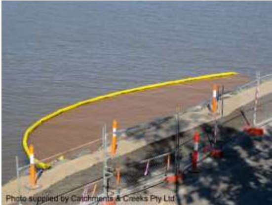
Riverwall repairs (Qld)
