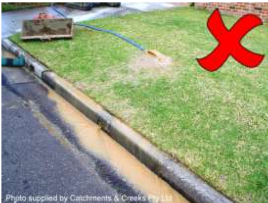
Sediment passes over saturated soil
