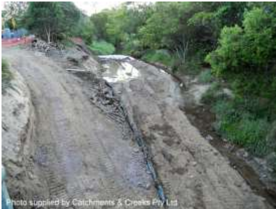
Isolation of the work area
