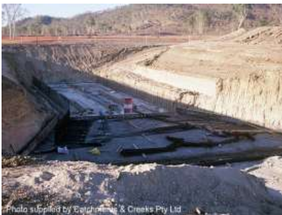
Construction of a culvert base slab (Qld)
