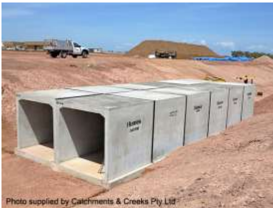
Culvert construction in a dry channel (NT)
