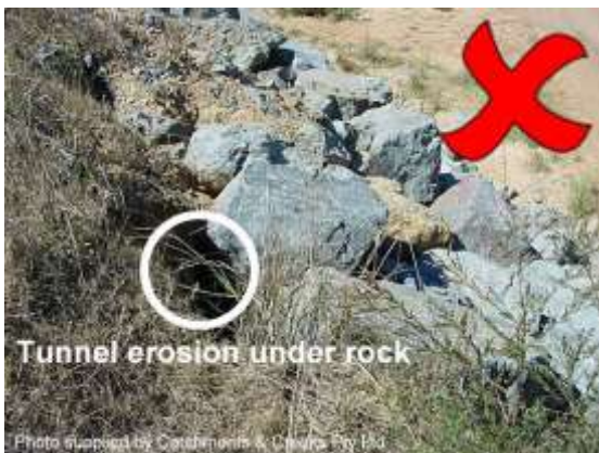
Tunnel erosion under rocks
