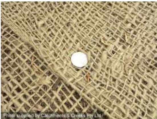
Jute mesh pinned to a creek bank
