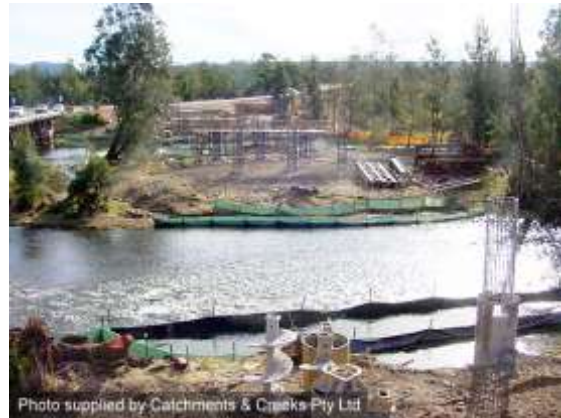
Bridge construction (NSW)
