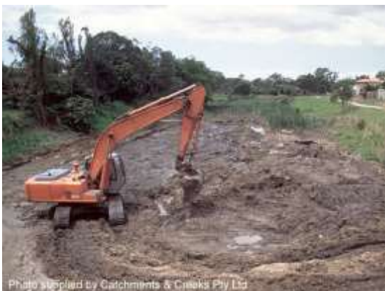
Creek de-silting (Qld)
