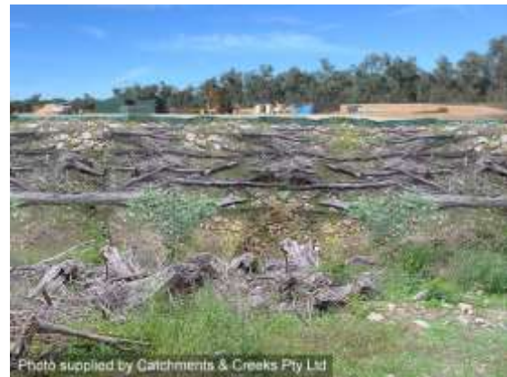
Brushwood used to stabilise a batter
