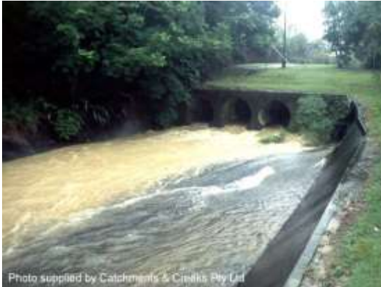
Sediment-laden stormwater runoff
