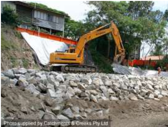
Photo supplied by Catchments & Creeks Pty Ltd Limited site access (Qld)
