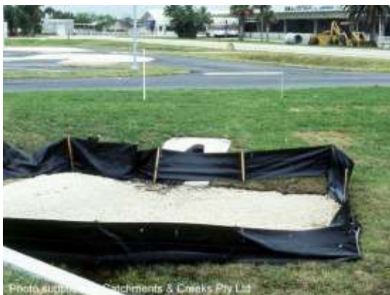
Gravel soakage (infiltration) pit (USA)
