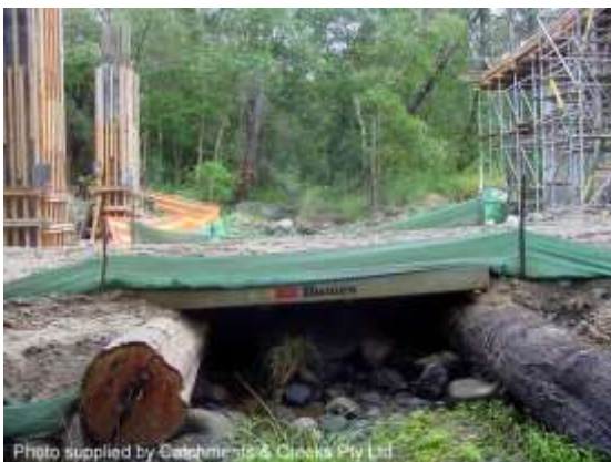
Temporary stream crossing (Qld)
