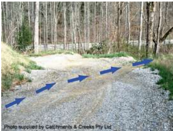
Flows diverted off access track
