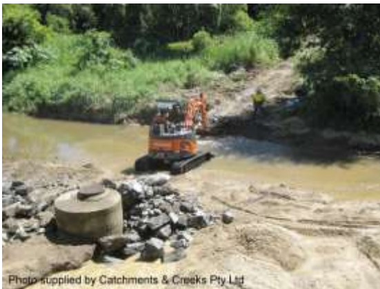
Maintenance of in-channel sewer pit
