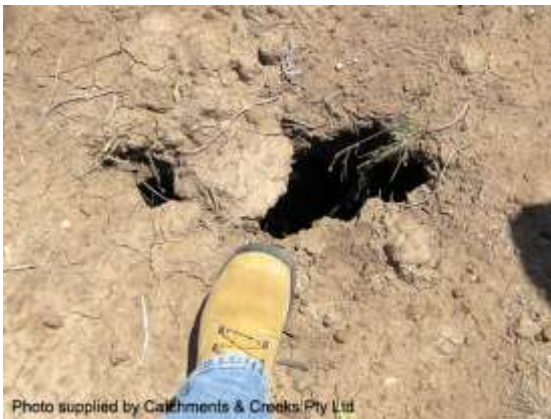
Deep rilling and tunnel erosion
