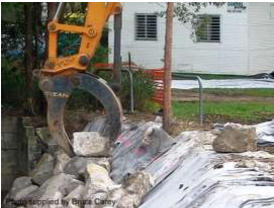
Rock placement over filter cloth (Qld)
