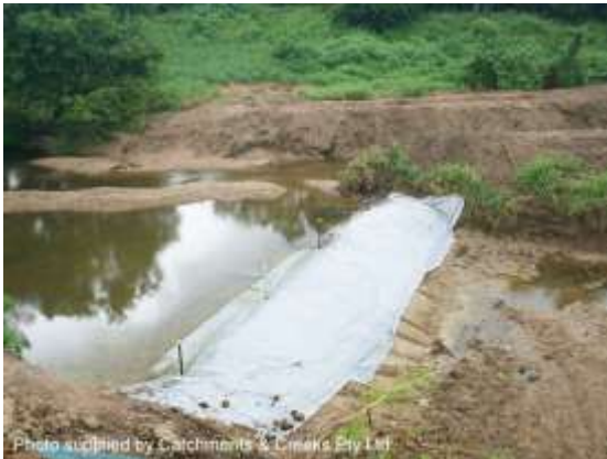
Cofferdam covered in filter cloth (Qld)
