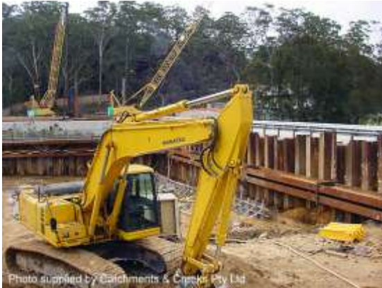
Sheet piling isolation barrier (NSW)
