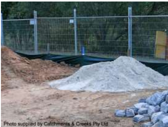
Sediment fence down-slope of stockpiles
