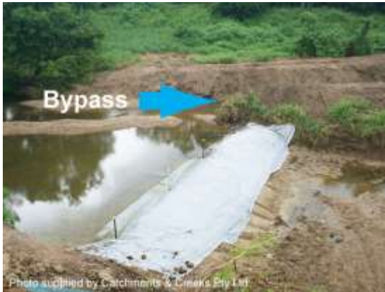
Earth cofferdam with bypass channel (Qld)
