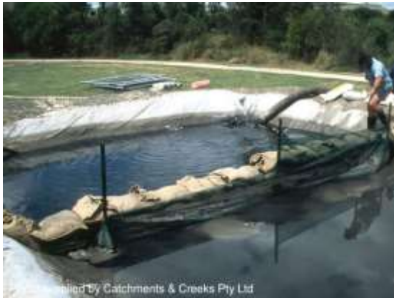
Stage 1 of settling pond (inlet)
