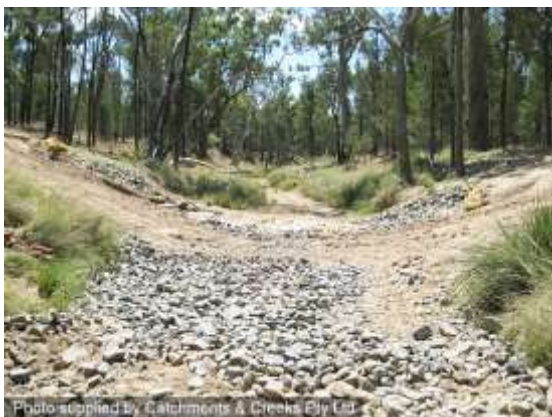
Rock stabilised vehicle crossing
