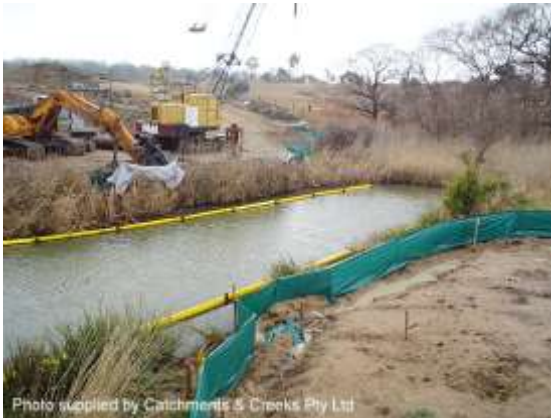
Sediment fence (Type 3 sediment trap)
