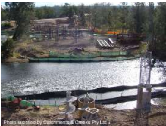
Bridge construction (NSW)
