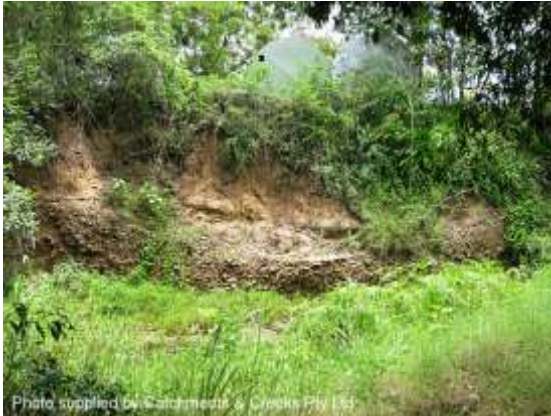
Bank scour (January 2015)
