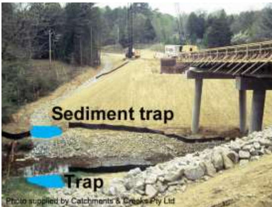
Rock filter dams (Type 2 sediment trap)
