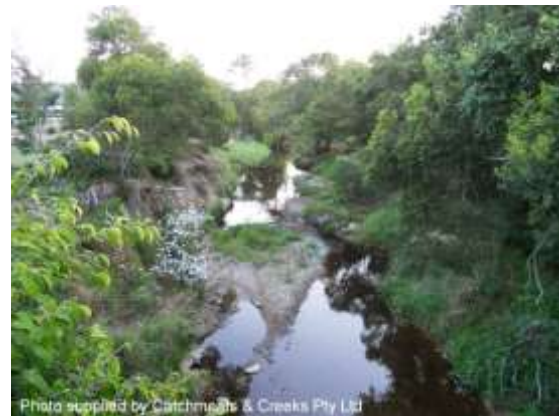
Erosion visible on the left bank, 2012
