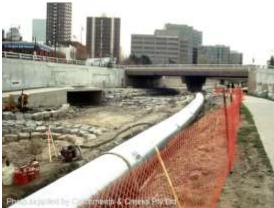
Stream flows pass through the steel pipe
