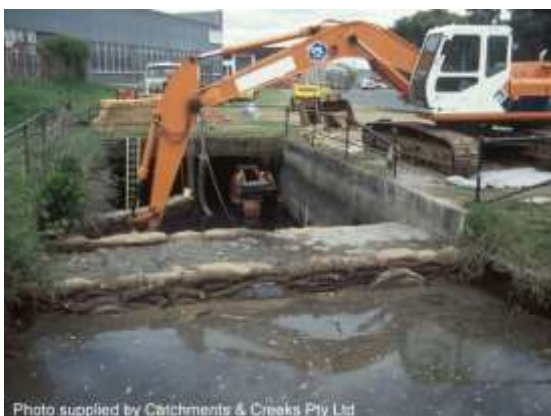
Cofferdam with tide gates (Qld)
