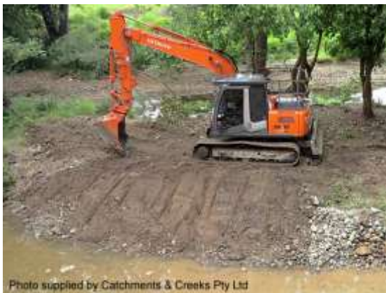
Trimming a creek bank prior to planting
