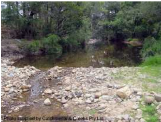
Constructed riffle u/s of a culvert (NSW)
