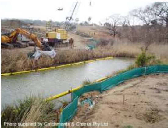
Bridge construction (NSW)
