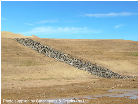
Rock-lined batter chute
