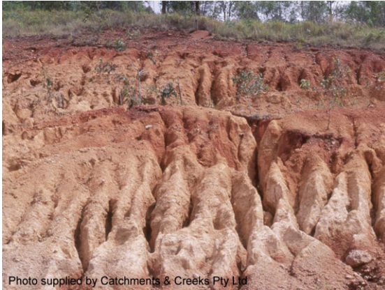
Erosion of a dispersive soil
