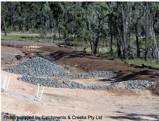
Velocity control check dams
