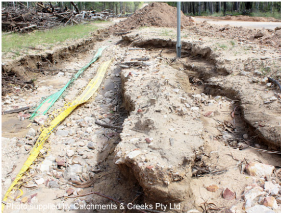
Erosion along a backfilled pipe trench
