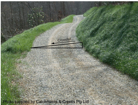
Gravel road with out-fall drainage
