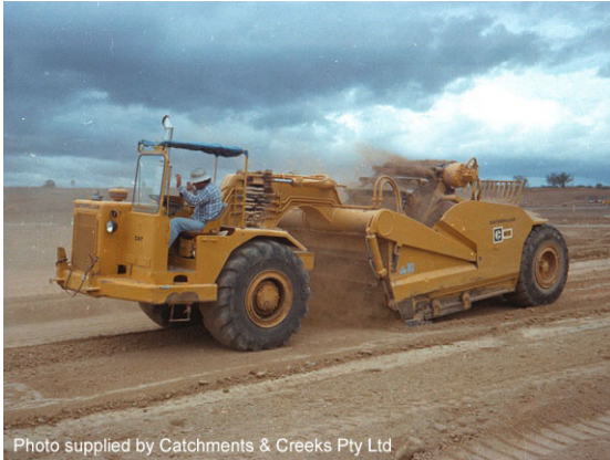
Scraper stripping soil
