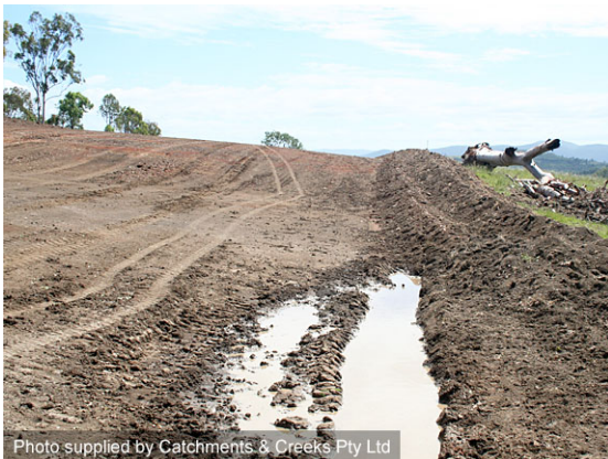
Flow diversion topsoil windrow
