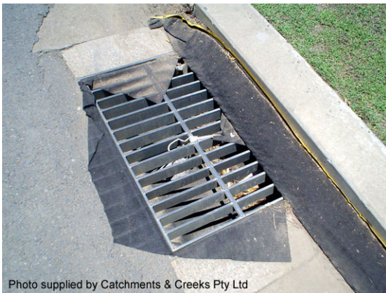
Gully bag sediment trap
