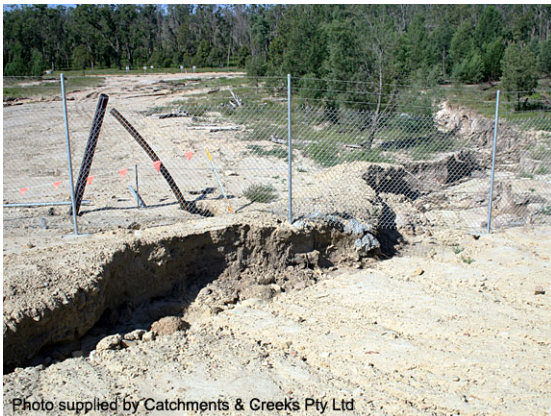
Gully erosion adjacent processing plant
