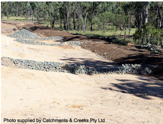
Velocity control check dams
