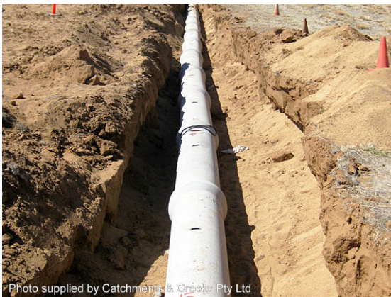
Installation of a stormwater pipeline
