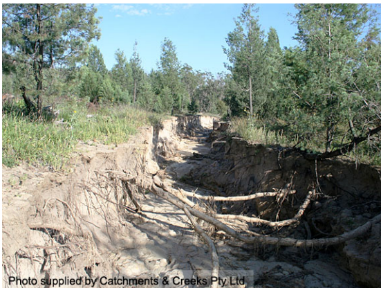
Recently formed gully erosion
