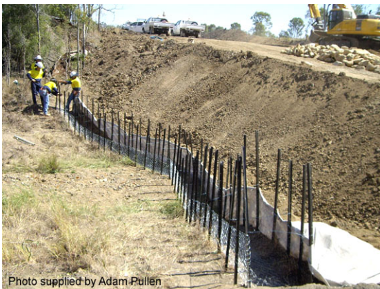
Construction of a sediment weir
