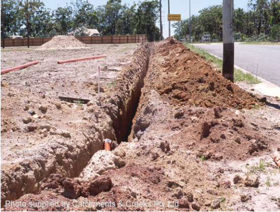
Domestic pipe installation
