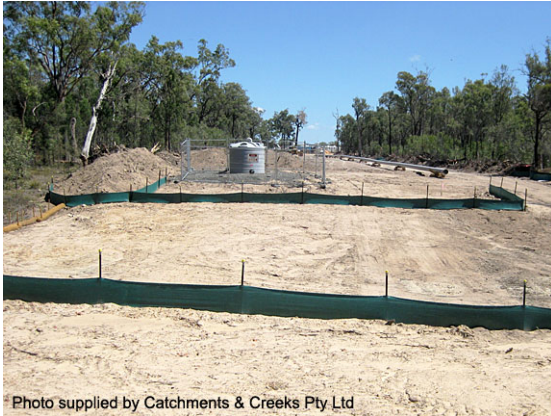
ESC measures on a pipeline RoW
