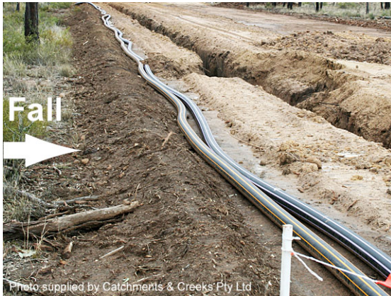
Topsoil windrow up-slope of trench
