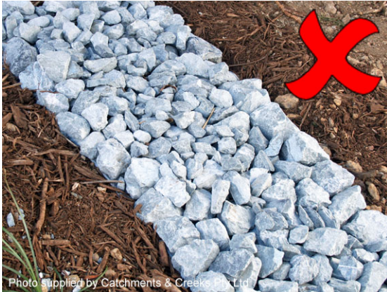
Rock-lined stormwater drain
