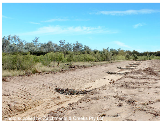
Rock check dams
