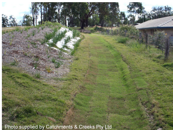
Wide, shallow, grass-lined drain
