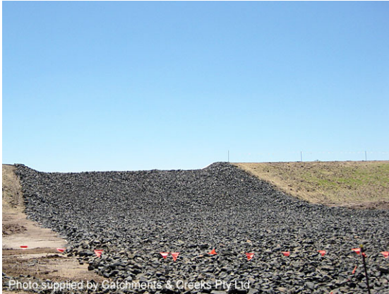
Spillway with well-defined weir profile
