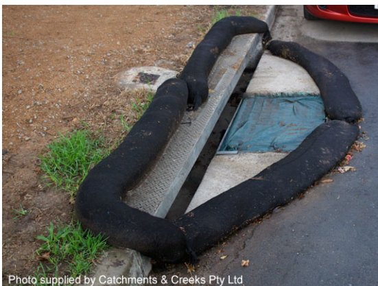
Sag-type kerb inlet protection
