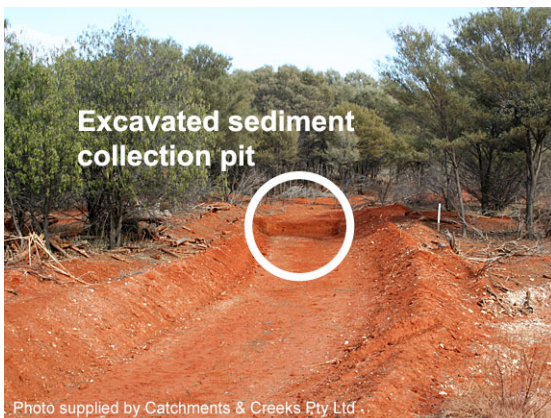
Excavated sediment sump
