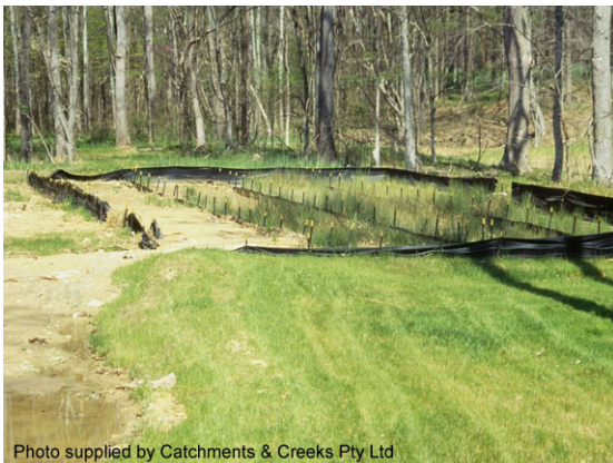
Coarse sediment trap
