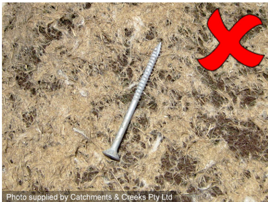
Wood screws used to anchor a blanket
