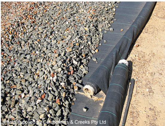
Placement of gravel over geotextile
