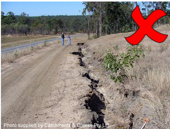
Catch drain cut into a dispersive soil
