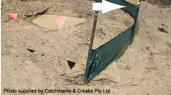
Sediment trap with no overflow weir
