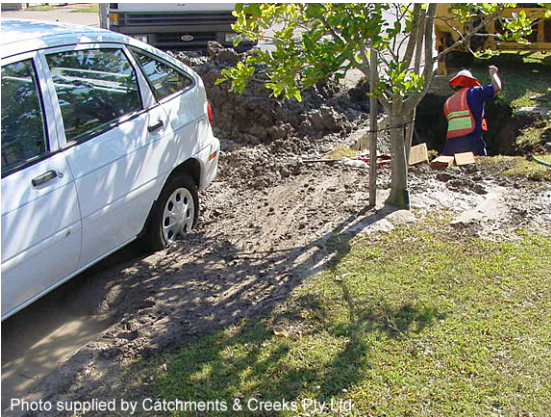
Repairing a pressure pipe failure
