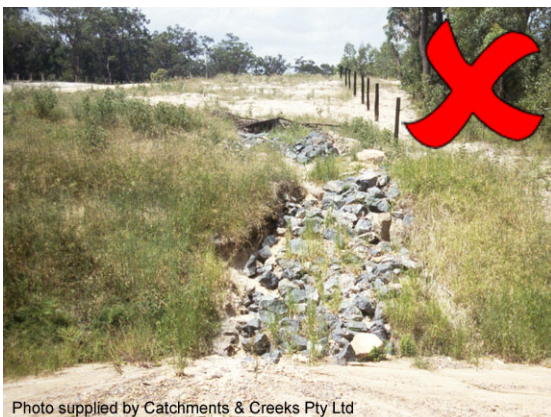
Batter chute placed on a dispersive soil
