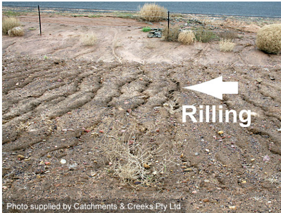
Sheet and rill erosion
