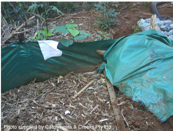
Damaged fence tagged for repair
