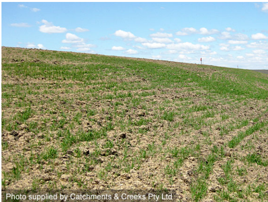
Grass establishment on embankment
