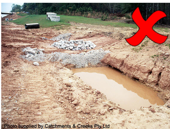
Sediment sump formed in dispersive soil
