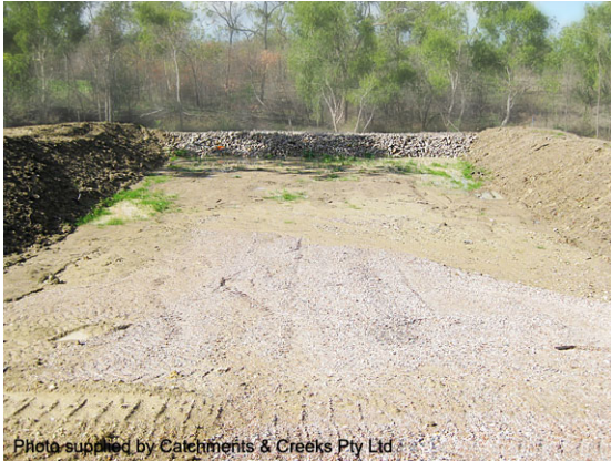
Rock filter dam
