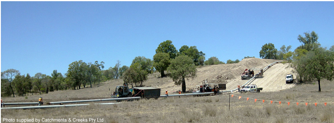
Pipe preparation prior to trenching
