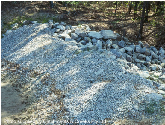
Rock filter dam - aggregate filter
