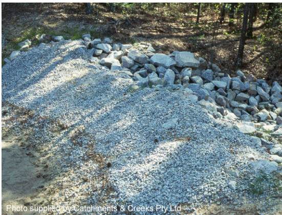
Rock filter dam with aggregate filter
