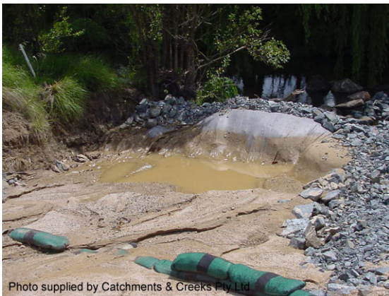
Rock filter dam - geotextile filter
