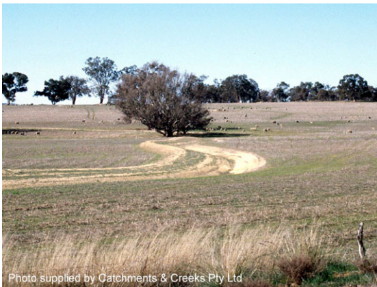
Flow diversion drain
