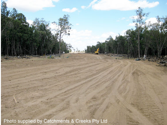
Cleared pipeline RoW
