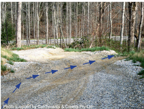
Cross bank drainage
