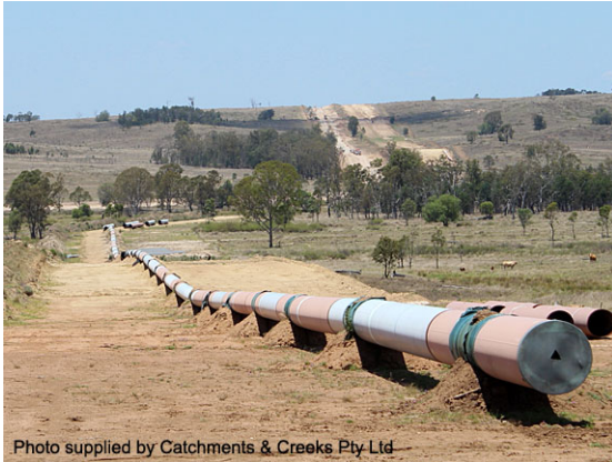
Pipeline prior to trenching
