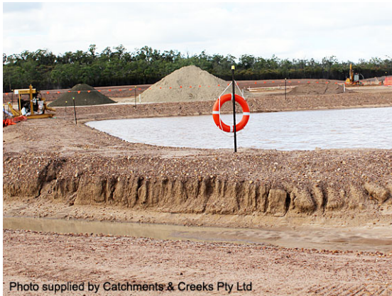
'Wet' type sediment basin
