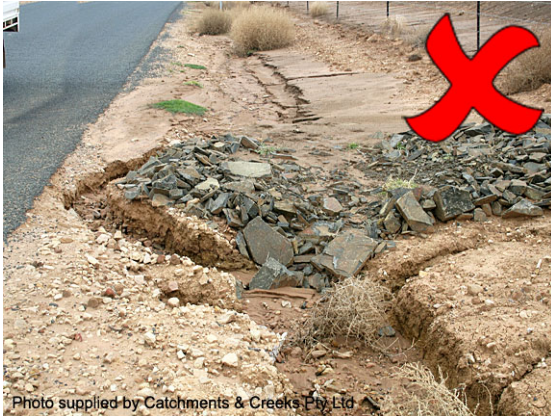
Rock check dam placed on dispersive soil
