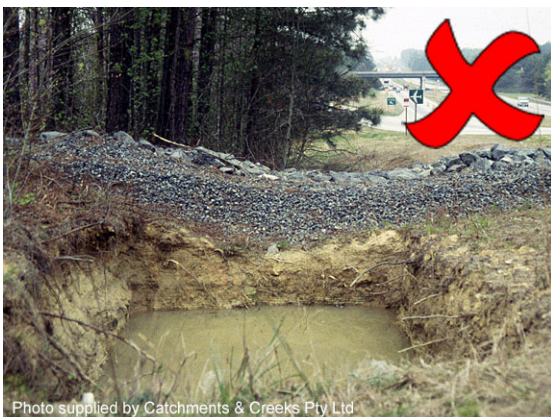
Excavated sediment trap
