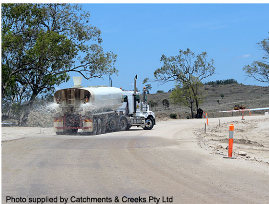
Water truck used for dust control
