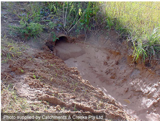
Sedimentation of drainage pipe
