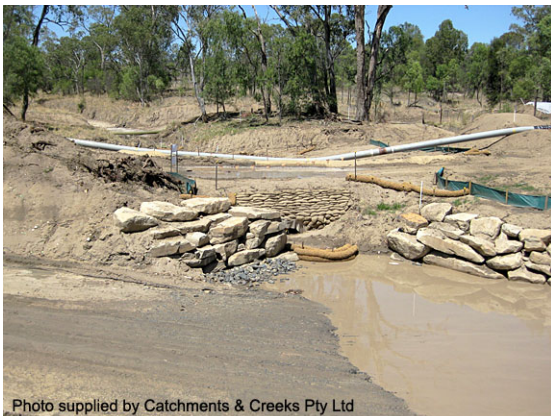
Pipeline crossing of a waterway
