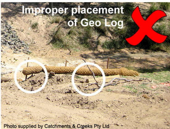
Flow allowed to pass under geo log
