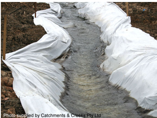
Temporary diversion drain
