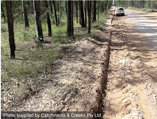
Sunken access road
