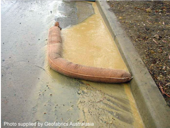
Sand-filled filter sock
