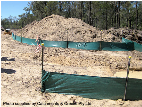
Sediment trap on pipeline RoW
