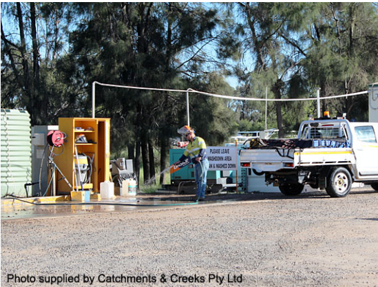
Vehicle wash-down area
