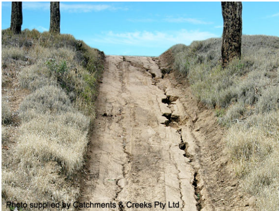
Rilling on a maintenance access track
