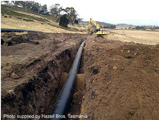
Installation of an irrigation pipeline
