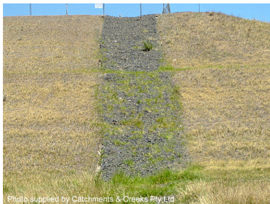
Rock-lined batter chute
