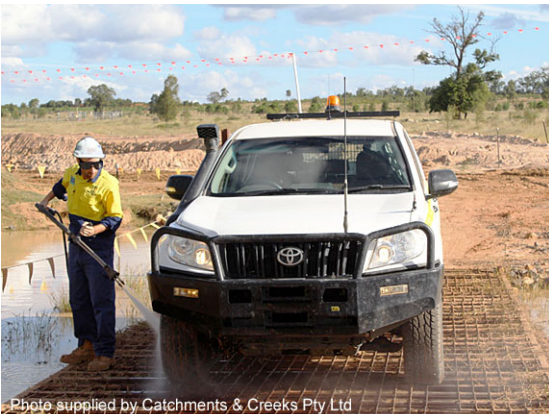
Vehicle wash-down area
