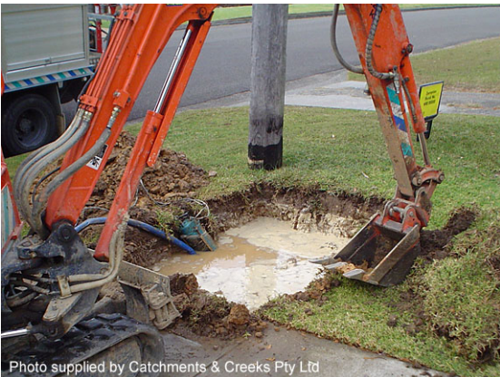
Pipe trench de-watering
