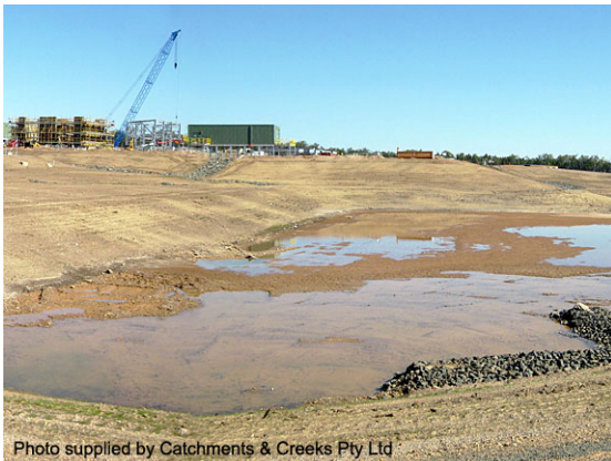
Sediment basin at a gas processing plant
