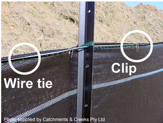
Sediment fence with top wire
