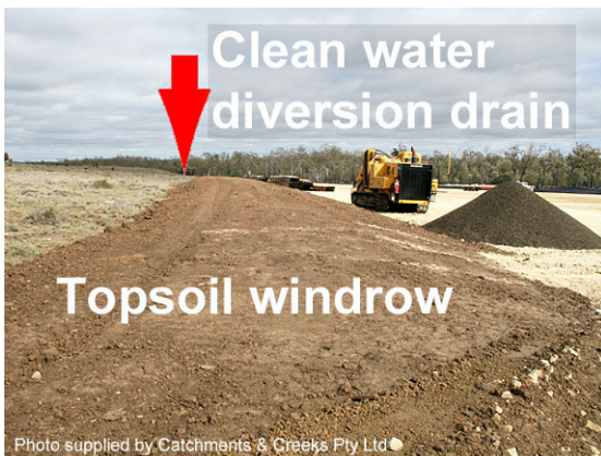
Topsoil windrow flow diversion bank
