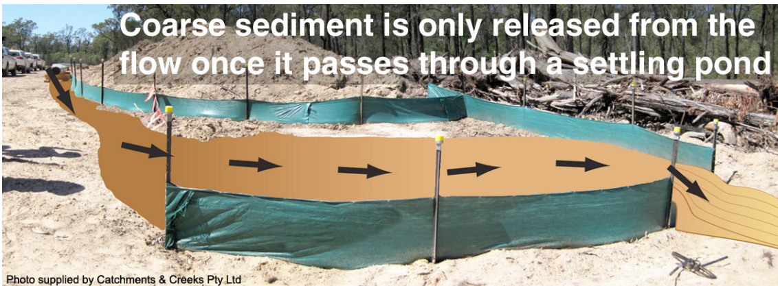
Sediment-laden water passes through the settling pond allowing sedimentation
