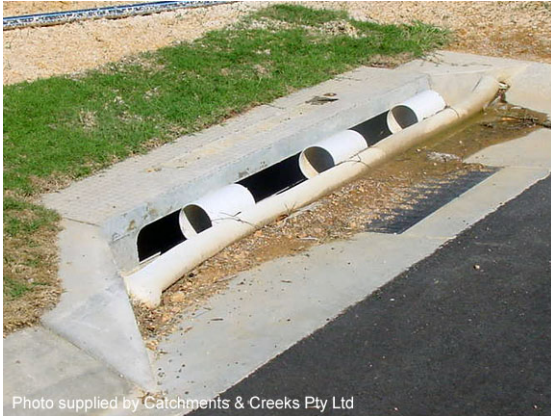
Sag inlet sediment trap
