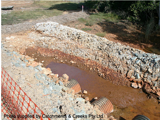
Rock filter dam with aggregate filter
