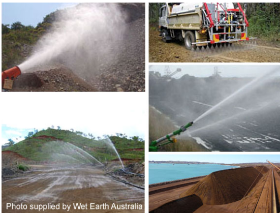
Application of soil binders
