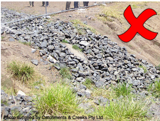
Rocks slipping down batter chute
