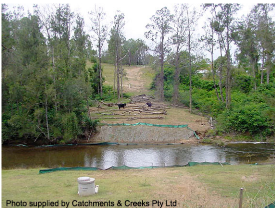
Rehabilitation of pipeline RoW
