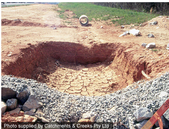
Excavated sediment sump
