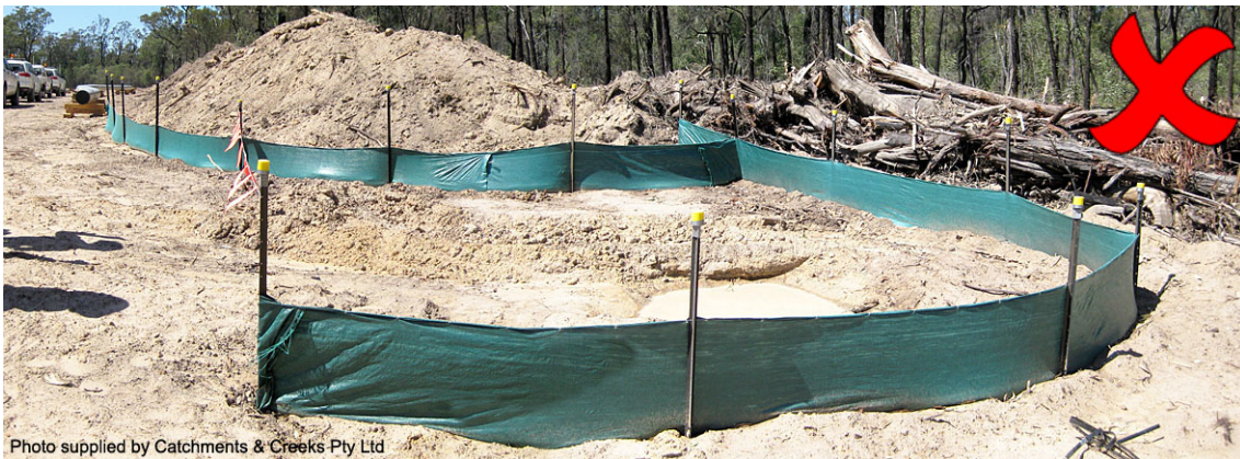
Inappropriate sediment trap set-up
