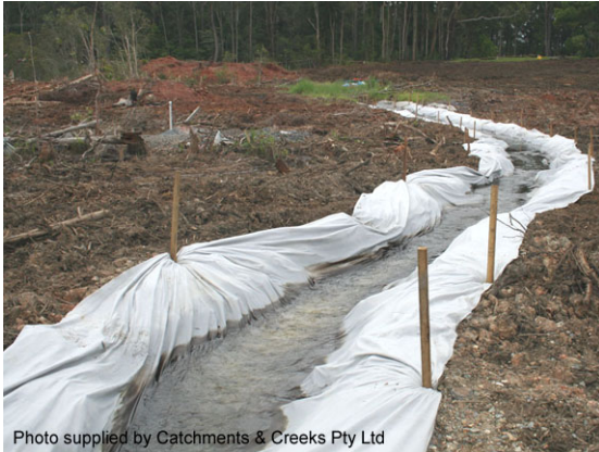
Clean water diversion drain
