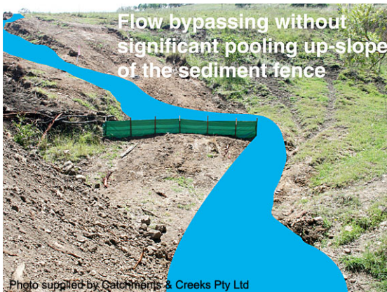
Sediment fence fails to capture sediment
