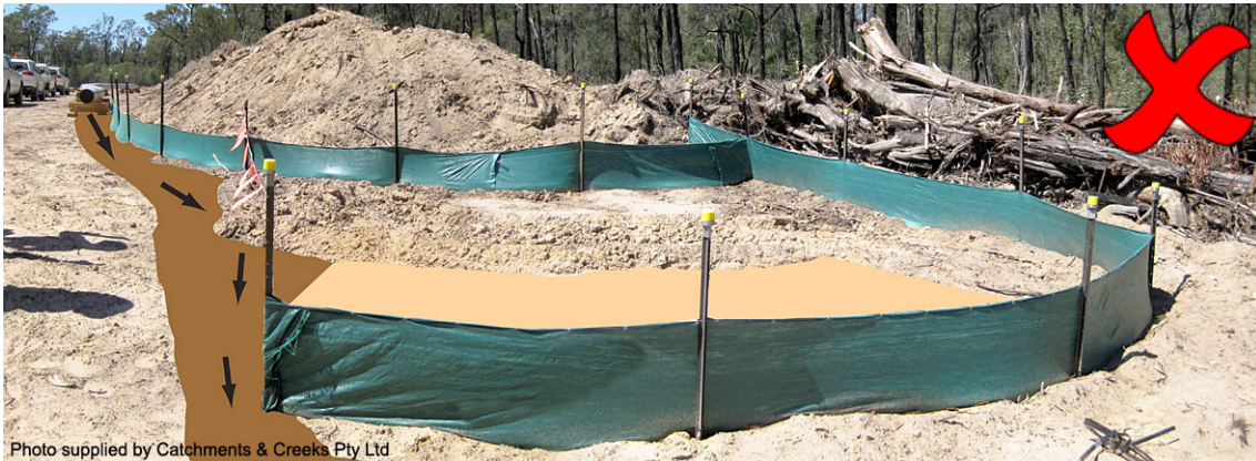
Once full, the sediment trap allows sediment-laden flow to bypass the trap
