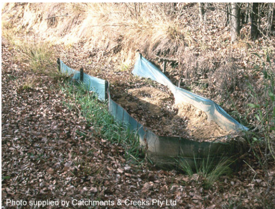
U-shaped sediment trap in steep drain
