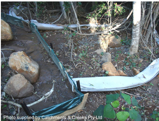
Filter tube dam sediment trap
