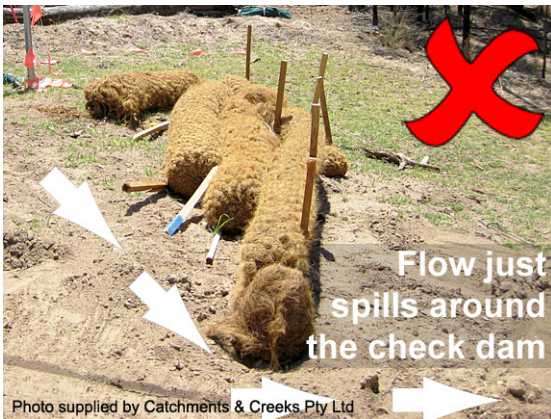
Flow allowed to pass around geo logs
