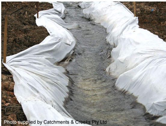
Filter cloth anchored with timber stakes
