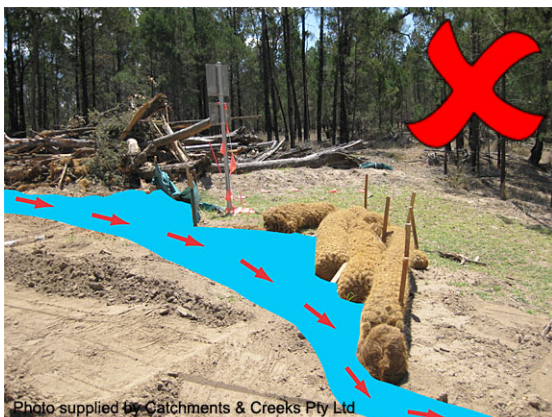
Stormwater runoff bypasses sediment trap
