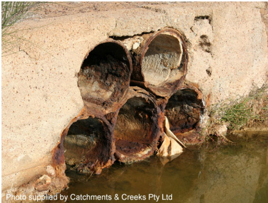
Culvert damaged by acidic water
