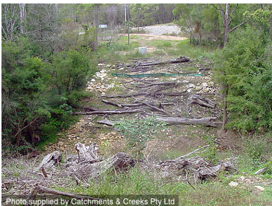
Placement of tree debris over RoW
