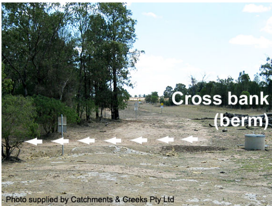
Cross drainage within pipeline RoW
