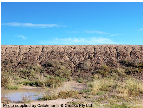
Rilling that extends to top of bank
