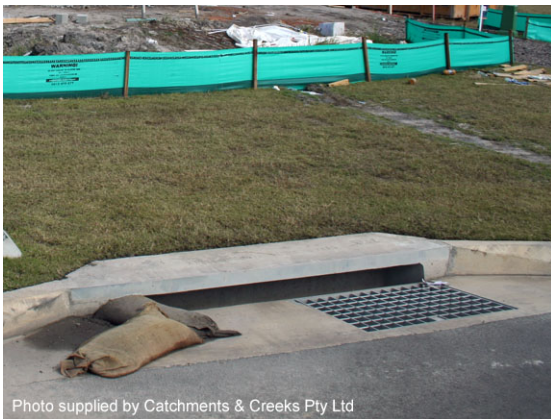
On-grade kerb inlet sediment trap
