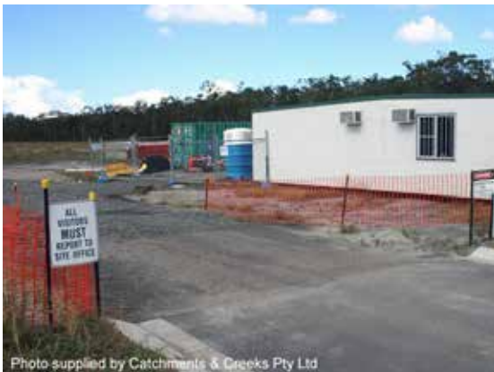
Site entry and office
