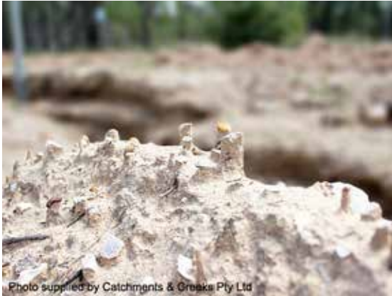
Evidence of raindrop impact erosion
