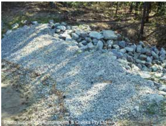
Rock filter dam with aggregate filter
