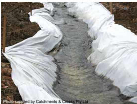
Filter cloth anchored with timber stakes
