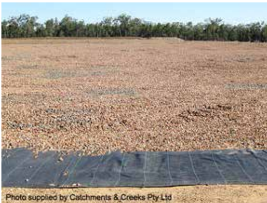
Gravelling of processing plant site
