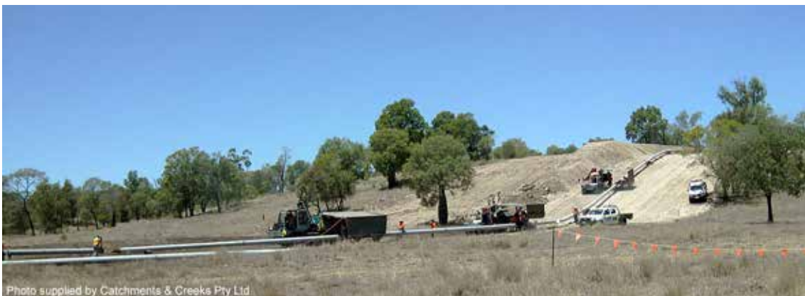
Pipe preparation prior to trenching
