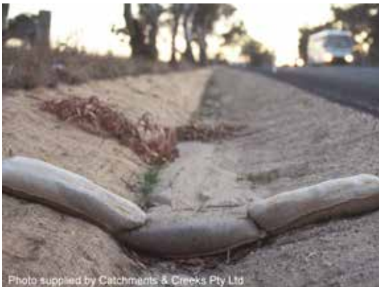
Sandbag check dam
