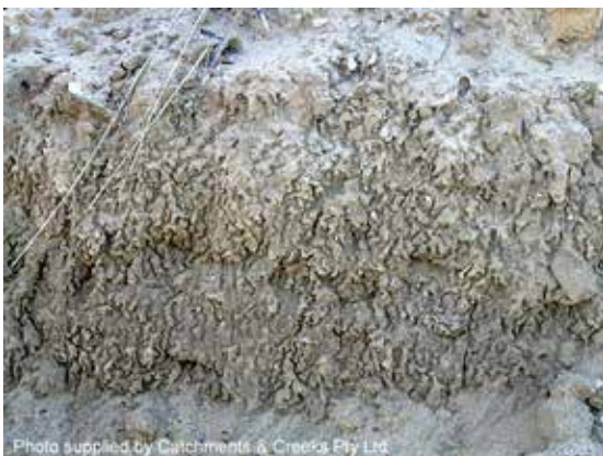
Bank not exposed to direct rainfall
