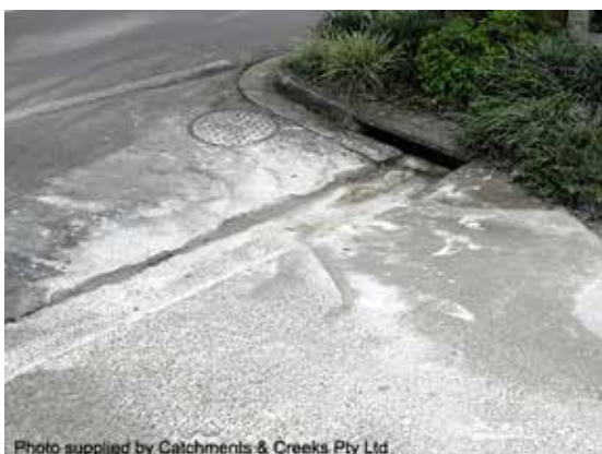
Deposition of cement wash-off on a road
