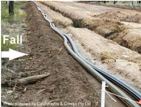
Topsoil windrow up-slope of trench
