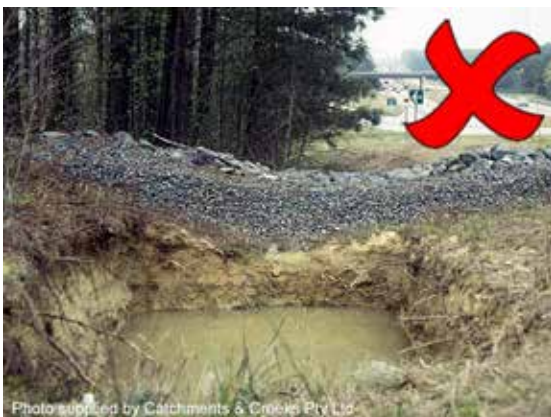
Excavated sediment trap
