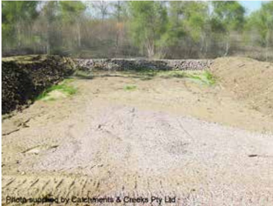
Rock filter dam
