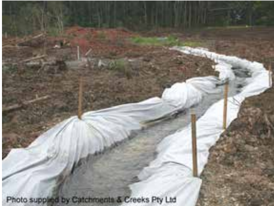
Clean water diversion drain
