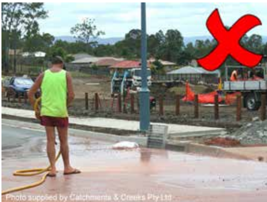
Poor maintenance practice
