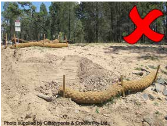
Geo log placed on steep slope
