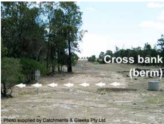
Cross drainage within pipeline RoW
