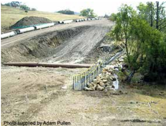
Sediment controls at waterway crossing
