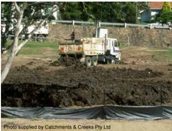
Soil being worked when it is too wet
