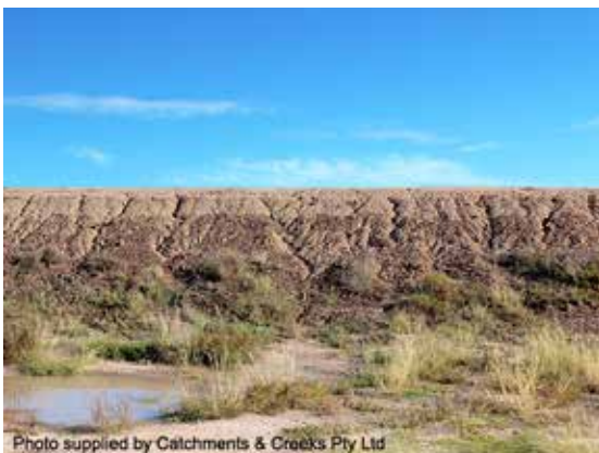
Rilling that extends to top of bank
