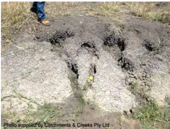
Deep rilling and tunnel erosion
