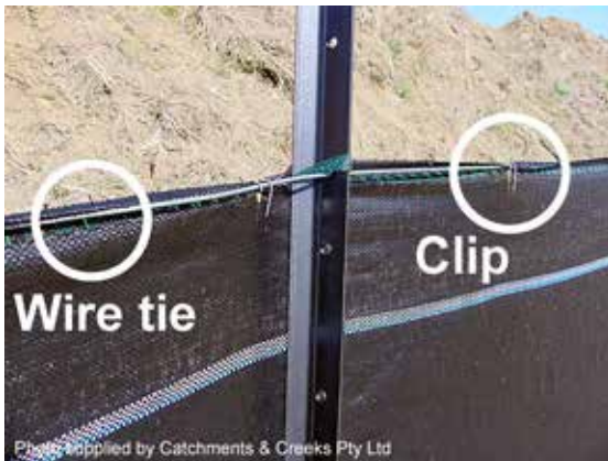
Sediment fence with top wire
