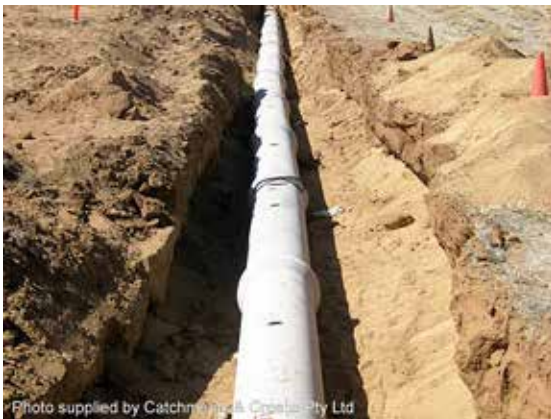
Installation of a stormwater pipeline
