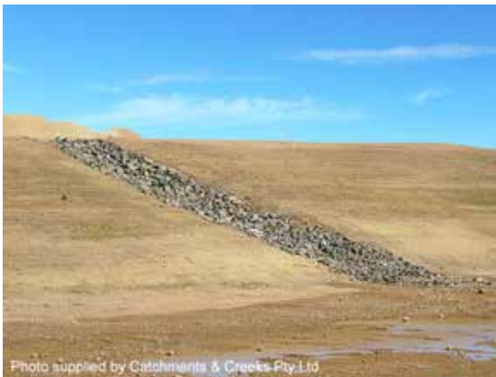
Rock-lined batter chute
