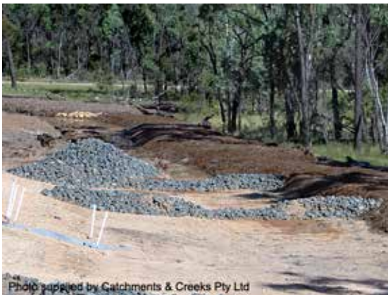
Velocity control check dams
