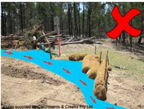
Stormwater runoff bypasses sediment trap
