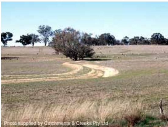
Flow diversion drain
