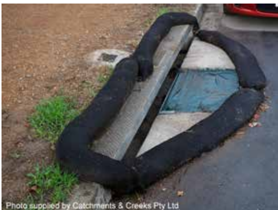
Sag-type kerb inlet protection
