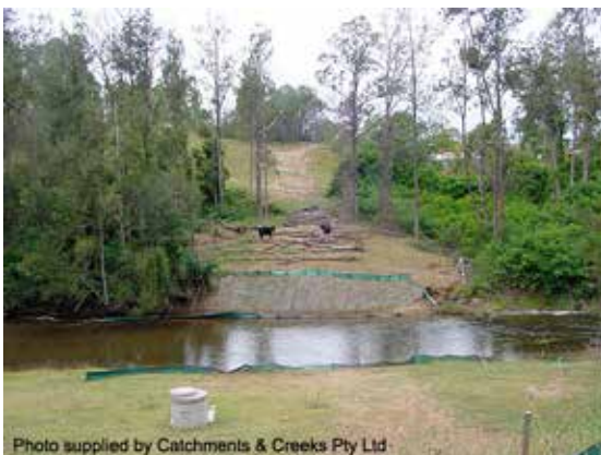
Rehabilitation of pipeline RoW
