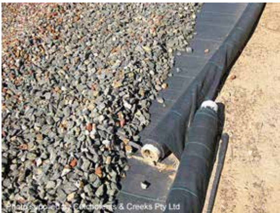
Placement of gravel over geotextile
