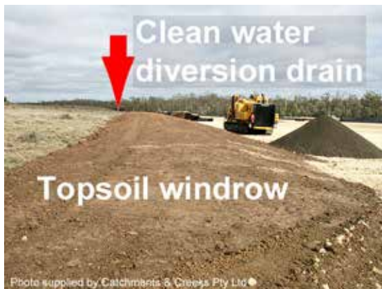
Topsoil windrow flow diversion bank
