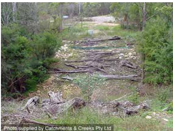
Placement of tree debris over RoW
