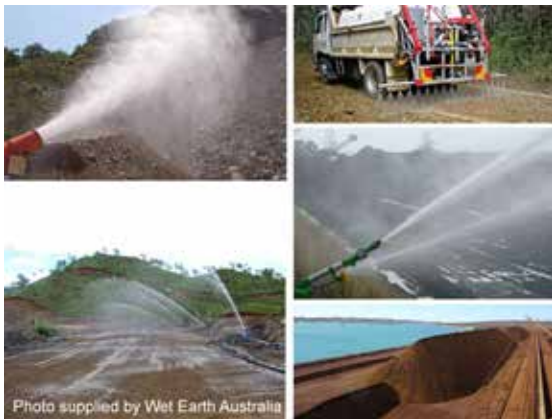
Application of soil binders
