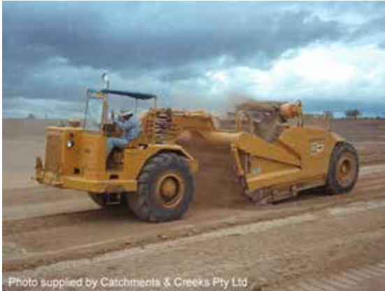
Scraper stripping soil
