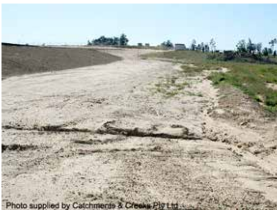
Rill erosion across an access track
