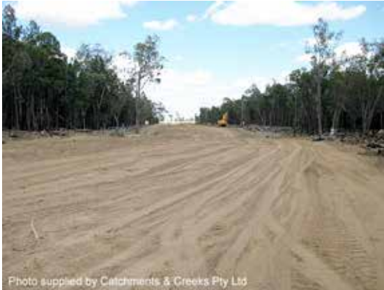
Cleared pipeline RoW
