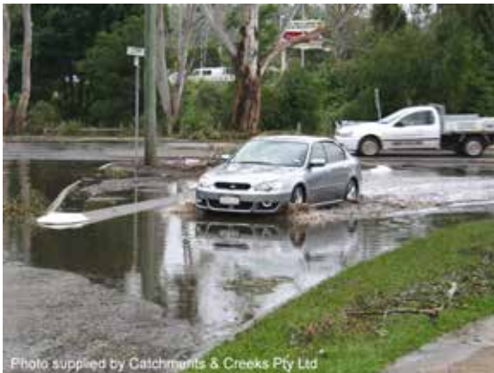
Flooded road surface
