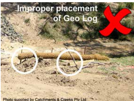
Flow allowed to pass under geo log
