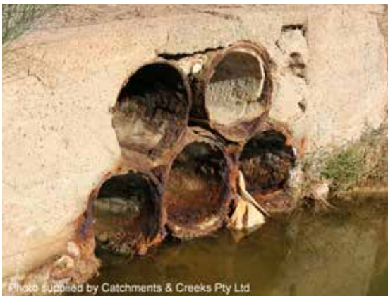
Culvert damaged by acidic water
