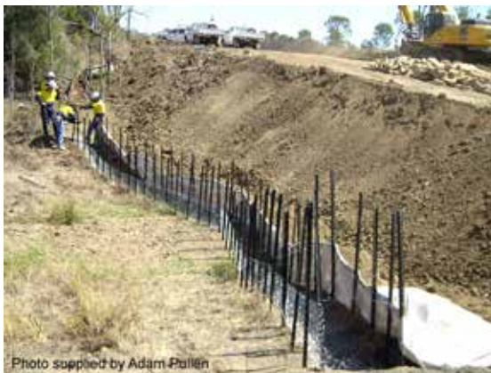
Construction of a sediment weir
