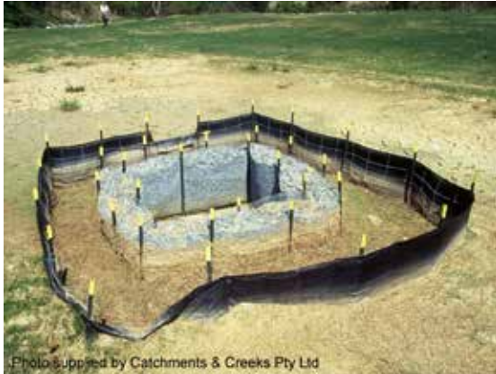
Sediment weir (field inlet protection)
