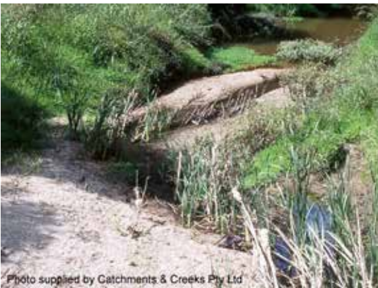
Deposition of coarse sediment in a creek
