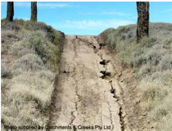
Rilling on a maintenance access track
