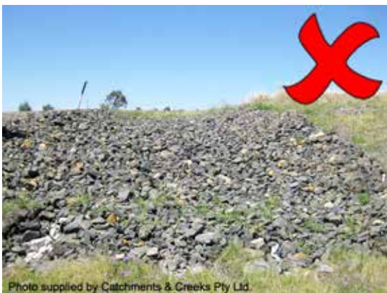
Inadequate rock size
