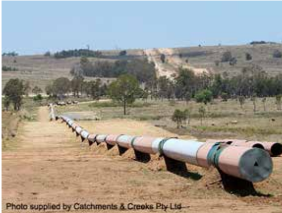
Assembled pipeline prior to trenching
