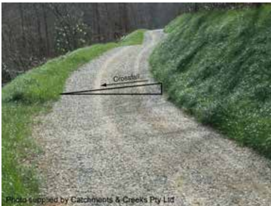
Gravel road with out-fall drainage
