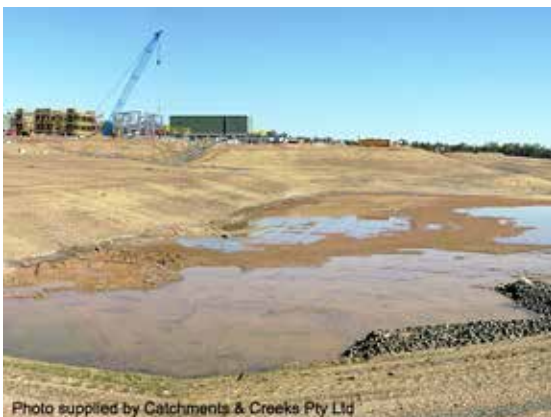
Sediment basin at a gas processing plant
