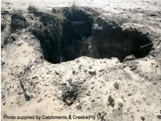
Entrance to tunnel erosion
