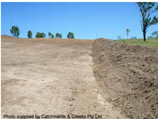
Topsoil windrow down-slope of RoW
