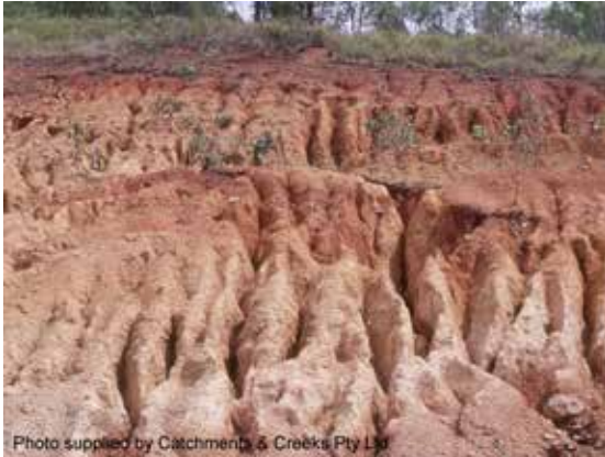
Erosion of a dispersive soil
