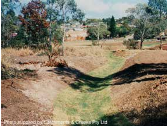
Turf lined diversion drain
