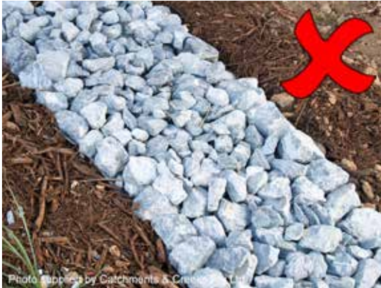
Rock-lined stormwater drain
