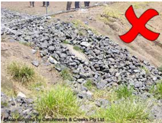
Rocks slipping down batter chute
