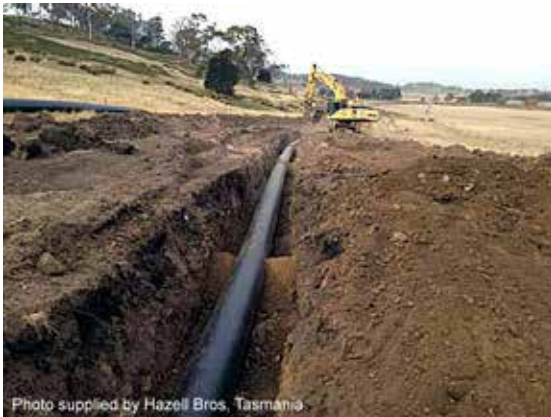
Installation of an irrigation pipeline
