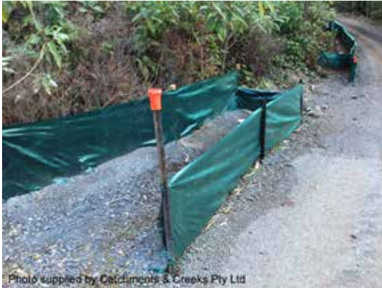
U-shaped sediment trap
