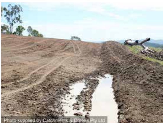
Flow diversion topsoil windrow
