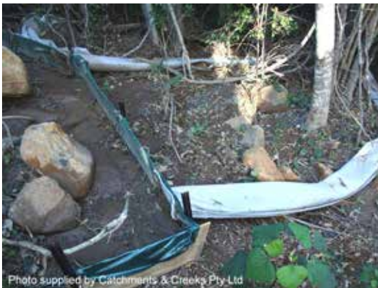
Filter tube dam sediment trap
