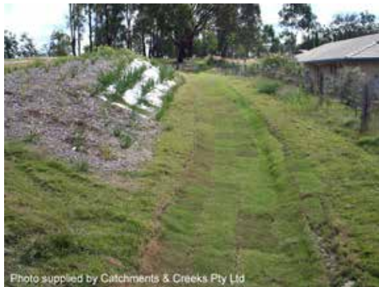
Wide, shallow, grass-lined drain
