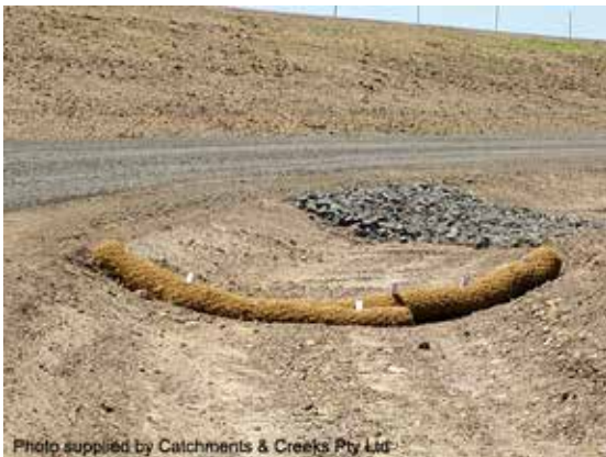
Geo-log check dam
