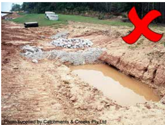
Sediment sump formed in dispersive soil
