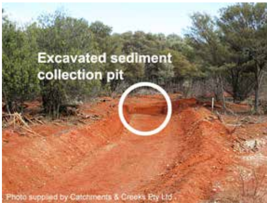
Excavated sediment sump
