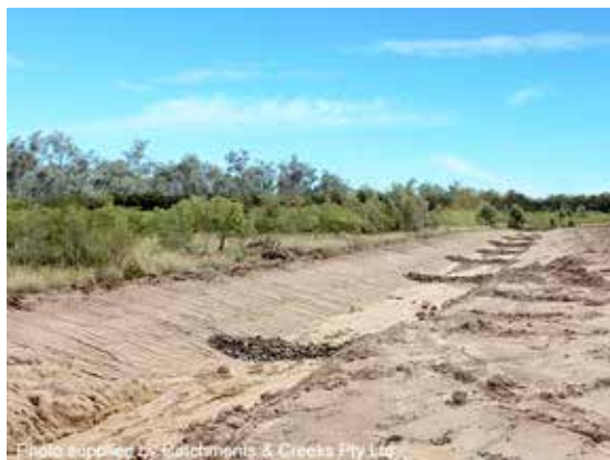
Rock check dams
