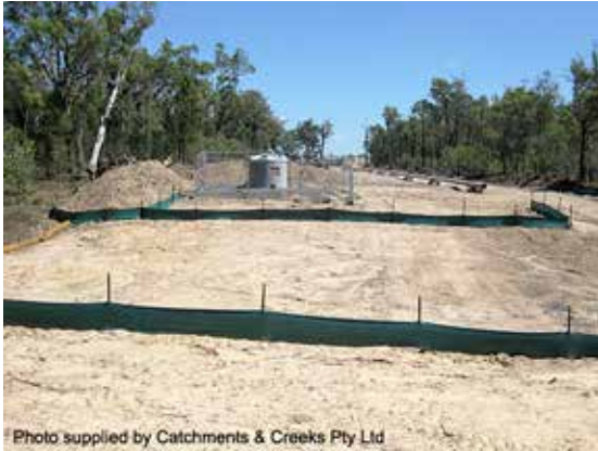
ESC measures on a pipeline RoW
