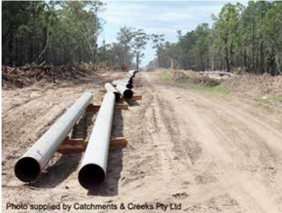
Pipeline installation project
