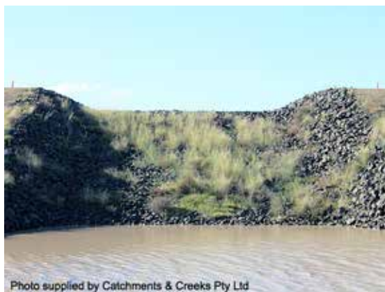
Energy dissipation pond
