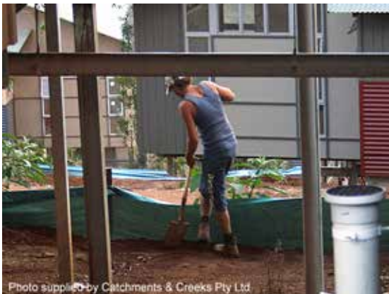
Maintenance of control measures
