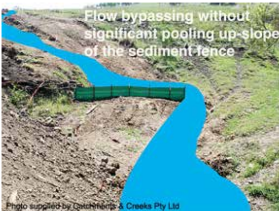
Sediment fence fails to capture sediment
