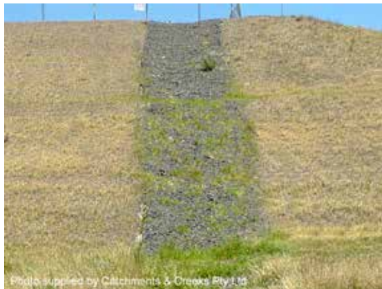
Rock-lined batter chute
