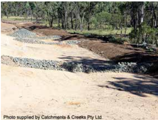
Velocity control check dams
