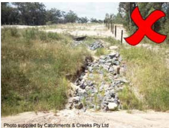
Batter chute placed on a dispersive soil
