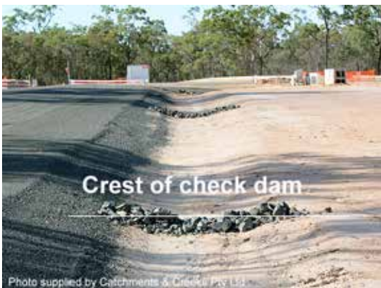
Rock check dam
