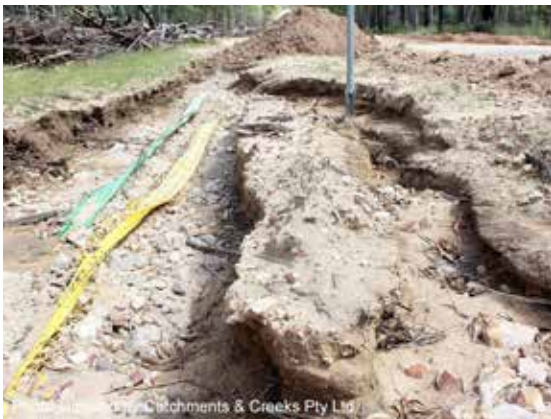
Erosion along a backfilled pipe trench
