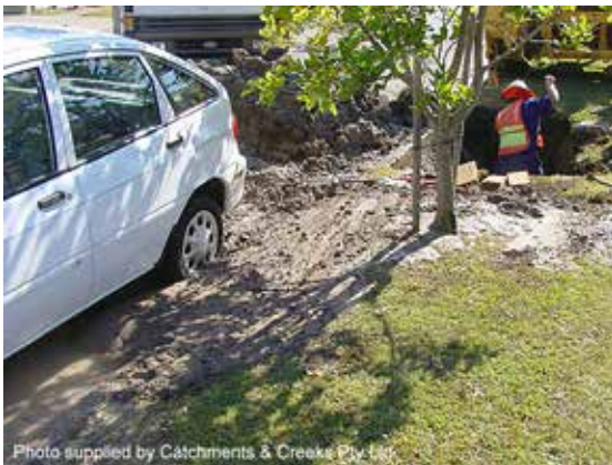
Repairing a pressure pipe failure
