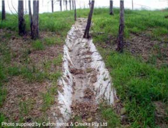
Geotextile lined drainage chute
