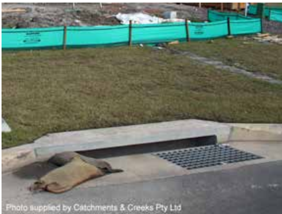
On-grade kerb inlet sediment trap
