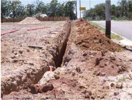
Domestic pipe installation
