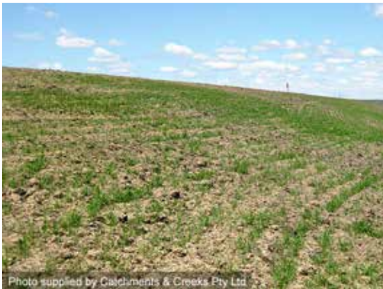
Grass establishment on embankment
