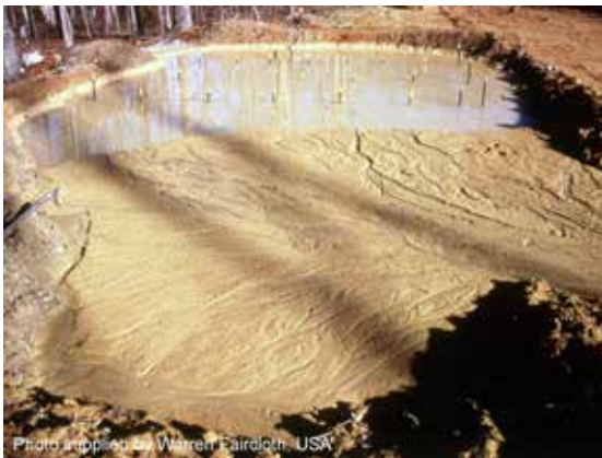
Sediment retained in a sediment trap
