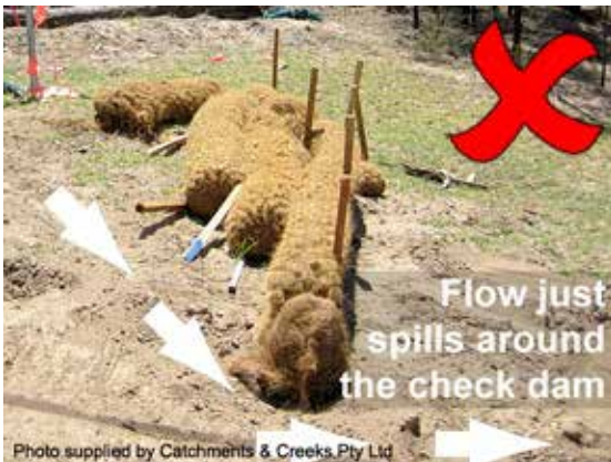
Flow allowed to pass around geo logs
