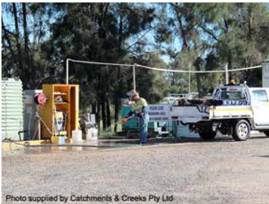
Vehicle wash-down area
