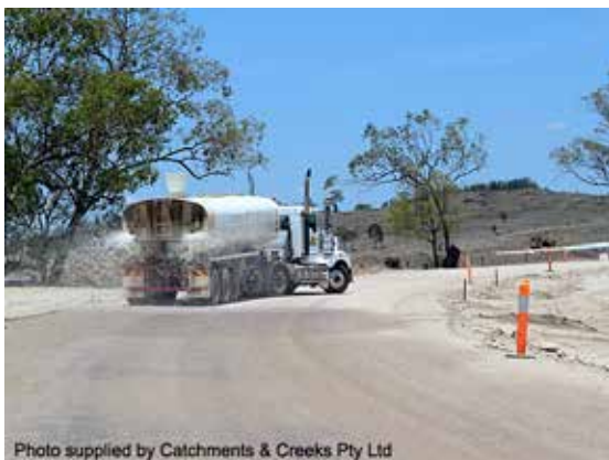
Water truck used for dust control
