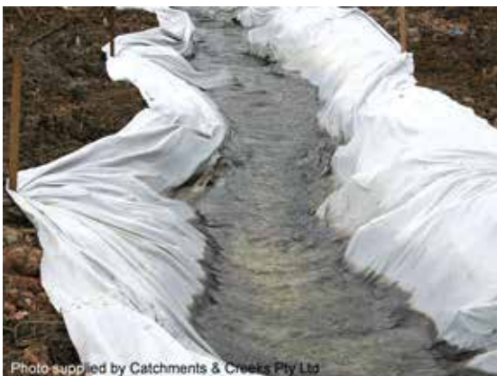
Temporary diversion drain
