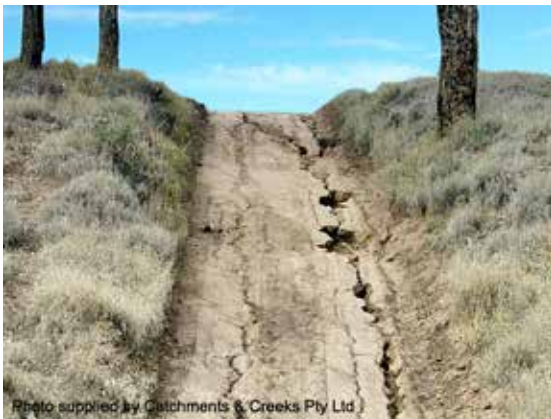
Steep, dispersive soil access track
