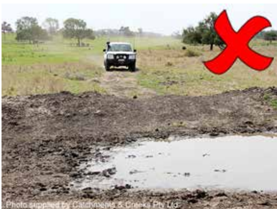
Water pooling at a cross bank
