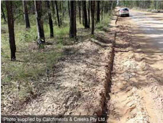
Sunken access road
