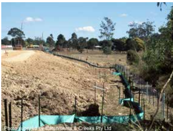
Placement of regular ‘returns’
