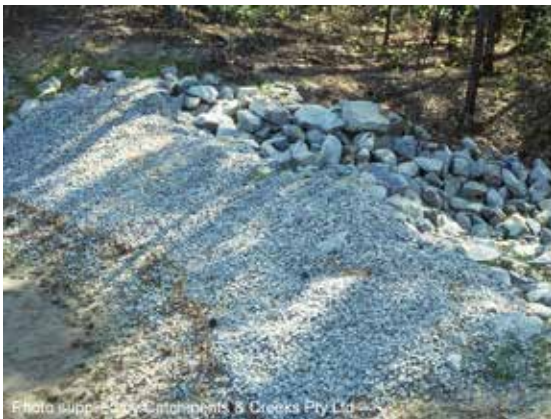
Rock filter dam - aggregate filter
