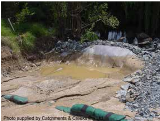
Rock filter dam - geotextile filter
