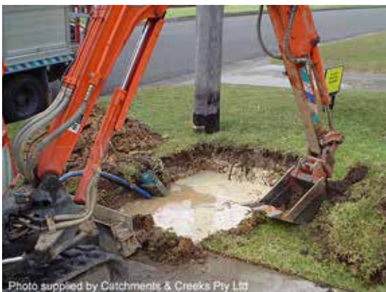
Pipe trench de-watering
