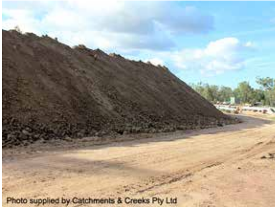
Topsoil stockpile
