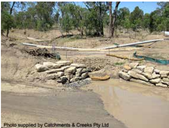
Pipeline crossing of a waterway
