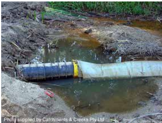
Filter tube attached to an embankment
