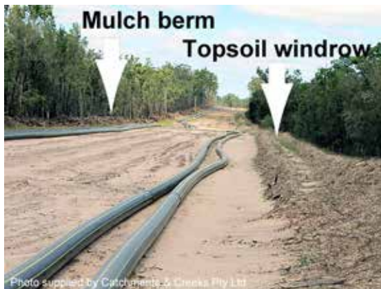
Pipeline prior to trenching
