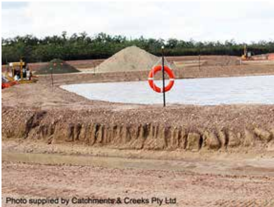
'Wet' type sediment basin
