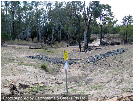
Rock stabilised vehicle crossing
