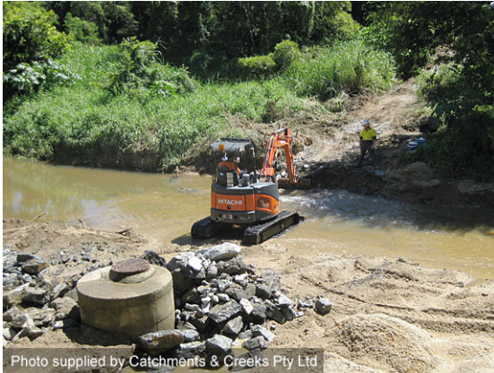
Instream construction works
