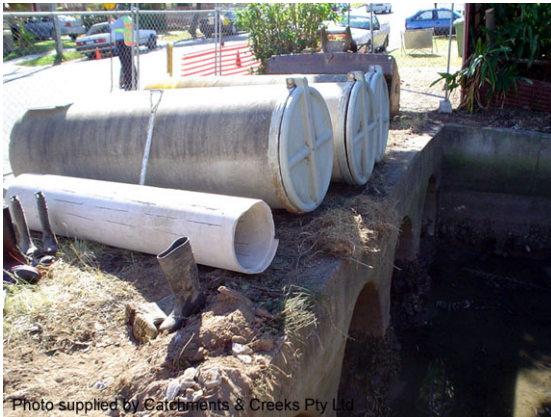
Floodgates prior to their installation
