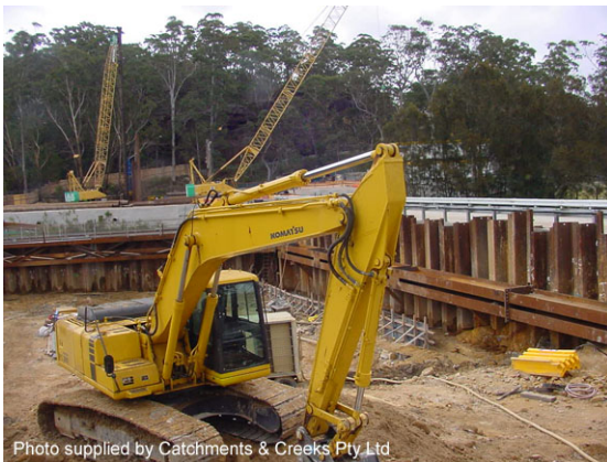
Use of sheet piling isolation barrier
