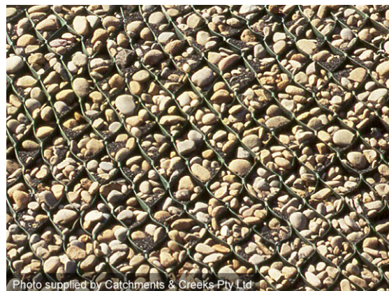
Cellular confinement system stabilisation
