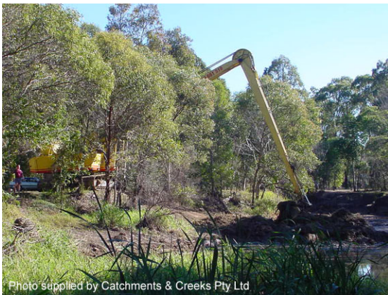
Use of a long-reach excavator
