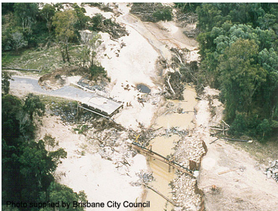
Flood damage to bridge & buried pipes
