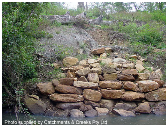
Non-vegetated rock stabilisation
