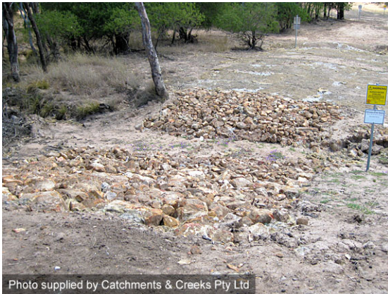
Rock stabilisation above pipeline
