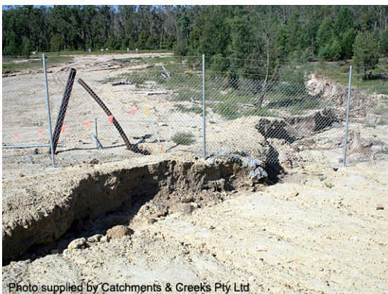
Gully erosion in slaking soil
