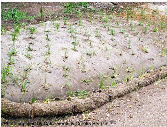
Coir 'geo-log' temporary toe protection
