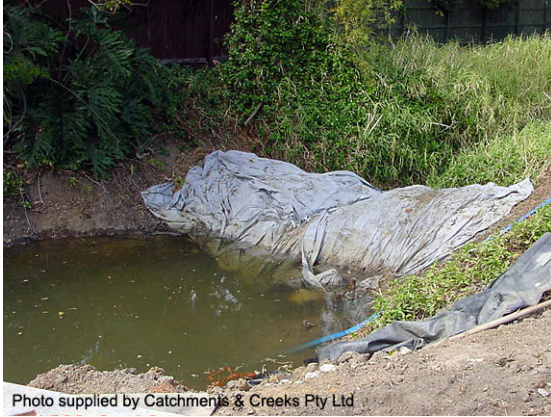
Instream rock filter dam
