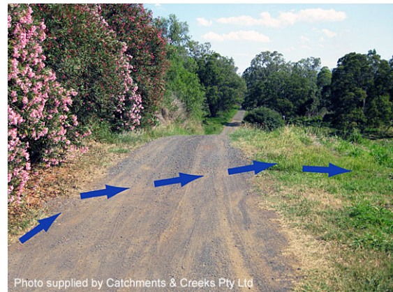
Cross bank placed at top of descent
