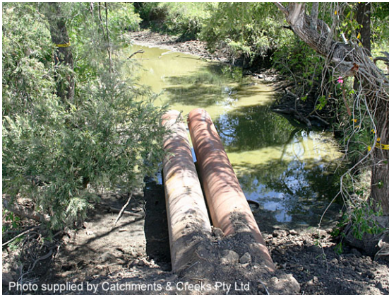
Gravity bypass pipe (flume) system
