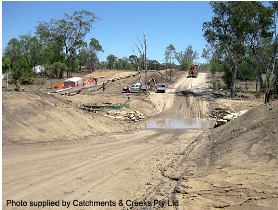
Vehicle access across a waterway
