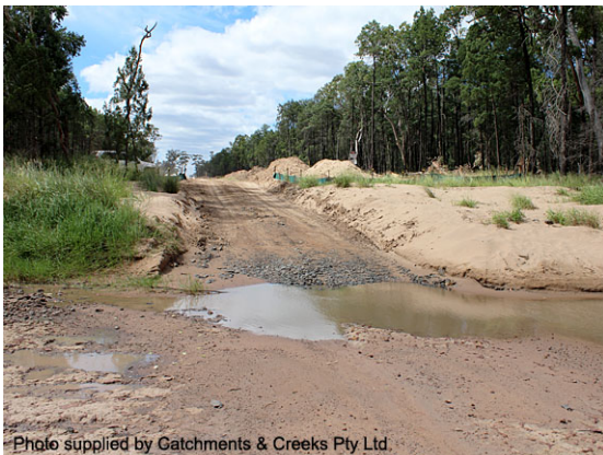
Crossing of a sand-based watercourse
