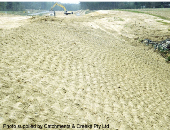
Roughened earth batter
