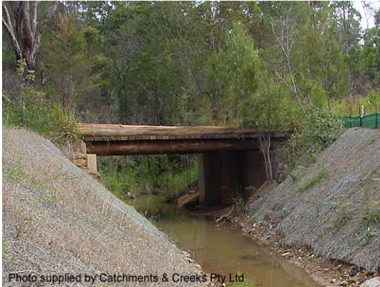
Permanent maintenance access bridge
