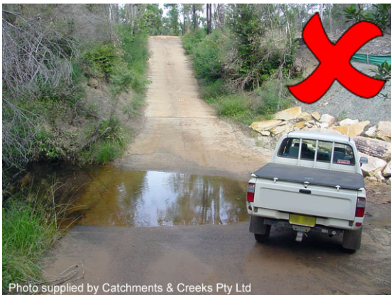
Concrete sealed 'ford' crossing
