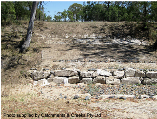
Rock stabilised pipe crossing
