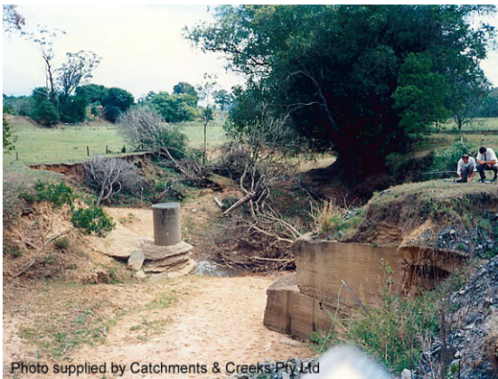
Pipeline exposed by migrating waterway
