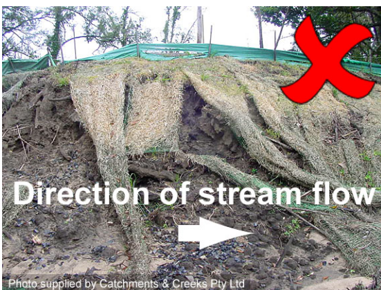
Failed erosion control mat
