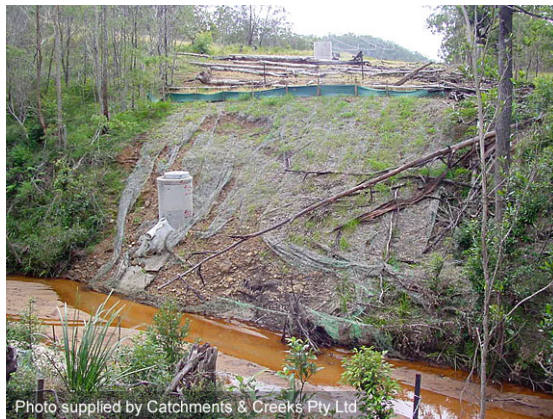
Non-vegetated rock stabilisation
