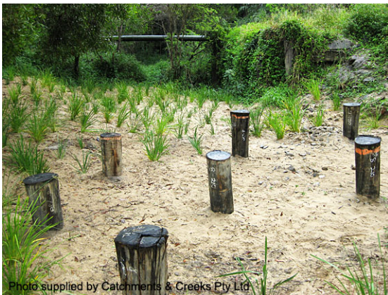
Pile filed in sand-based waterway
