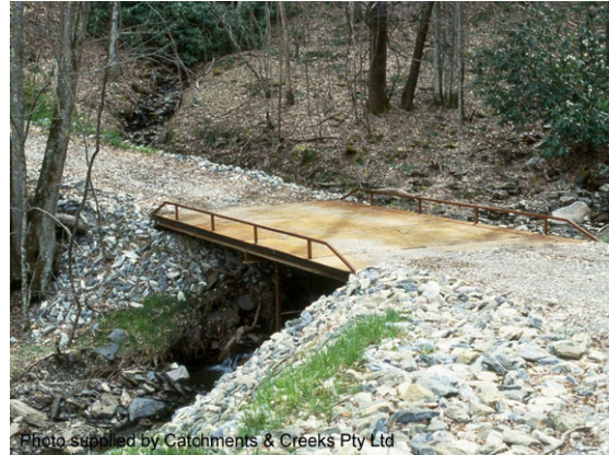
Permanent maintenance access bridge
