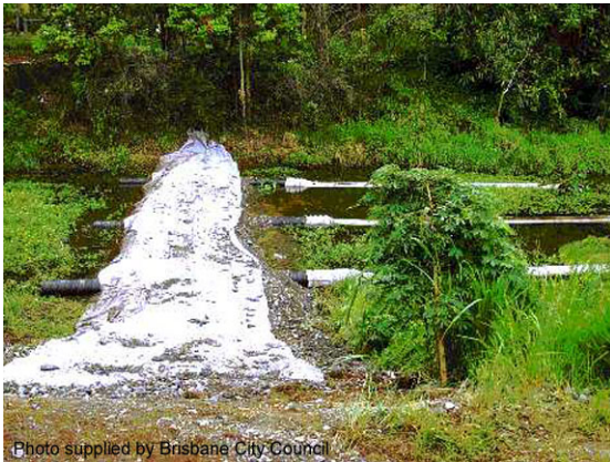
Rock filter dam with filter tubes
