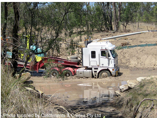
Ford crossing of an alluvial waterway
