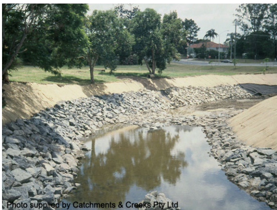
Rock stabilisation on channel bend
