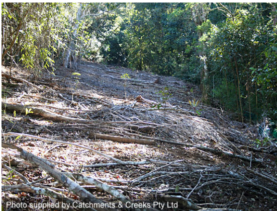
Placement of woody debris
