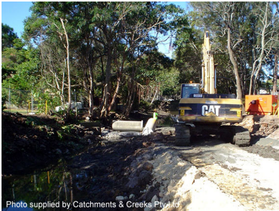
Construction of a cofferdam
