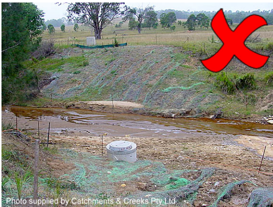
Use of synthetic reinforced mats
