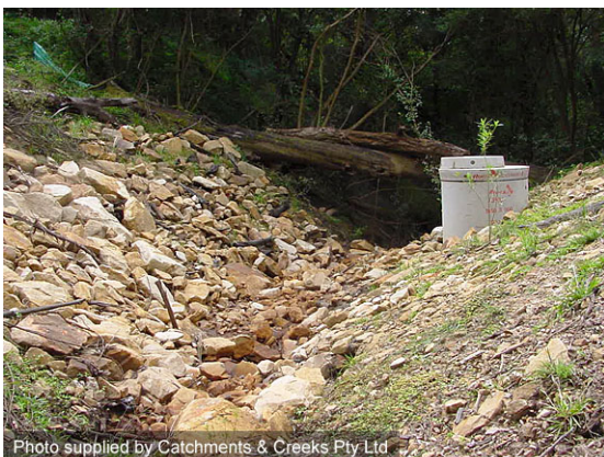
Rock-lining adjacent access pit
