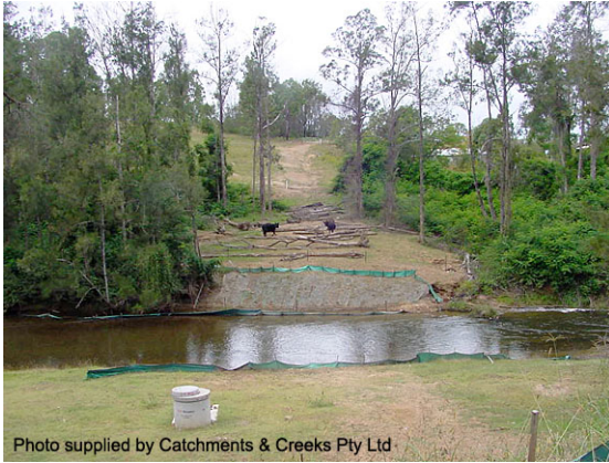
Rehabilitated pipeline crossing
