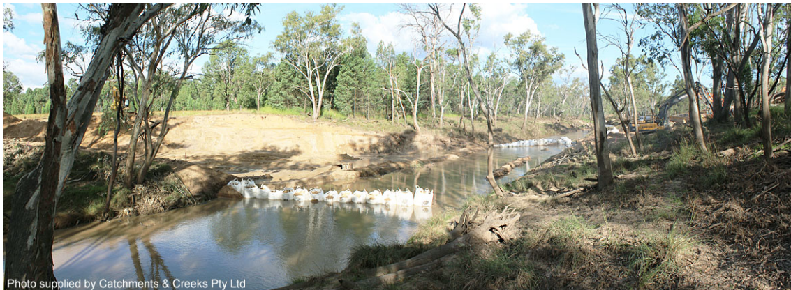
Construction of pipeline crossing of a waterway with riparian 'values'
