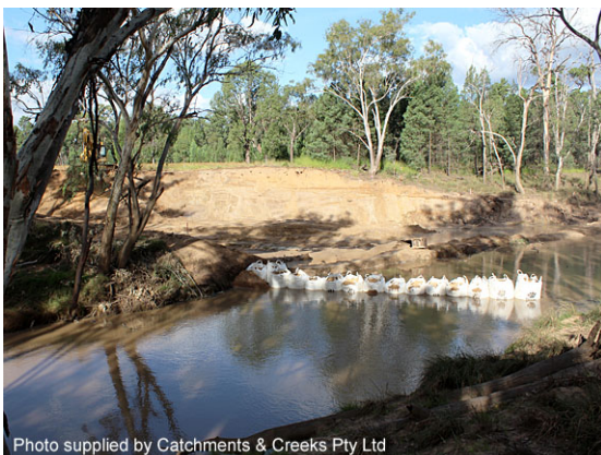
Construction of a pipeline crossing
