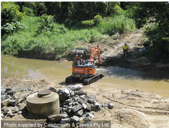
Works within a sandy waterway
