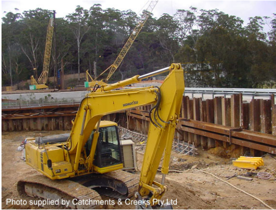
Sheet piling isolation barrier
