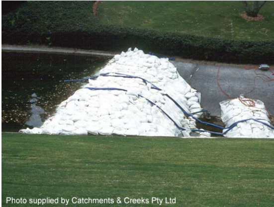
Sandbag cofferdam in concrete drain
