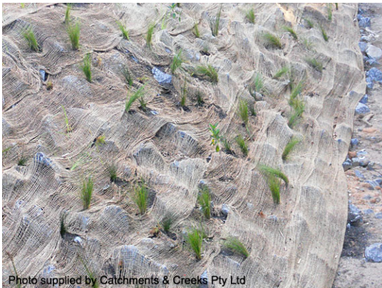
Planted rock covered with jute mesh
