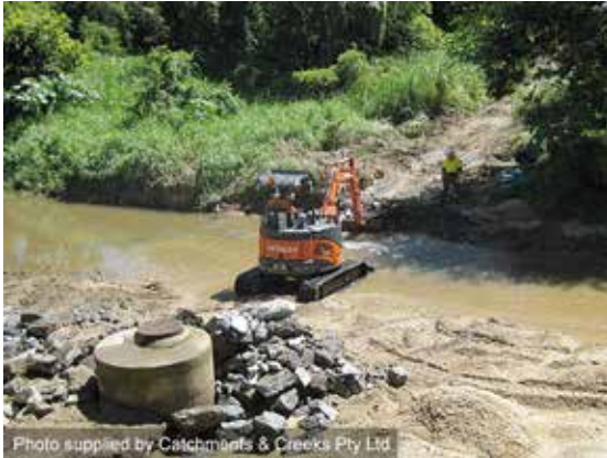
Instream construction works
