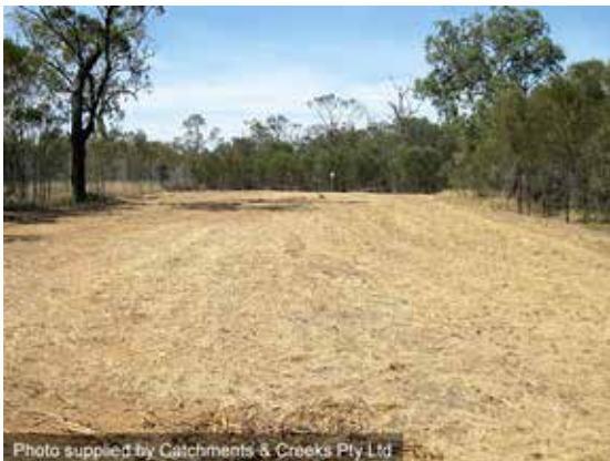
Establishment of grass cover over RoW
