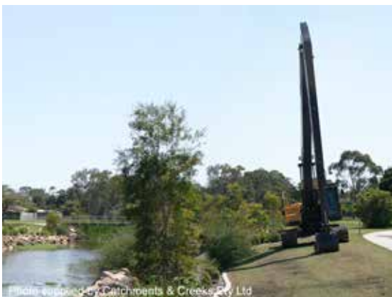
Long reach excavator
