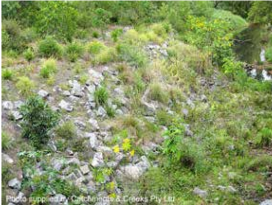
Planted rock-stabilised creek bank
