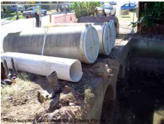
Floodgates prior to their installation
