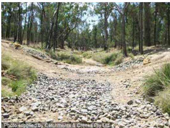
Rock stabilised vehicle crossing
