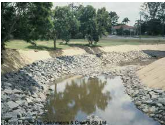
Rock stabilisation on channel bend
