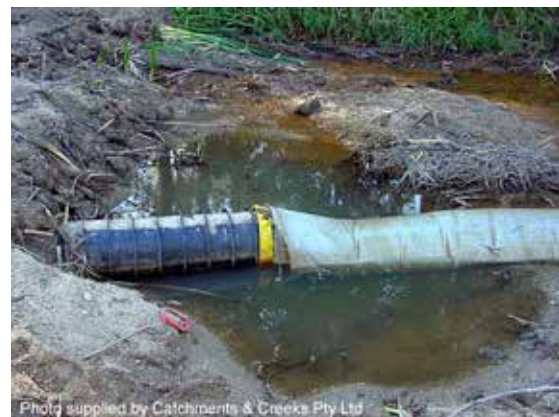
Filter tube connected to ribbed pipe
