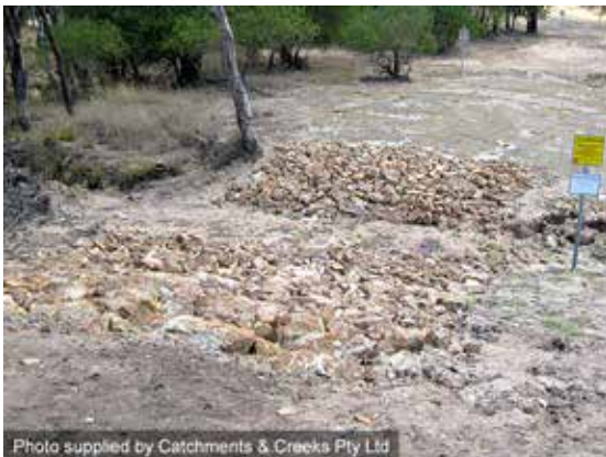
Rock stabilisation above pipeline
