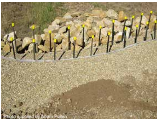
Sediment control weir
