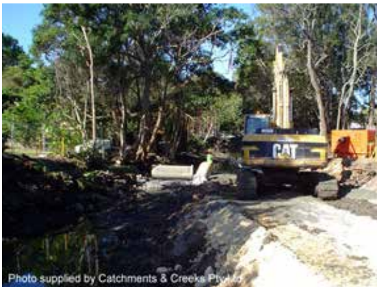
Construction of a cofferdam
