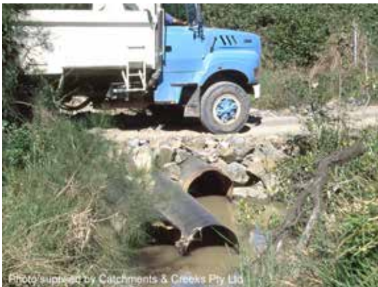
Temporary culvert crossing
