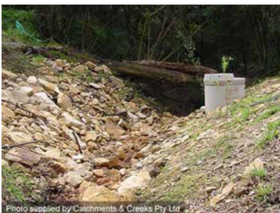
Rock-lining adjacent access pit
