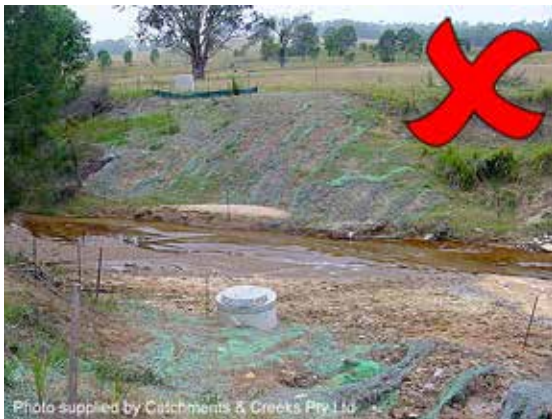
Use of synthetic reinforced mats
