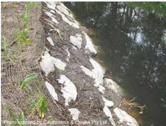
Voids filled with soil ready for planting
