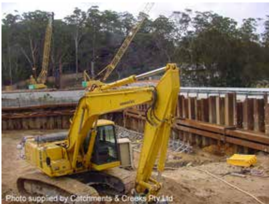
Use of sheet piling isolation barrier
