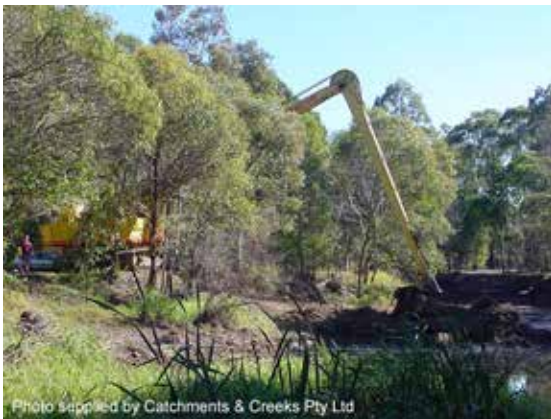
Use of a long-reach excavator
