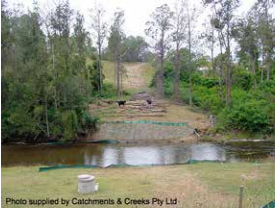
Rehabilitated pipeline crossing
