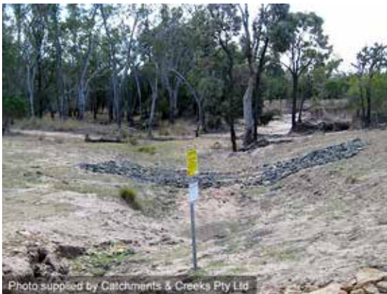
Rock stabilised vehicle crossing
