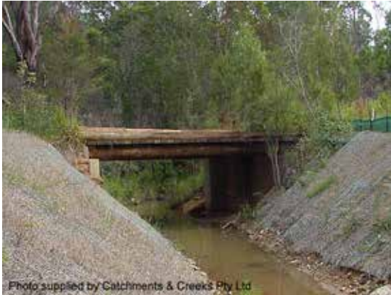
Permanent maintenance access bridge
