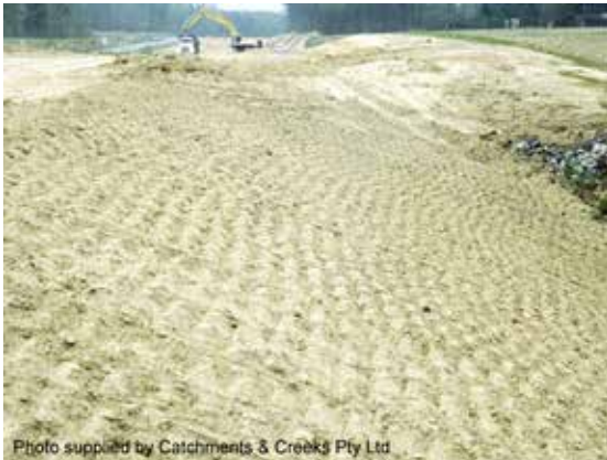
Roughened earth batter
