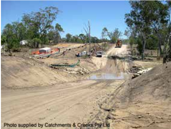
Vehicle access across a waterway
