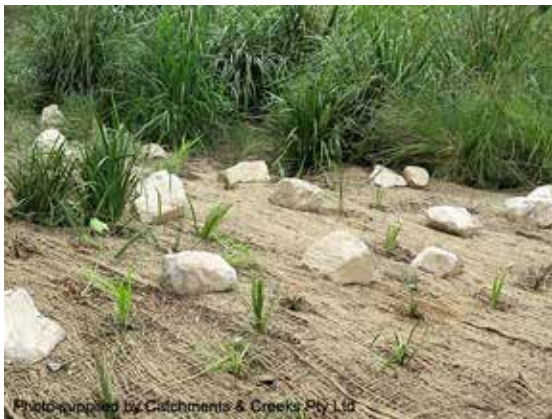
Erosion control jute mesh
