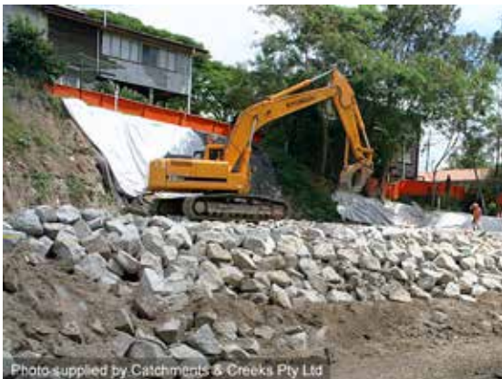
Rock placement over filter cloth
