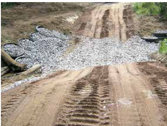
Ecoflex 'E-pave' stabilisation system
