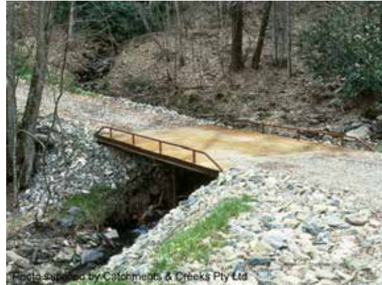
Permanent maintenance access bridge
