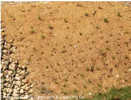
Bonded fibre matrix
