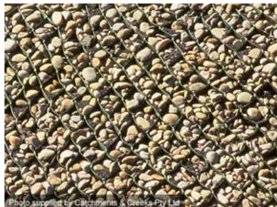
Cellular confinement system stabilisation
