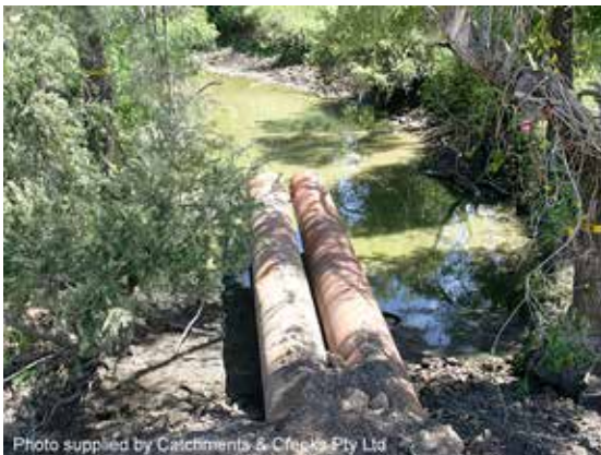
Gravity bypass pipe (flume) system
