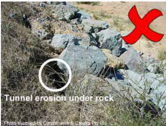
Tunnel erosion under rocks
