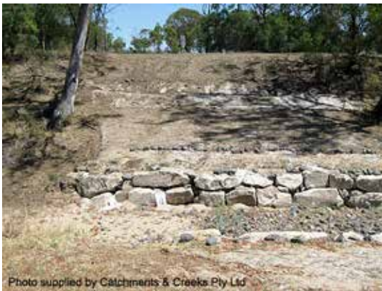
Rock stabilised pipe crossing
