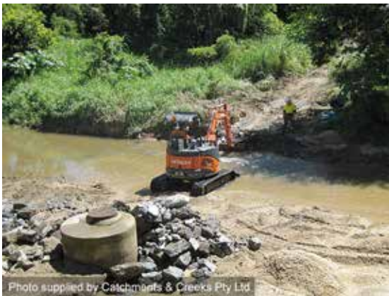
Works within a sandy waterway
