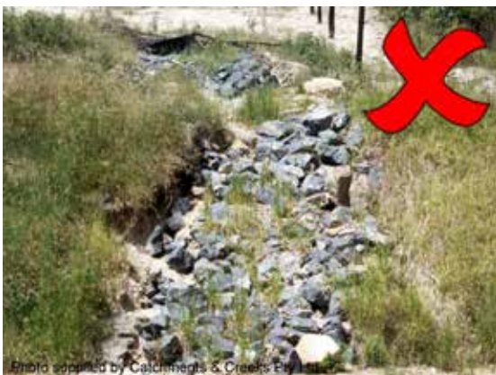
Rock placed on a dispersive soil bank
