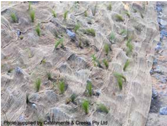
Planted rock covered with jute mesh
