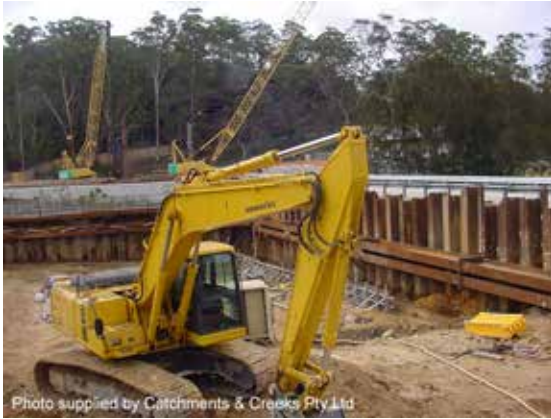
Sheet piling isolation barrier
