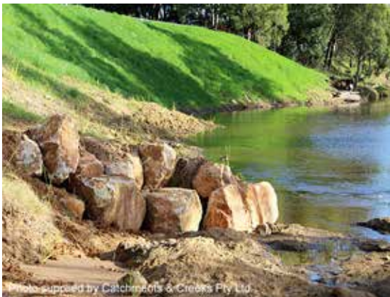
Rock flow control groyne
