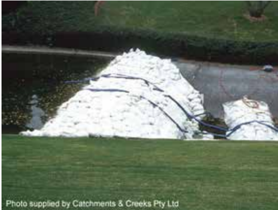
Sandbag cofferdam in concrete drain
