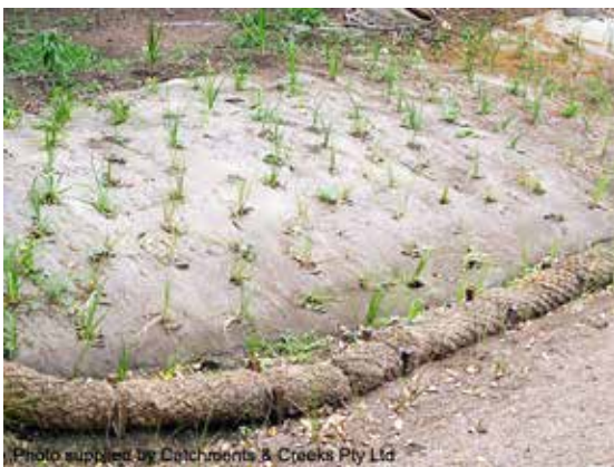
Coir 'geo-log' temporary toe protection
