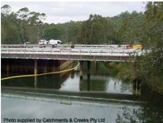
Navigation maintained around works
