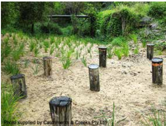
Pile field in sand-based waterway
