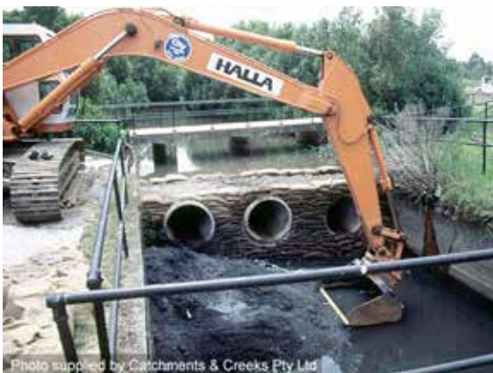
Works within a tidal waterway
