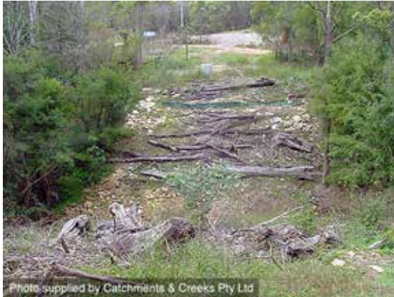
Bank stabilisation measures
