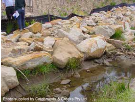
Larger rocks forming toe protection
