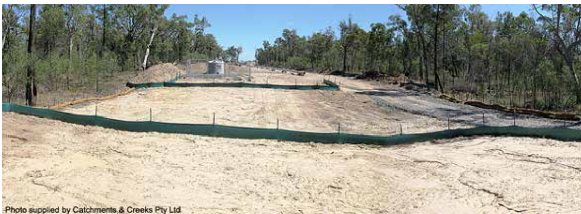
Example of a pipeline crossing a drainage line
