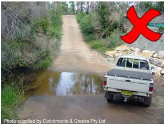
Concrete sealed 'ford' crossing
