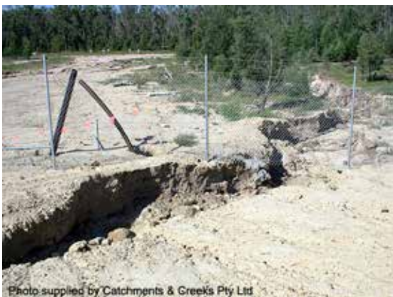
Gully erosion in slaking soil
