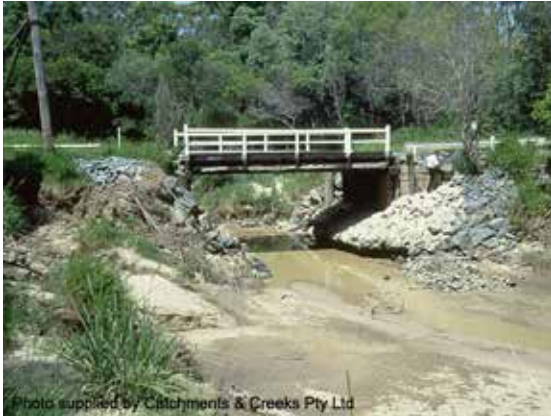
Timber bridge prior to 1996 flood
