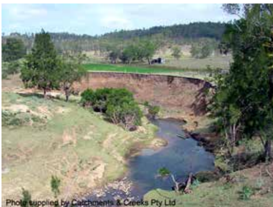
High, unstable river bank
