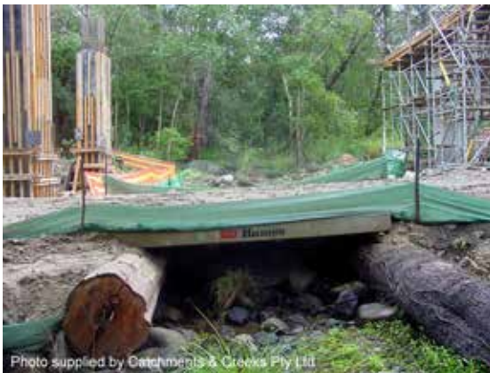
Temporary bridge crossing
