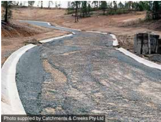
Storm damage to pavement road base
