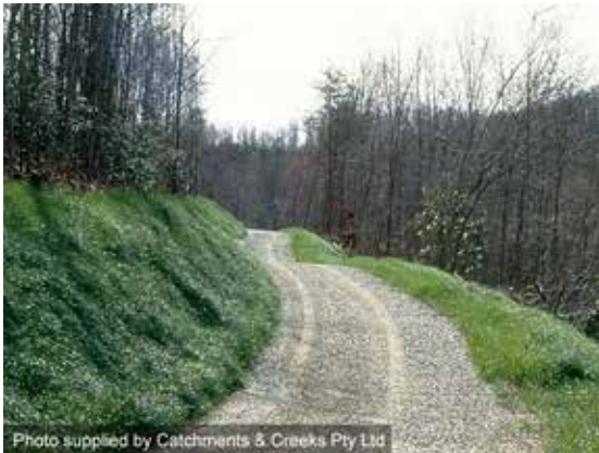
Gravelled access road
