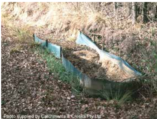
U-shaped sediment trap in steep drain
