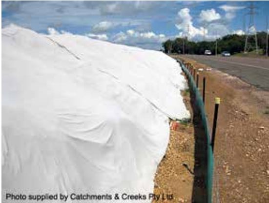
Covering of long-term soil stockpile
