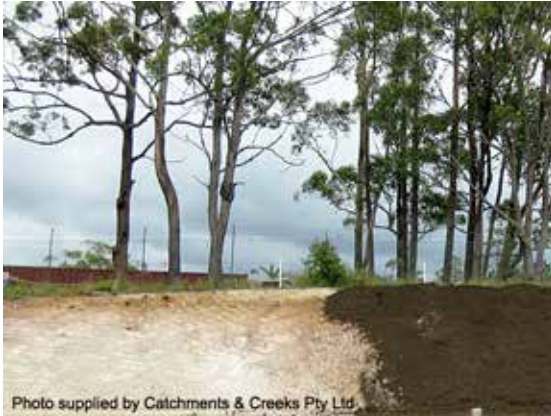
Topsoil placement
