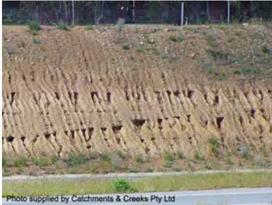
Severe rilling within a dispersive soil
