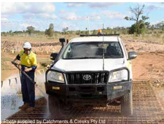
Vehicle wash-down area
