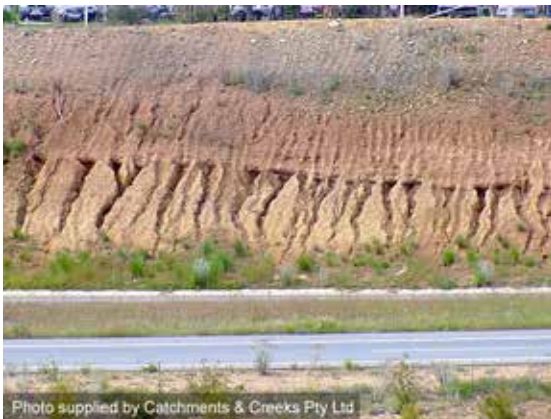
Rilling limited to a given soil horizon
