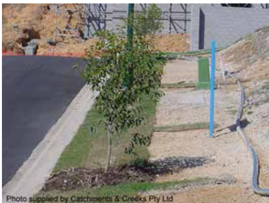
Placement of lateral turf strips
