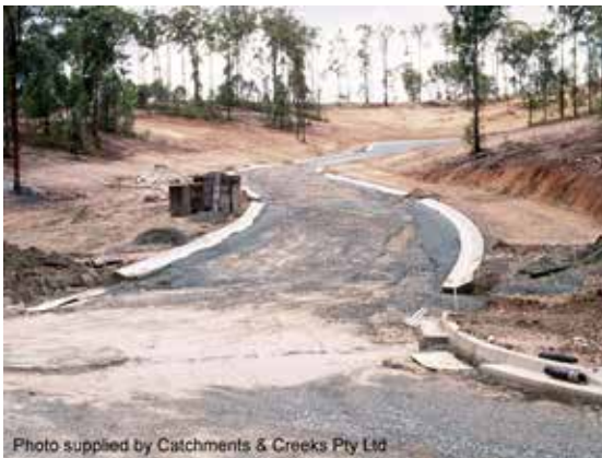
Storm damage to pavement road base
