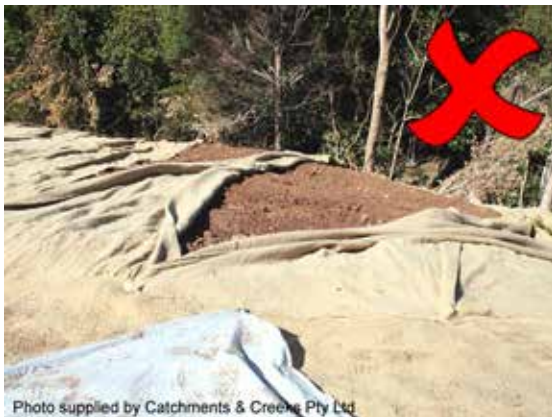
Blankets displaced by wind
