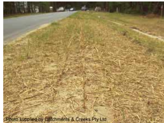
Crimped straw mulch
