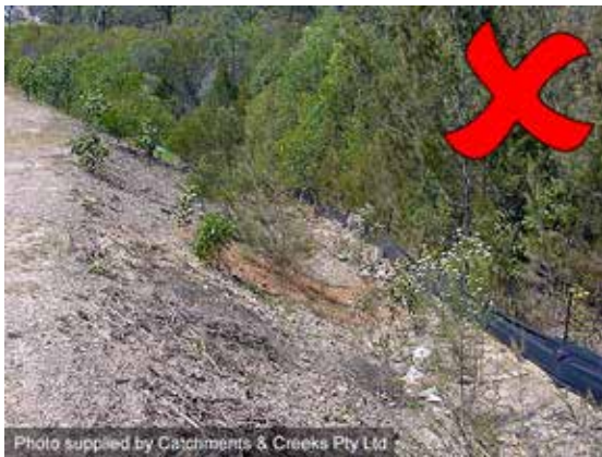
Poor veg growth on heavily-compacted soil
