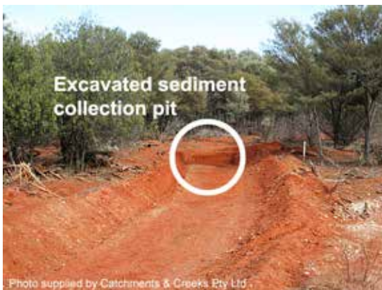
Excavated sediment sump
