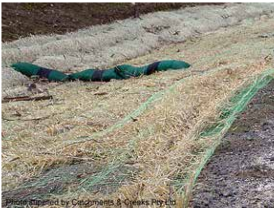
Temporary erosion control mat
