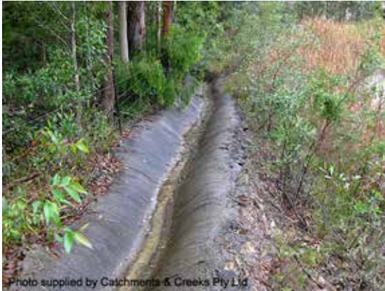
Permanent catch drain
