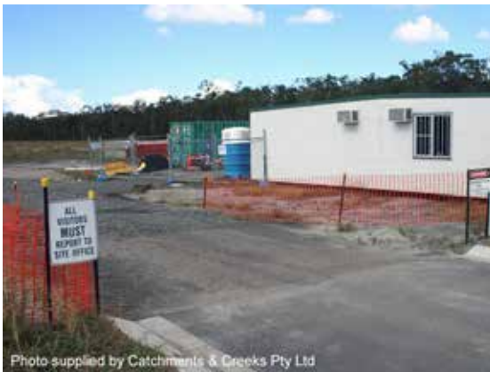
Site entry and office
