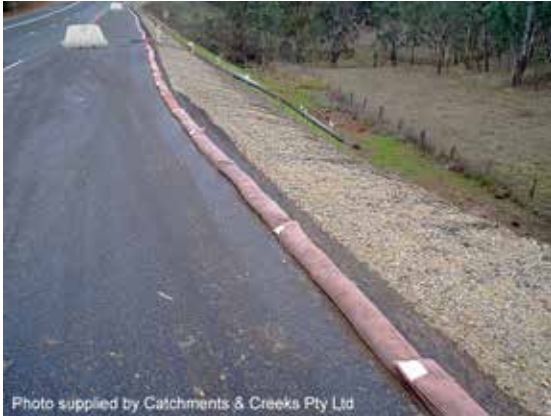
Filter sock flow diversion berm
