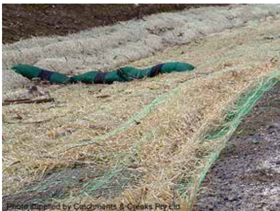
Non UV-stabilised synthetic composite mat
