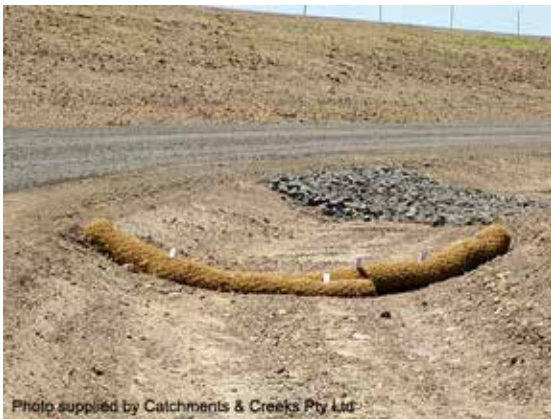
Geo-log check dam
