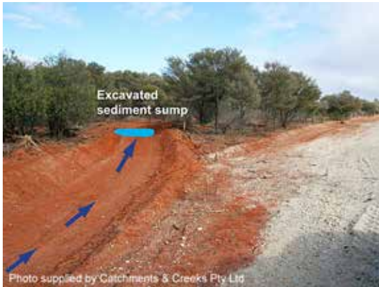
Excavated sediment sump
