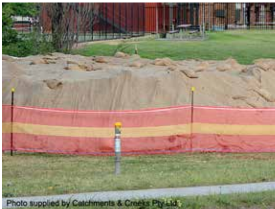
Long-term stockpile covered with jute
