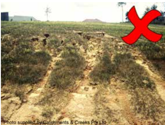
Erosion of recently seeded surface
