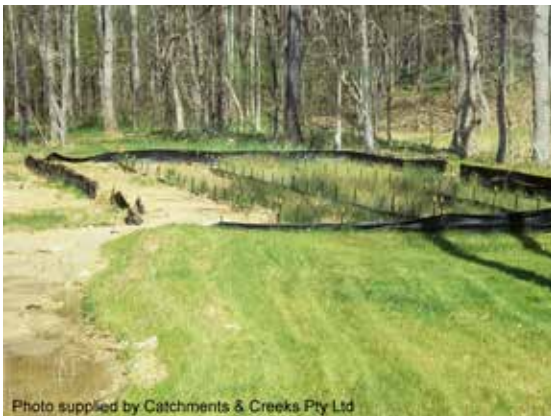
Coarse sediment trap
