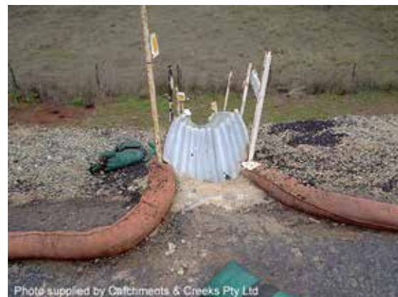
Concrete water seal at chute inlet
