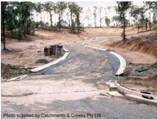
Storm damage to road works
