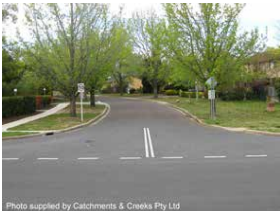
Sealed urban road
