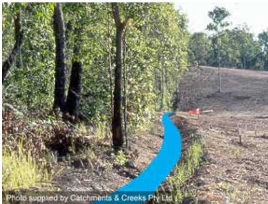
Flow diversion using a catch drain
