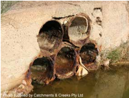
Culvert damaged by acidic water
