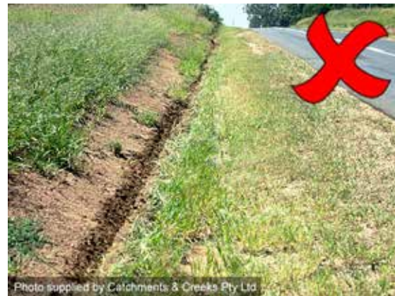
Mechanical disturbance of batter toe
