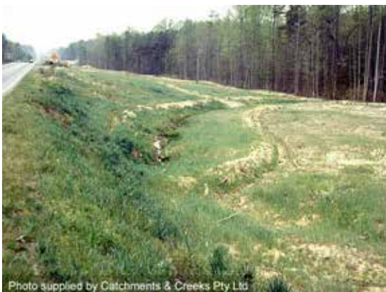
Full vegetation clearing
