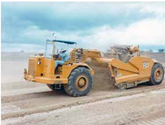
Topsoil stripping
