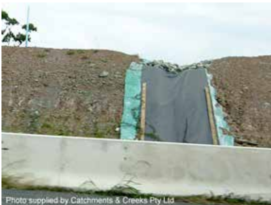
Temporary plastic sheet batter chute
