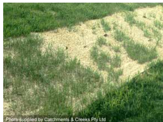
Grass establishing on a thick blanket
