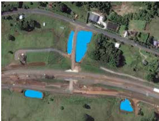
Sediment basins on road construction
