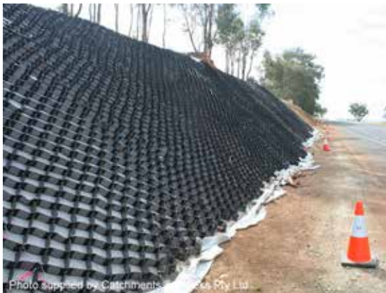
Installation on road batter
