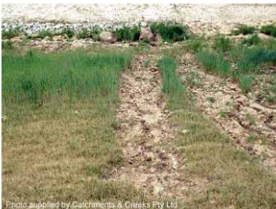
Rill erosion on newly formed fill batter
