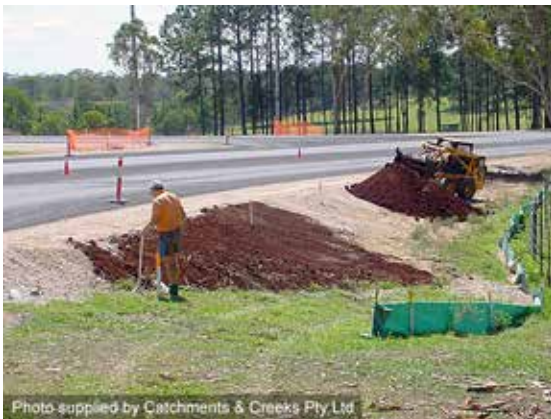
Replacement of topsoil
