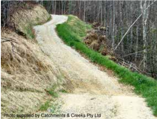
Permanent maintenance access road
