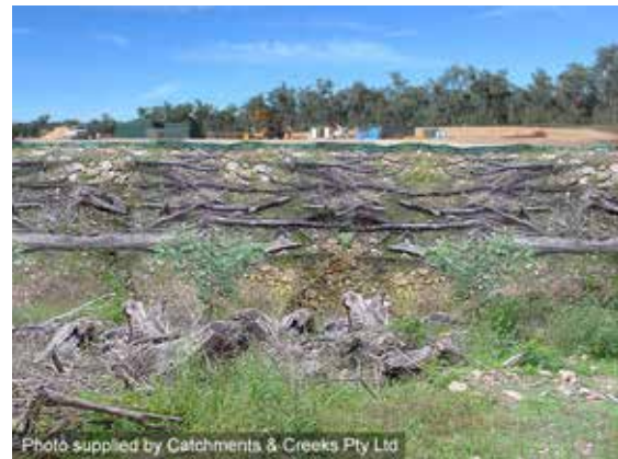
Brushwood used to stabilise a batter
