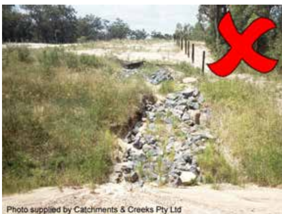
Batter chute placed on a dispersive soil
