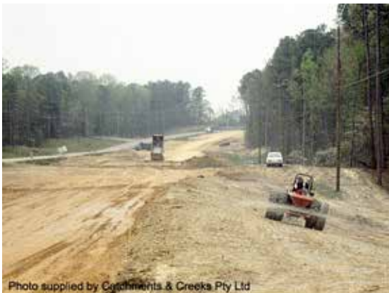
Amelioration of subsoils
