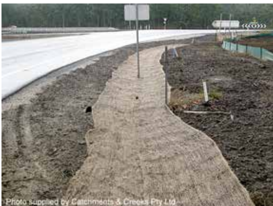
Jute mesh channel lining
