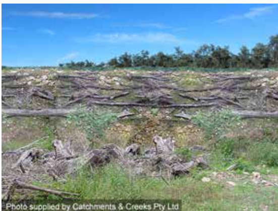
Woody debris placed along a fill batter
