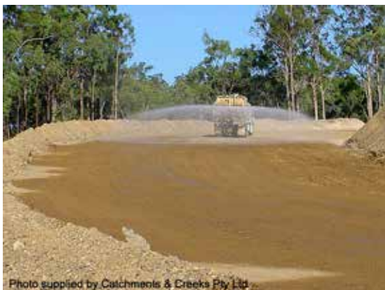
Water truck used for dust control
