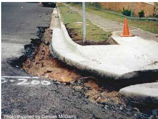
Storm damage to road works
