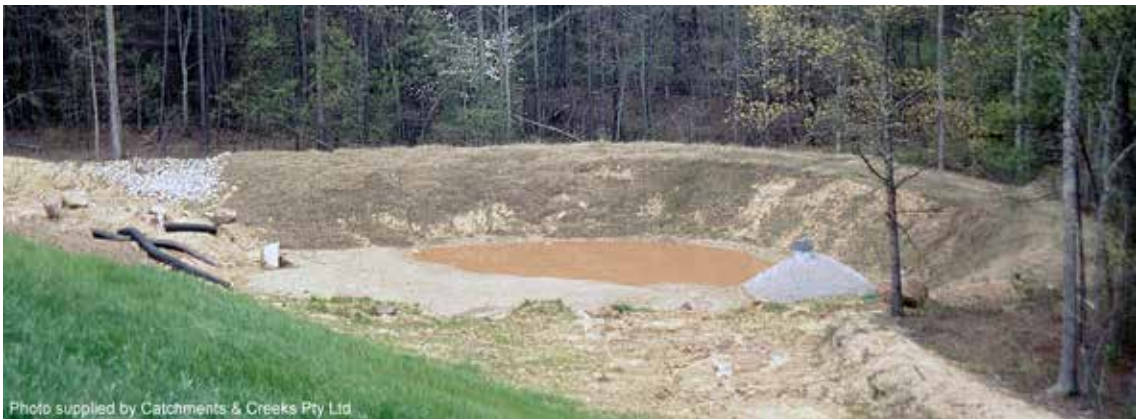
Type C sediment basin with riser pipe outlet (1995)
