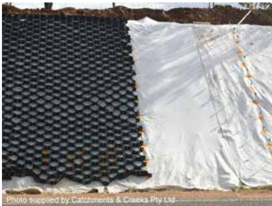
Installation on road batter
