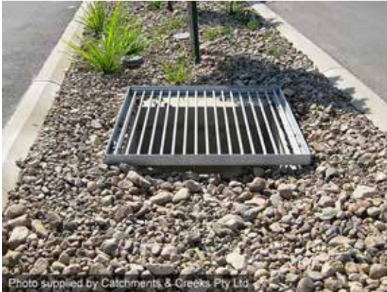
Field inlet located within median strip
