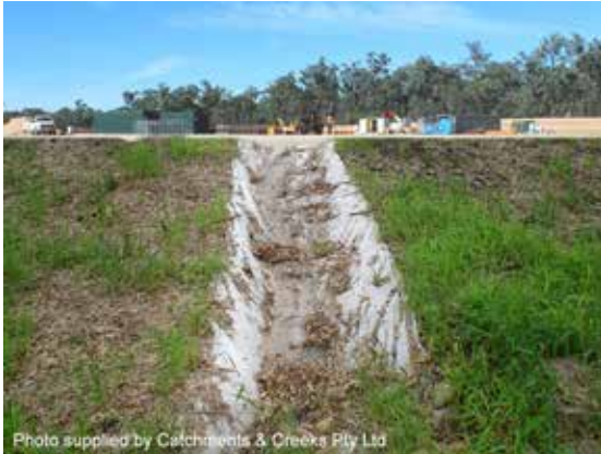
Filter cloth lined batter chute
