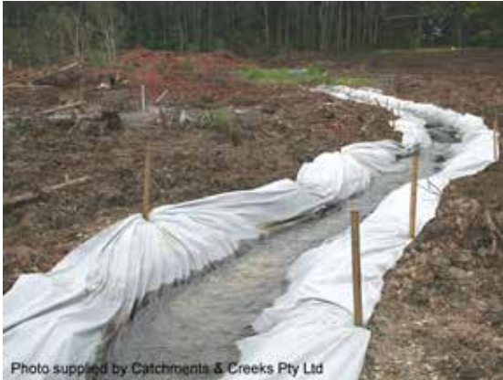
Clean water flow diversion
