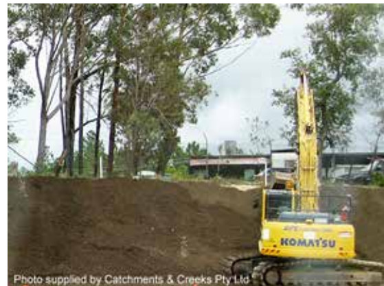
Placement of topsoil
