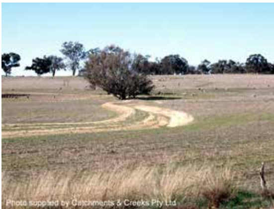
Flow diversion channel
