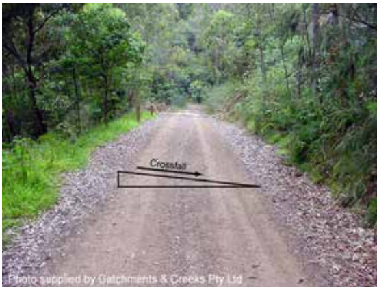
Dirt road with in-fall drainage
