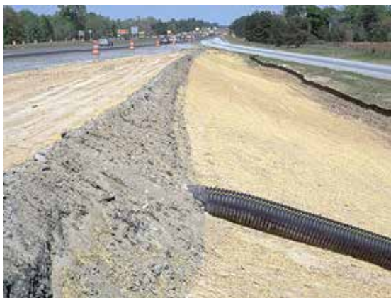
Flow control berm at pipe inlet
