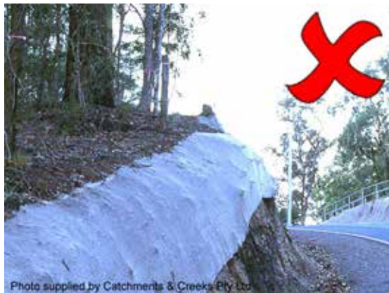
Blanket stretched over irregular ground
