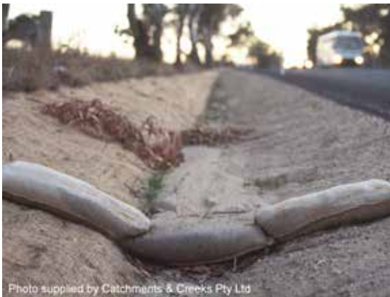
Sandbag check dam
