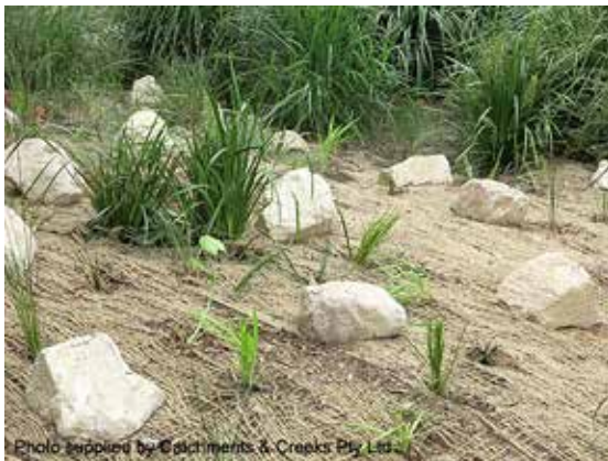
Jute mesh anchored with rocks
