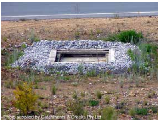
Block & aggregate drop inlet protection
