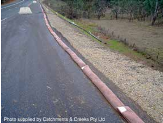
Temporary flow diversion berm
