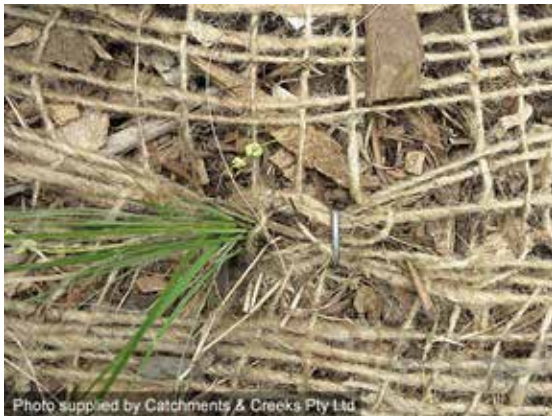
Jute mesh anchoring loose mulch
