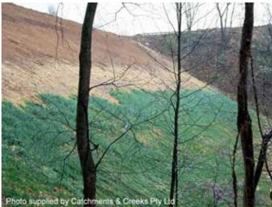
Staged revegetation of road batter
