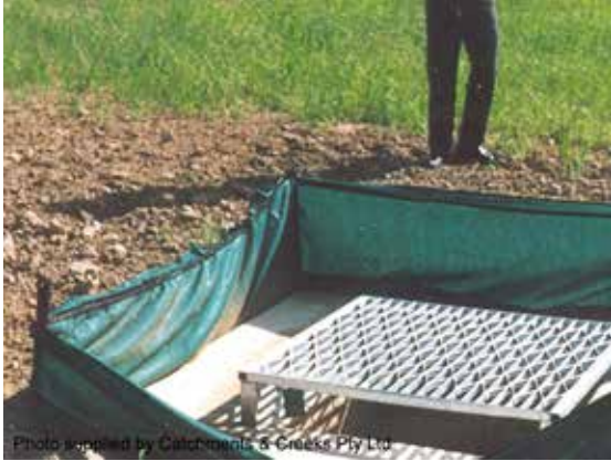
Fabric drop inlet protection
