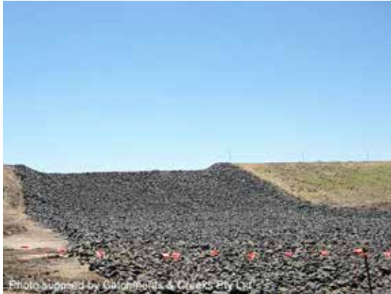
Spillway with well-defined weir profile
