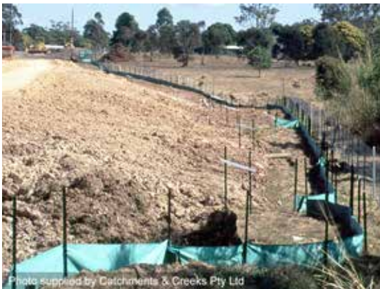
Sediment fence (Type 3)
