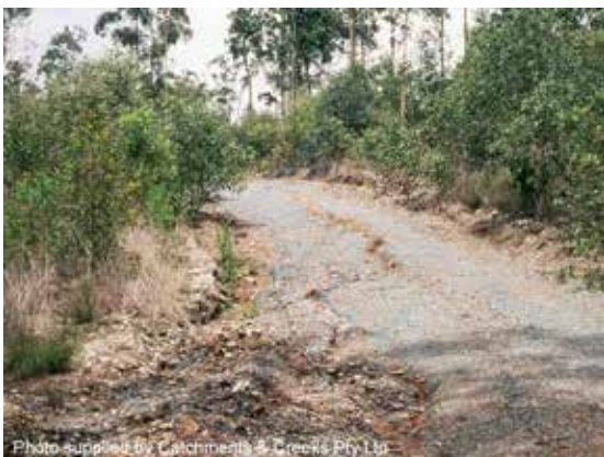
Damage to construction access road
