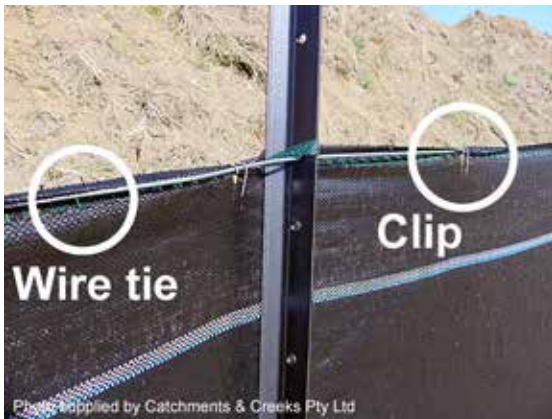
Sediment fence with top wire
