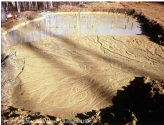
Sediment retained in a basin
