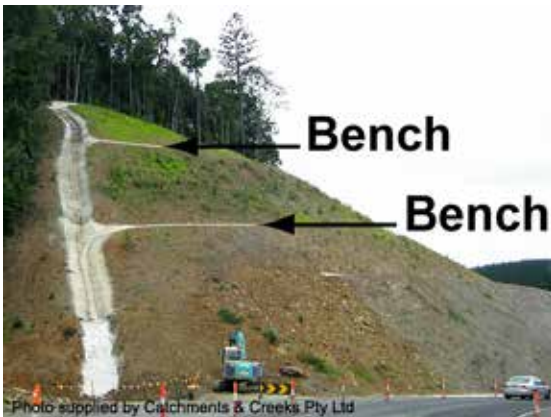
Benched cut batter
