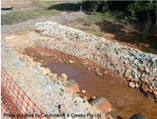
Rock filter dam with aggregate filter
