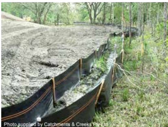
Double sediment fence
