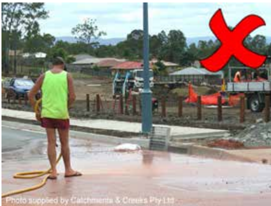
Poor maintenance practice
