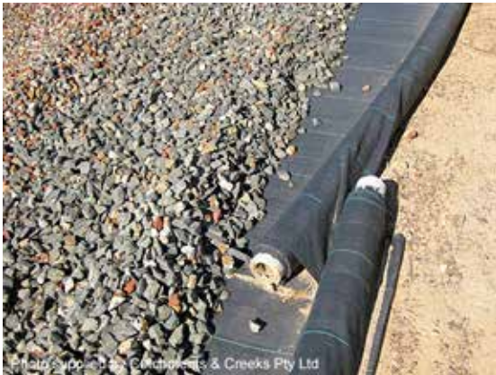
Placement of gravel over geotextile
