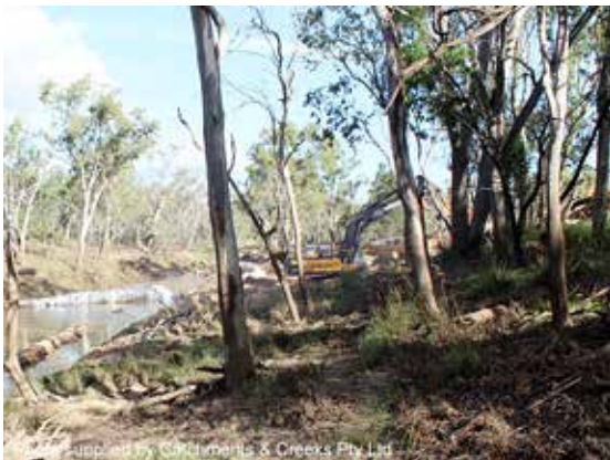
Land clearing adjacent a waterway
