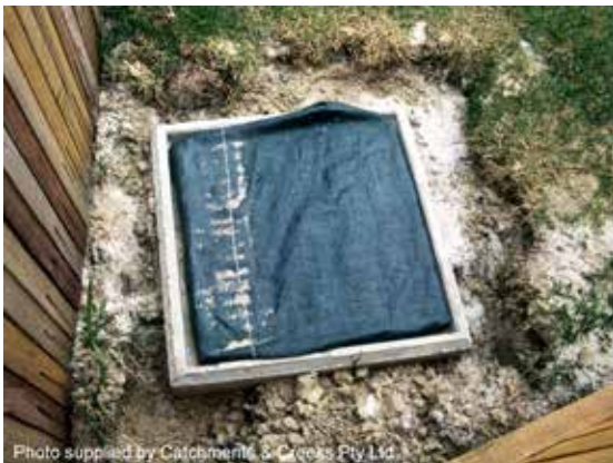
Fabric wrap inlet protection
