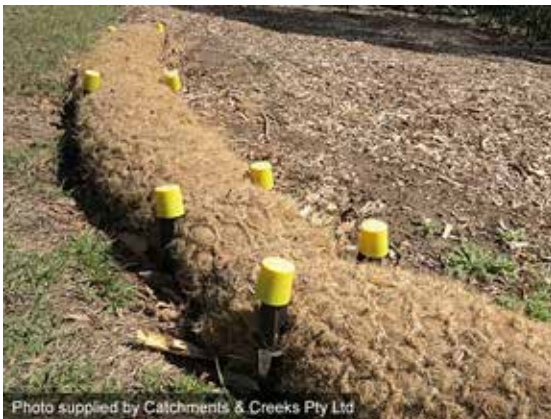
Geo log flow diversion
