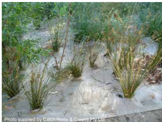
Tube stock planted into a thick blanket
