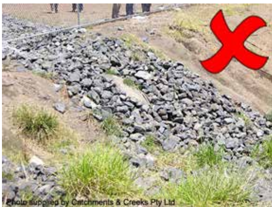
Rocks slipping down batter chute
