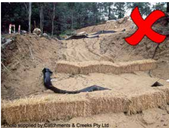
Stormwater traps placed on site access
