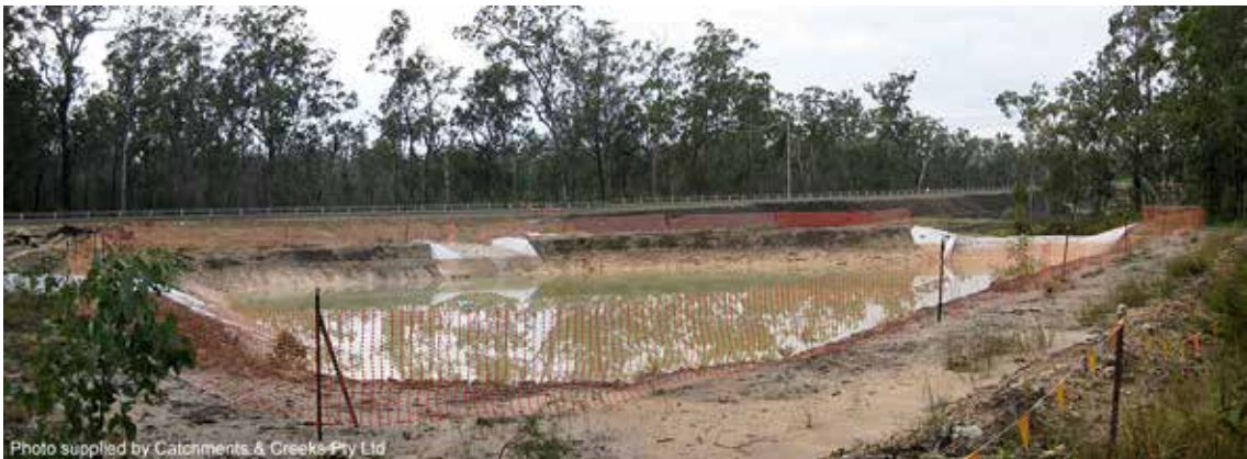
Type C sediment basins with siphon pipe decant system (2017)
