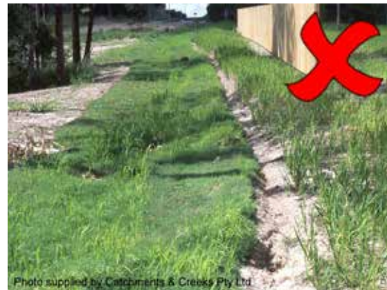
Rilling along the edge of turf
