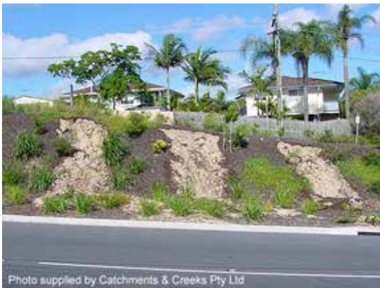
Storm damage to road batter
