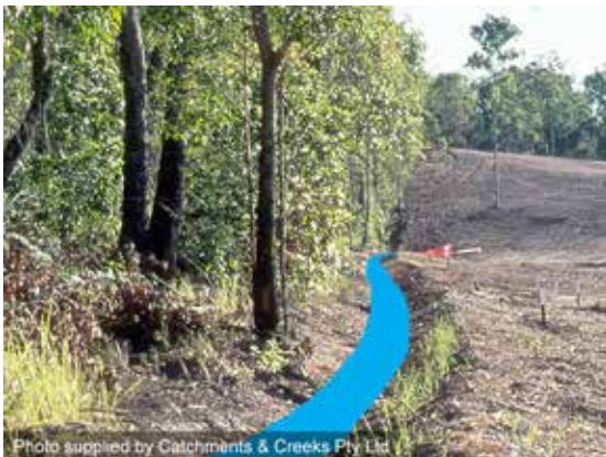
Catch drain used to divert run-on water
