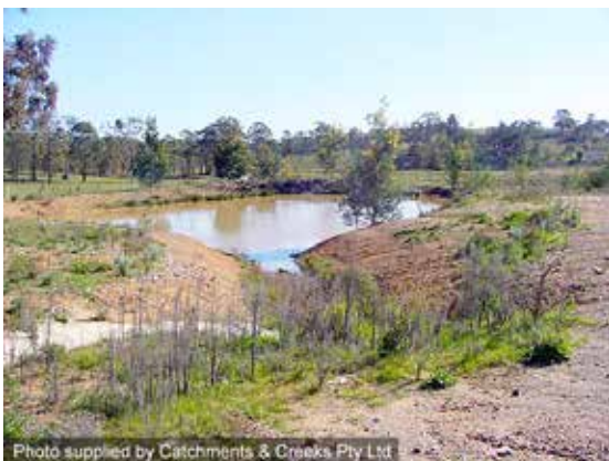
Post-construction farm dam
