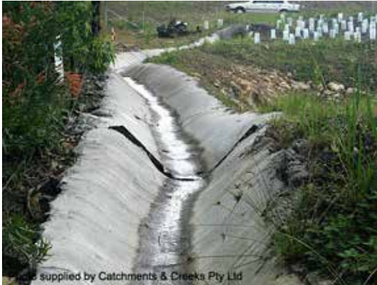
Concrete-lined catch drain
