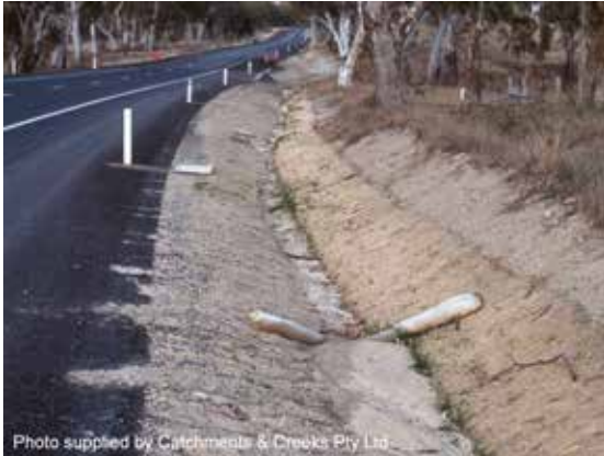
Sandbag check dams
