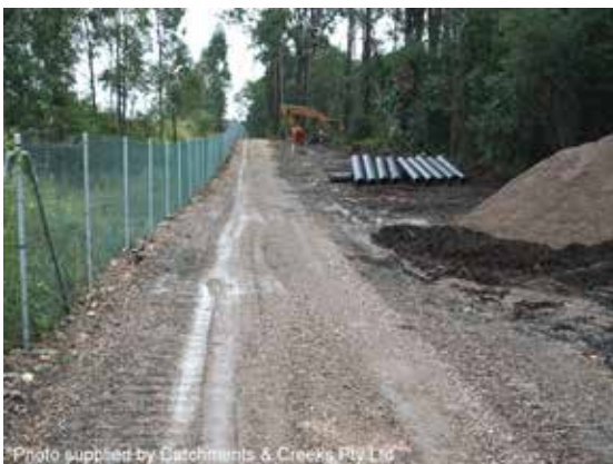
Unsealed construction access road
