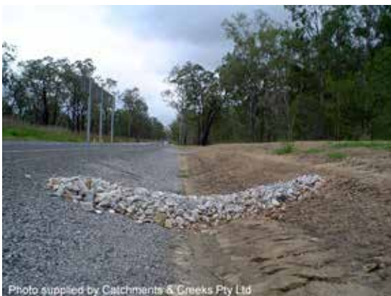
Rock check dam
