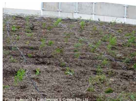
Revegetated stair-stepped batter
