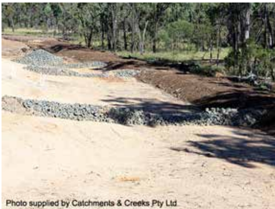
Velocity control check dams
