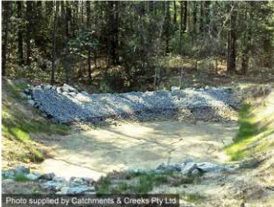
Rock filter dam - aggregate filter
