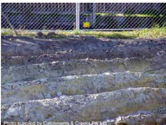
Stair-stepping of steep batter
