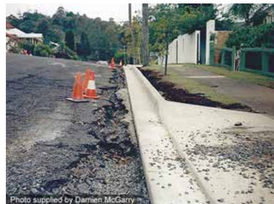
Storm damage to road works
