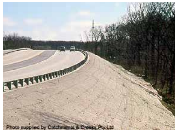
Erosion control blankets
