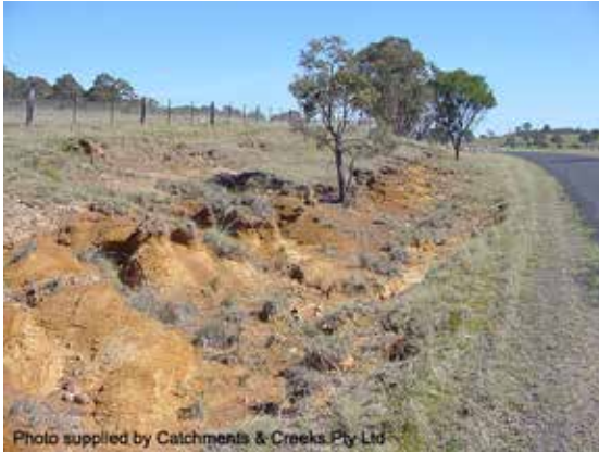
Erosion of a dispersive soil
