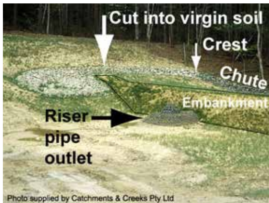
Spillway formed within virgin soil
