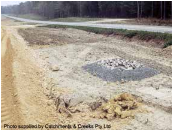
Rock & aggregate drop inlet protection
