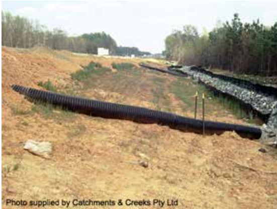
Temporary and permanent road drainage
