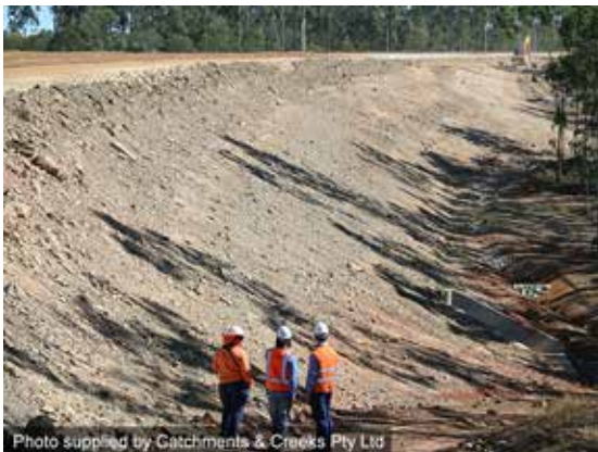
Road batter awaiting stabilisation
