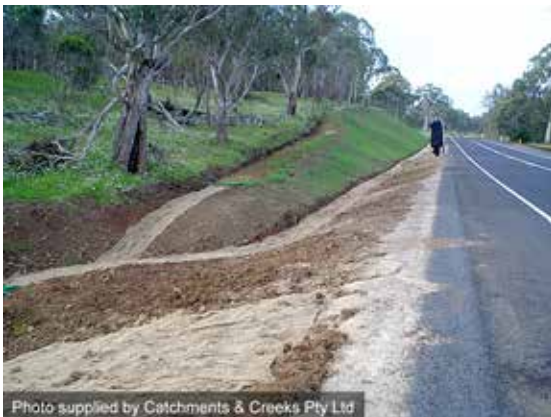
Flow diversion drains
