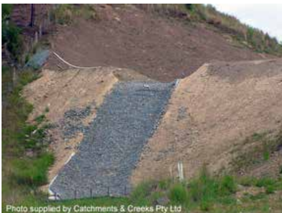
Mattress-lined sediment basin spillway
