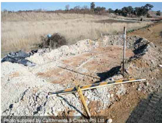
Concrete truck wash-out point
