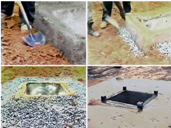
Excavated drop inlet protection
