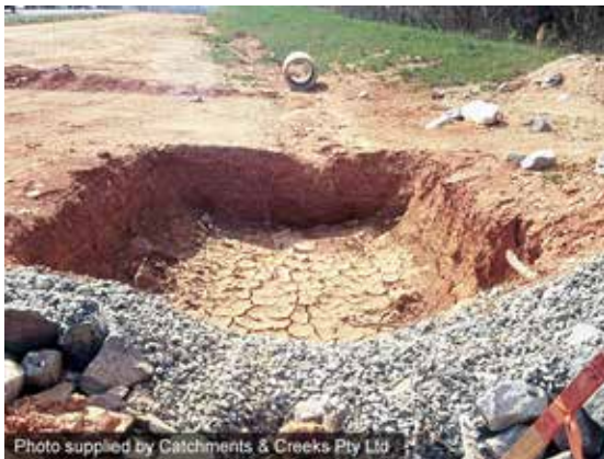
Excavated sediment sump
