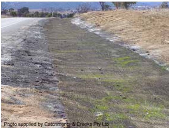
Jute mesh with bitumen seal
