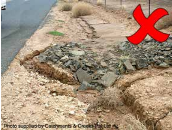
Rock check dam placed on dispersive soil
