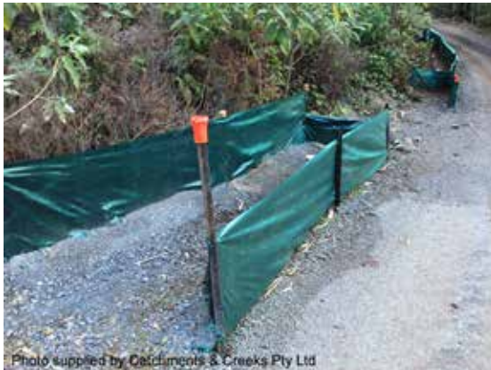
U-shaped sediment trap
