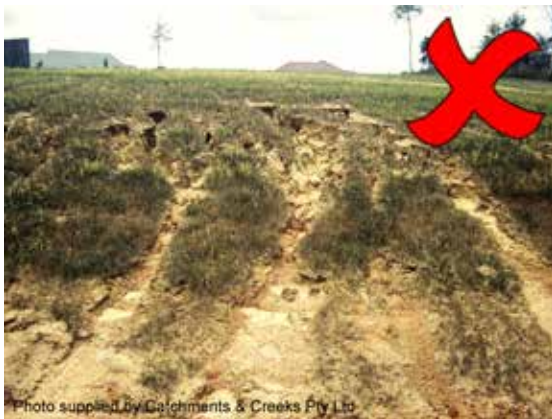
Failed revegetation of a dispersive soil
