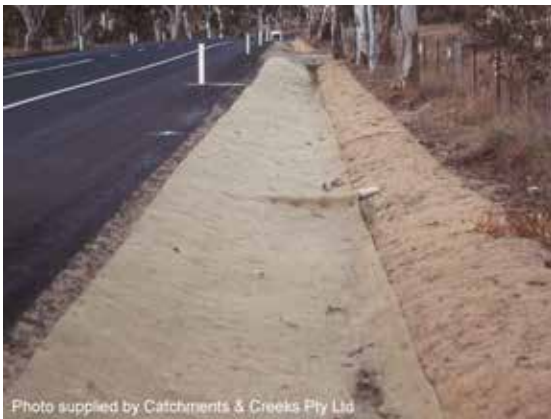
Jute erosion control mat
