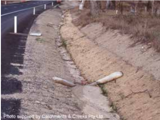
Check dam sediment trap
