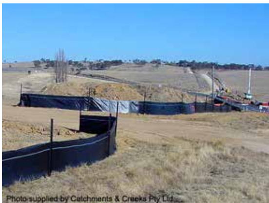
Sediment control down-slope of stockpile
