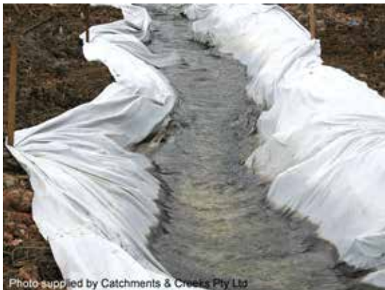
Filter cloth anchored with timber stakes
