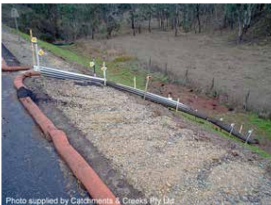
Corrugated iron batter chute
