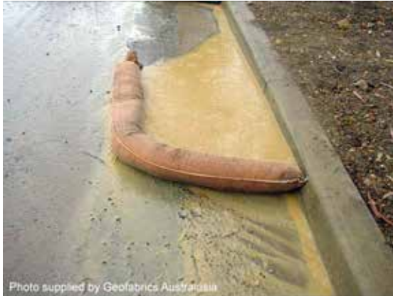
Sand-filled filter sock
