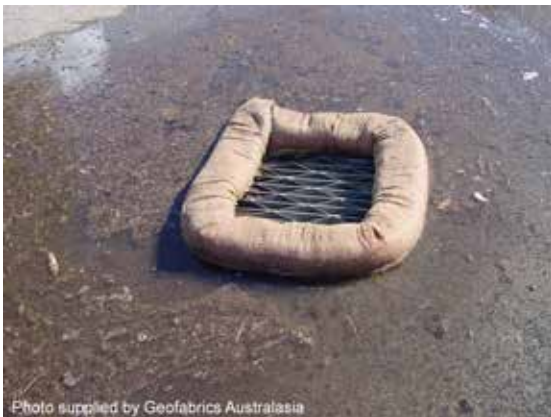
Filter sock drop inlet protection
