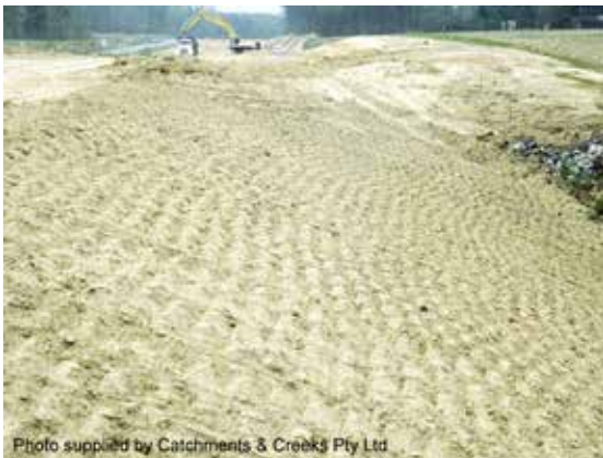
Roughened earth batter
