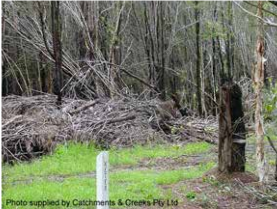
Brushwood barrier sediment trap
