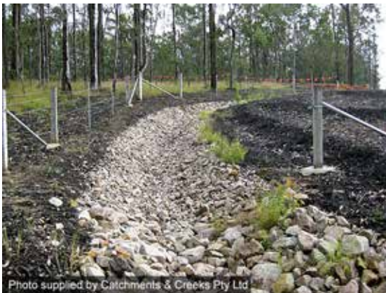
Rock-lined catch drain
