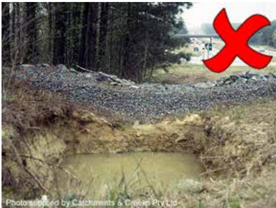
Excavated sediment trap
