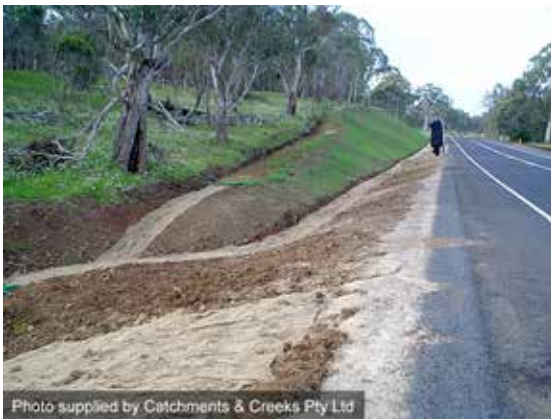
Catch drain and table drain
