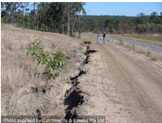
Bench cut into a dispersive soil
