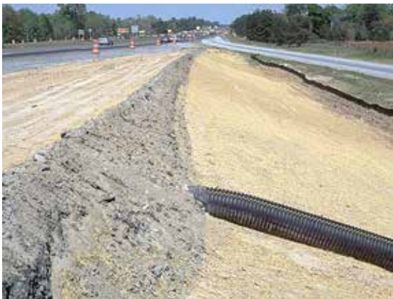
Topsoil flow diversion bank
