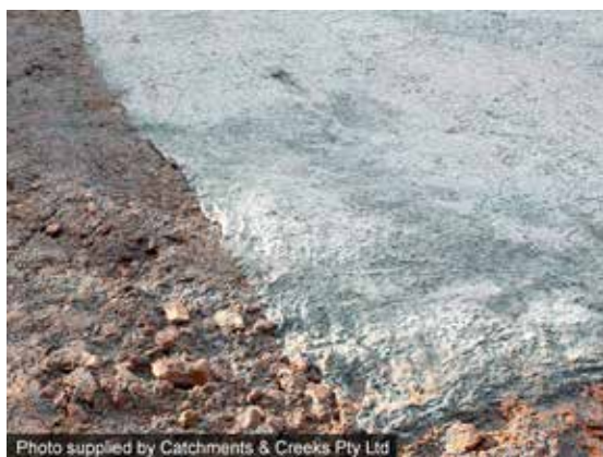
Thick blanket seeded with BFM
