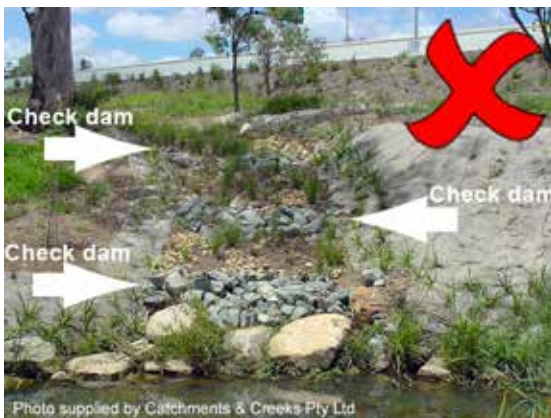
Check dams placed on a batter chute
