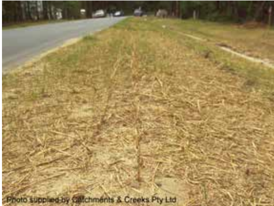
Straw mulching of road shoulder
