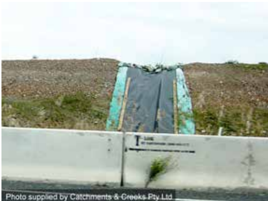
Temporary batter chute
