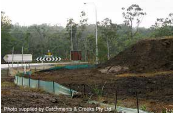
Stockpile placed up-slope of road works
