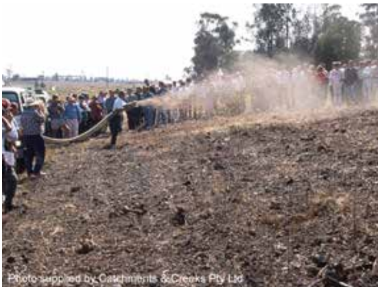
Straw mulching of a road batter
