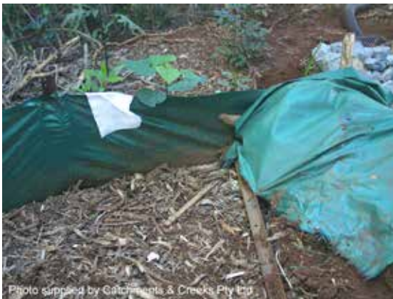
Damaged fence tagged for repair
