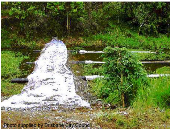
Rock filter dam with filter tubes
