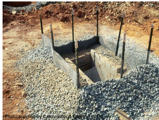
Mesh & aggregate drop inlet sediment trap
