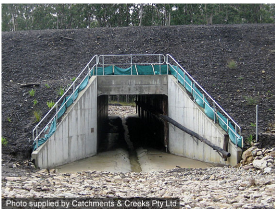
Fauna passage culverts
