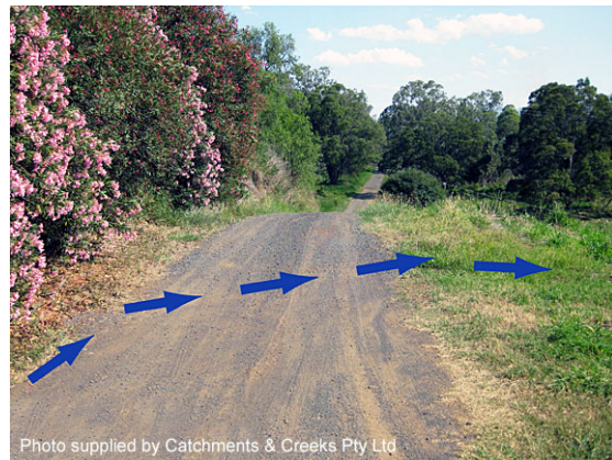
Cross bank placed at top of descent
