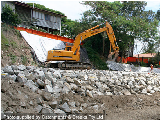
Rock placement over filter cloth
