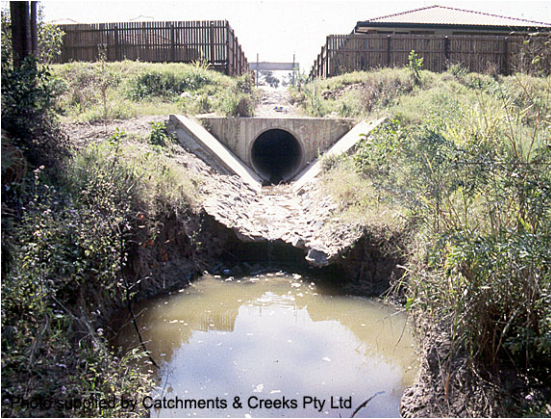
Pipe outlet pre-construction
