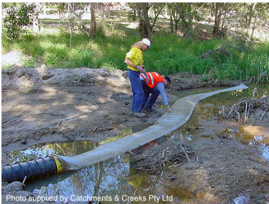
In-stream sediment control system
