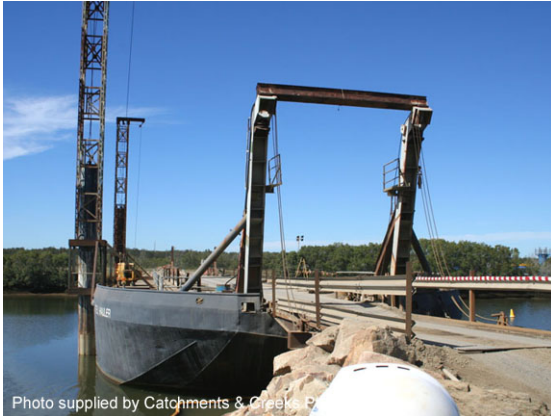
Barge crossing of tidal inlet
