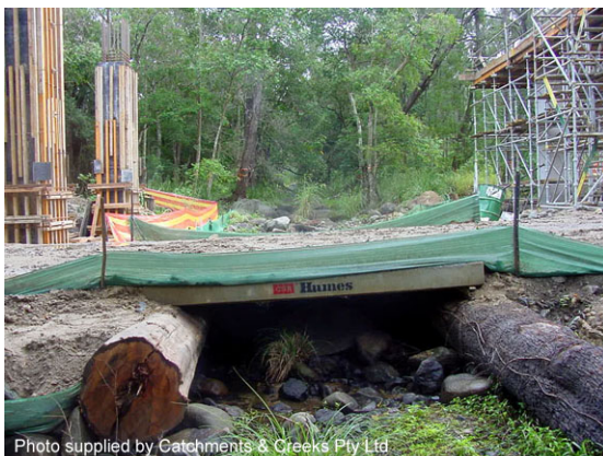
Temporary stream crossing
