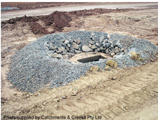
Rock & aggregate drop inlet sediment trap
