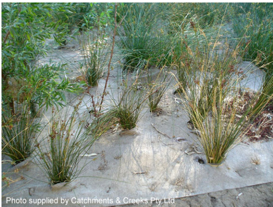
Jute erosion control blanket
