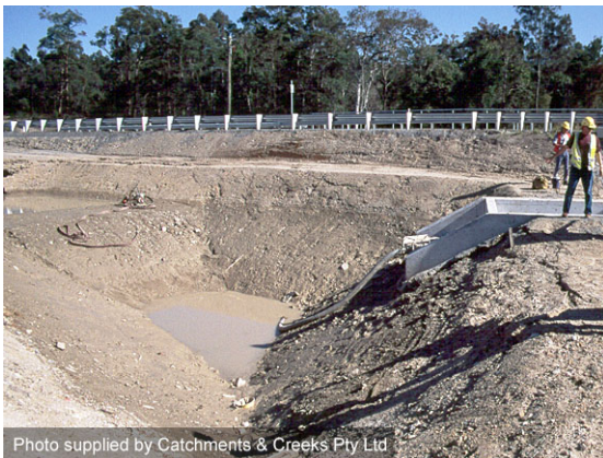
Sediment basins (Type 1 sediment trap)
