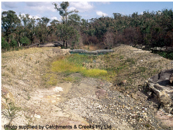
Type 2 sediment trap (1994)
