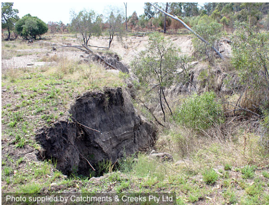
Lateral bank erosion
