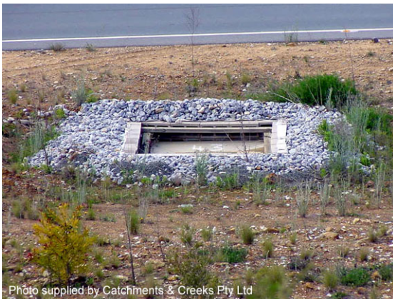
Block & aggregate drop inlet trap
