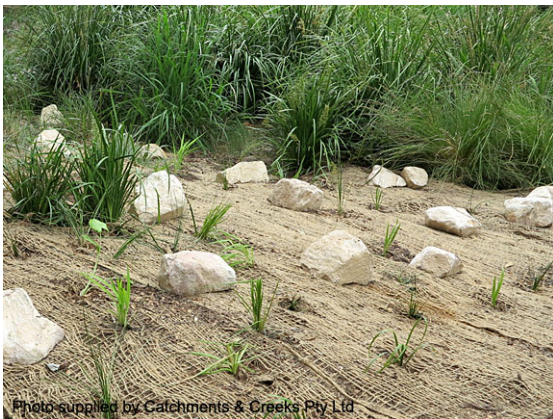
Jute mesh with additional rock anchors
