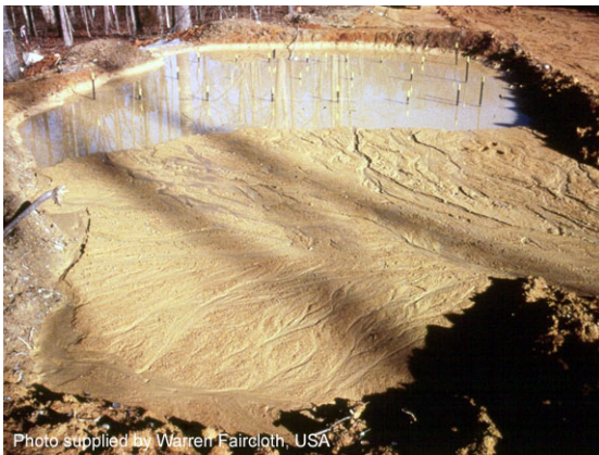
Sediment retained in a sediment trap
