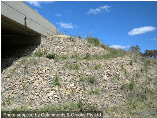
Vegetated rock mattresses
