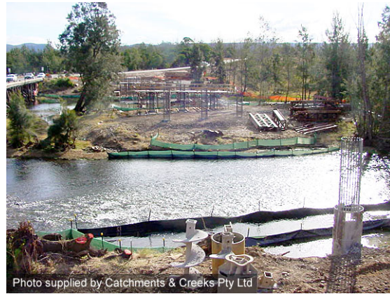
Photo supplied by Catchments & Creeks Pty Ltd
