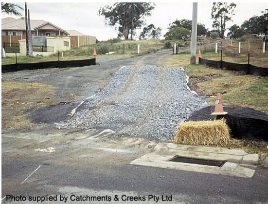
Rock pad with flow diversion berm
