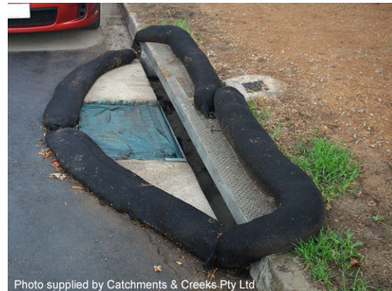
'Sag' kerb inlet sediment trap
