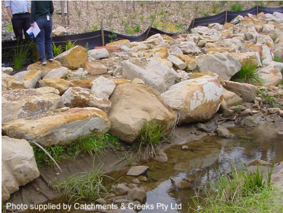
Larger rocks forming toe protection
