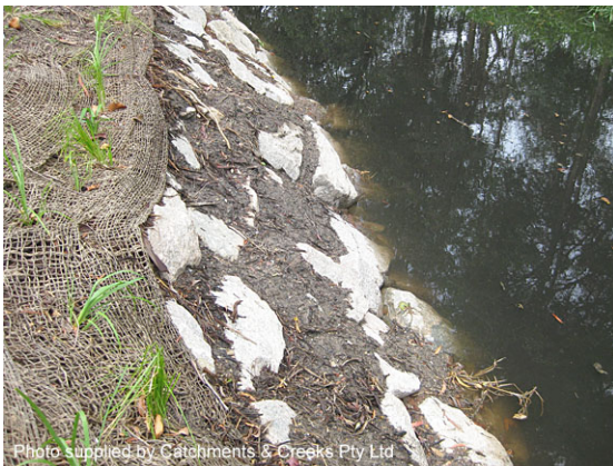
Voids filled with soil ready for planting
