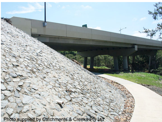
Grouted stone pitched abutment
