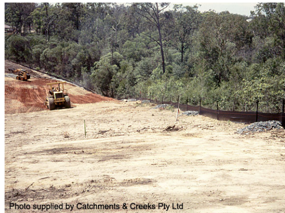
Sediment fence with rock check dams
