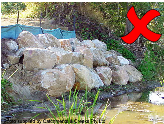
Poorly placed rocks on creek bank
