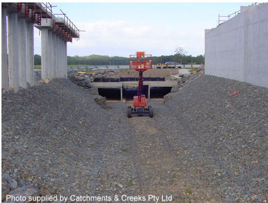
Non-vegetated rock mattresses
