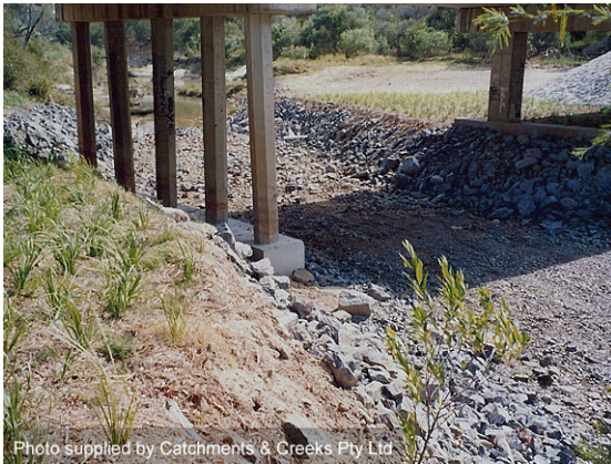
Rock stabilisation of bed and banks
