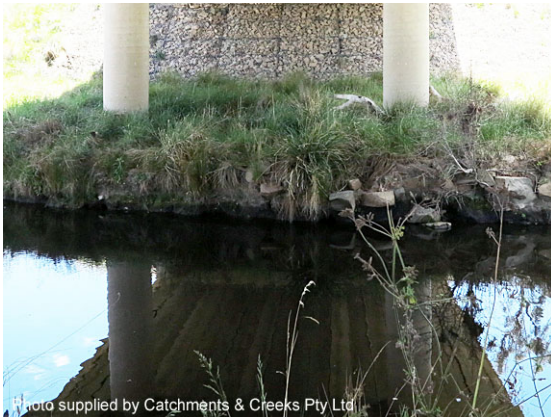
Vegetated rock stabilisation
