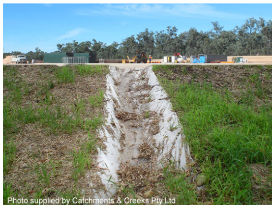
Temporary batter chute
