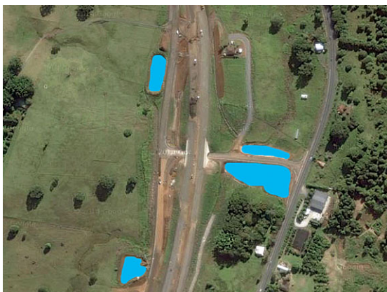
Rural road construction
