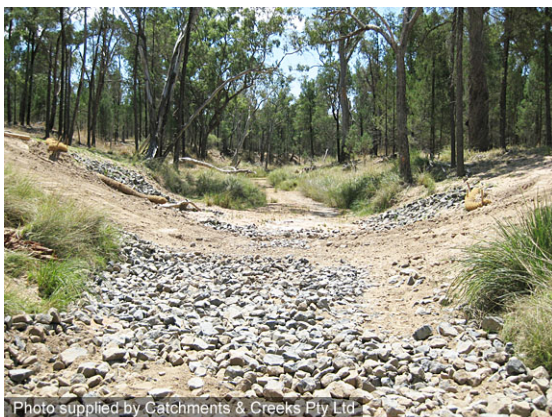
Rock stabilised vehicle crossing
