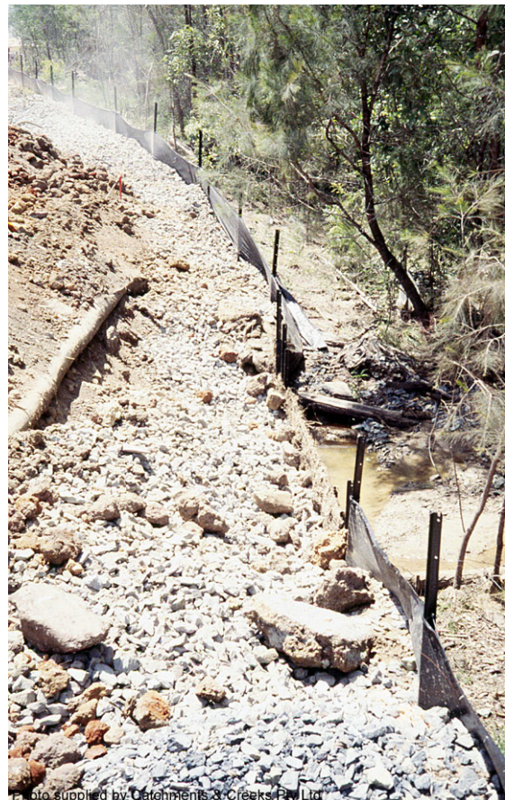
Spill-through weir & aggregate filter
