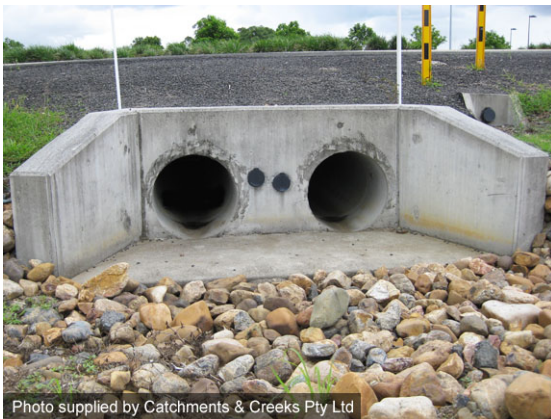
Minor culvert crossing
