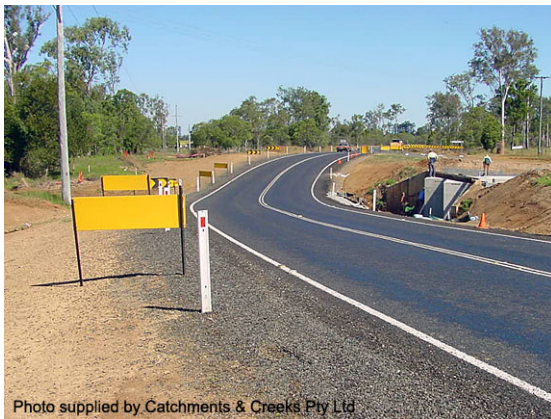
Temporary bypass road
