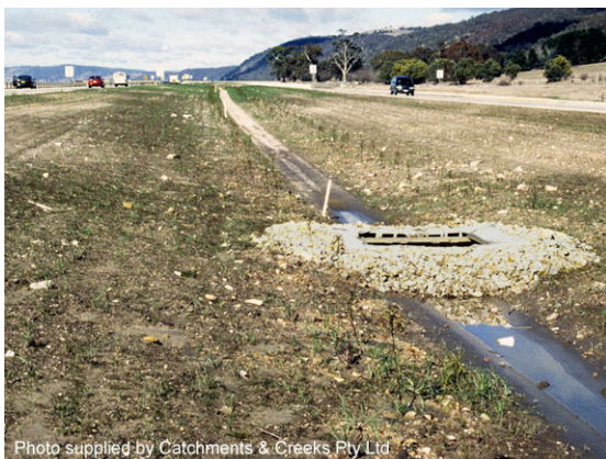
Drop inlet sediment trap
