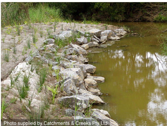
Vegetated rock stabilisation of bank
