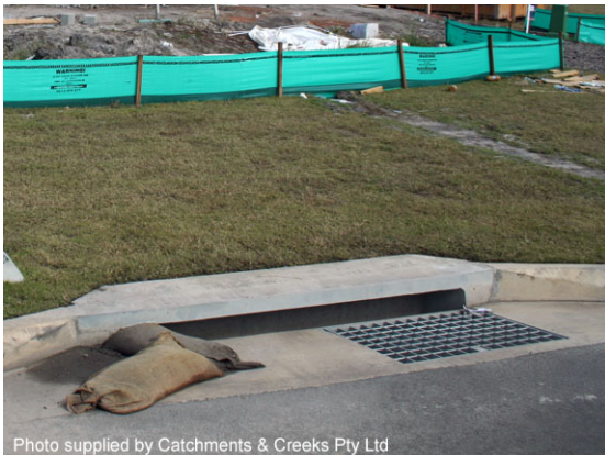
'On-grade' kerb inlet sediment trap
