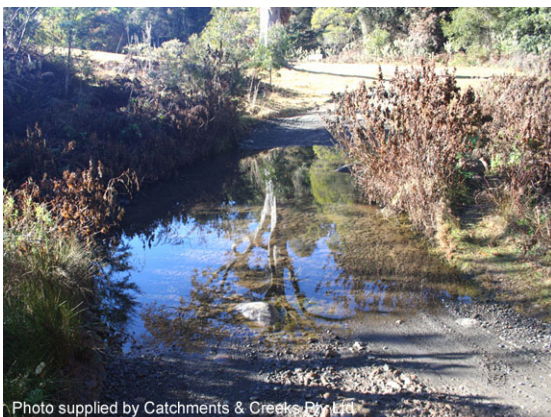
Ford crossing of alluvial stream
