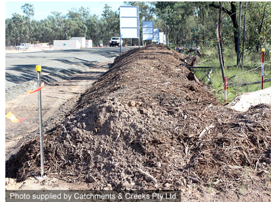
Mulch berm sediment barrier
