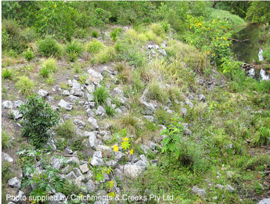
Planted rock-stabilised creek bank
