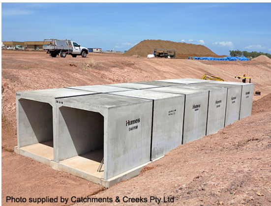
Culvert construction in a dry channel
