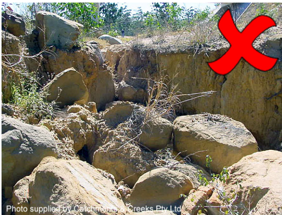
Collapsed dispersive soil bank
