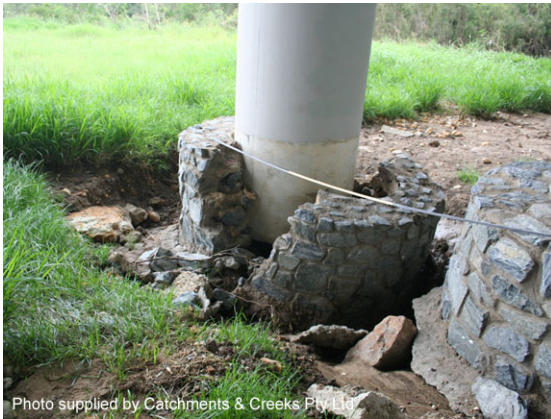
Flood damage to bridge pier
