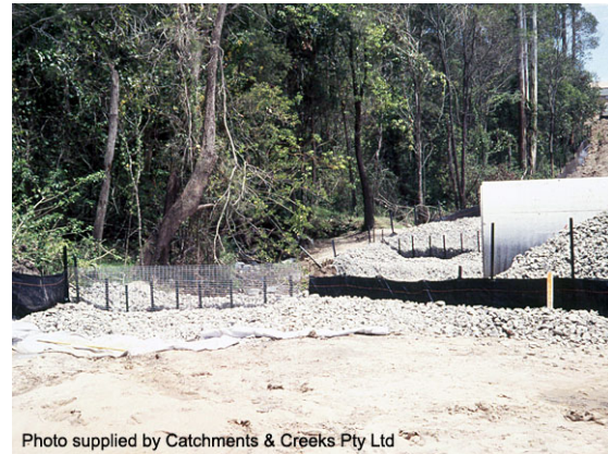
Rock filter dam outlet structure
