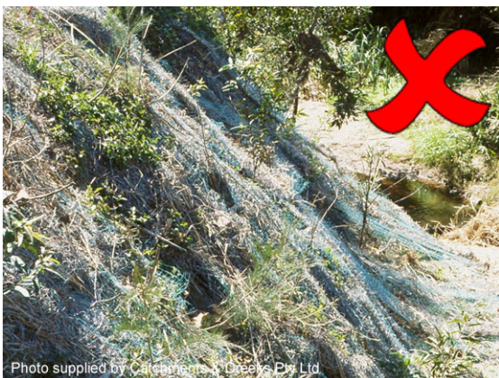
Synthetic reinforced erosion control mat
