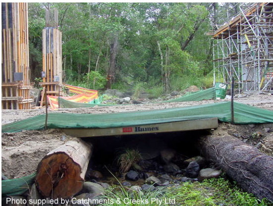
Temporary access construction bridge
