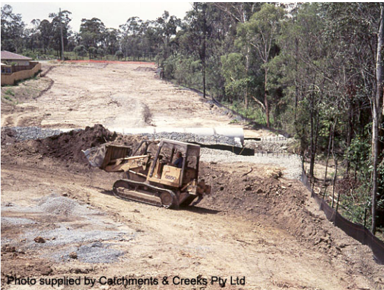
Excavating a sediment basin
