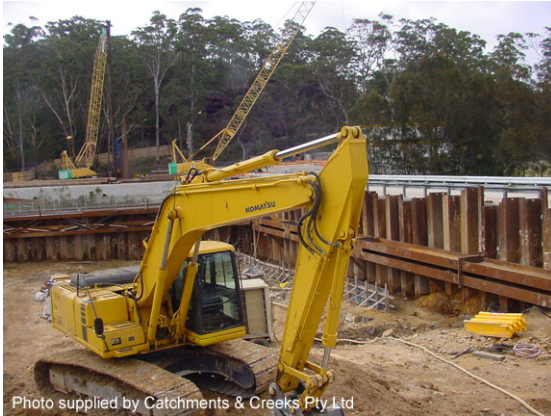
Sheet piling isolation barrier
