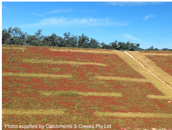
Turf filter strips placed along the contour
