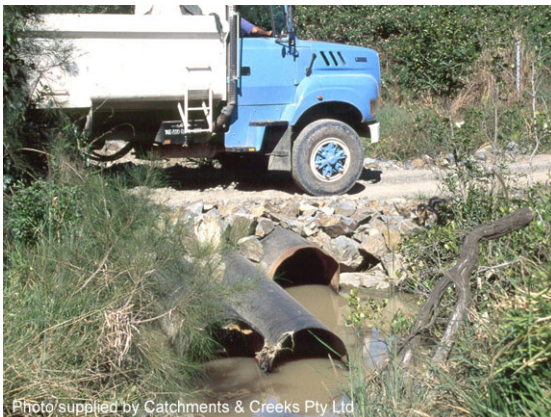
Temporary pipe culvert
