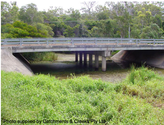
Concrete abutments
