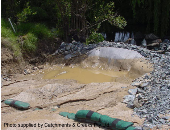
Rock filter dam (Type 2 sediment trap)
