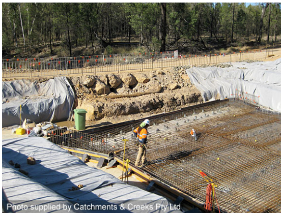
Construction of a culvert base slab
