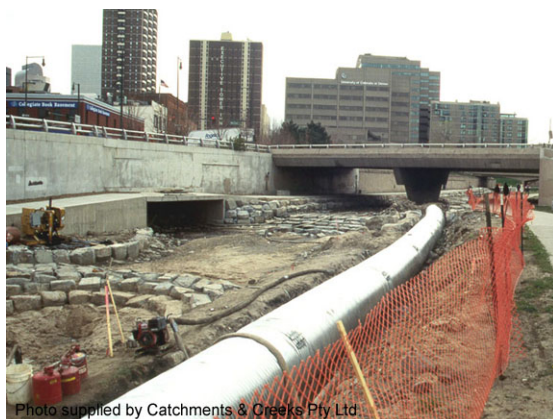
Instream works with piped-flow bypass
