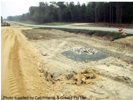
Type 2 drop inlet sediment trap
