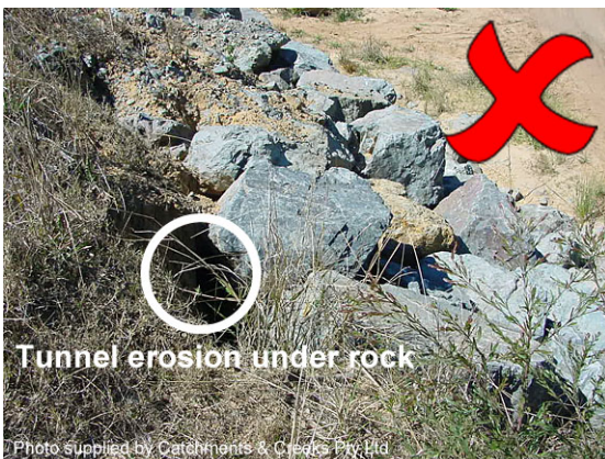
Tunnel erosion under rocks
