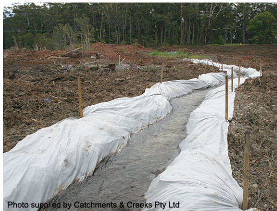
Clean water cross-drainage system
