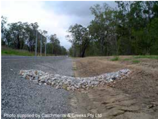
Velocity control check dam
