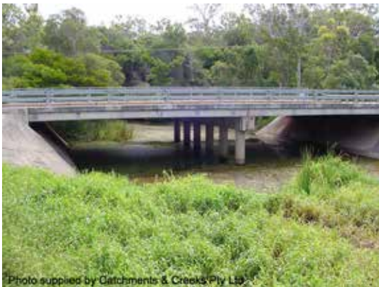
Concrete abutments
