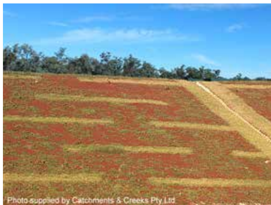
Turf filter strips placed along the contour
