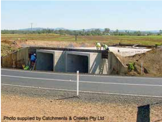
Culvert construction
