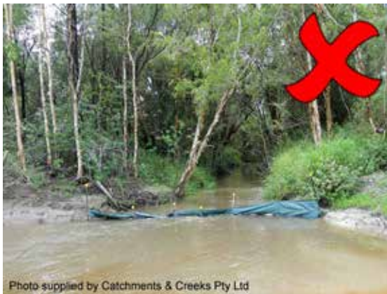
Inappropriate in-stream sediment control
