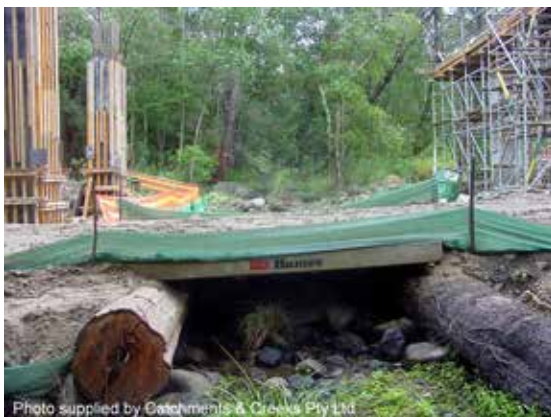
Temporary stream crossing
