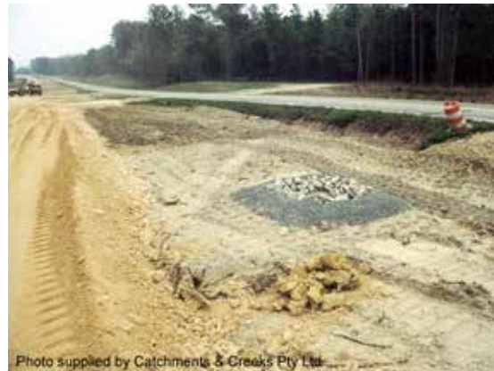
Rock & aggregate drop inlet sediment trap
