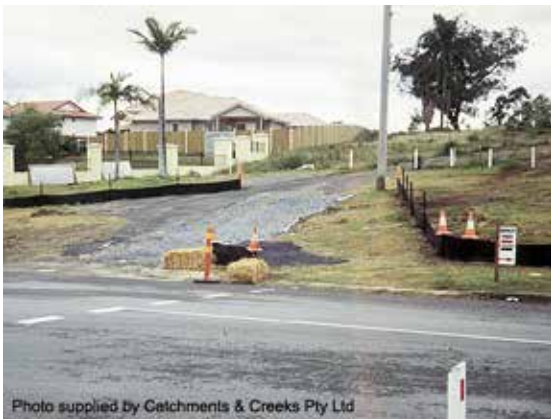
Heavy vehicle site entry point
