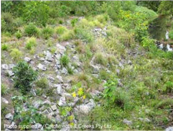
Planted rock-stabilised creek bank
