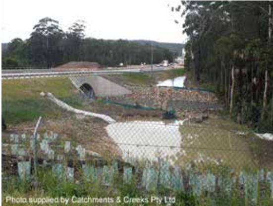
Sediment basins (Type 1 sediment trap)
