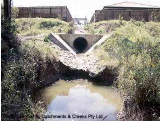
Pipe outlet pre-construction
