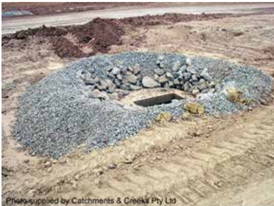
Rock & aggregate drop inlet sediment trap
