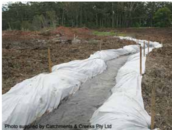
Clean water cross-drainage system
