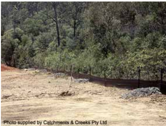
Check dams adjacent a sediment fence
