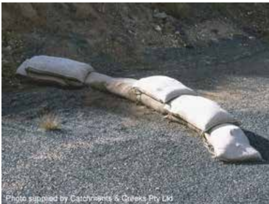
Check dam sediment trap
