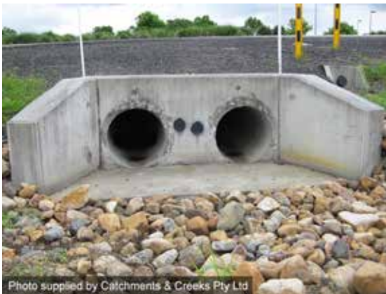
Minor culvert crossing
