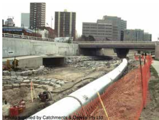
Instream works with piped-flow bypass
