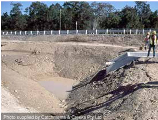
Sediment basins (Type 1 sediment trap)
