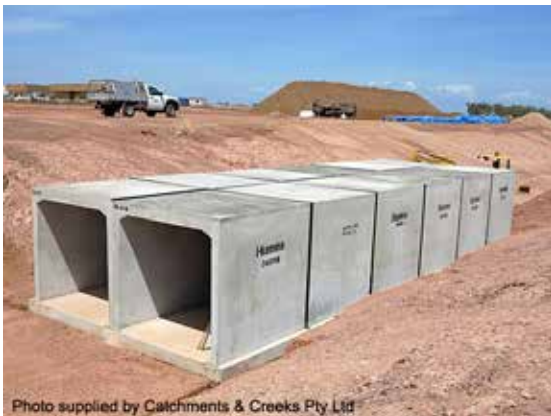
Culvert construction in a dry channel
