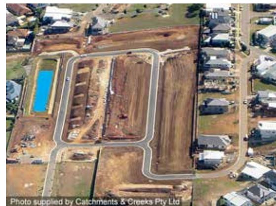
Residential road construction
