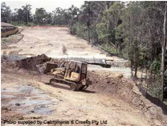
Excavating a sediment basin
