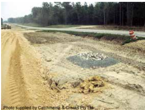
Type 2 drop inlet sediment trap
