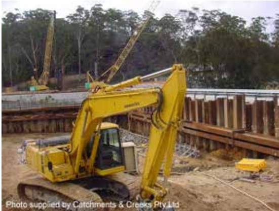
Sheet piling isolation barrier
