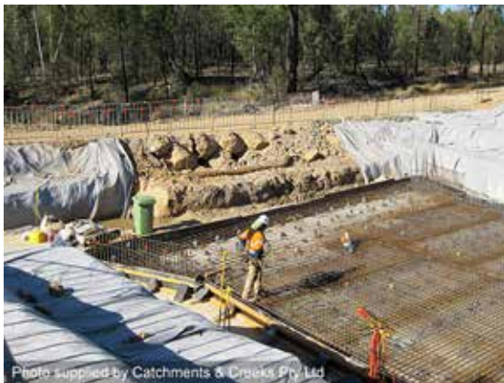
Construction of a culvert base slab
