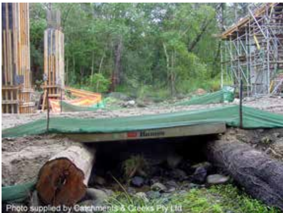
Temporary access construction bridge
