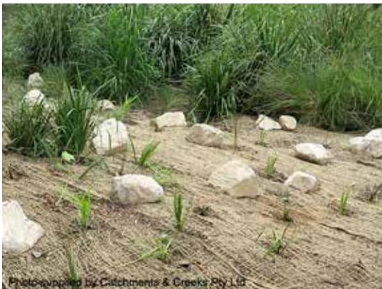
Jute mesh with additional rock anchors
