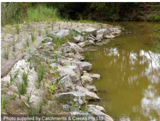
Vegetated rock stabilisation of bank
