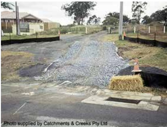
Rock pad with flow diversion berm
