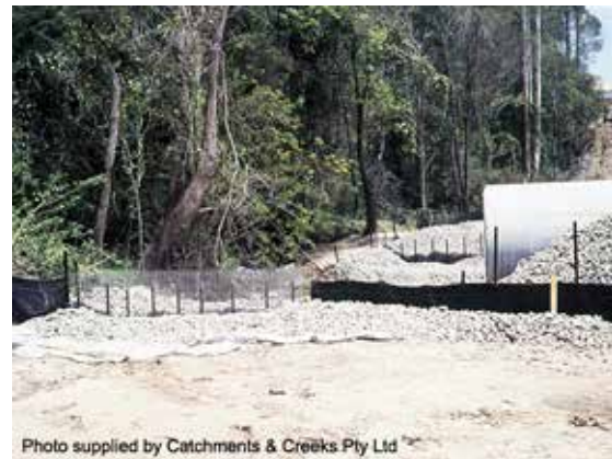
Rock filter dam outlet structure
