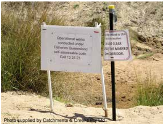
Signage at in-stream works
