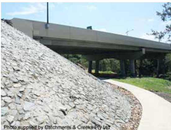
Grouted stone pitched abutment
