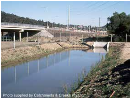
Sediment basin (Type 1 sediment trap)
