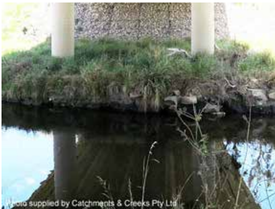
Vegetated rock stabilisation
