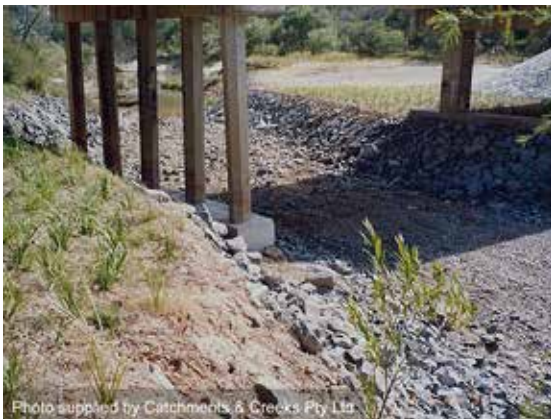
Rock stabilisation of bed and banks
