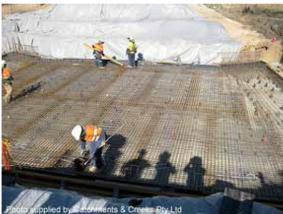
Construction of a culvert base slab
