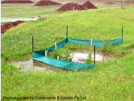
Sediment fence (Type 3 sediment trap)
