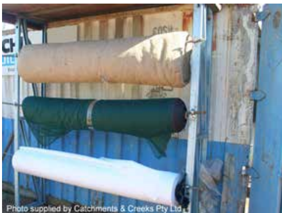
Stockpile essential ESC materials
