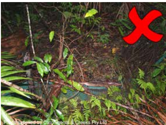
Sediment fence located in bushland
