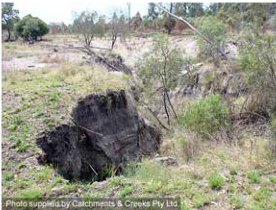
Lateral bank erosion
