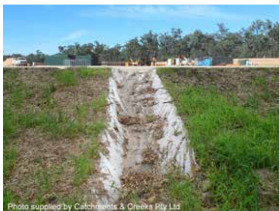
Temporary batter chute
