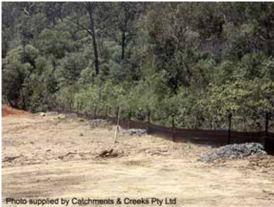
Sediment fence with rock check dams
