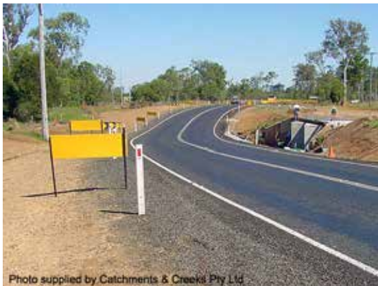
Temporary bypass road
