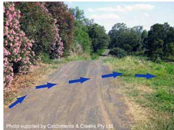
Cross bank placed at top of descent
