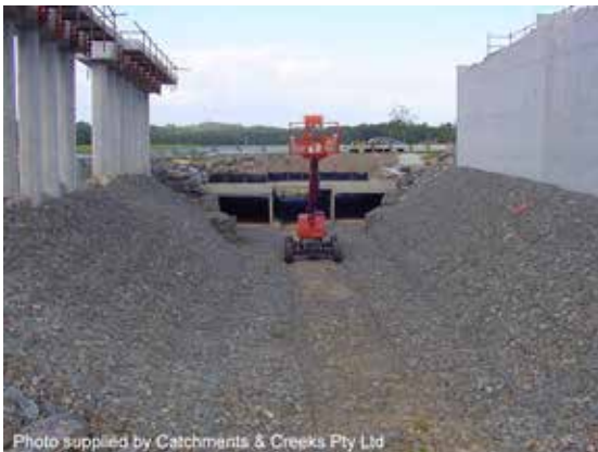
Non-vegetated rock mattresses
