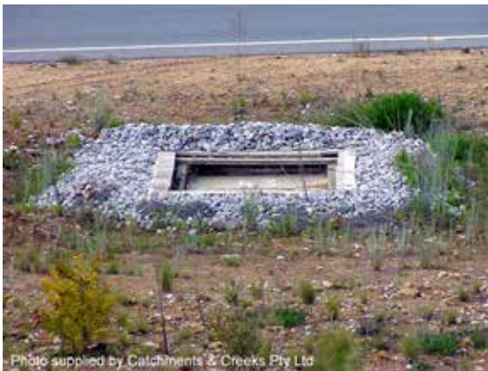
Block & aggregate drop inlet trap
