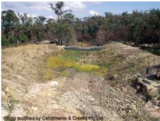
Type 2 sediment trap (1994)
