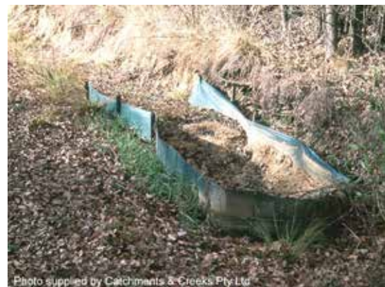
U-shaped sediment trap on steep slope
