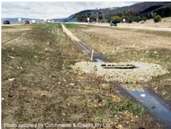
Drop inlet sediment trap
