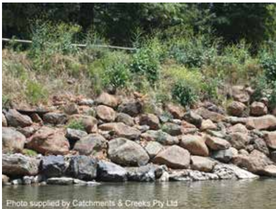
Partial vegetated bank stabilisation
