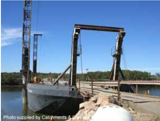
Barge crossing of tidal inlet
