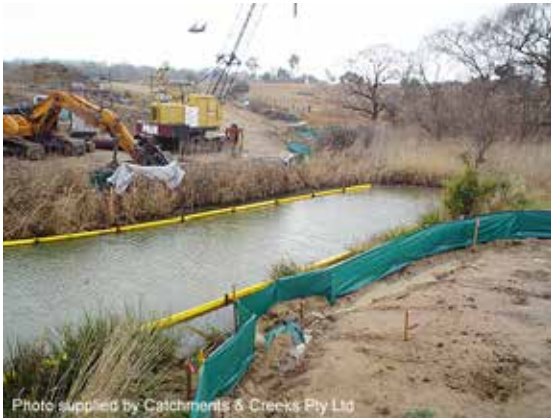
Sediment fence (Type 3 sediment trap)
