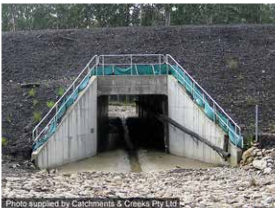
Fauna passage culverts
