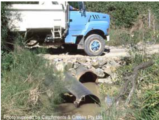
Temporary pipe culvert
