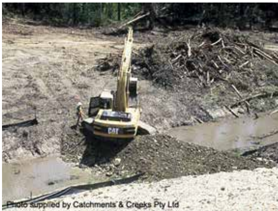
Cofferdam construction
