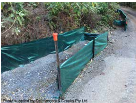
U-shaped sediment trap on mild slope
