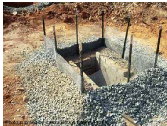
Mesh & aggregate drop inlet sediment trap
