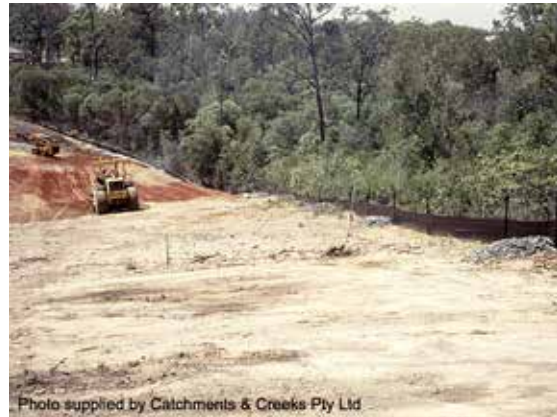
Sediment fence with rock check dams
