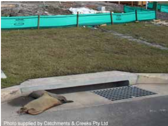
'On-grade' kerb inlet sediment trap
