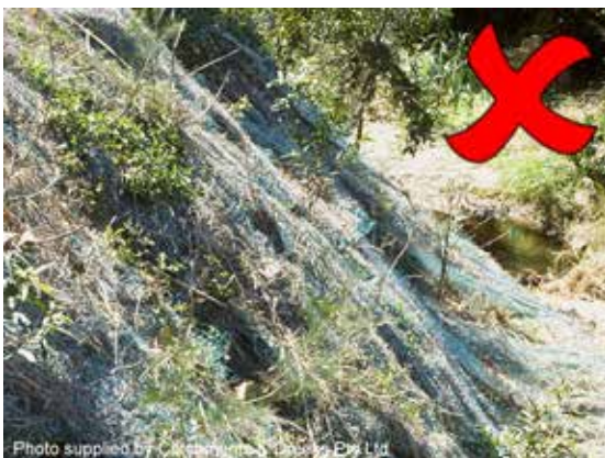
Synthetic reinforced erosion control mat
