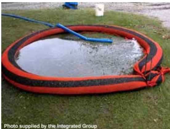
Compost-filled filter sock/berm
