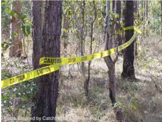
Identification of non disturbance area
