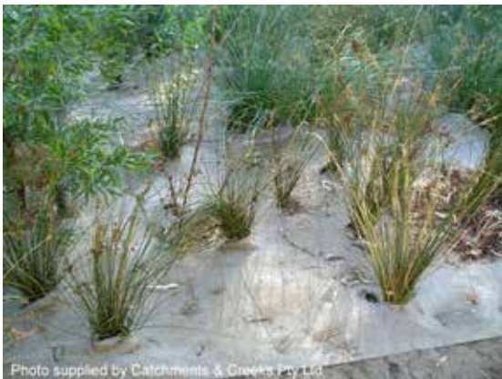
Jute erosion control blanket
