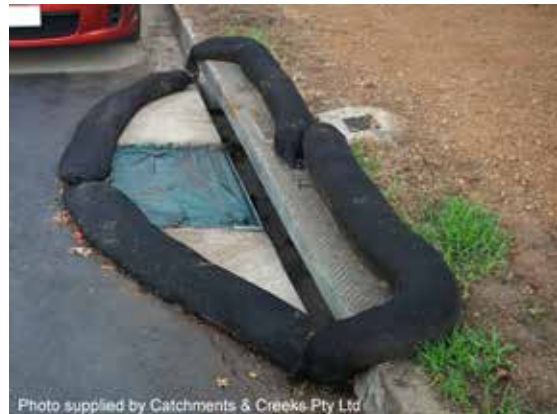
'Sag' kerb inlet sediment trap
