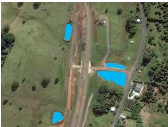
Rural road construction
