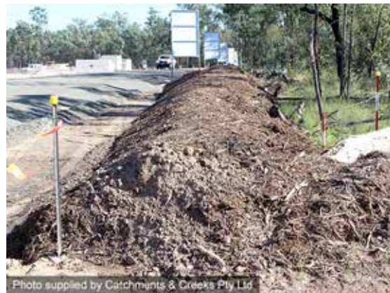
Mulch berm sediment barrier
