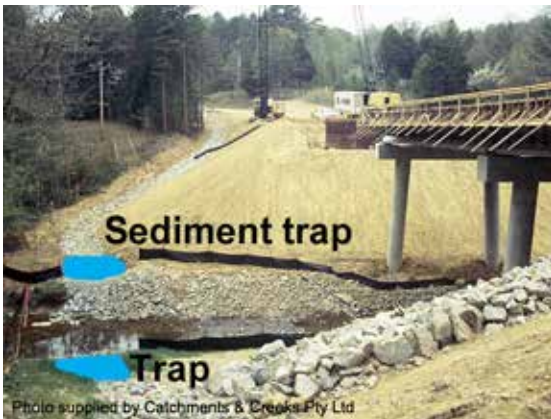
Rock filter dams (Type 2 sediment trap)
