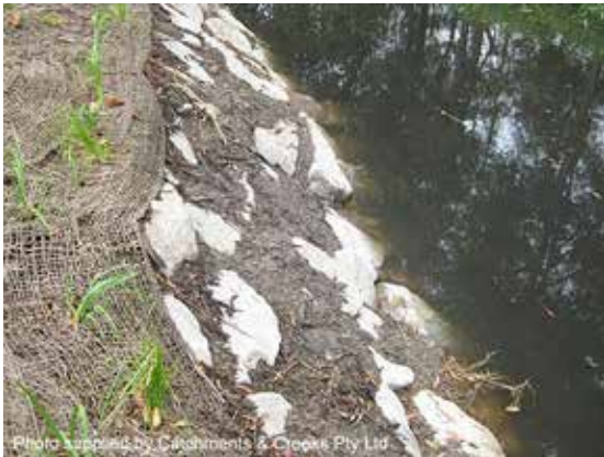
Voids filled with soil ready for planting
