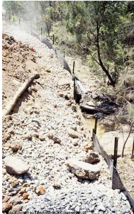
Spill-through weir & aggregate filter
