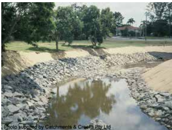
Rock stabilisation on channel bend
