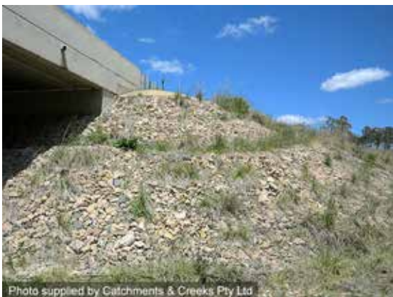
Vegetated rock mattresses
