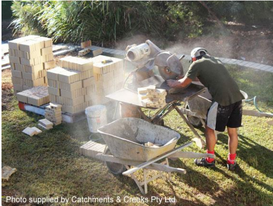
Cutting materials over grass surface
