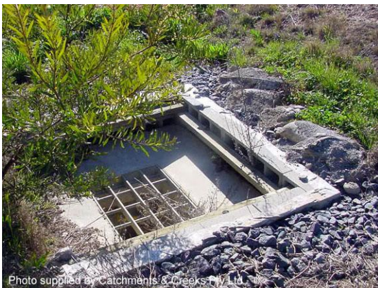
Block & aggregate drop inlet protection
