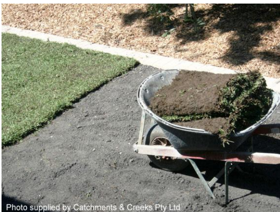
Turfing finished soil profile
