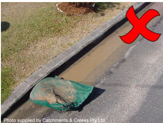
Insufficient sediment control
