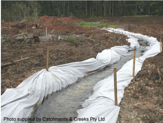
Temporary, filter cloth-lined drain
