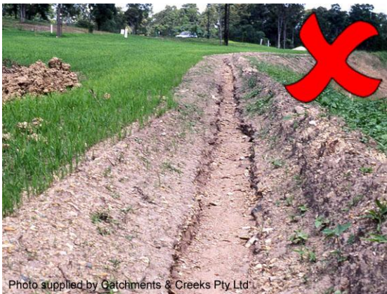
Erosion of an open soil drain
