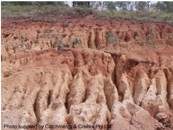
Erosion of a dispersive soil
