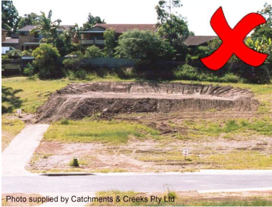
'Cut-and-fill' construction
