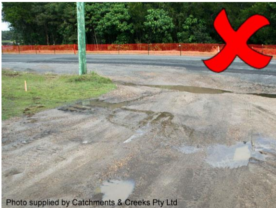
Entry/exit pad in need of maintenance
