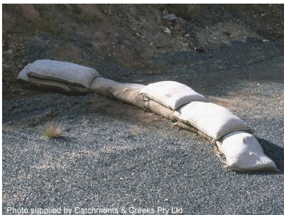
Sandbag sediment trap
