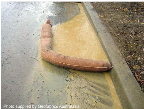
Filter sock sediment trap
