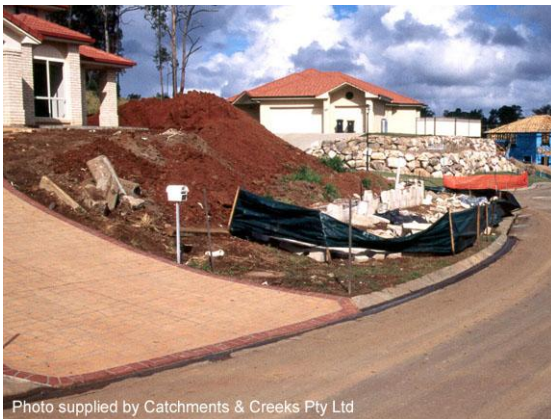
Sediment fence placed on verge
