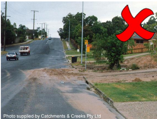
Sediment deposition on roadway
