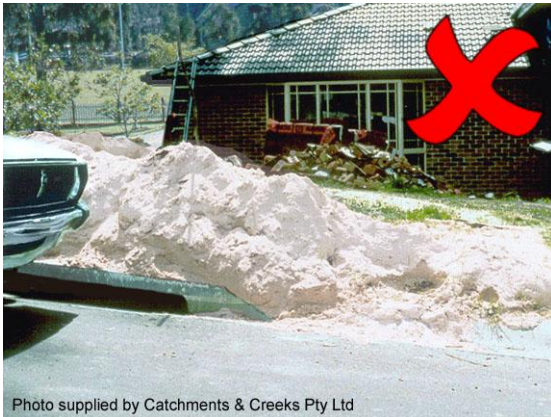
Poorly located sand stockpile
