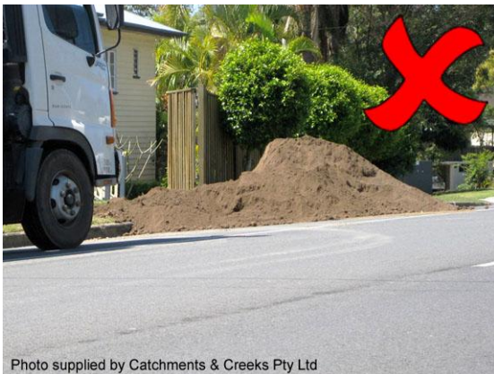
Topsoil stockpiled on roadway
