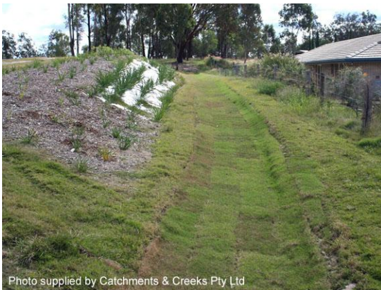
Turfed drainage channel
