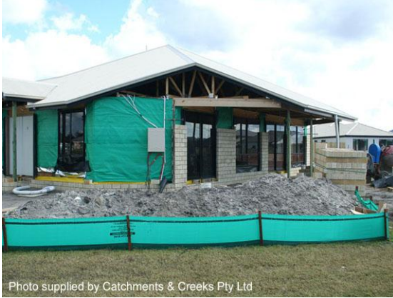
Stockpile up-slope of sediment fence
