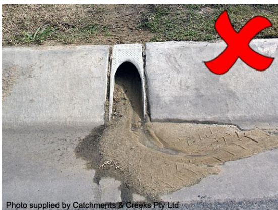
Sediment released from stormwater pipe
