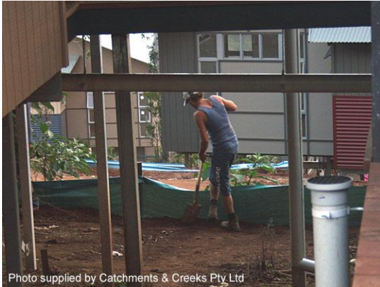
Maintenance of a sediment fence
