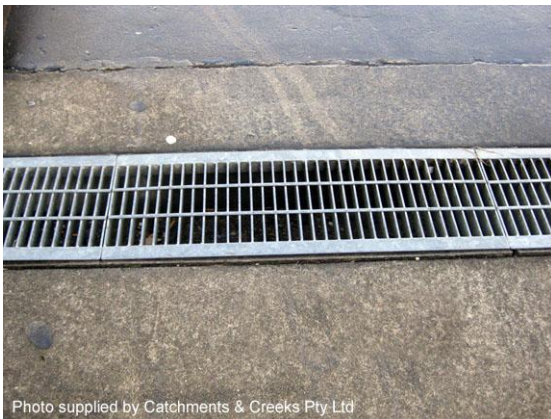
Grated stormwater inlet
