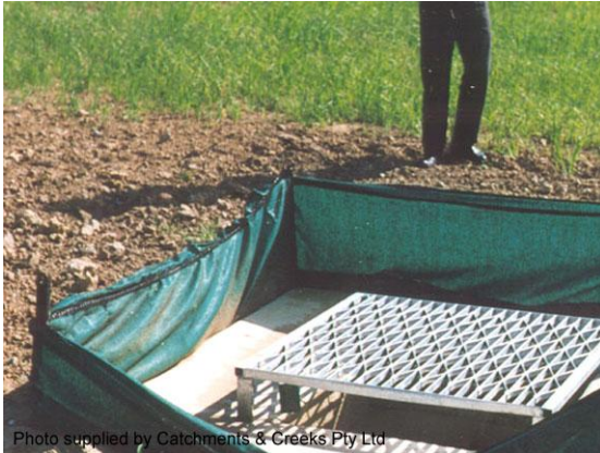
Fabric drop inlet protection
