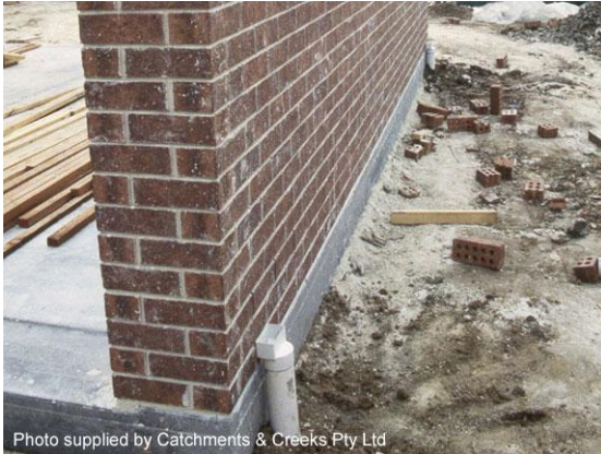
Permanent sub-surface drainage installed
