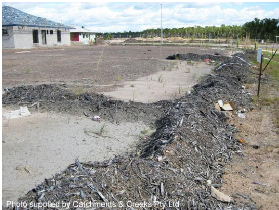
Mulch berms must be used with caution
