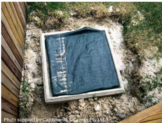
Fabric wrap inlet protection
