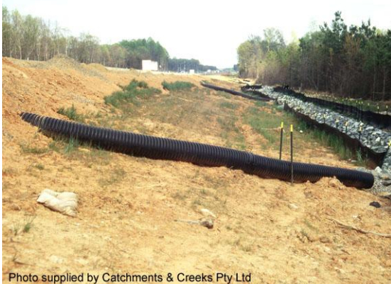
Slope drain
