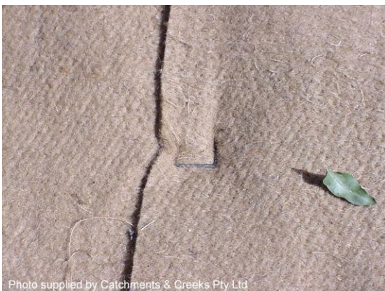
Temporary (jute) erosion control blanket
