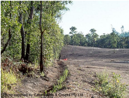
Catch drain formed up-slope of work site
