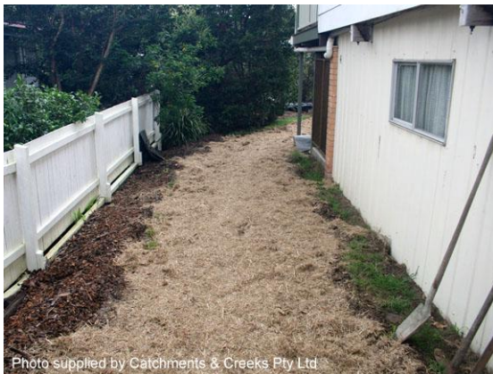
Mulching of disturbed site access pathway
