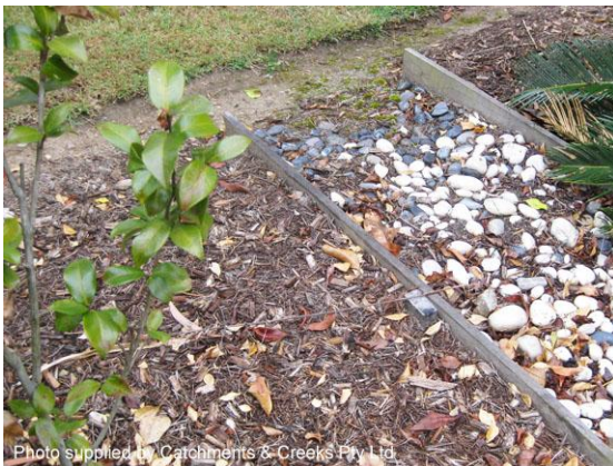
Rock mulched drain through garden bed
