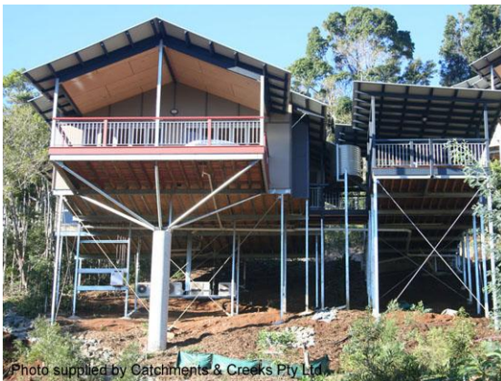
Pole home being built on a steep site
