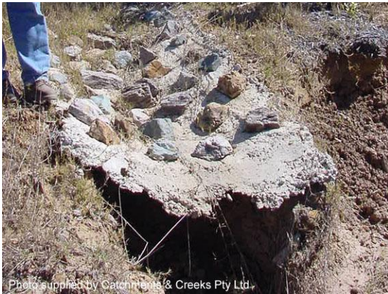
Tunnel erosion under concrete drain
