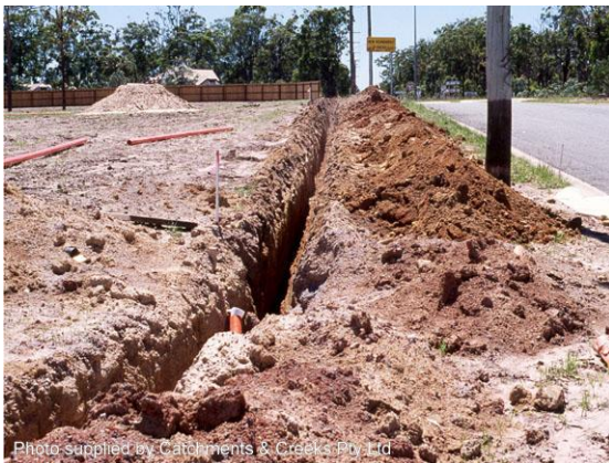
Excavated service trench
