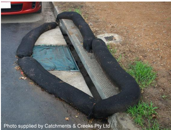
Sag inlet sediment trap
