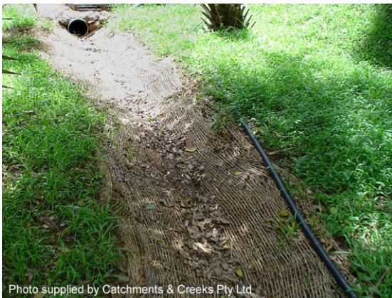
Stormwater drain lined with jute mesh
