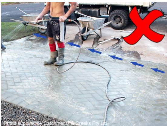
Cement wash flowing to kerb
