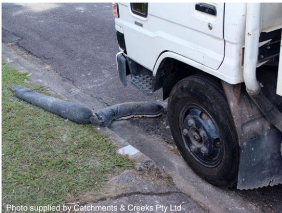
Silt socks placed in kerb
