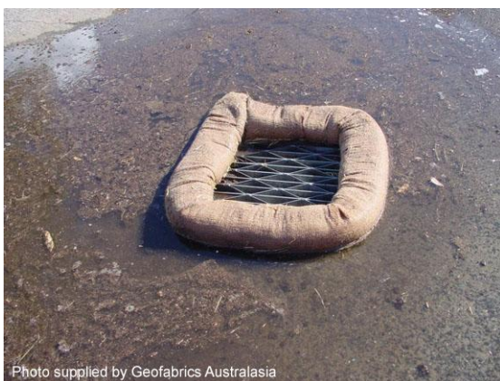
Filter sock drop inlet protection
