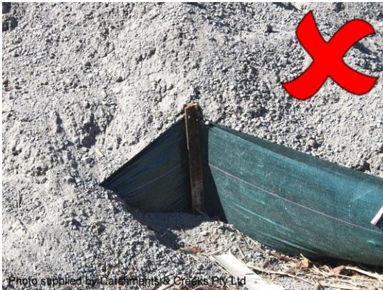
Earth spilling over a sediment fence
