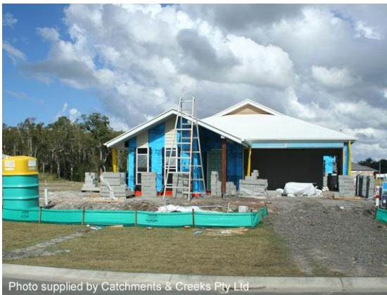
Sediment control measures
