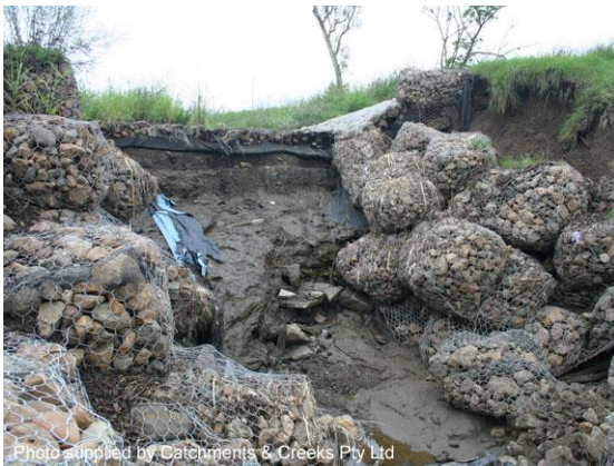
Failed gabion overflow spillway
