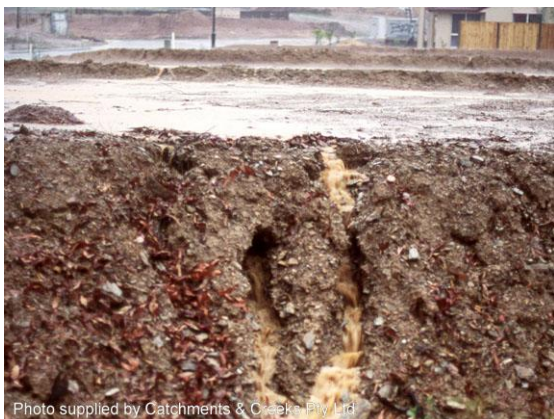
Clayey soil building pad
