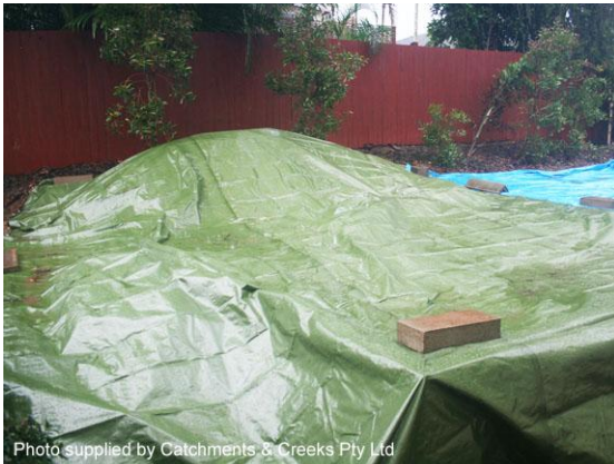
Stockpile covered during wet weather
