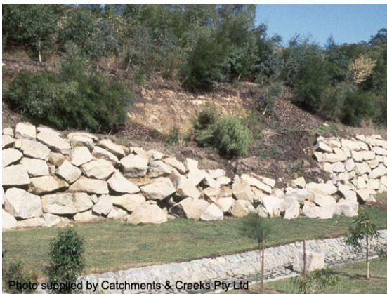
Failed rock retaining wall
