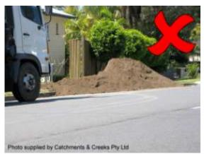
Topsoil stockpiled on roadway
