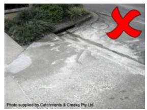
Cement wash-off from concreting works
