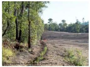
Catch drain formed up-slope of work site
