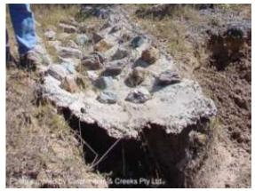
Tunnel erosion under concrete drain
