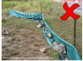
Toe of fabric incorrectly anchored
