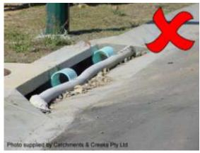
Inappropriate on-grade sediment trap
