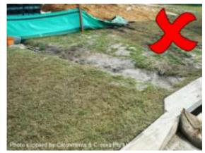
Poorly backfilled service trench
