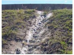
Geotextile-lined drainage chute
