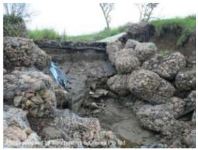
Failed gabion overflow spillway
