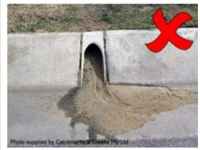
Sediment released from stormwater pipe
