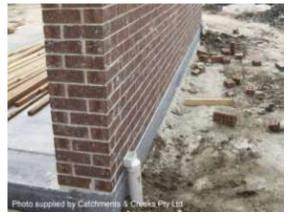
Permanent sub-surface drainage installed
