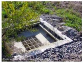
Block & aggregate drop inlet protection
