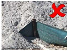
Earth spilling over a sediment fence
