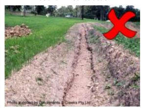
Erosion of an open soil drain
