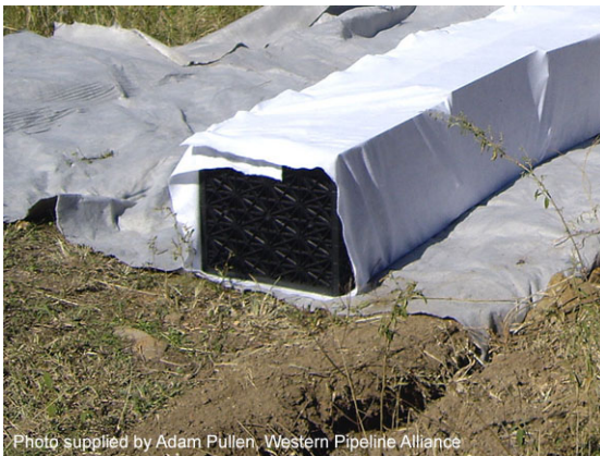
Modular sediment trap being installed
