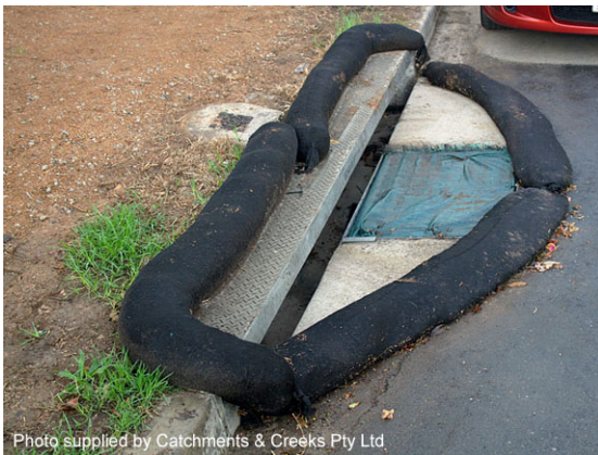
Sag inlet sediment trap
