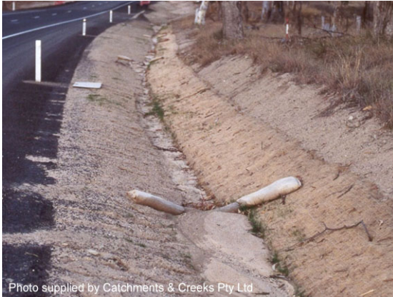
Check dam sediment trap
