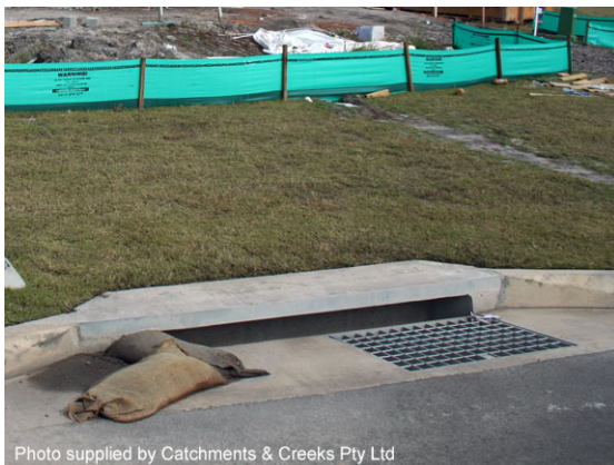
On-grade kerb inlet sediment trap
