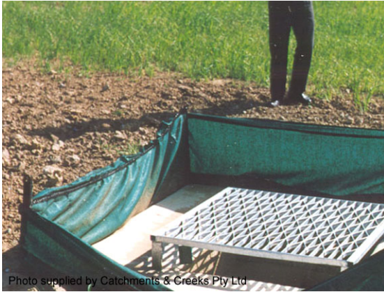
Fabric drop inlet protection
