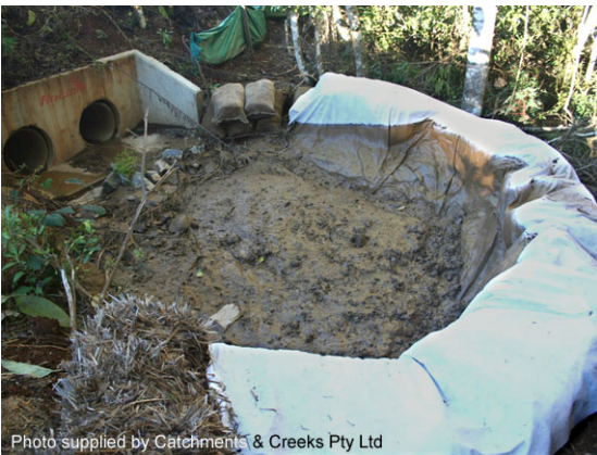
Straw bale barrier
