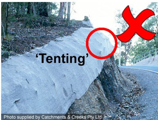
Blanket stretched over rough ground
