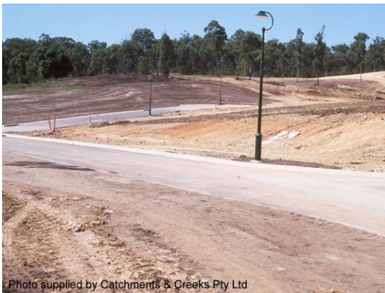
Replacement of topsoil
