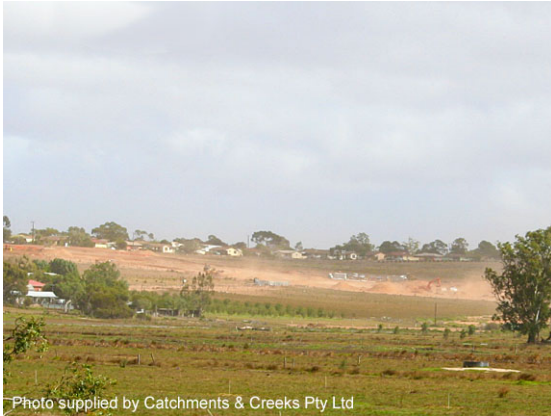
Dust generated on a construction site
