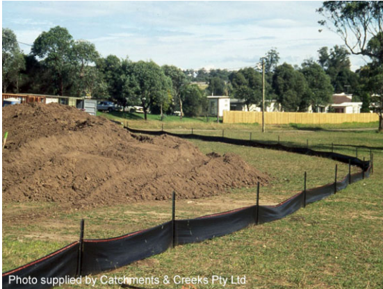
Stockpiling of topsoil
