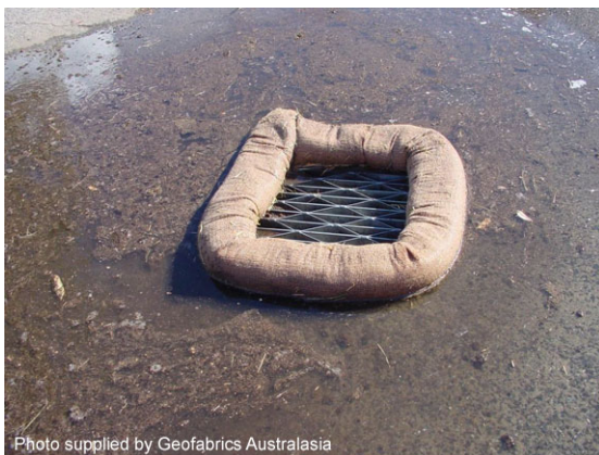
Filter sock drop inlet protection
