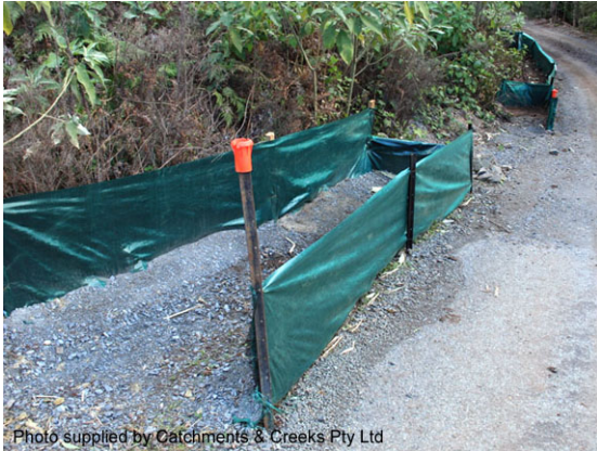
U-shaped sediment trap
