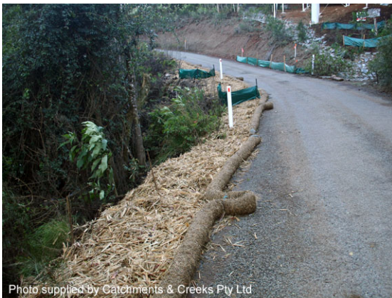
Fibre roll sediment trap
