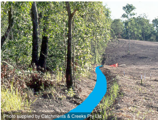
Flow diversion using a catch drain
