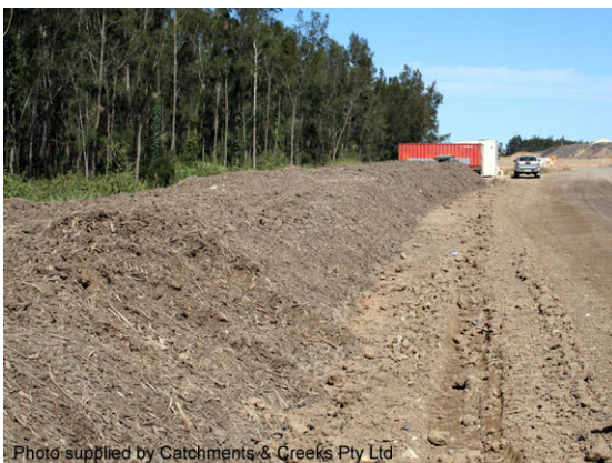
Mulch berm sediment control measure
