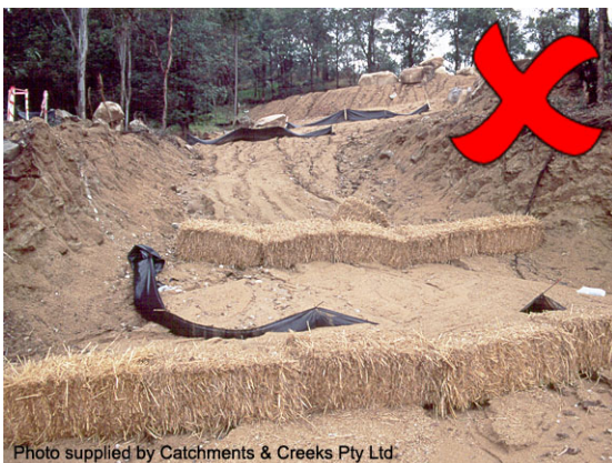
Failed sediment traps on steep ramp
