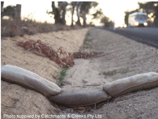
Sandbag check dam
