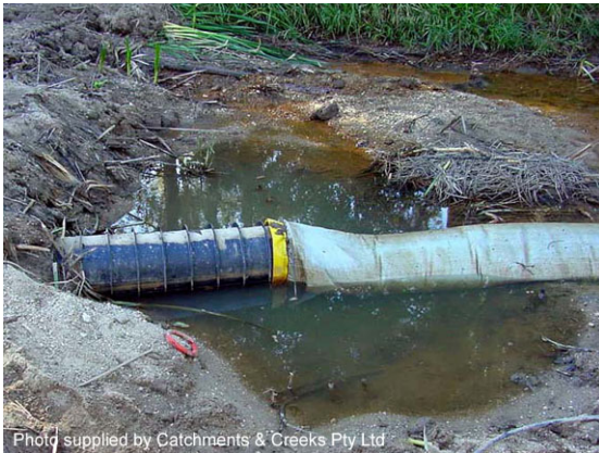
Filter tube attached to an embankment
