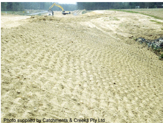
Roughened earth batter
