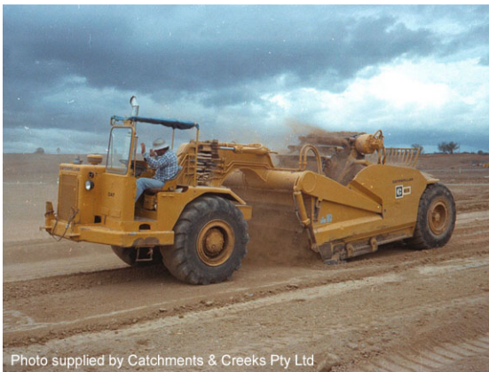
Scraper stripping soil
