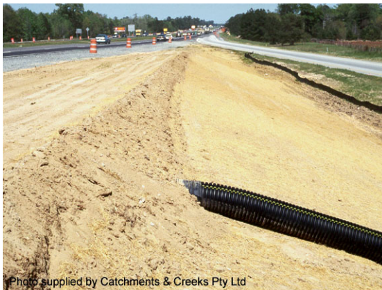
Flow diversion bank controlling flow entry
