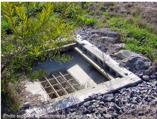
Block & aggregate drop inlet protection
