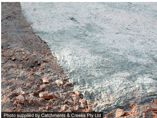
Thick blanket seeded with BFM
