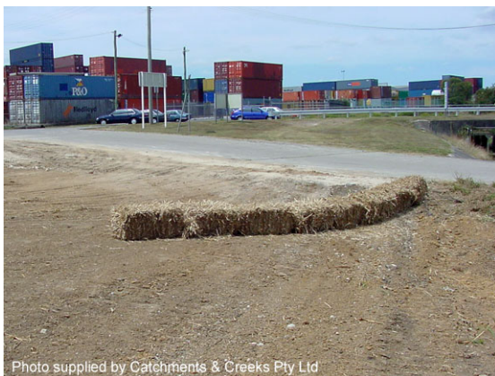
Straw bale flow diversion bank under construction (yet to be staked)
