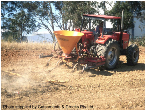
Seeding road batter
