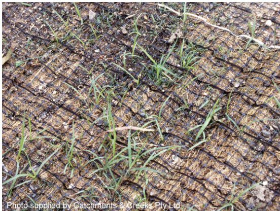
Turf reinforcement mat
