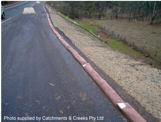
Sandbag flow control berm
