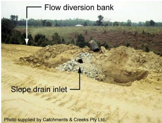
Sediment traps each side of pipe inlet
