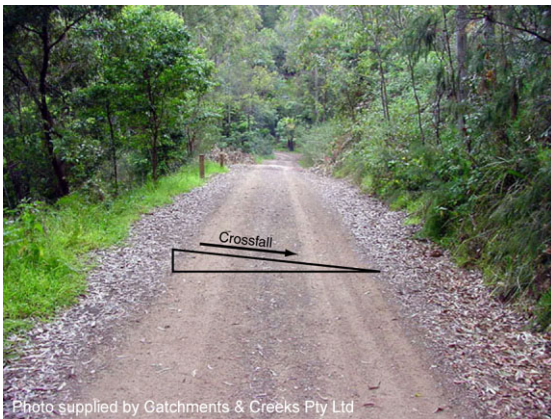
Dirt road with in-fall drainage
