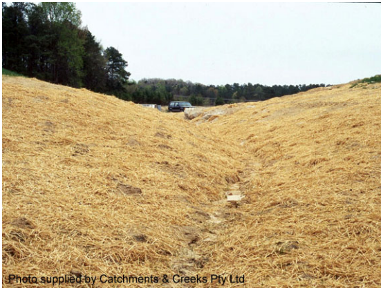
Soil stabilisation with stabilised mulch
