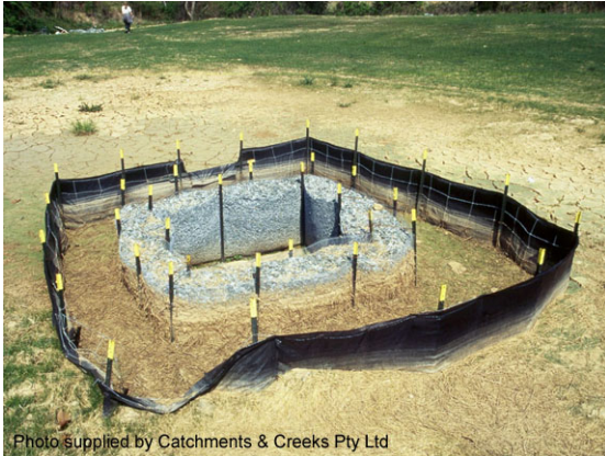
Sediment weir (field inlet protection)
