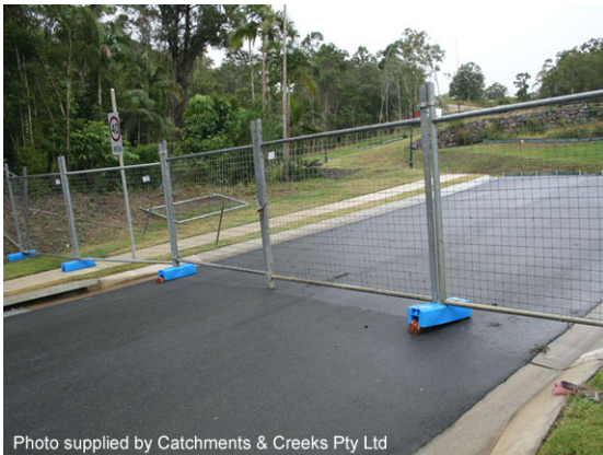
Temporary site fencing
