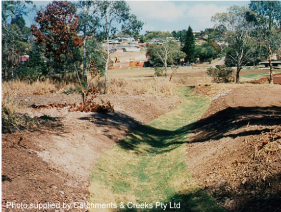
Turf lined diversion drain
