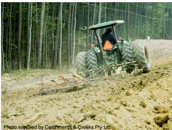
Scarifying the soil surface
