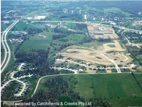
Staged land clearing
