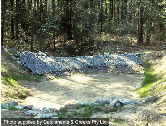
Rock filter dam - aggregate filter
