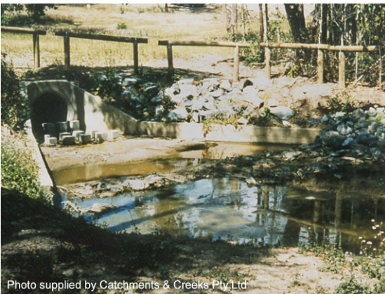
Excavated sediment trap
