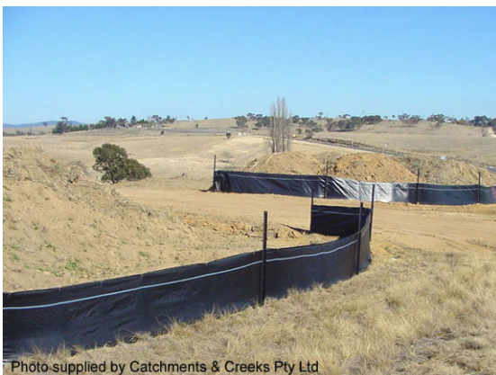
Sediment control down-slope of stockpile
