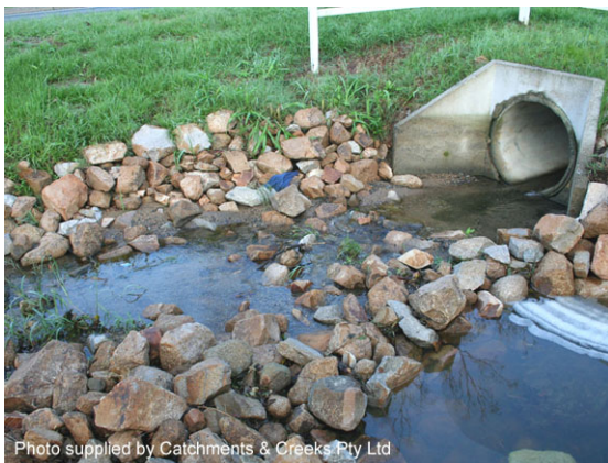
Rock pad outlet structure
