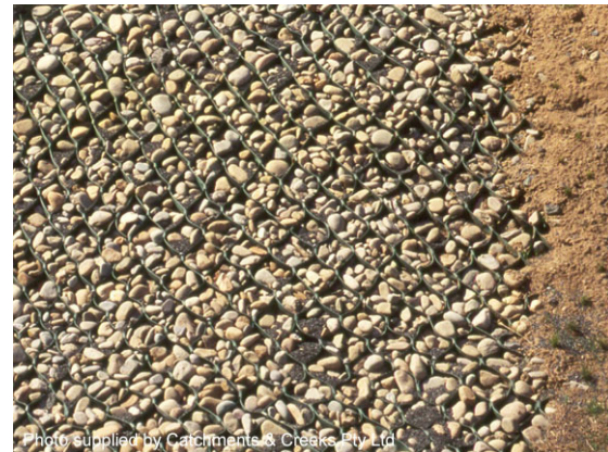
Gravelled batter slope
