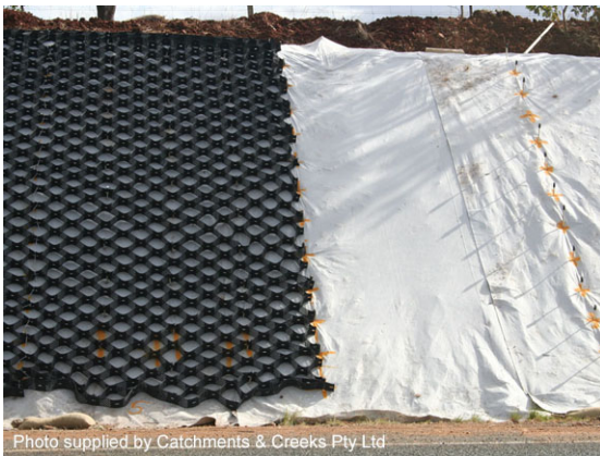
Installation on road batter
