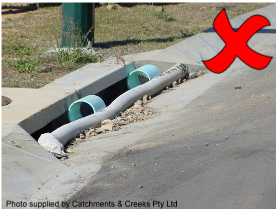
Inappropriate on-grade sediment trap
