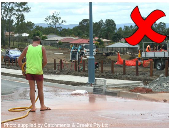
Hosing down road surface
