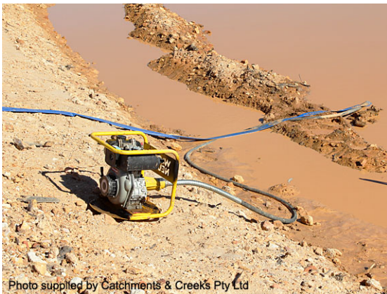
De-watering of sediment basin
