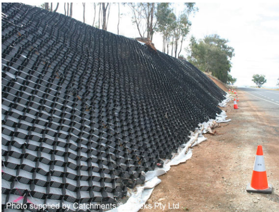
Installation on road batter
