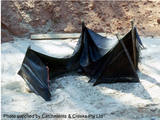
Damage to a drop-inlet sediment trap
