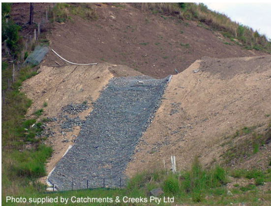
Rock mattress lined spillway chute
