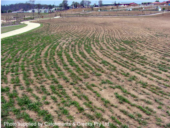
Application of a temporary grasses
