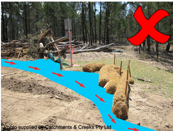
Stormwater runoff bypasses sediment trap
