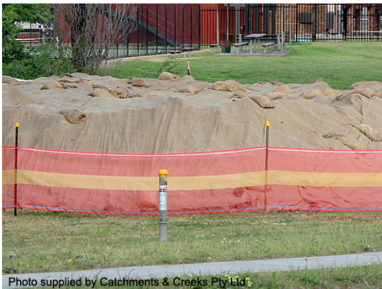
Long-term stockpile covered with jute
