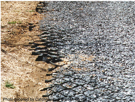
Gravelled car park
