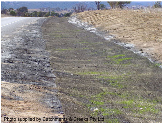
Jute mesh with bitumen seal
