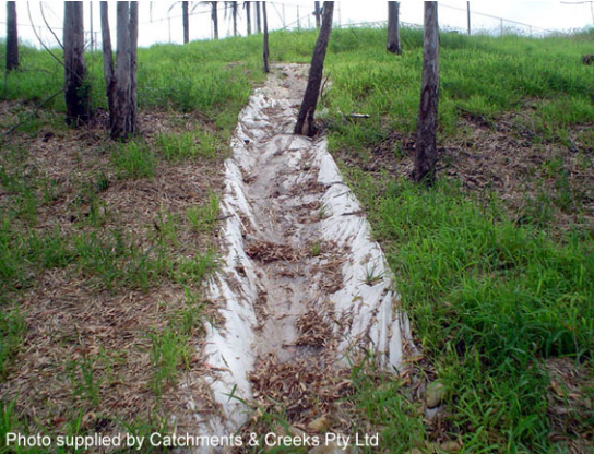
Geotextile lined drainage chute
