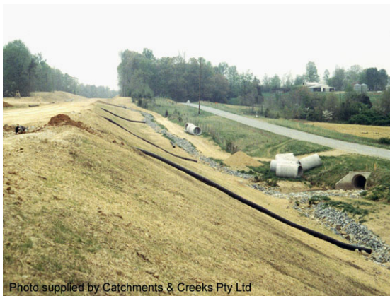
Slope drains on newly seeded batter
