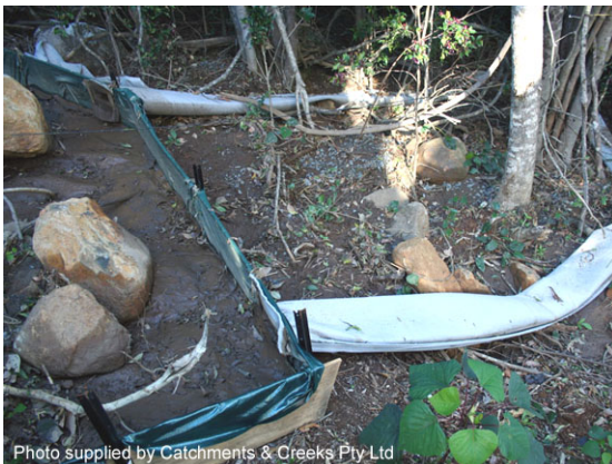
Filter tube dam sediment trap
