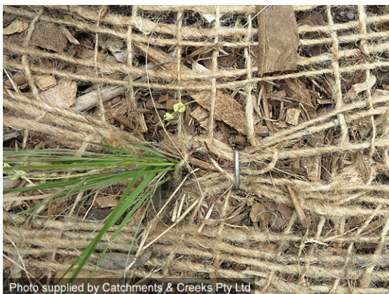
Jute mesh anchoring loose mulch
