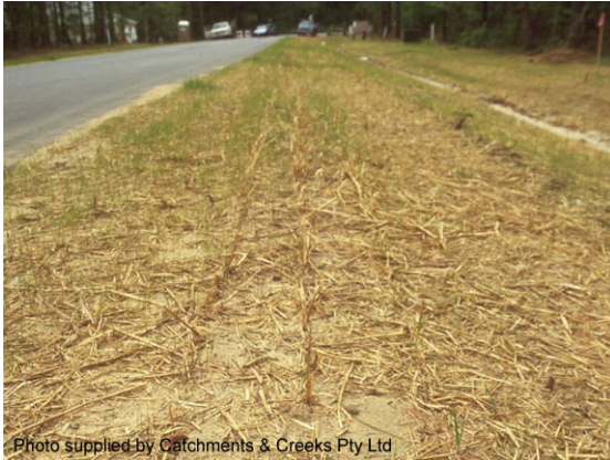
Straw mulching of road shoulder
