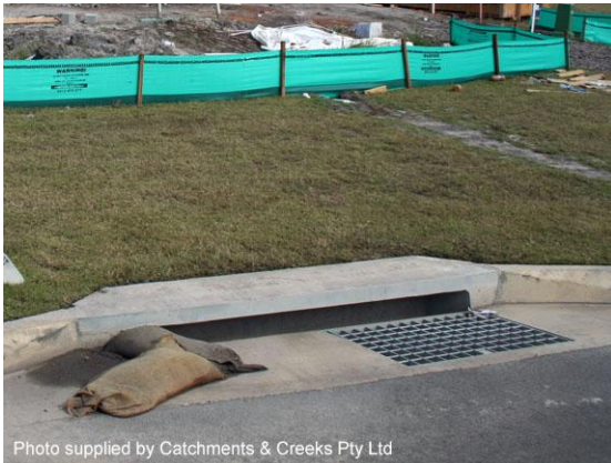
On-grade kerb inlet sediment trap
