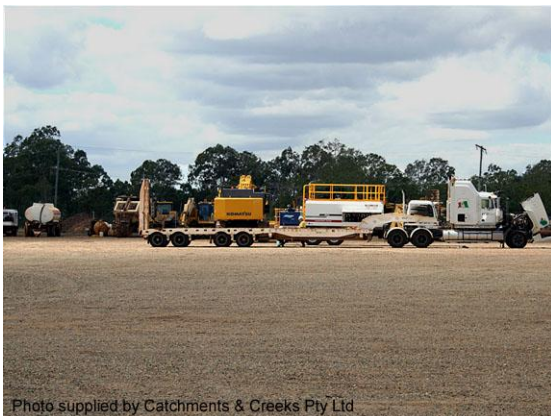
Gravelled work compound
