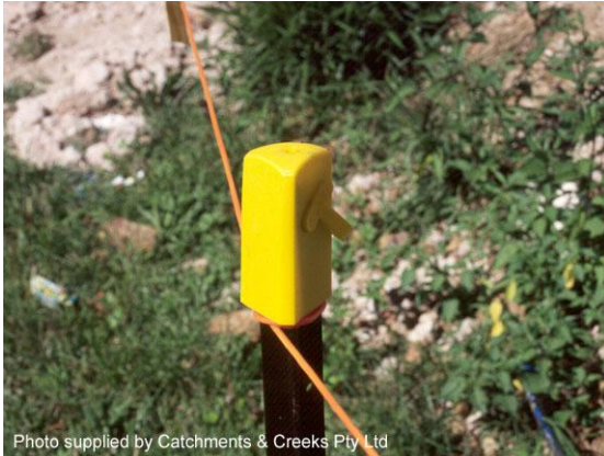
Safety cap on sediment fence stake
