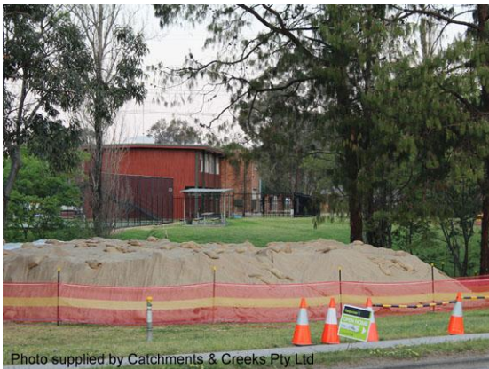
Stockpile covered with jute blankets
