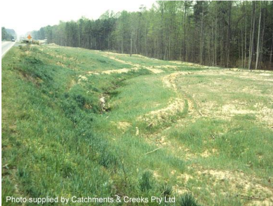
Temporary grassing of road works
