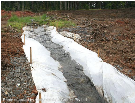
Diversion of "clean" run-on water
