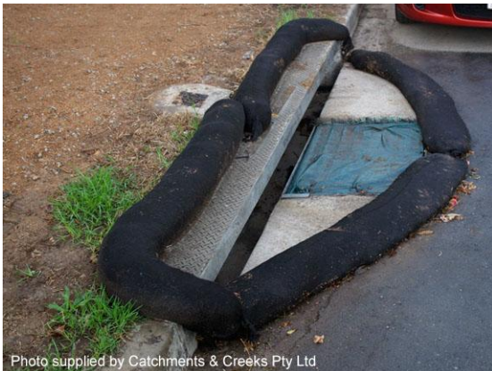
Sag-type kerb inlet protection
