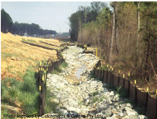
Protection of permanent storm drain
