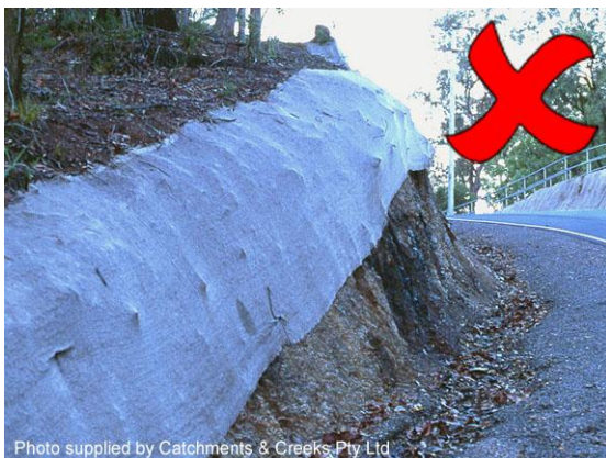
Poorly applied blanket
