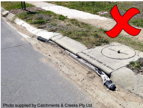
Sediment trap blocking inflows
