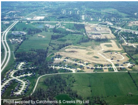
Staged land clearing
