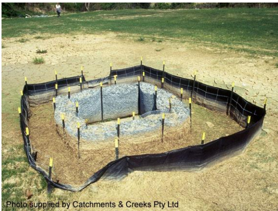
Sediment weir field inlet control
