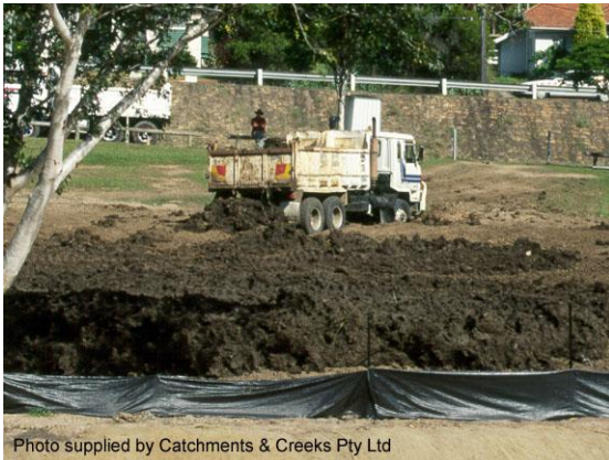
Soil being worked when it is too wet
