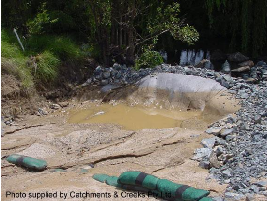
Rock filter dam with geotextile filter
