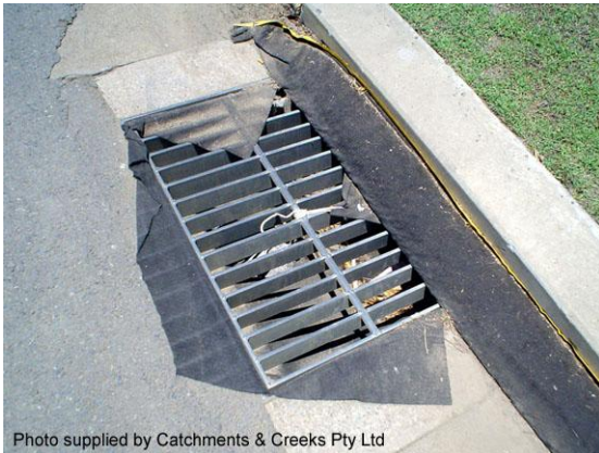
Gully bag sediment trap
