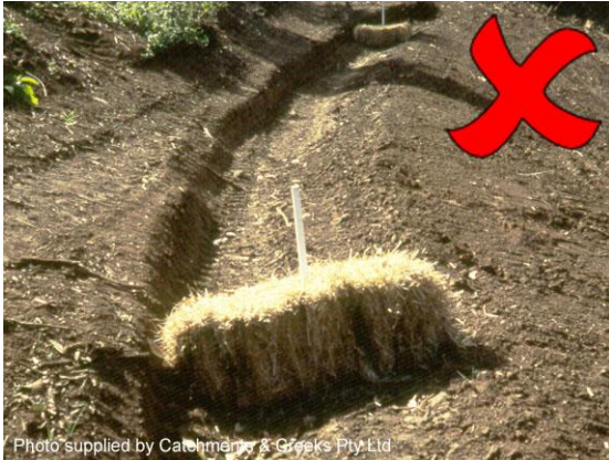
Bales should not be used to slow the flow
