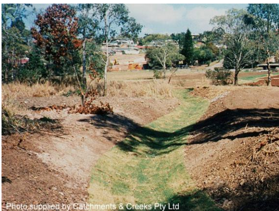
Early establishment of a diversion drain
