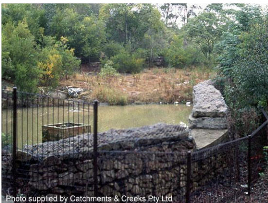
Wetland formed from sediment basin
