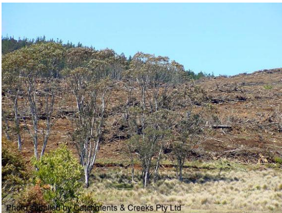
Tree clearing with minimal soil disturbance
