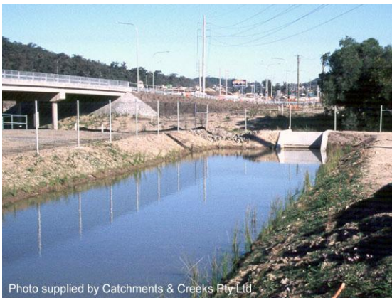
“Wet” type sediment basin
