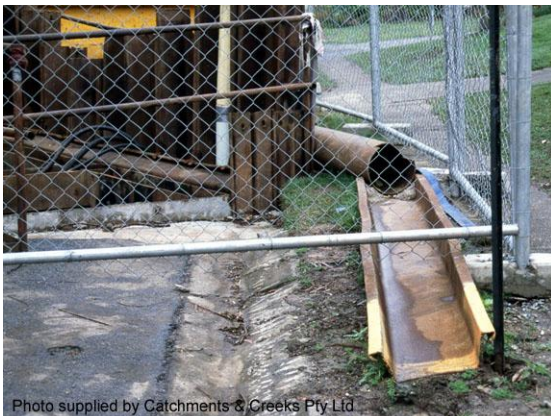
Stormwater diverted around a pit
