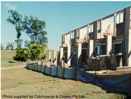
Sediment fence adjacent a building site
