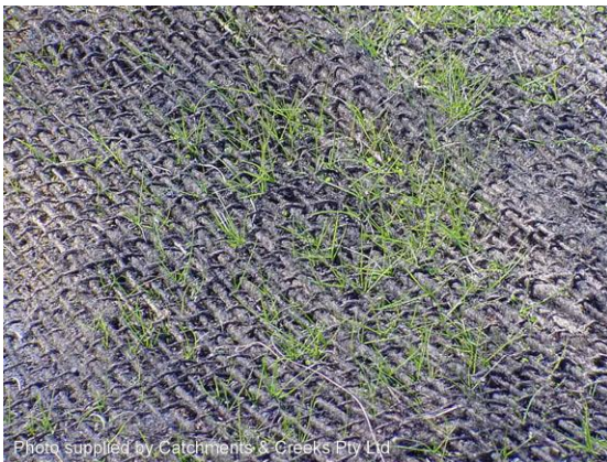
New grass growth through a jute mesh
