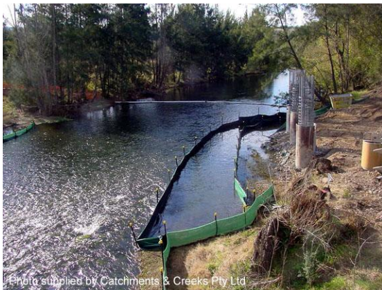
Sediment fence isolation barrier
