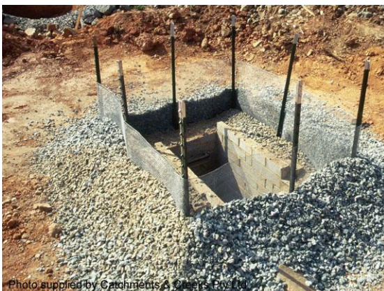
Mesh and aggregate drop inlet protection
