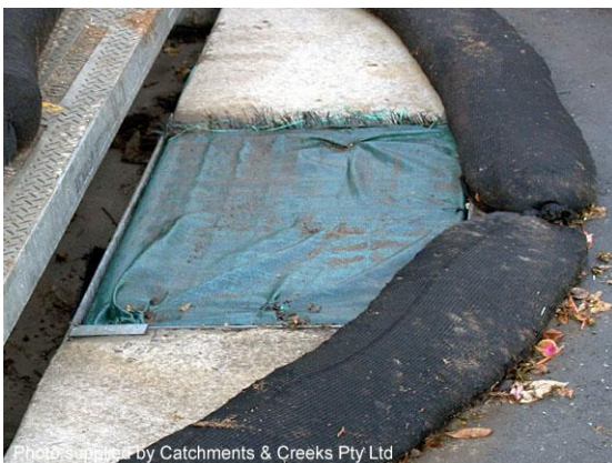
Inappropriate use of fabrics
