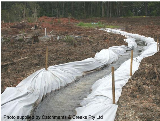
Temporary drain lined with filter cloth
