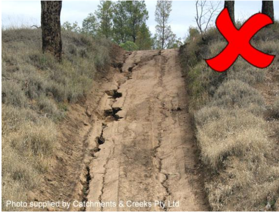
Drainage damage to an access road
