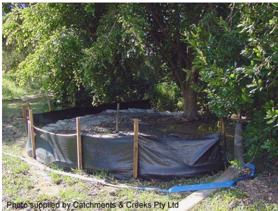
Off-stream filter pond
