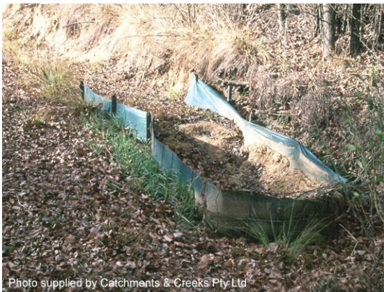
U-shaped sediment trap
