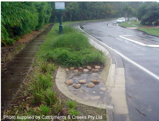
Roadside bio-filtration cell
