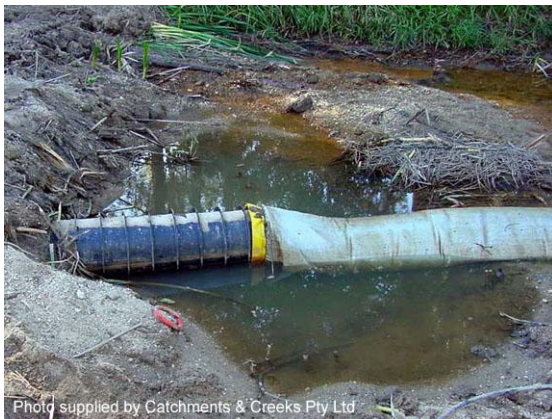
Filter tube dam
