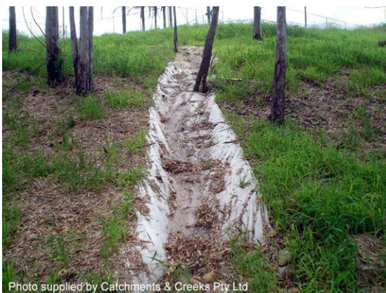
Batter chute lined with filter cloth
