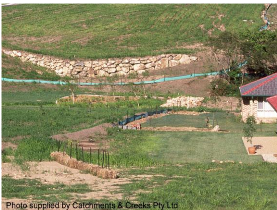
Straw bales diverting stormwater runoff
