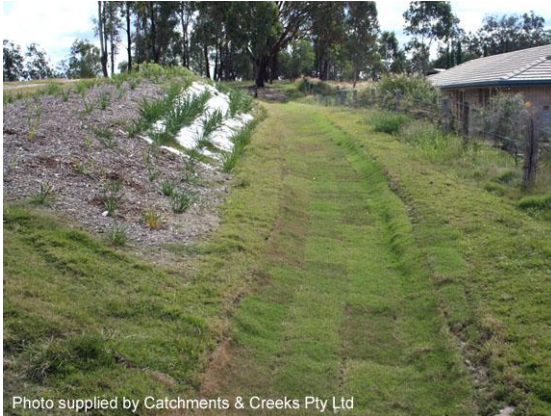
Wide, shallow, grass-lined drain
