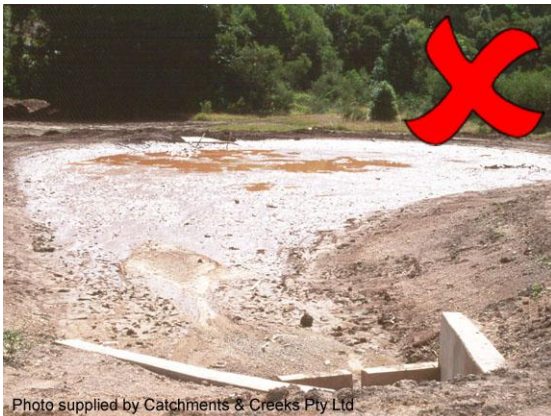
Undersized sediment basin
