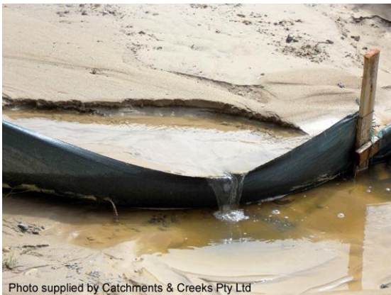
Sediment fence with settled sediment
