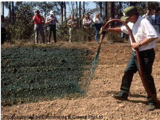
Demonstration of hydro-seeding
