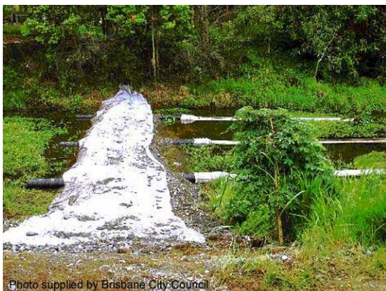
In-stream rock filter dam with filter tubes
