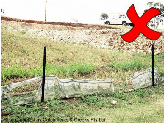
Sediment fence well past its 'use-by' date
