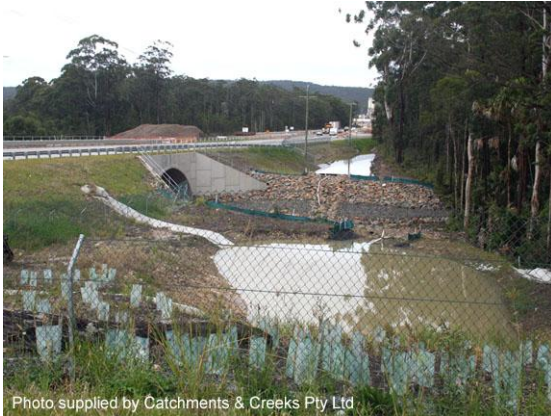
Post-construction sediment basins
