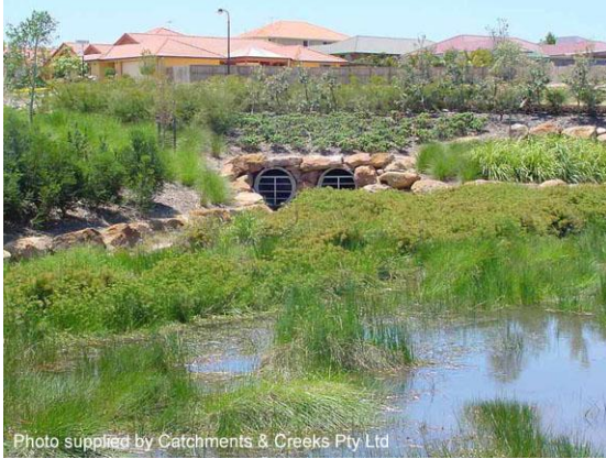
Urban stormwater treatment wetland
