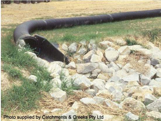
Diversion drain outlet structure
