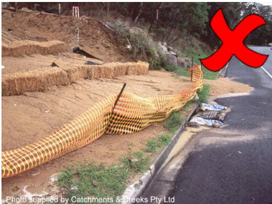
Failed sediment control measures
