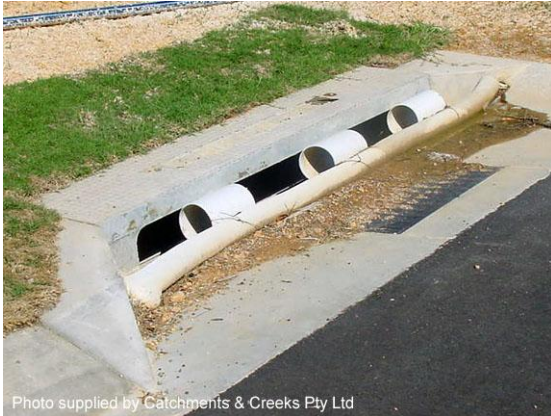
Sag inlet sediment trap
