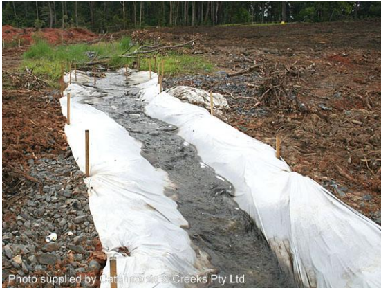
Control of “clean” run-on water
