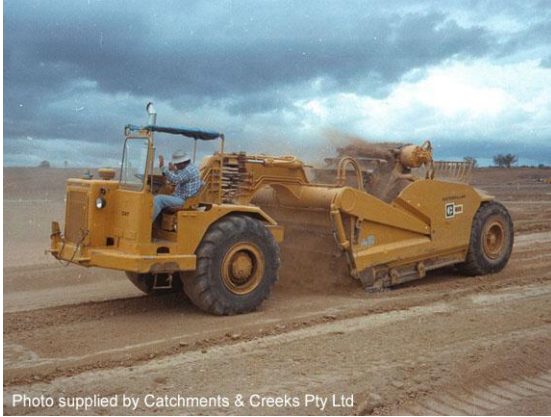
Scraper stripping soil
