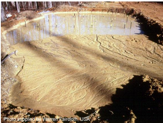
Sediment retained in a basin
