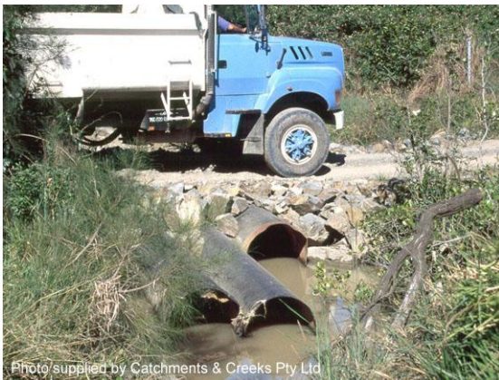
Temporary culvert crossing
