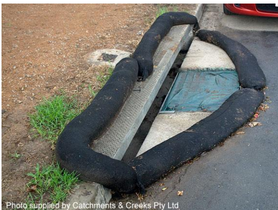
Sag inlet sediment trap
