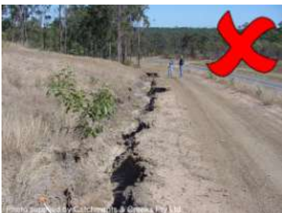
Batter drain cut into a dispersive soil
