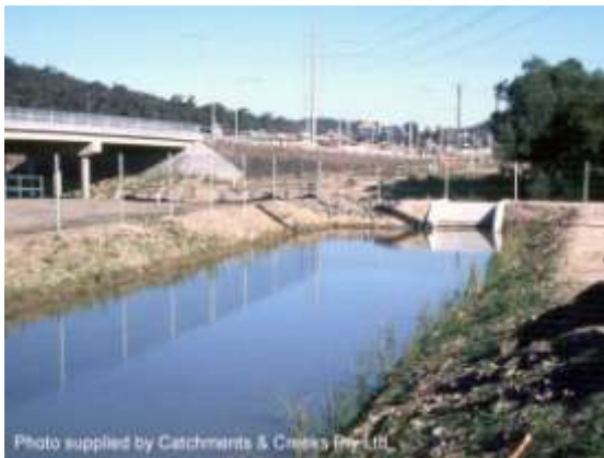
Photo supplied by Catchments & Creeks Pty Ltd “Wet” type sediment basin
