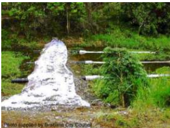
Instream rock filter dam with filter tubes
