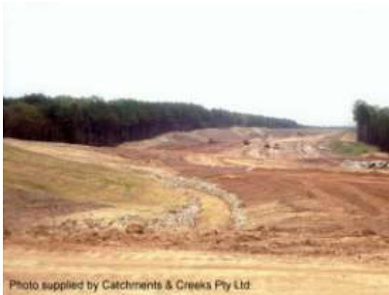
Prompt revegetation of road batters
