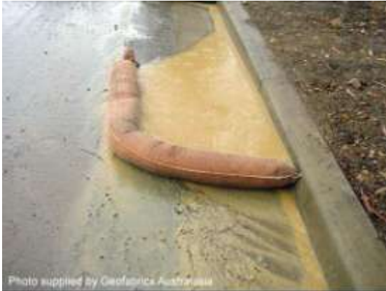
Sand-filled filter sock
