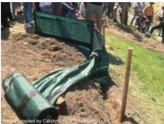
Installation of a sediment fence
