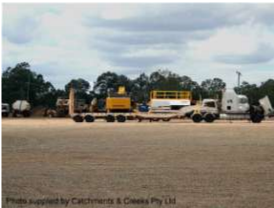
Gravelled work compound
