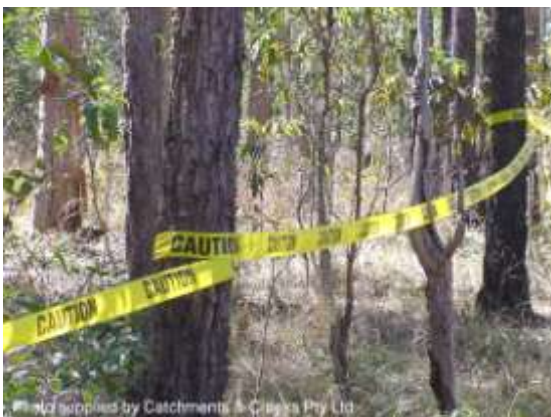
Marking the limits of clearing
