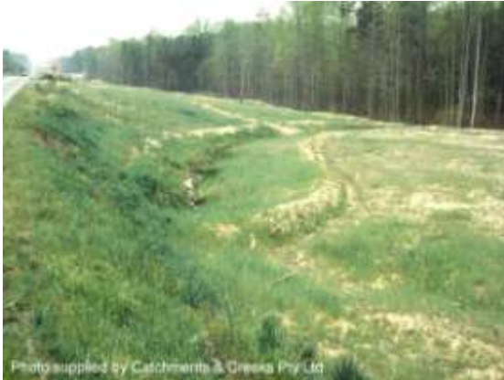
Temporary grassing of road works
