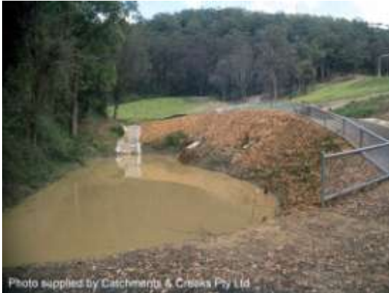
Basin with limited maintenance access
