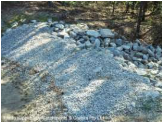
Rock filter dam with aggregate filter
