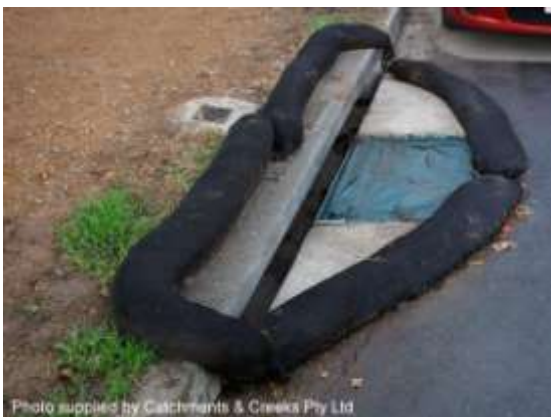
Sag-type kerb inlet protection
