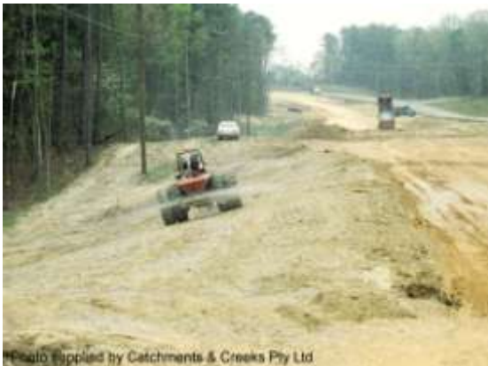
Slope being prepared for revegetation
