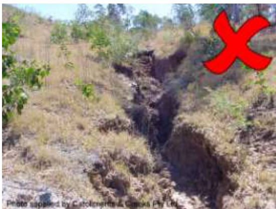
Failed drain in a dispersive soil
