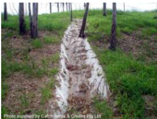
Batter chute lined with filter cloth
