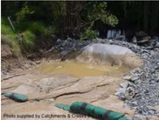
Photo supplied by Catchments & Creeks Pty Ltd Rock filter dam with geotextile filter
