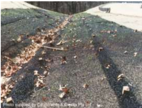
Turf reinforcement mat
