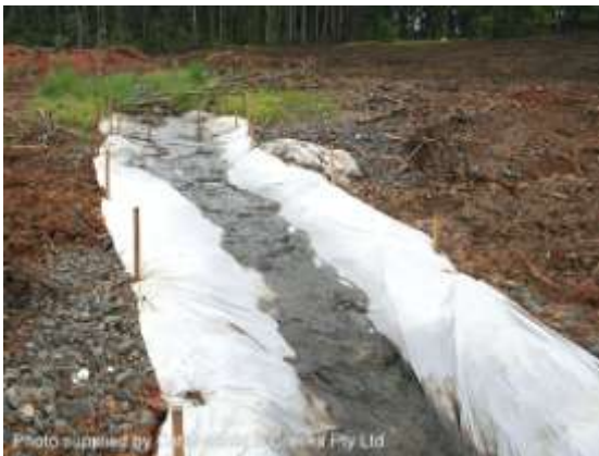
Diversion of "clean" run-on water
