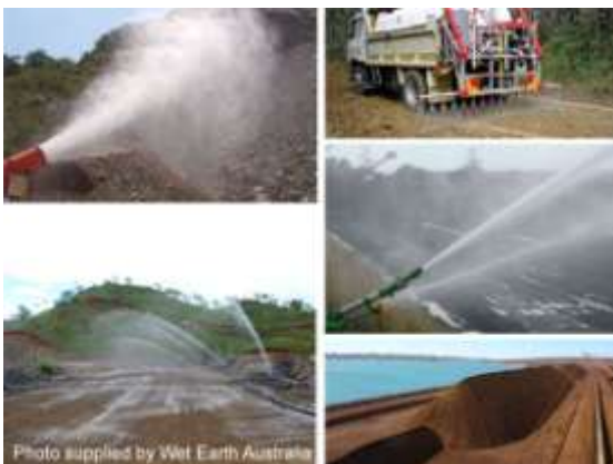
Use of dust control soil binders
