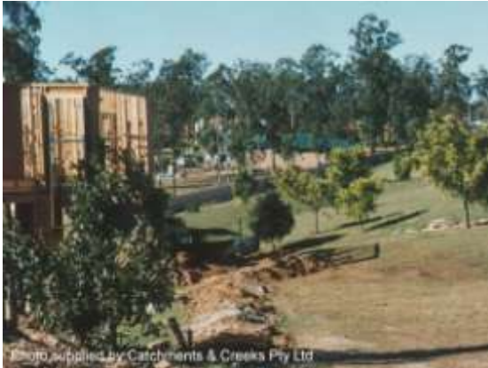
Flow diversion bank
