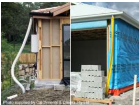
Temporary downpipes
