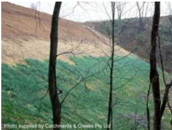
Staged exposure and rehabilitation
