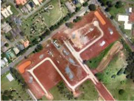
Construction site with sediment basins
