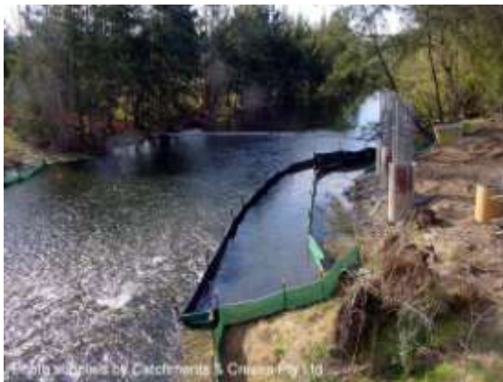
Sediment fence isolation barrier
