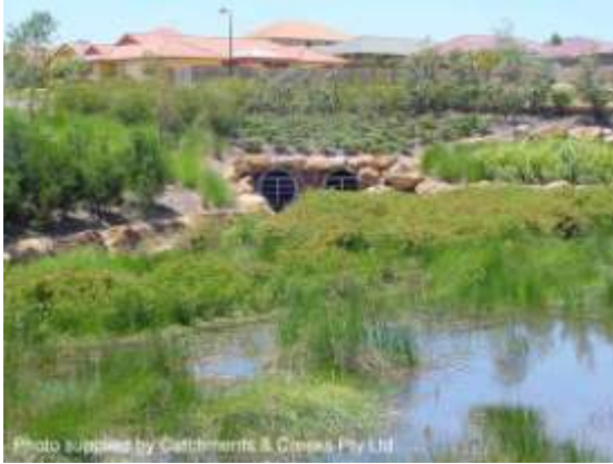
Urban stormwater treatment wetland
