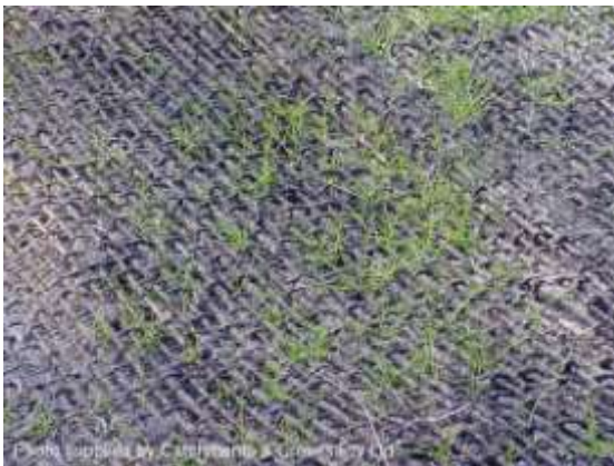
New grass growth through a jute mesh
