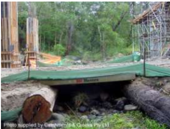
Temporary bridge crossing
