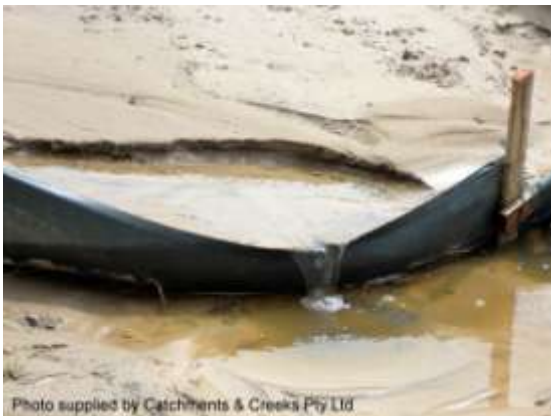
Sediment fence with settled sediment
