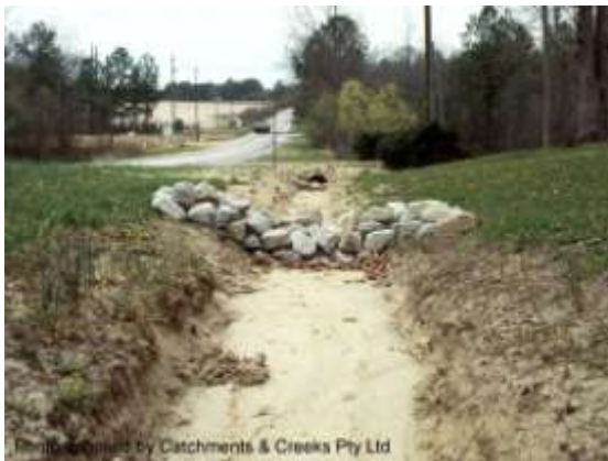
Rock check dam
