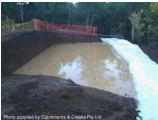
Basin full and ready to overflow
