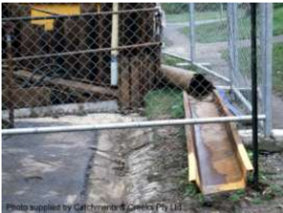
Stormwater diverted around a pit
