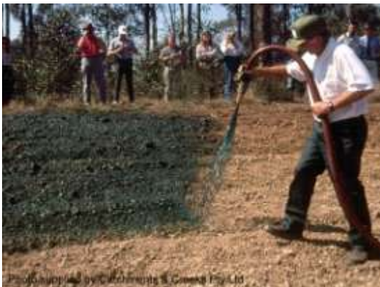
Demonstration of hydro-seeding
