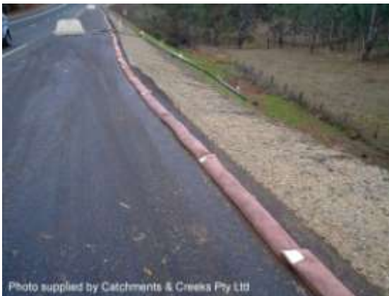
Temporary flow diversion system
