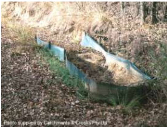
U-shaped sediment trap
