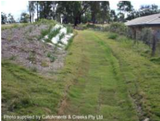
Wide, shallow, grass-lined drain
