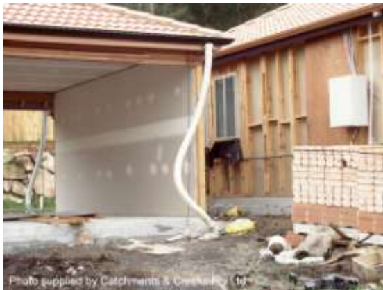
Temporary roof water connection
