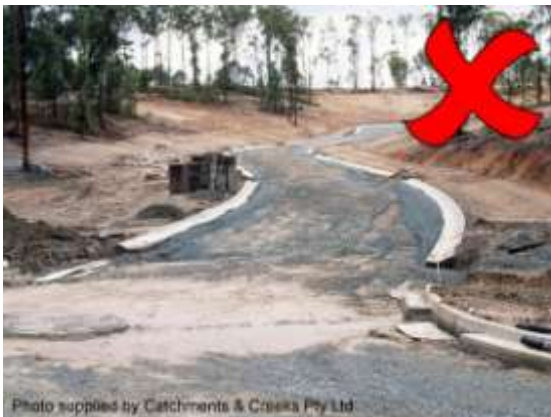
Site with limited drainage & erosion control
