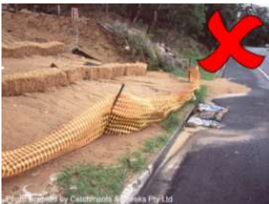
Failed sediment control measures
