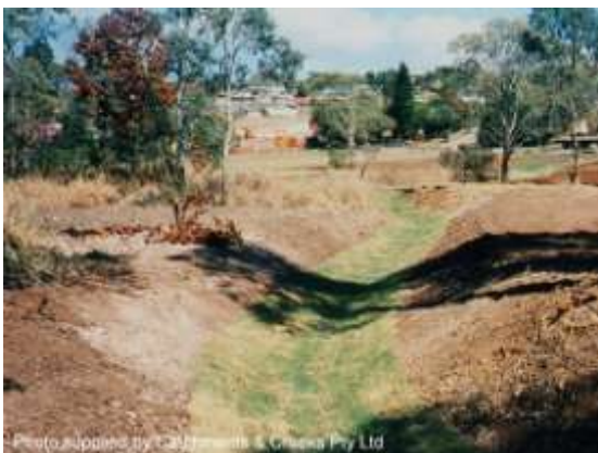
Early establishment of a diversion drain
