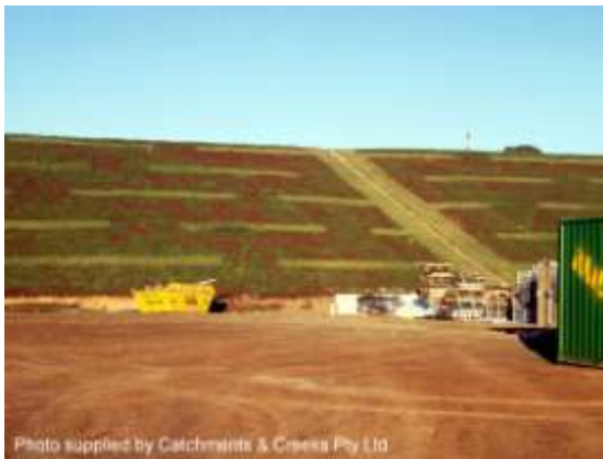
Turf filter strips on steep slope
