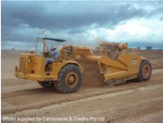
Scraper stripping soil
