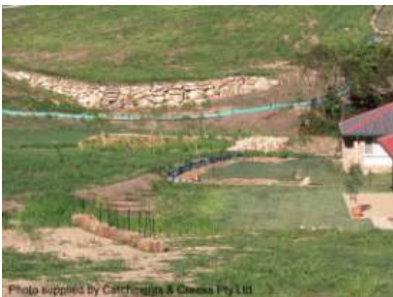
Straw bales diverting stormwater runoff
