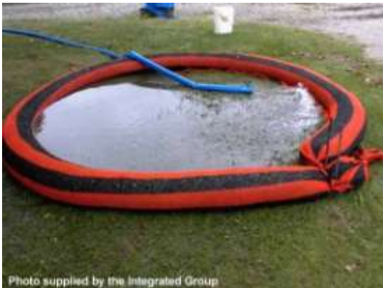
Compost-filled filter sock
