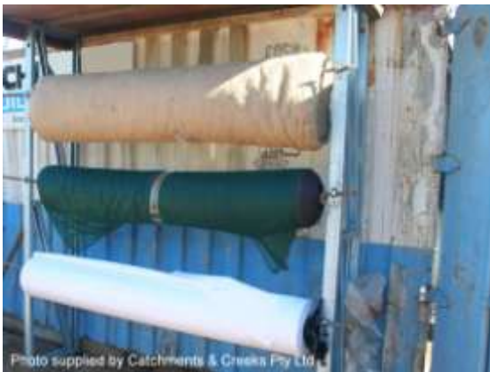
On-site stockpile of ESC fabrics
