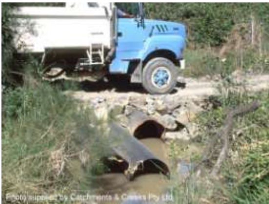
Temporary culvert crossing
