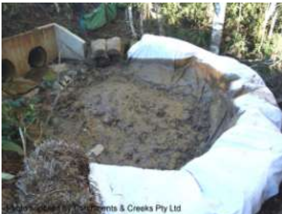
Straw bale sediment trap on a steep slope
