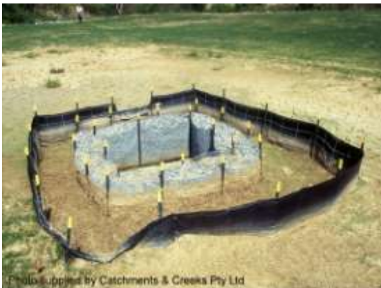
Sediment weir field inlet control
