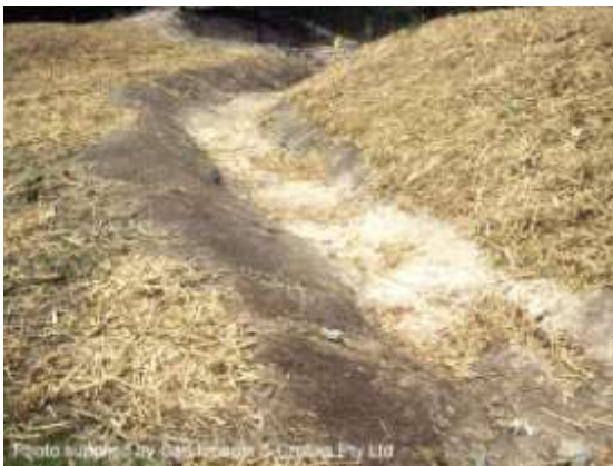
Loss of mulch by storm flows
