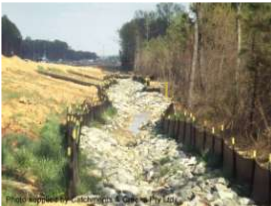
Protection of permanent storm drain
