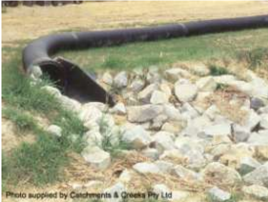
Diversion drain outlet structure
