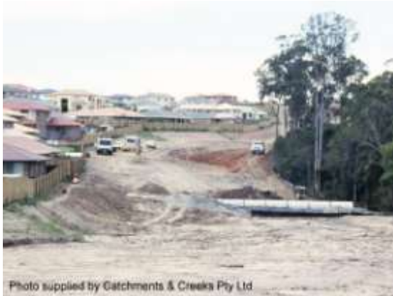
Early installation of stormwater pipe
