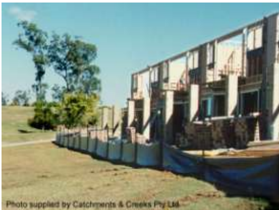
Sediment fence adjacent a building site
