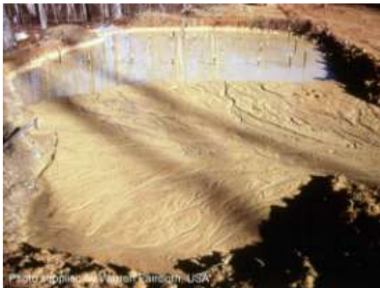
Sediment retained in a basin
