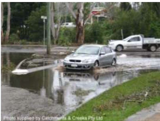
Flooded road surface
