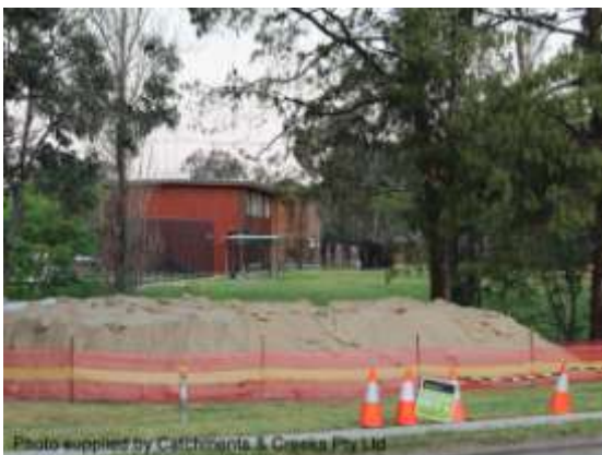
Stockpile covered with jute blankets
