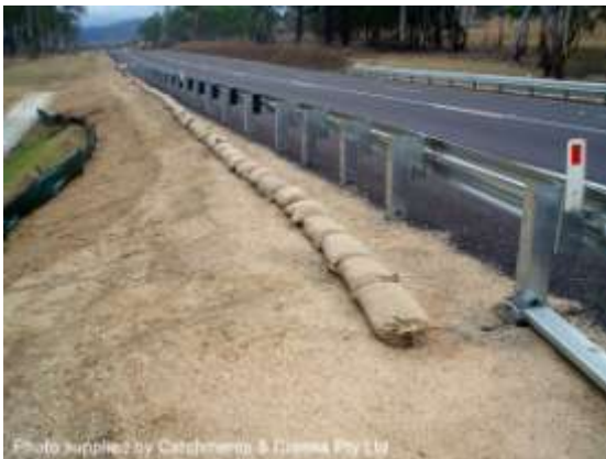
Road runoff diverted away from a slope
