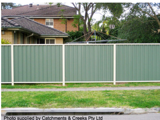
Raised fencing over an overland flow path
