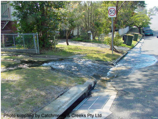
Failure of a water supply pipe
