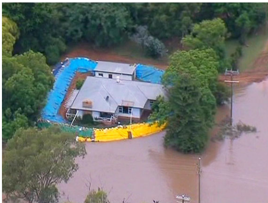
Temporary flood levee
