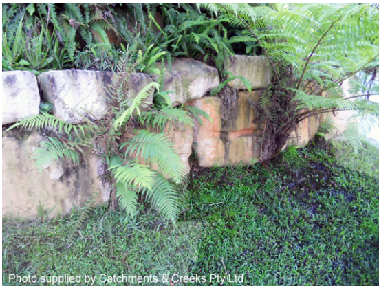
Groundwater weeping from retaining wall
