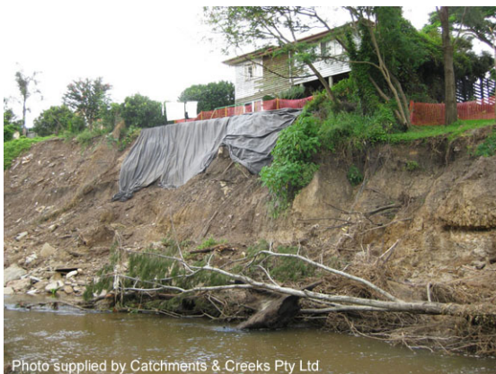
Creek bank failure
