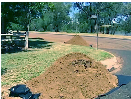
Roadside stormwater inlets covered
