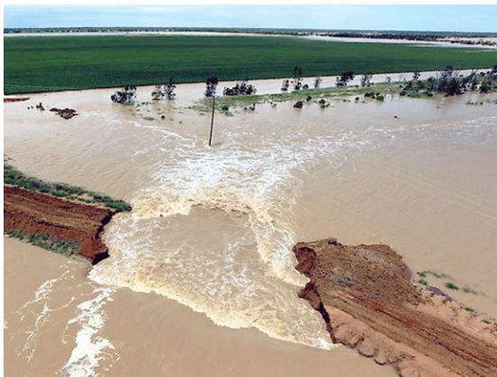
Failure of earth embankment
