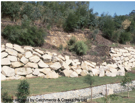
Failed rock retaining wall
