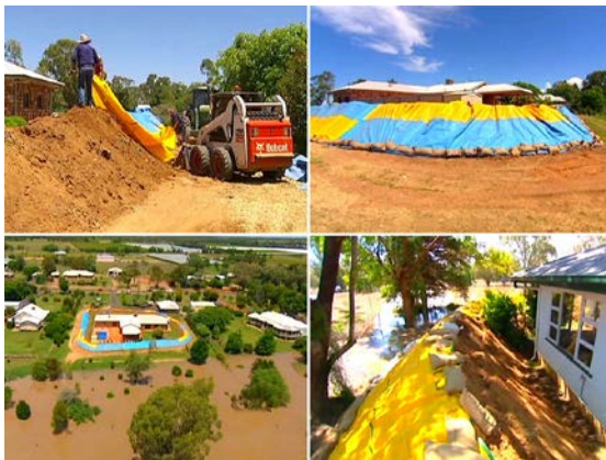
Construction of temporary flood levee
