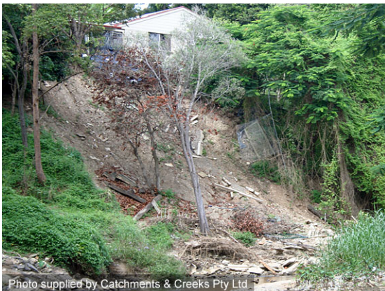
Bank erosion on outside of channel bend
