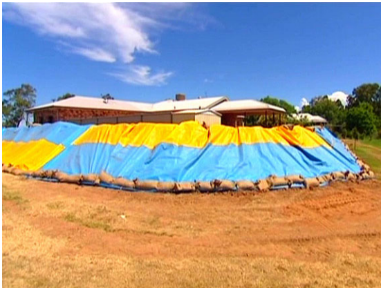
Anchorage of plastic sheeting
