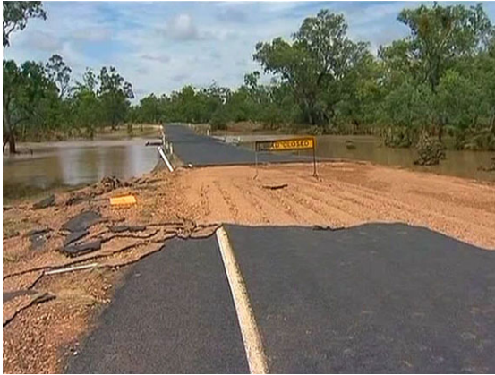
Asphalt lifted from roadway
