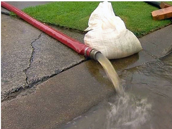
Pumping floodwaters from an enclosure
