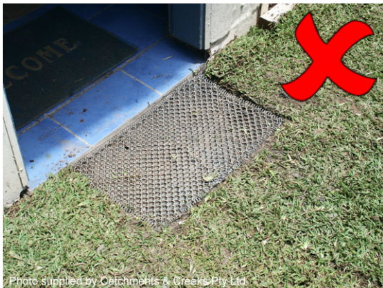
Floor level set below adjacent ground
