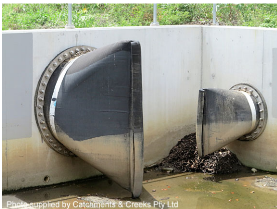
Rubber 'duckbill' backflow control
