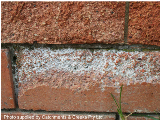
Salt damage to brickwork
