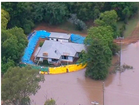
Temporary earth levee
