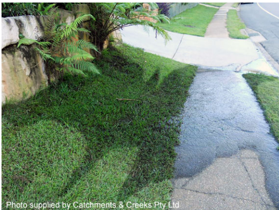
Groundwater seepage from a rock wall
