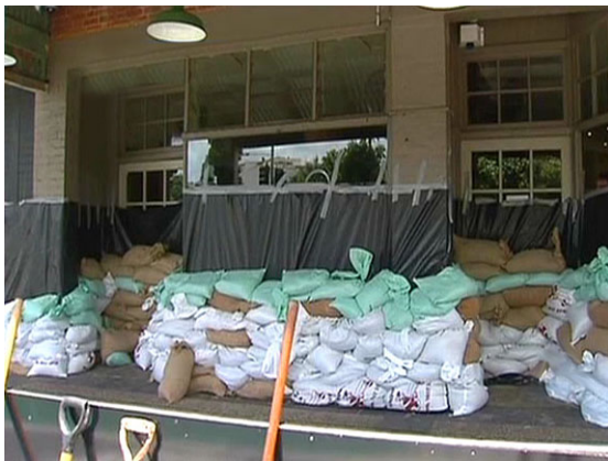
Flood-proofing of low-level building
