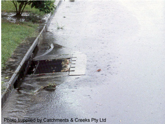
Photo supplied by Catchments & Creeks Pty Ltd Roadside kerb inlet to stormwater pipe
