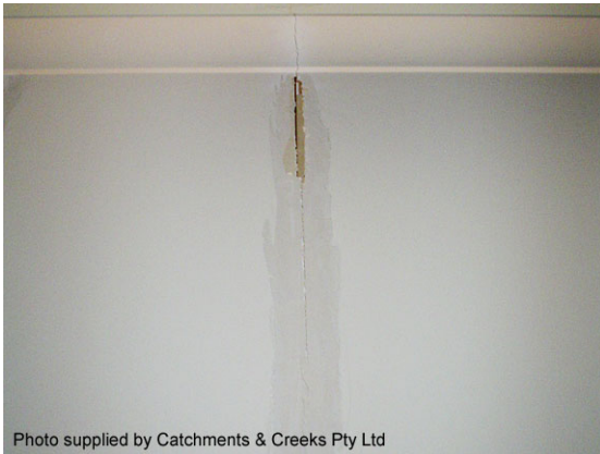
Wall cracking
