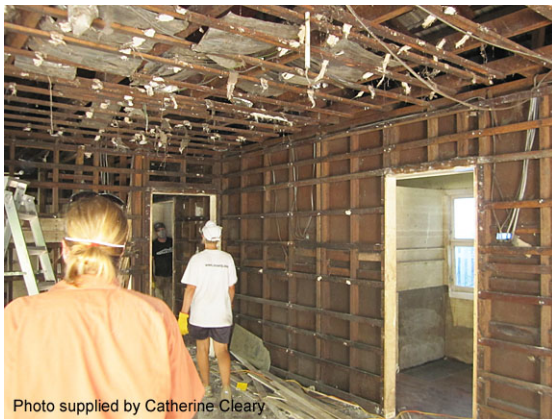
Removal of wall and roof cladding
