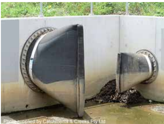
Rubber 'duckbill' backflow control
