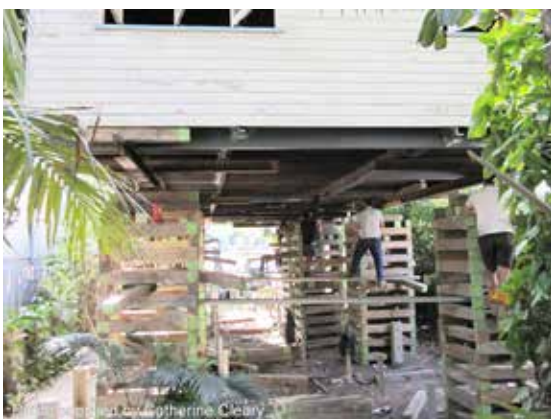
Raising a flood-prone house
