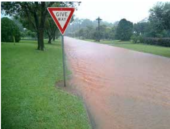
Flow along roadway during major storm
