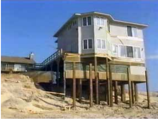
Elevated beach-front property
