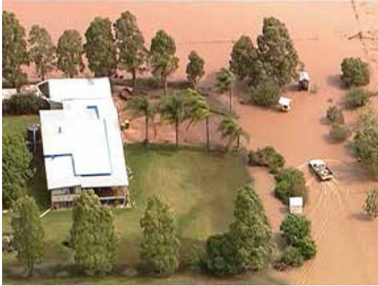
Building on elevated ground
