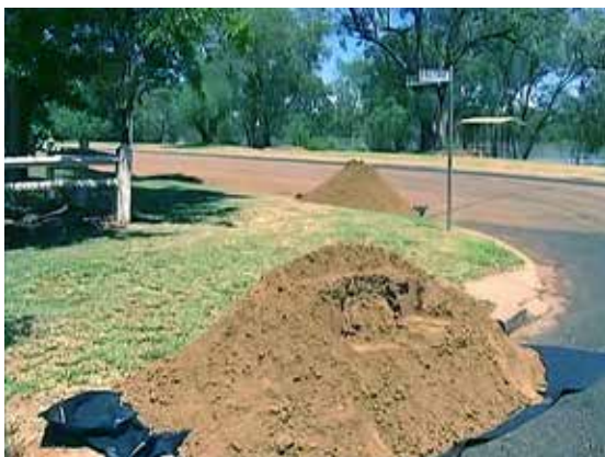
Roadside stormwater inlets covered
