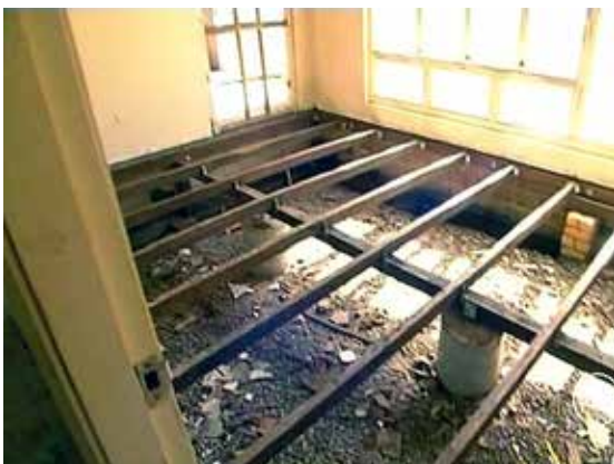
Removal of flooring
