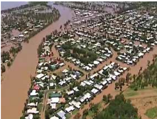
Floodwater backing up into the floodplain
