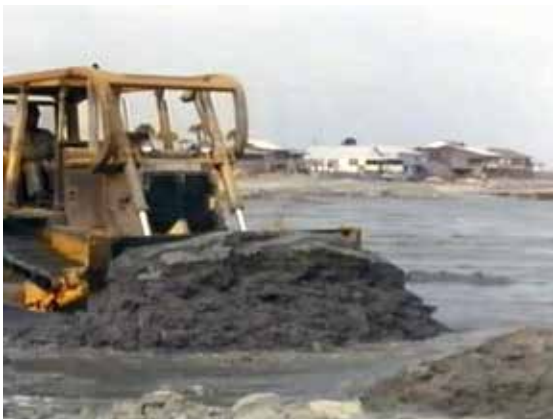
Reshaping of beachfront
