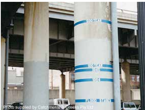
Historic flood marker
