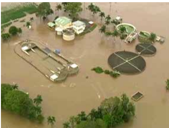
Flooded sewerage treatment plant
