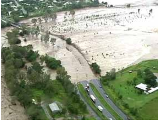
Flooded road crossing
