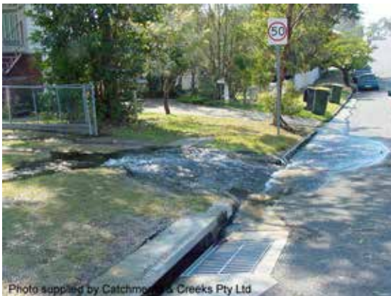
Failure of a water supply pipe
