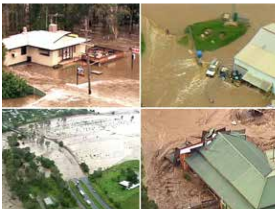
Flood and storm damage
