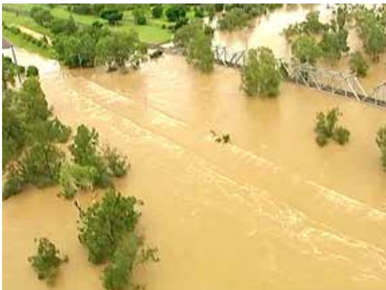
Flooding at Emerald, Queensland, 2011
