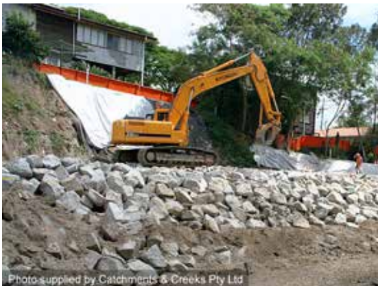
Bank stabilisation works
