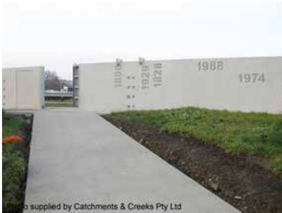
Flood control levee, Launceston
