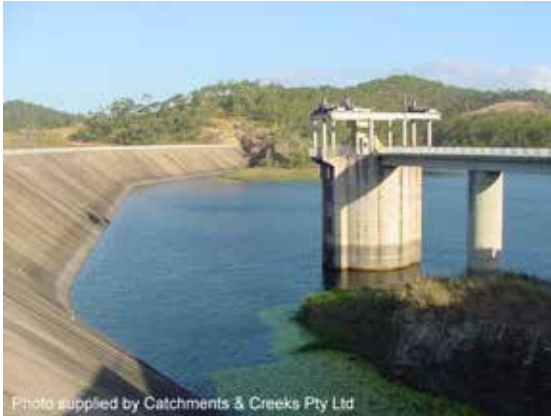
Water supply dam
