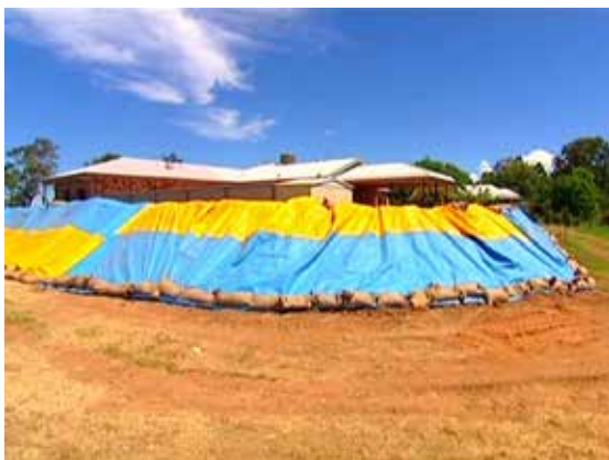
Anchorage of plastic sheeting
