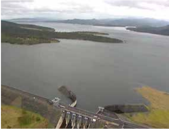
Flood control dam
