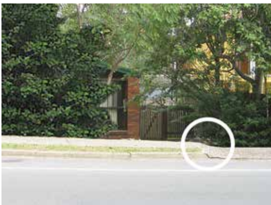
Driveway entry lowered below footpath
