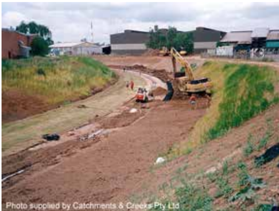
Channelisation of urban waterway
