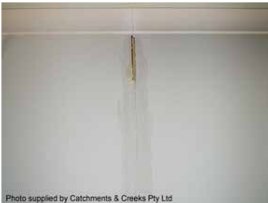
Wall cracking
