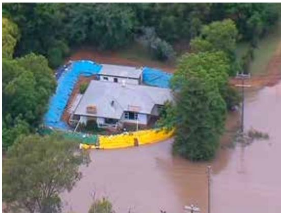
Temporary flood levee
