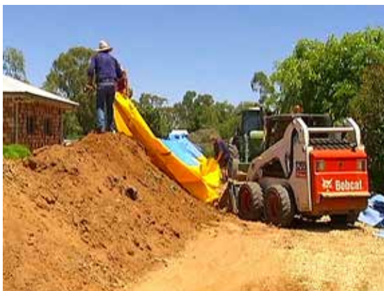
Preparation for imminent rural flooding
