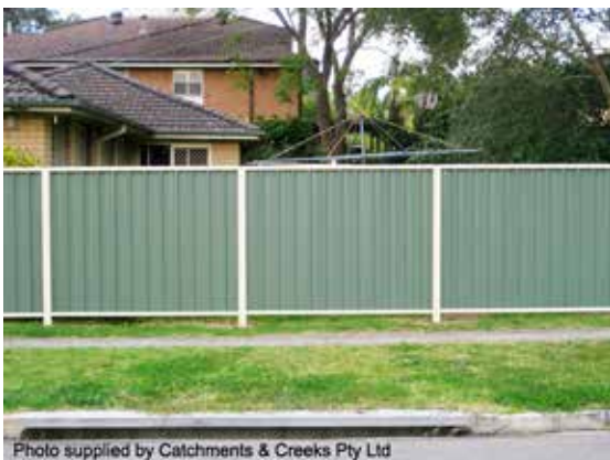
Raised fencing over an overland flow path
