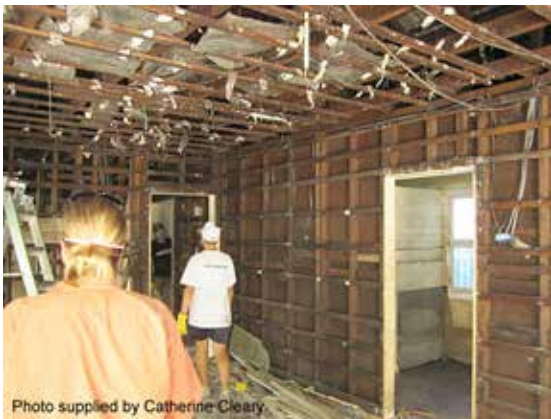
Removal of wall and roof cladding
