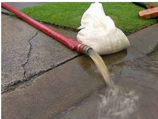
Pumping floodwaters from an enclosure
