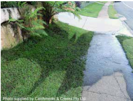
Groundwater seepage from a rock wall
