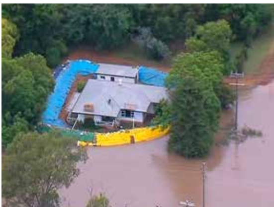
Temporary earth levee
