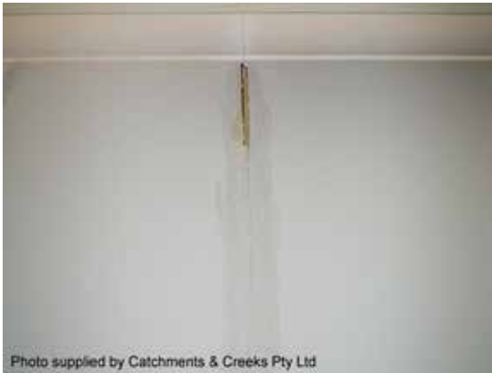
Wall cracking
