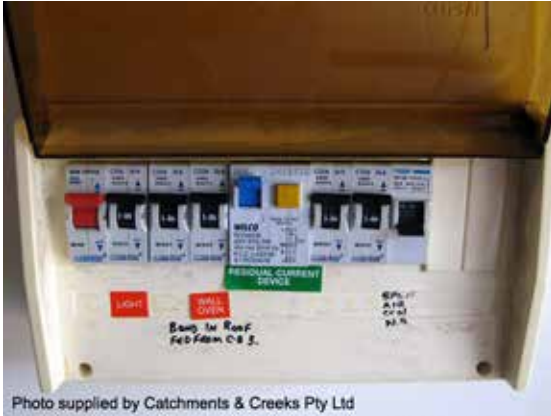
Circuit breaker electrical switchboard
