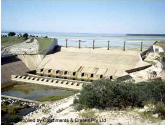
Storage dam without flood control gates
