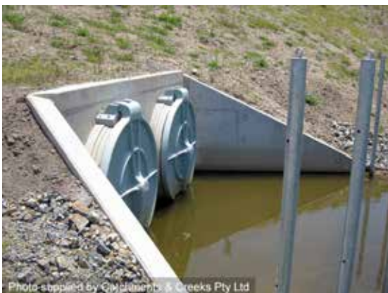
Backflow control gates
