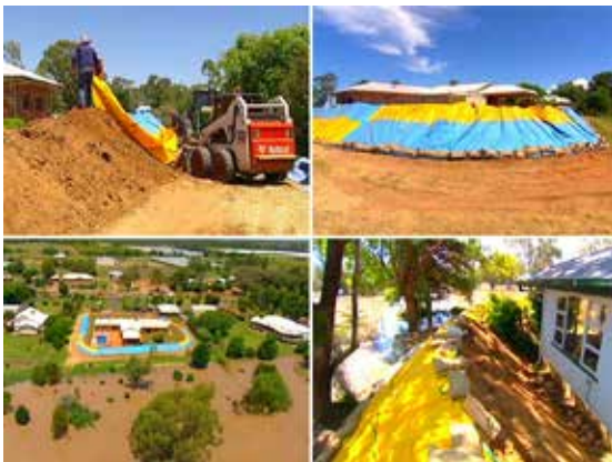
Construction of temporary flood levee
