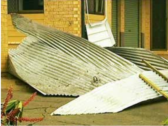
Displaced roofing material
